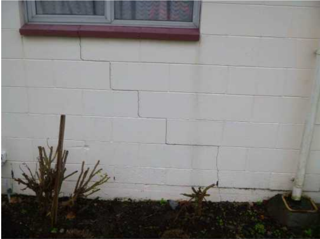
Photo 11: Back elevation of unit 6, step cracking of brick wall and foundation crack
