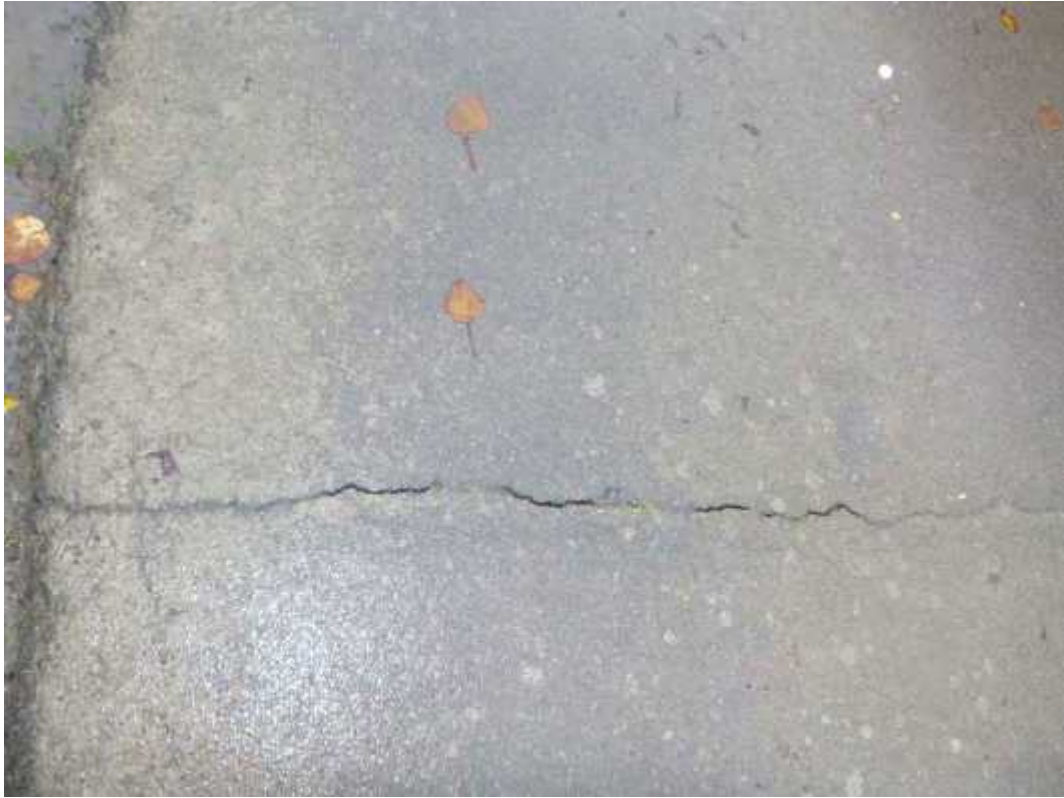
Photo 25: Pavement cracking on access road
