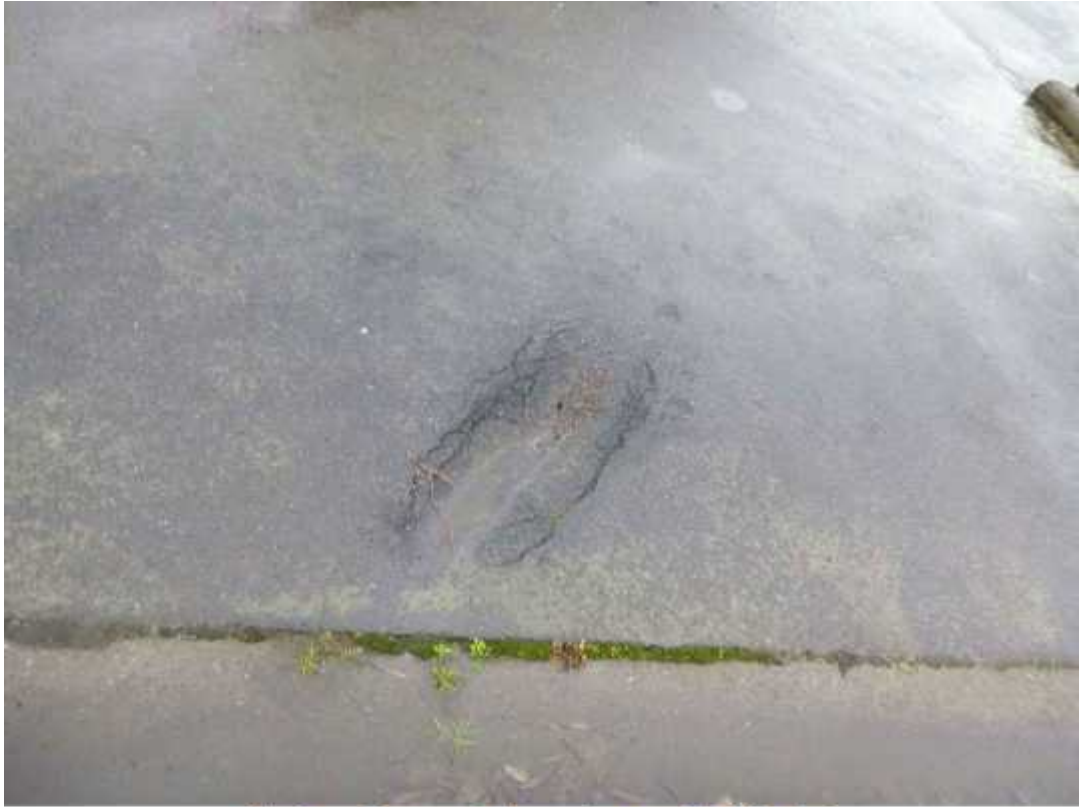
Photo 17: Pavement depression north of Block C
