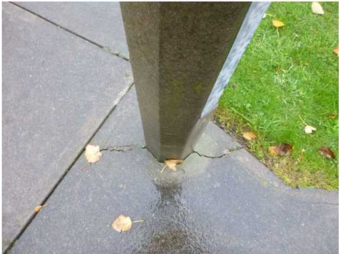
Photo 8: Crack at lamp post adjacent unit 1
