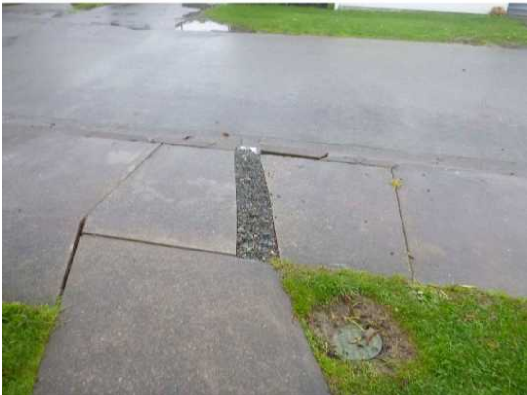
Photo 14: Separation of concrete path and curb damage
