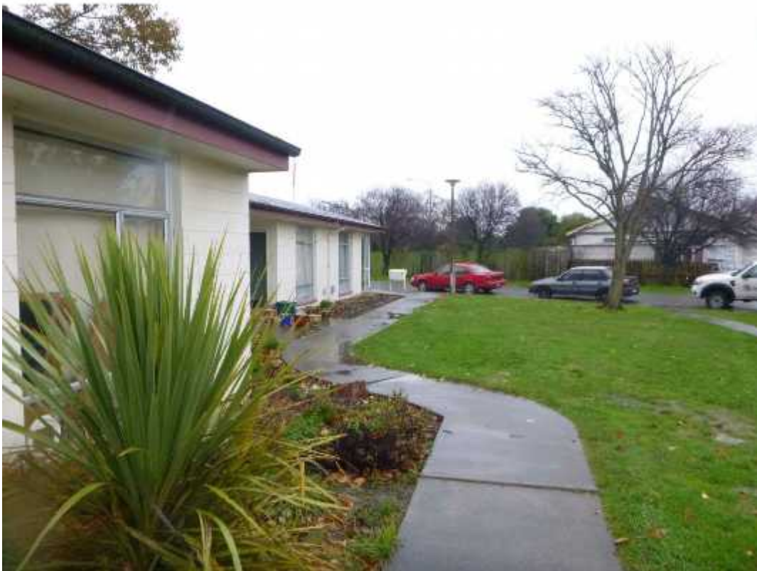
Photo 6: Front elevation of Block A, differential settlement of concrete path and liquefaction sand evident
