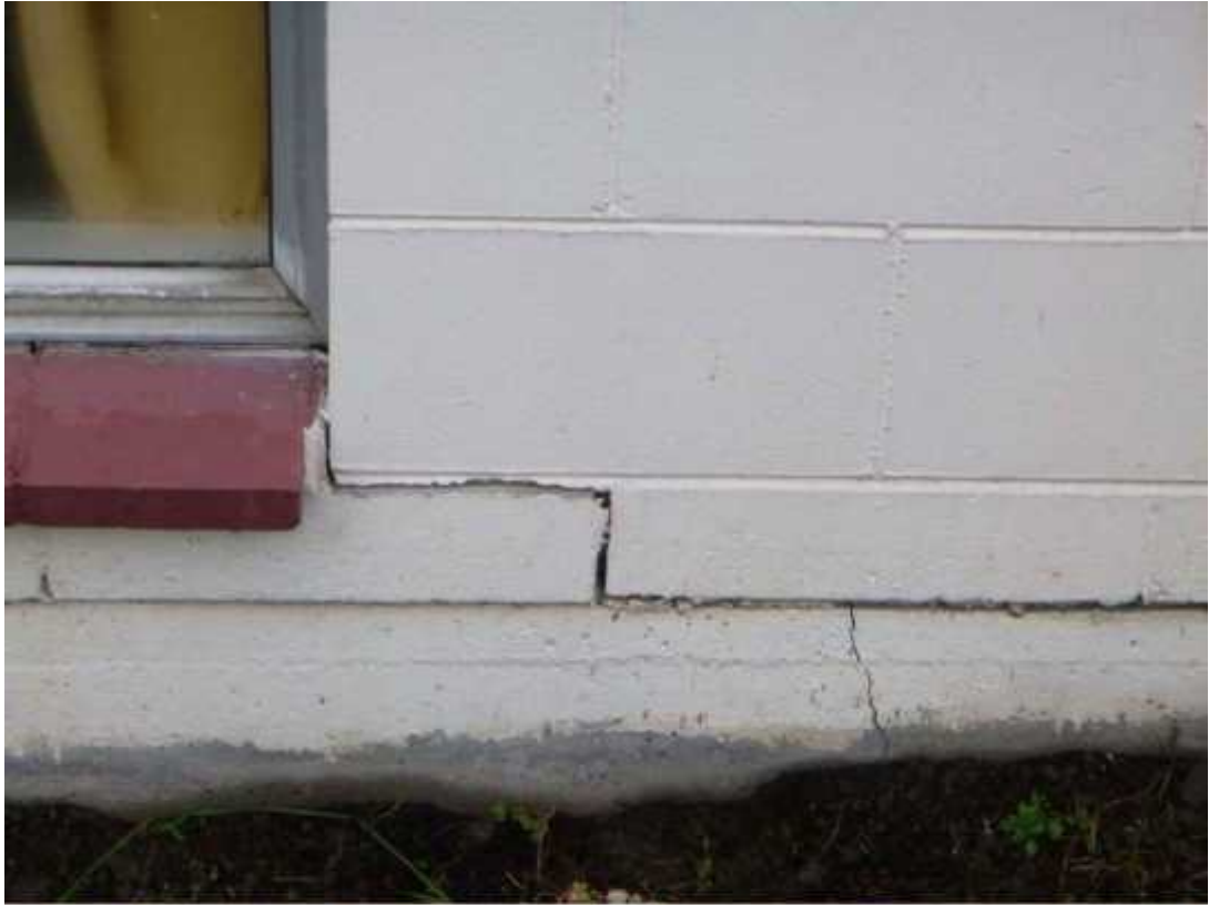
Photo 23: Cracking of brick veneer and foundation, north west corner beneath window of unit
