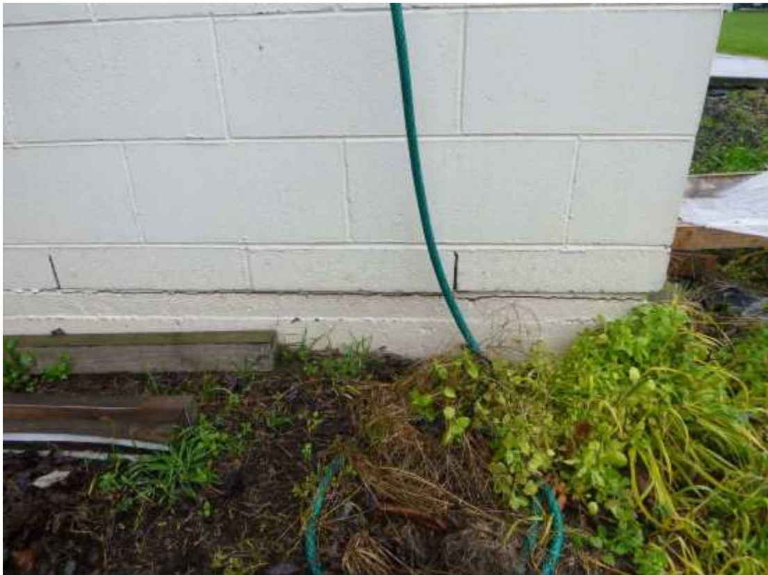
Photo 21: Cracking between brick veneer and foundation, north east corner of unit 19
