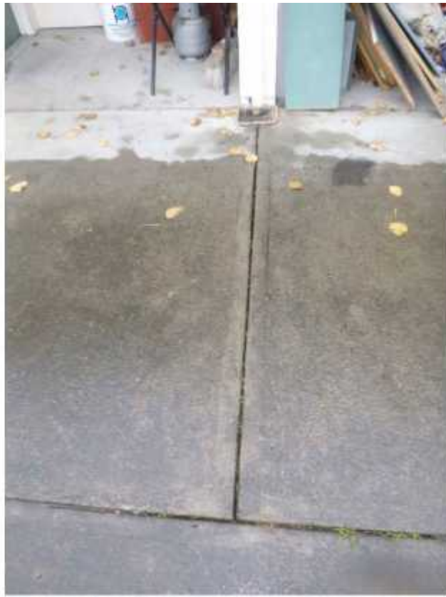
Photo 5: Spreading of concrete porch, up to 8mm
