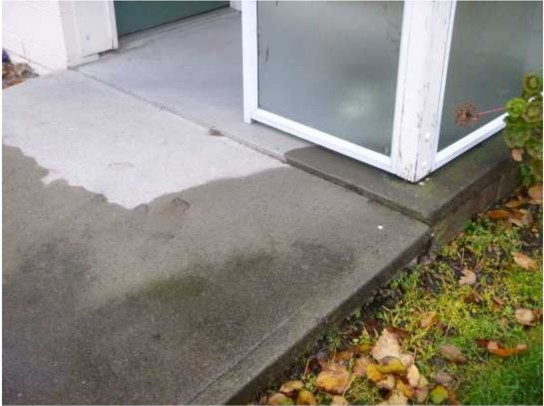
Photo 7: Front porch unit 1, differential settlement
