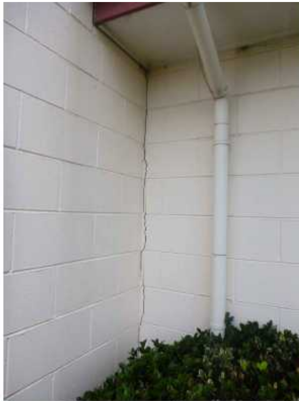
Photo 19: Brick veneer crack between unit 17 & 18
