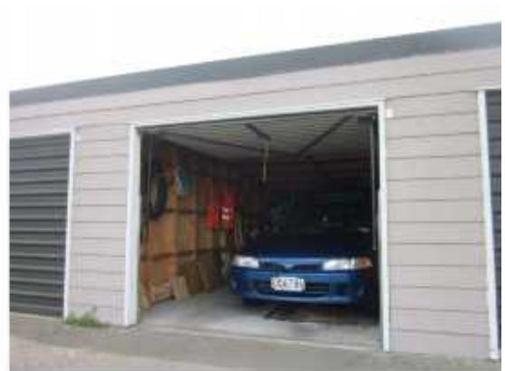
PHOTO 55: Block I – View into garage No 7.
