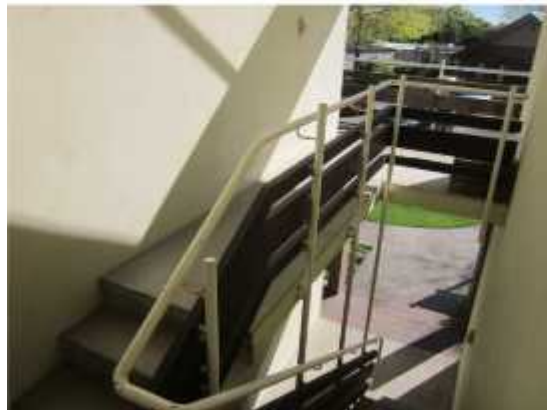
PHOTO 7: Block A – View at the concrete stair in the central part of the block – from half landing
