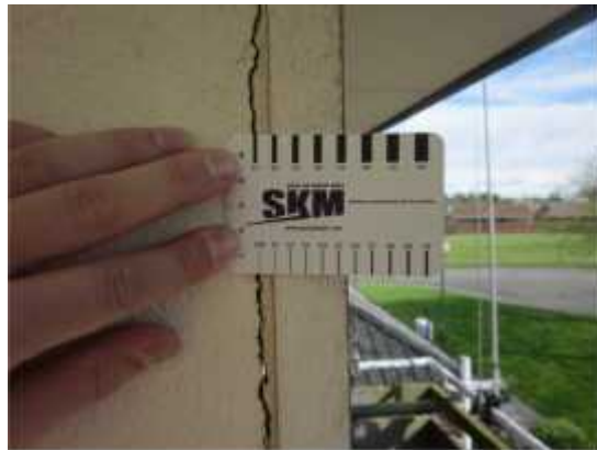
PHOTO 25: Block A – Detail of Photo 6. Timber planks separated from the end of the concrete wall.
