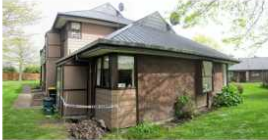
PHOTO 14: Block B – Exterior view of the property – side wing
