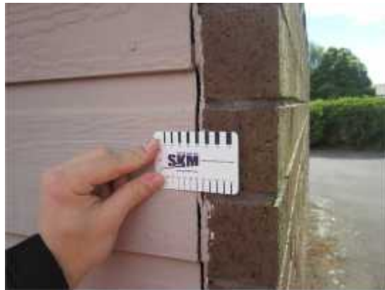
PHOTO 58: Block H - Gap has developed between weatherboards and brick veneer to the rear corner of Garage 1
