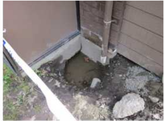
PHOTO 15: Detail of Photo 14 – view at concrete foundations (drainage repair works – not EQ related damage)
