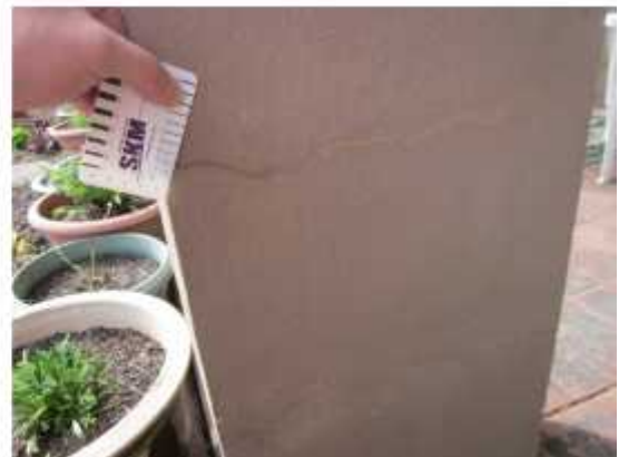
PHOTO 28: Block B – Hairline cracking in concrete column to the front elevation.
