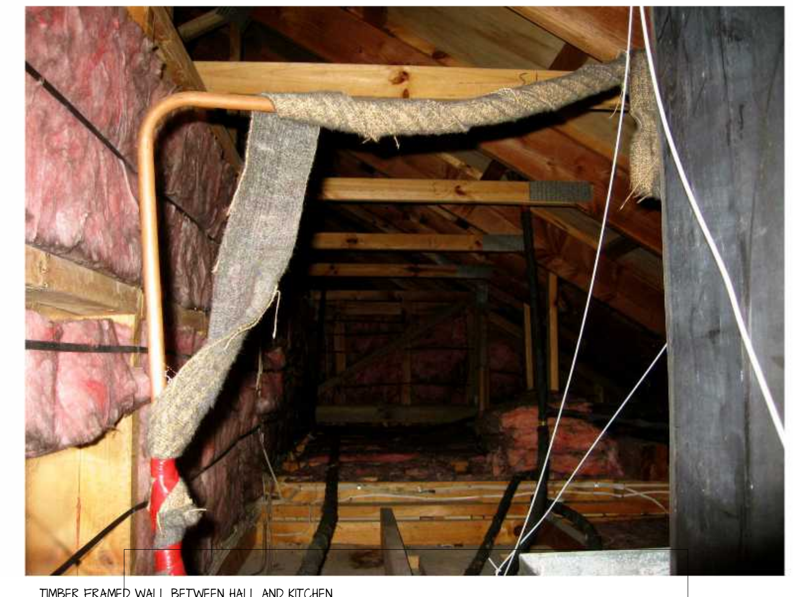
TIMBER FRAMED WALL BETWEEN HALL AND KITCHEN
