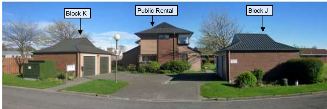
PHOTO 64: Blocks J & K (garages) – Exterior south-east view of the property.
