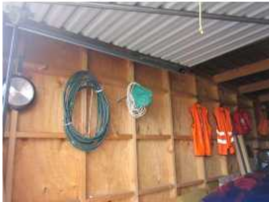
PHOTO 56: Block I – View into garage No 7.
