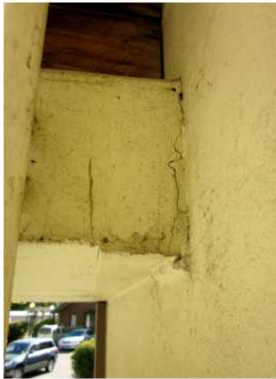
PHOTO 21: Block A - Hinge has developed at the angle support to slab to wall transition.
