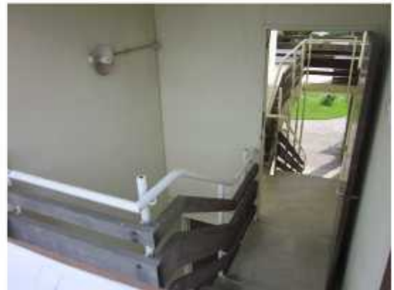
PHOTO 8: Block A – View at the concrete stair in the central part of the block – from rear balcony
