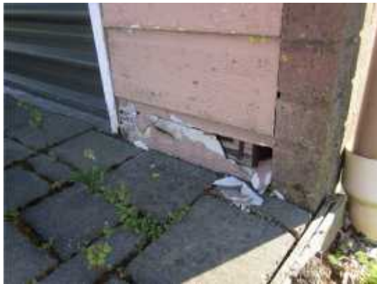
PHOTO 71: Block J - Weatherboard to the bottom of the front elevation is crushed and is spalling off
