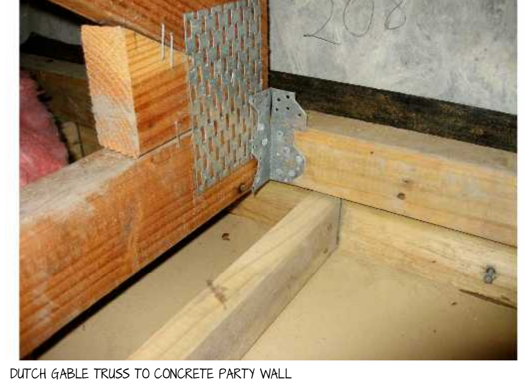
DUTCH GABLE TRUSS TO CONCRETE PARTY WALL
