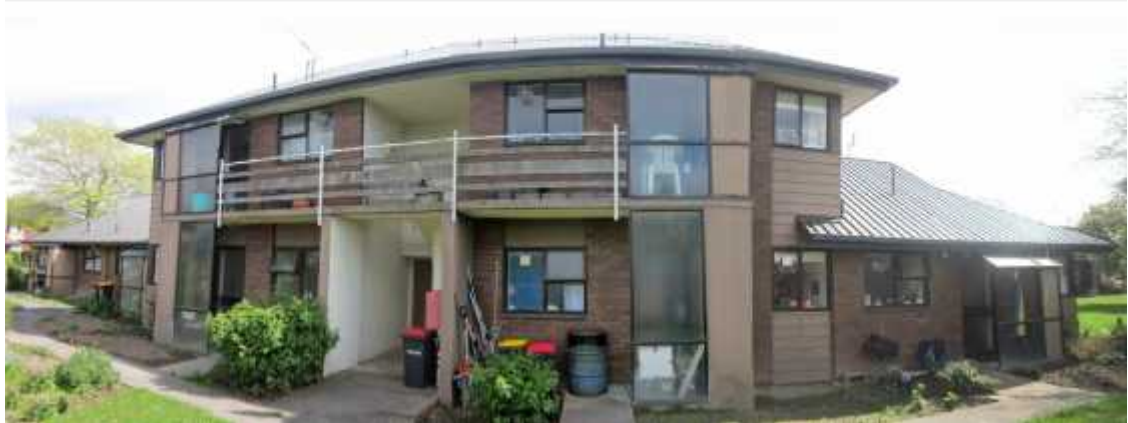
PHOTO 18: Block C – Exterior view of the property – rear
