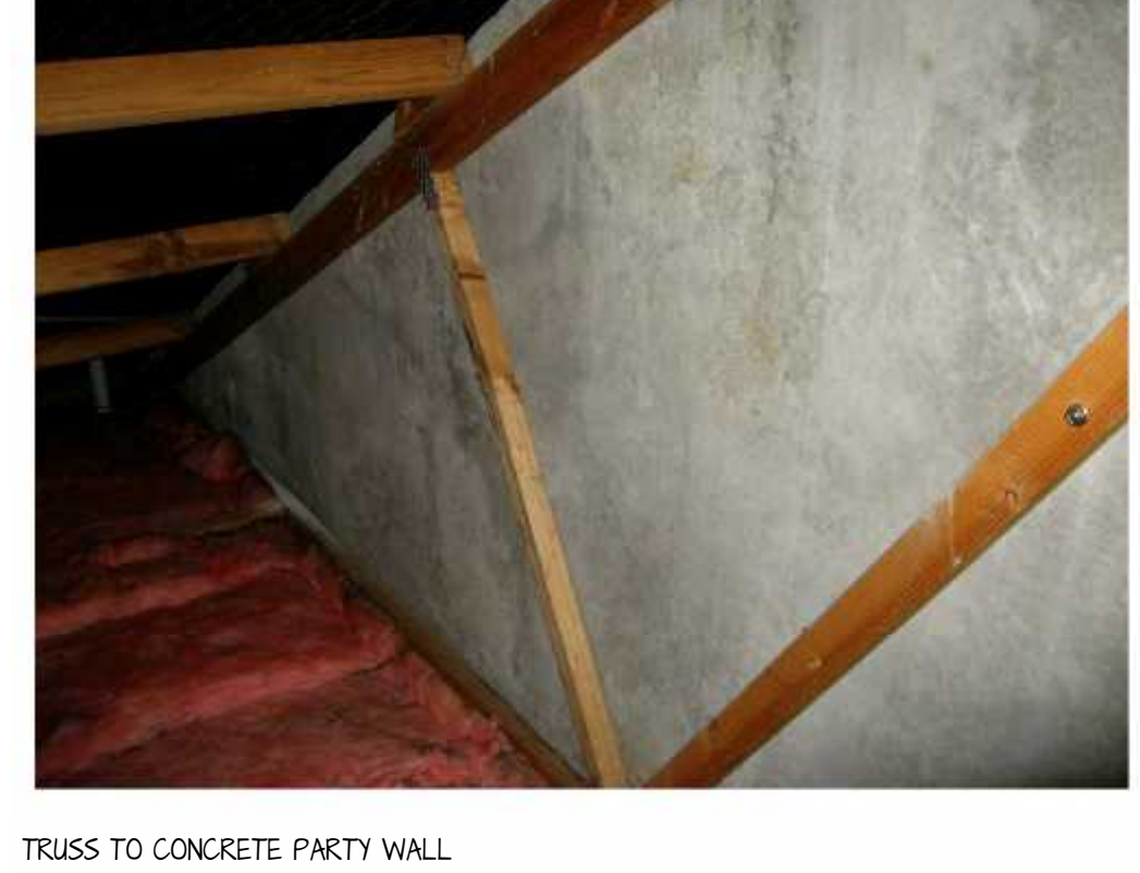
TRUSS TO CONCRETE PARTY WALL
