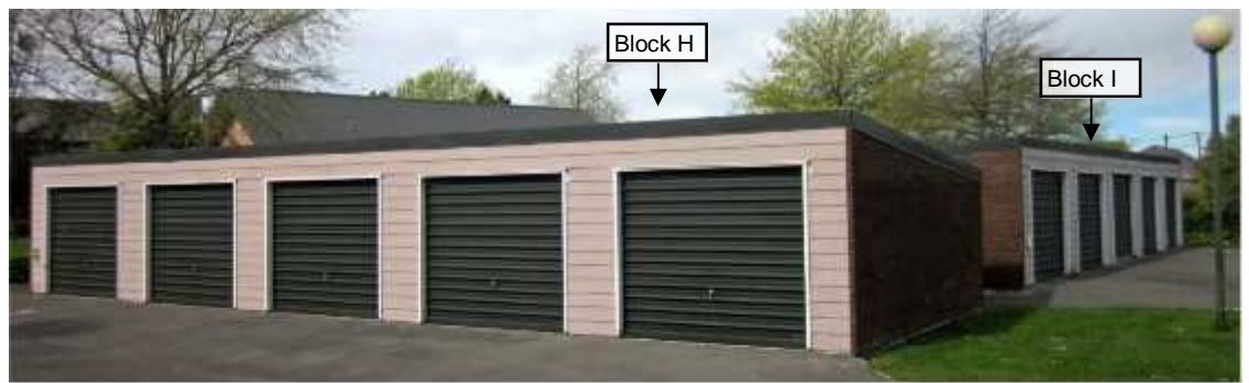
PHOTO 51: Blocks H & I (garages) – Exterior north view of the property.
