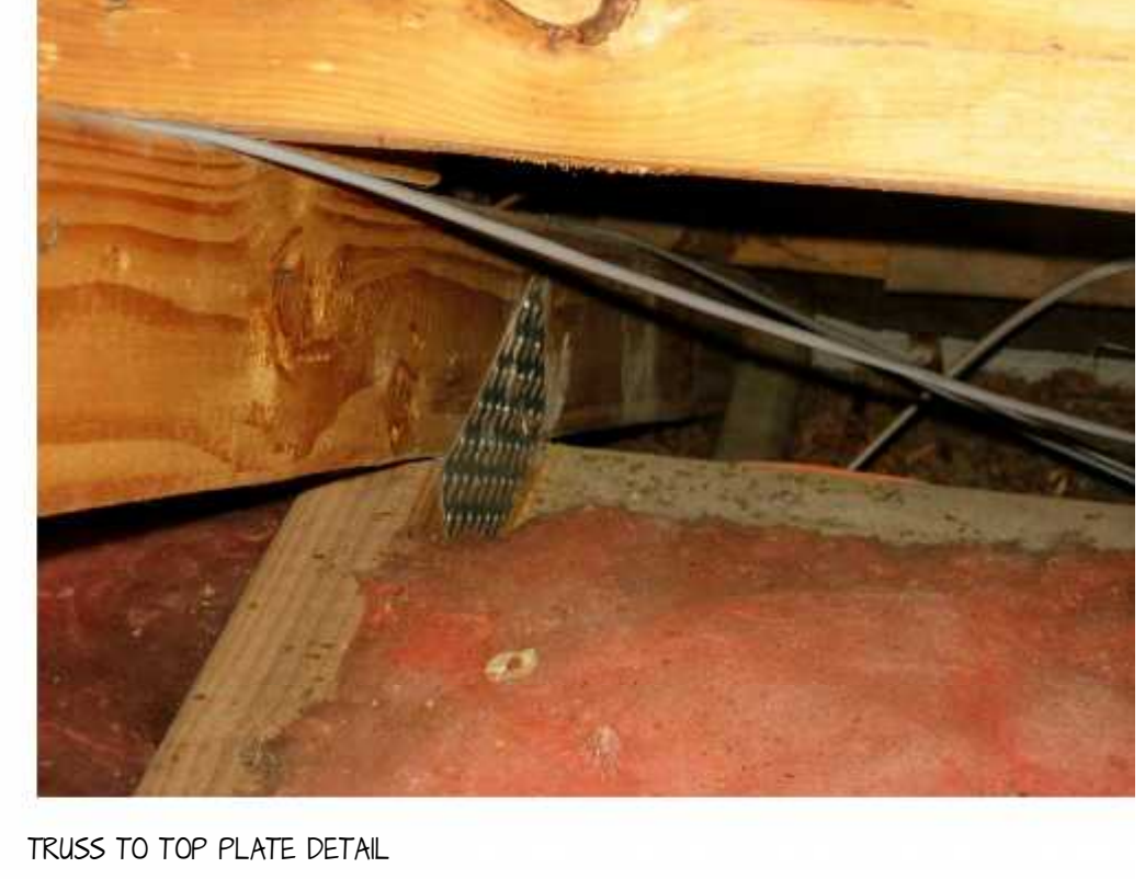
TRUSS TO TOP PLATE DETAIL
