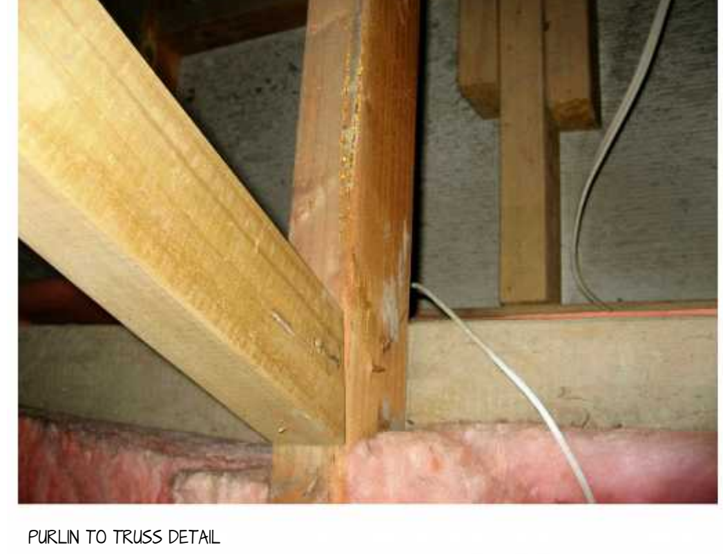
FURLIN TO TRUSS DETAIL
