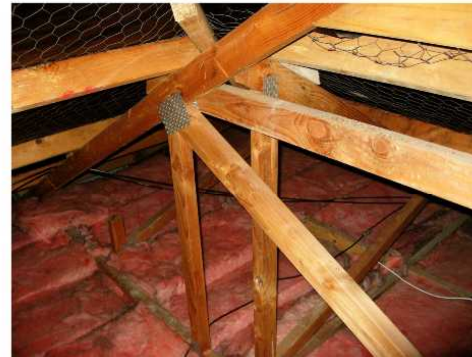
TRUSS CONNECTION AT DUTCH GABLE END
