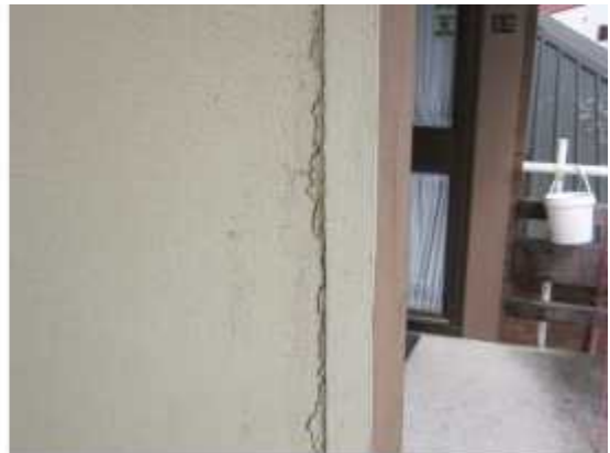
PHOTO 30: Block B – Timber planks separated from the end of the concrete wall.
