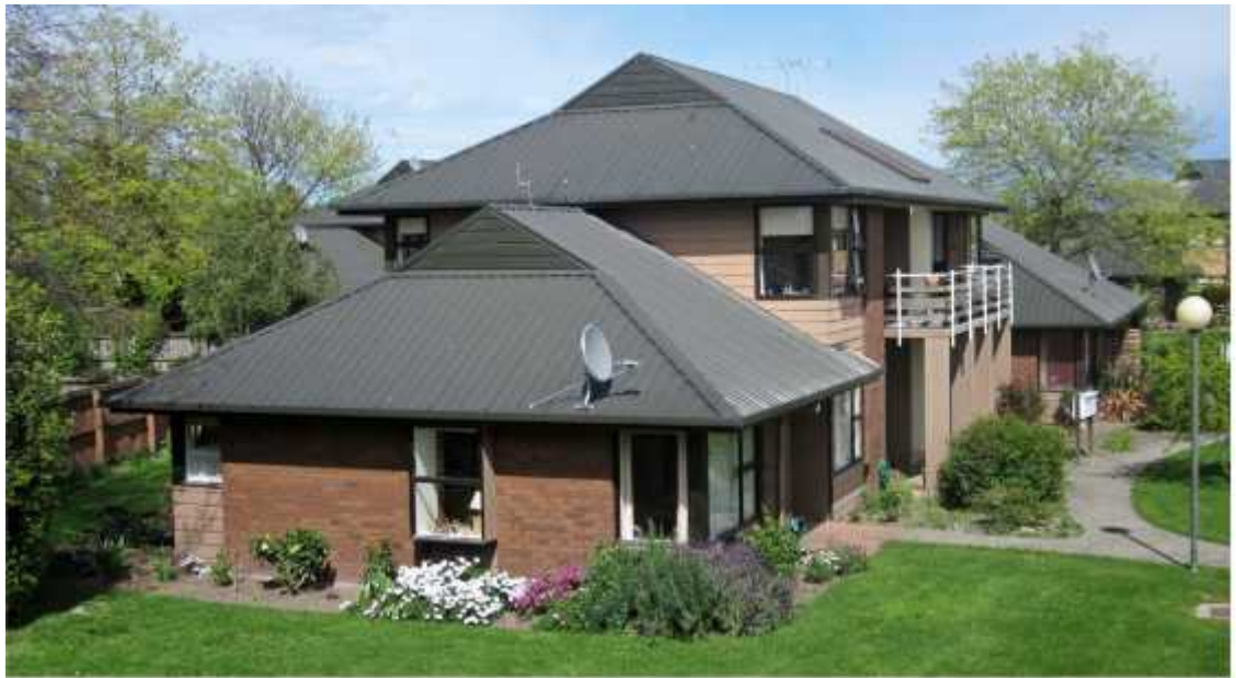
PHOTO 17: Block C – Exterior view of the property – side wing
