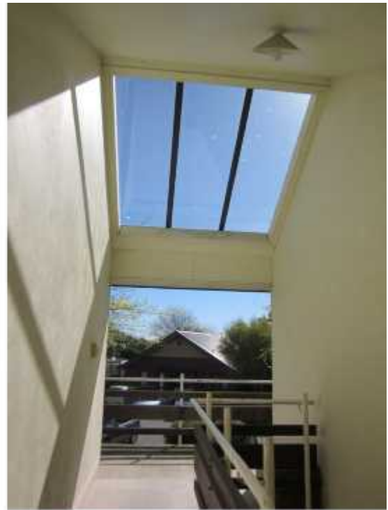
PHOTO 10: Block A – View at the skylight above the central stair
