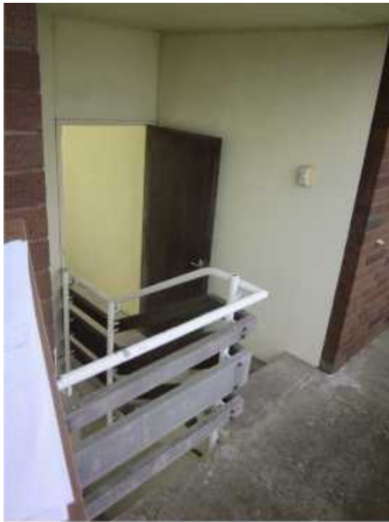
PHOTO 9: Block A – View at the concrete stair in the central part of the block – from rear balcony
