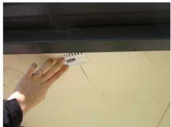
PHOTO 24: Block A - Cracking to lining to underside of the roof overhang
