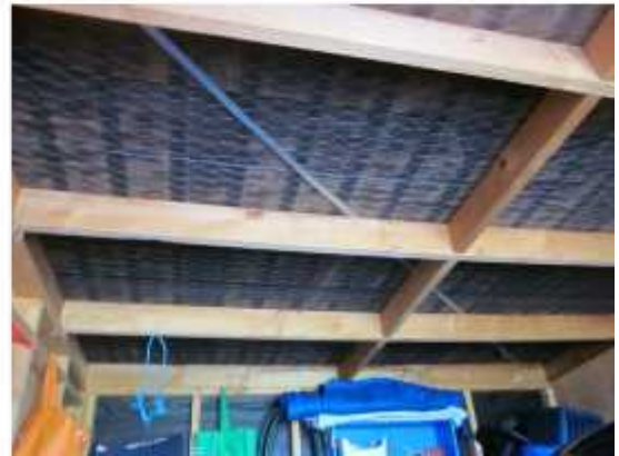
PHOTO 57: Block I – View into garage No 7.
