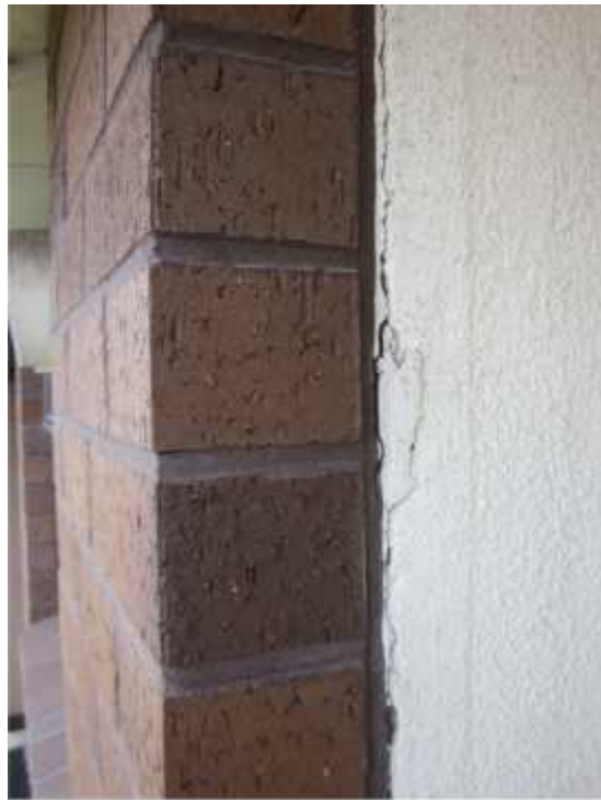
PHOTO 33: Block C - Brick veneer separated from the concrete wall - rear of the building upstairs
