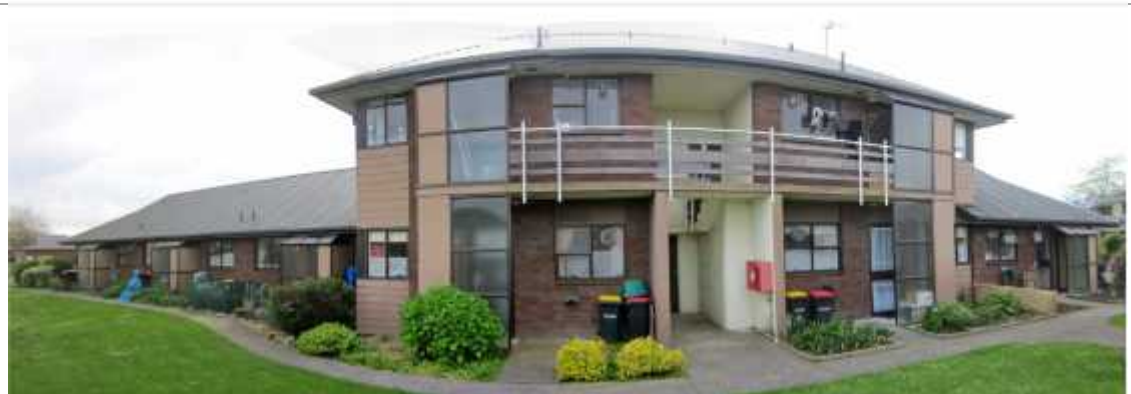
PHOTO 4: Block A – Exterior view of the property - rear
