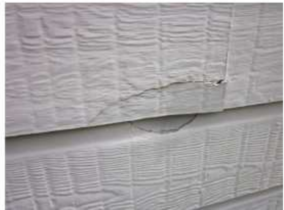
PHOTO 61: Block I – Weatherboard ruptured on the rear elevation.
