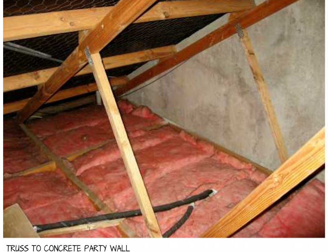
TRUSS TO CONCRETE PARTY WALL
