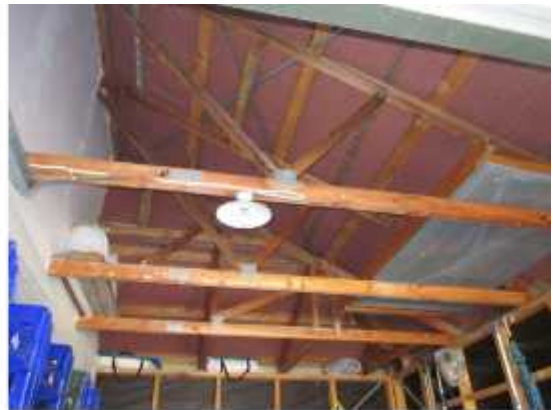
PHOTO 68: Block J – Interior view of the property (roof trusses and bracing).
