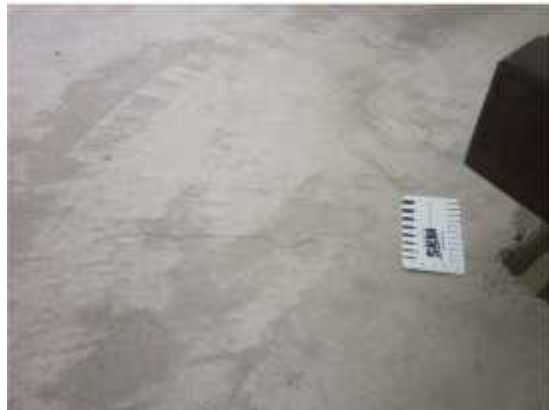
PHOTO 35: Block D – Detail of Photo 34.
