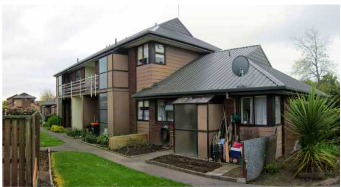
PHOTO 3: Block A – Exterior view of the property - rear
