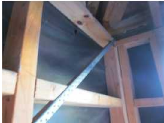
PHOTO 69: Block J – Interior view of the property (wall bracing – angle brace).
