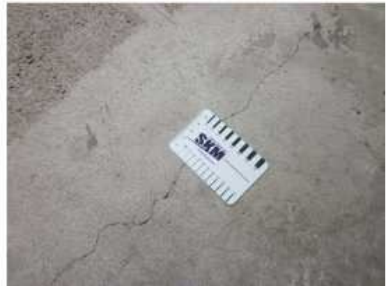
PHOTO 36: Block D – Detail of Photo 34.
