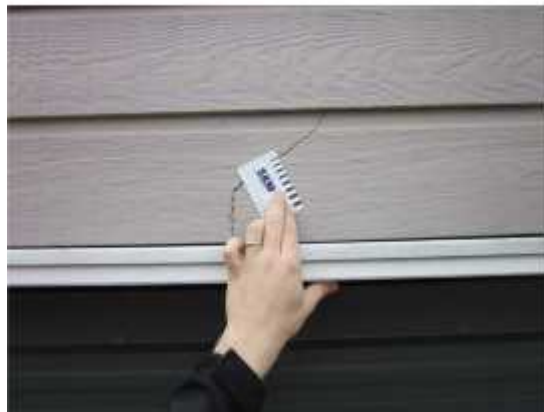
PHOTO 60: Block I – Weatherboard cracked on the front elevation.
