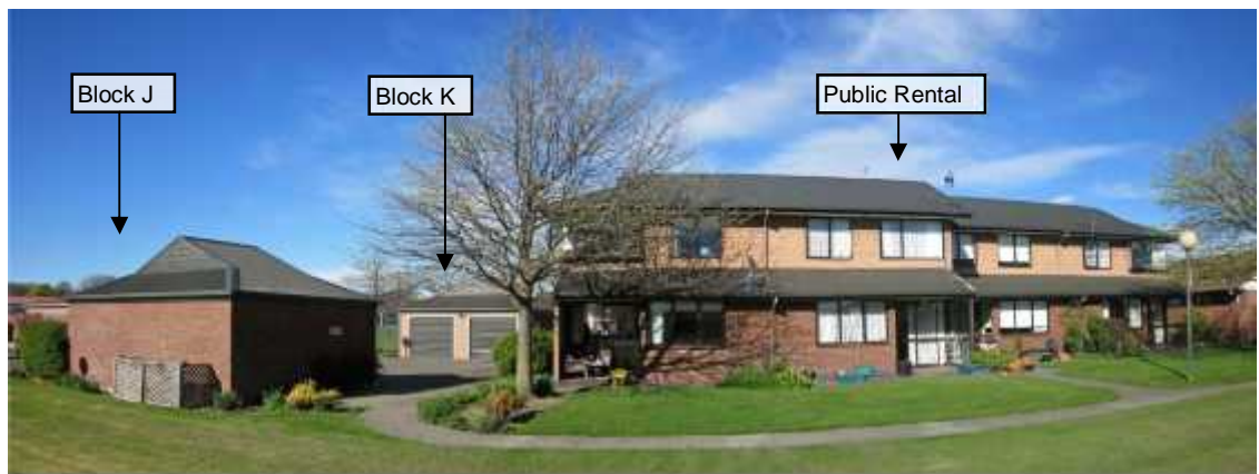
PHOTO 37: Public Rental (to the right) – Exterior north-east view of the property. Blocks J & K (garages) to the left
