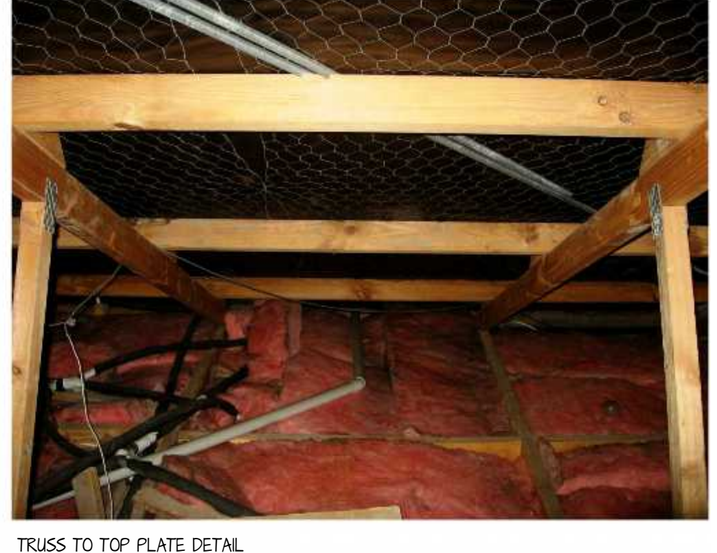
TRUSS TO TOP PLATE DETAIL
