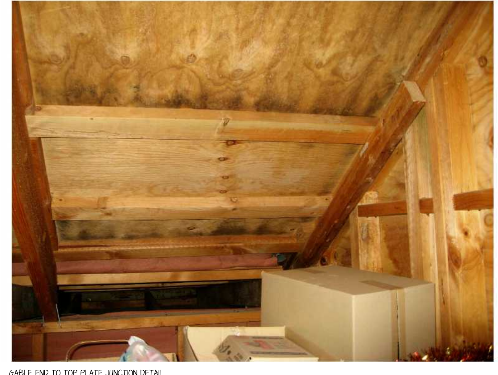
GABLE END TO TOP PLATE JUNCTION DETAIL
