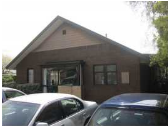
PHOTO 45: Resident's Lounge – Exterior south view of the property (gable).
