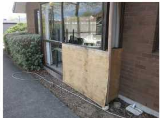
PHOTO 50: Resident's Lounge – Broken glazing (south-west gable).
