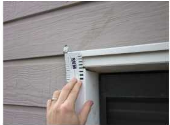
PHOTO 63: Block I – Garage door frame ruptured in corners.
