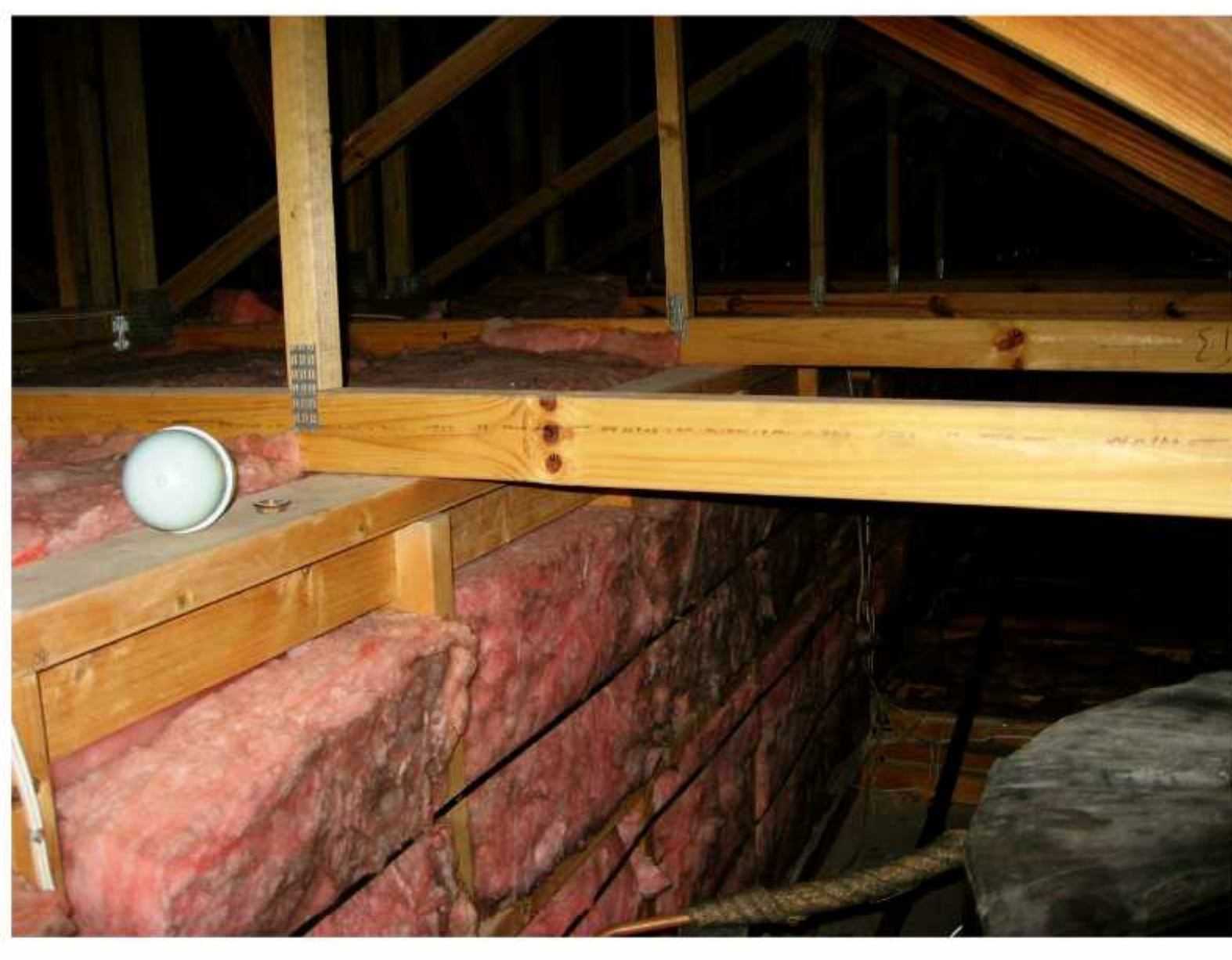
TRUSS TO INTERNAL WALL BETWEEN HALL AND KITCHEN
