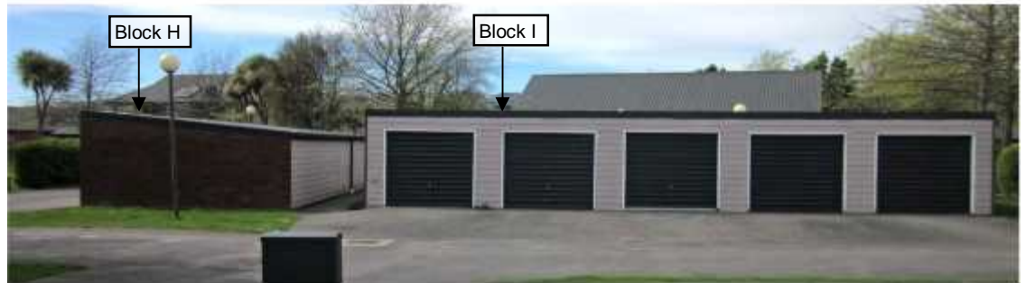
PHOTO 52: Blocks H & I (garages) – Exterior west view of the property.
