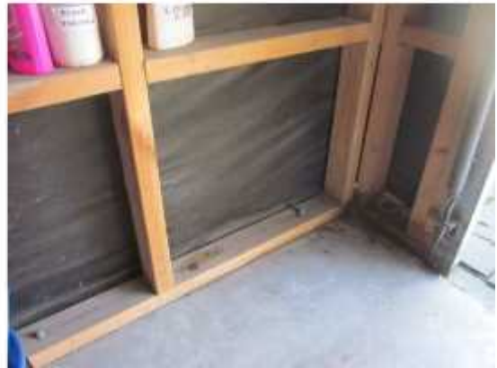
PHOTO 70: Block J – Interior view of the property (wall bracing – angle brace).
