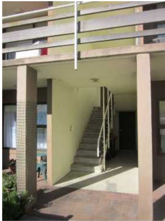
PHOTO 5: Block A – View at the concrete stair in the central part of the block - front
