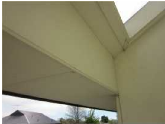
PHOTO 29: Block B – Cracking in ceiling panels to the underside of the skylight
