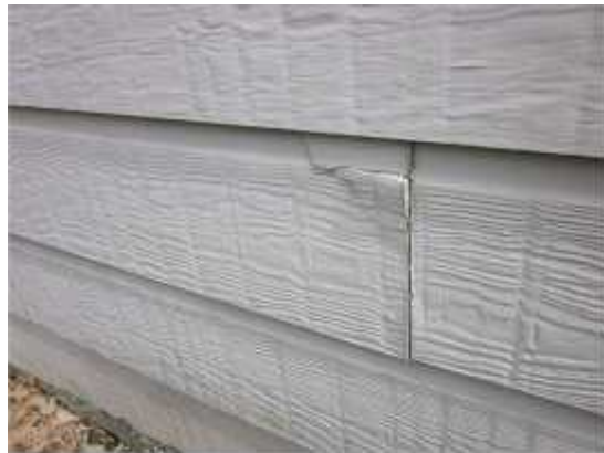
PHOTO 62: Block I – Weatherboard ruptured on the rear elevation.
