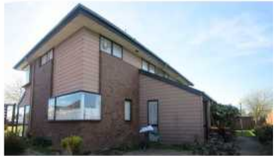
PHOTO 40: Public Rental – Exterior east view of the property.
