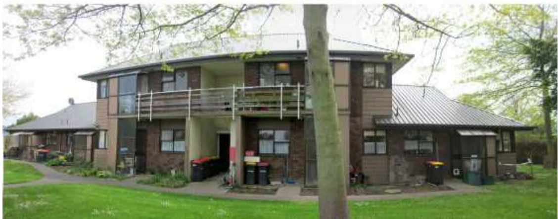
PHOTO 13: Block B – Exterior view of the property - rear
