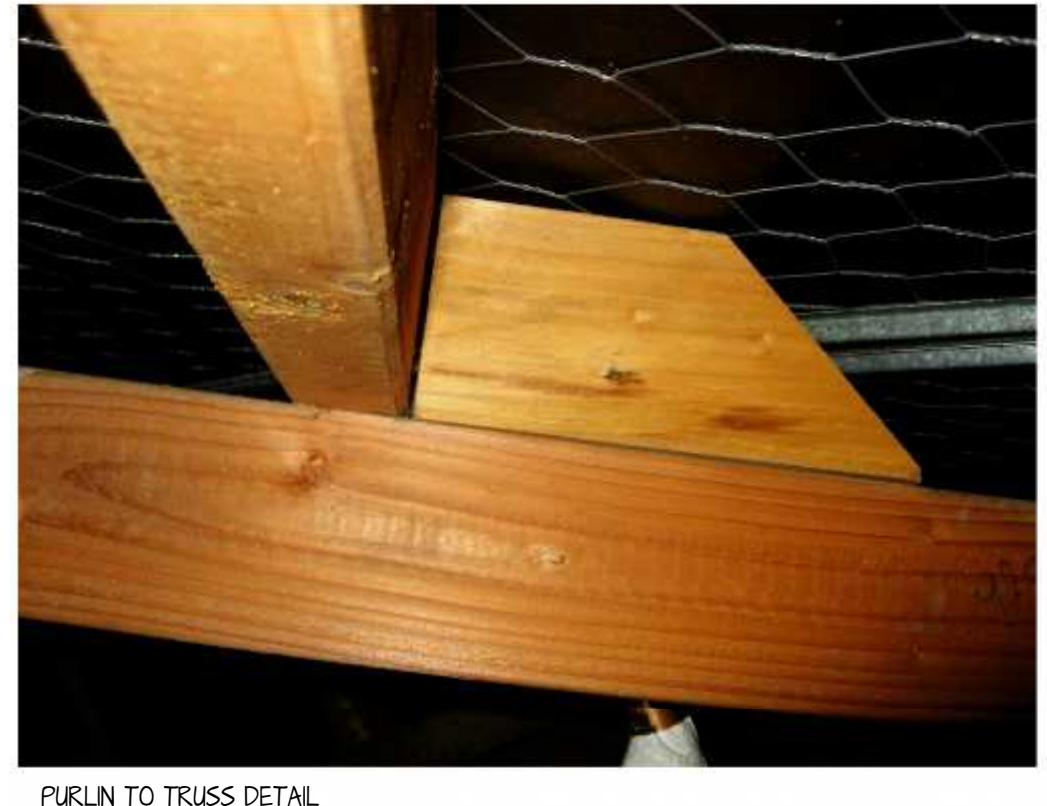
FURLIN TO TRUSS DETAIL
