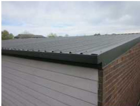
PHOTO 54: Block H – typical view at roof.
