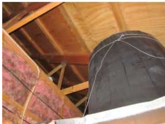
PHOTO 49: Resident's Lounge – View into roof space.
