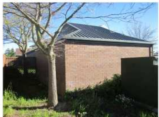
PHOTO 66: Block K - Exterior south view of the property.
