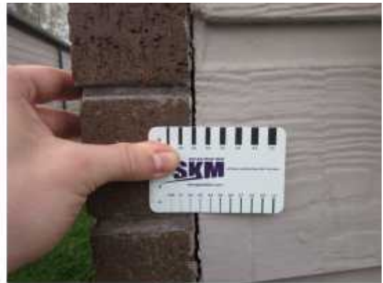
PHOTO 59: Block I - Gap has developed between weatherboards and brick veneer to the front corner of Garage 6
