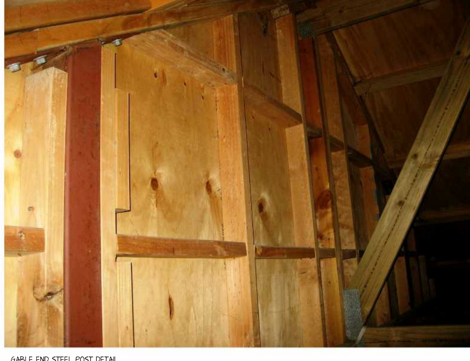
GABLE END STEEL POST DETAIL
