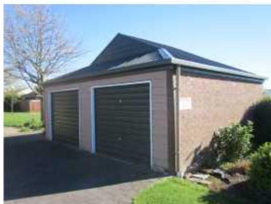
PHOTO 65: Block J - Exterior south view of the property.
