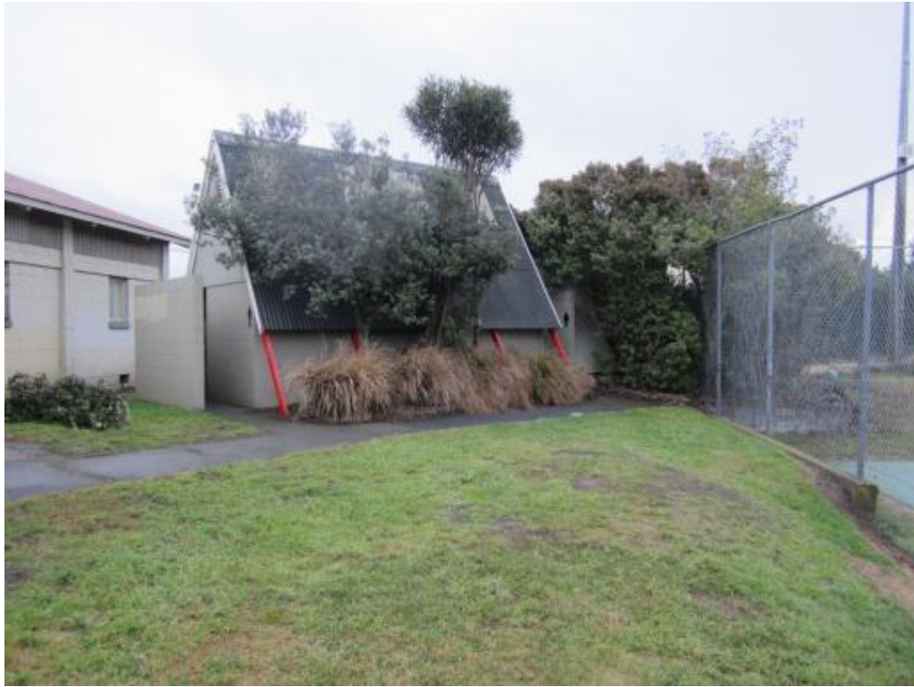
Photo 1. View of toilets from the east.
