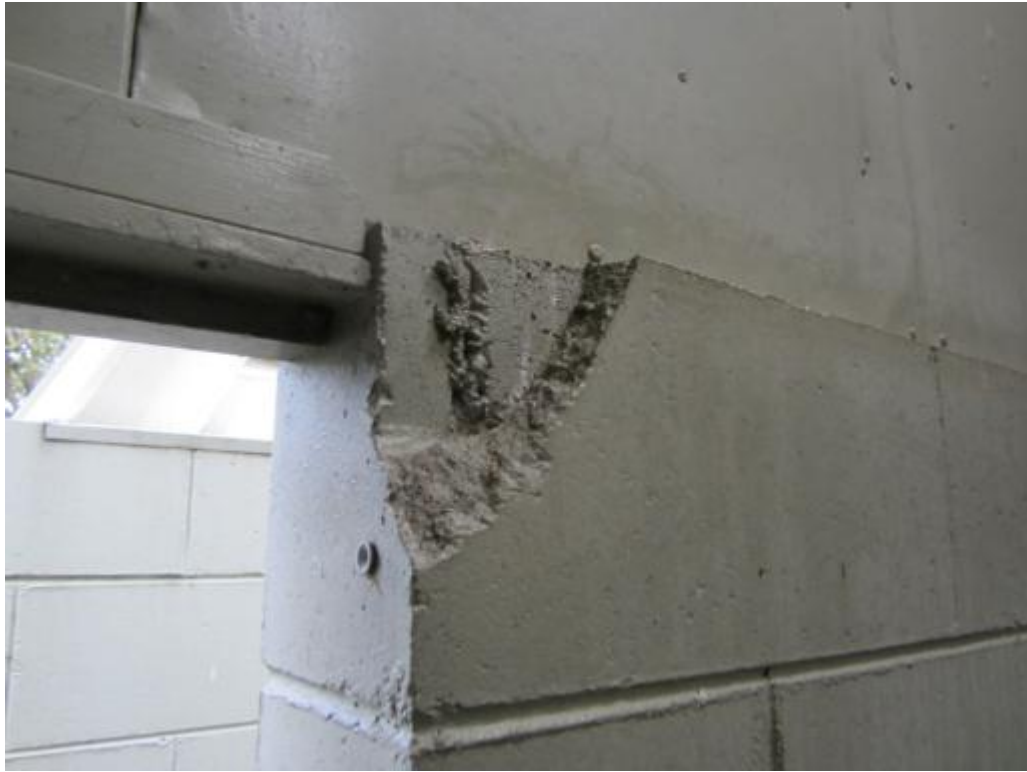
Photo 3. Broken block corner exposing concrete of bond beam within.
