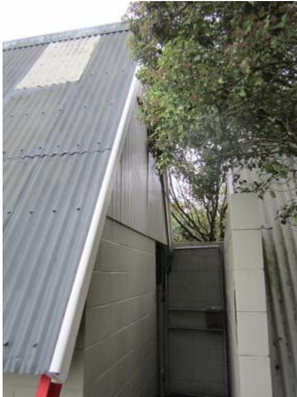
Photo 2. Gable and entrance wing walls.
