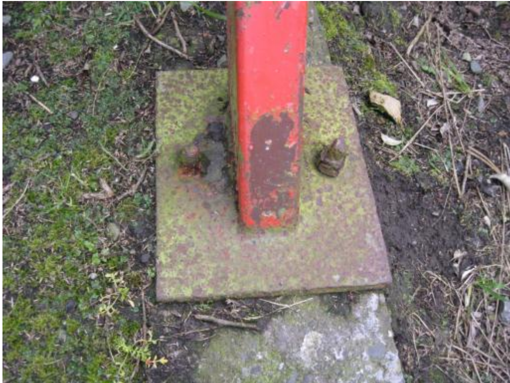
Photo 6. Excessive corrosion of base-plate bolts.
