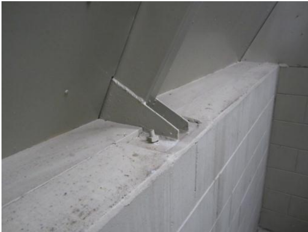
Photo 4. A-frame connection to bond beam.
