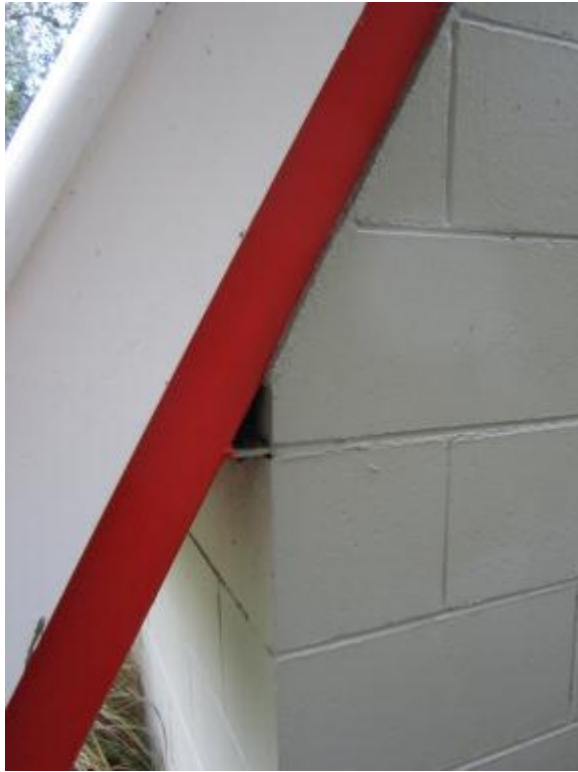
Photo 7. RHS framing gable wall at corner of building.
