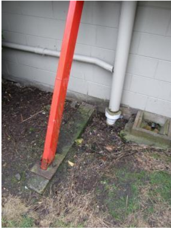
Photo 5. A-frame RHS supported on tip of ground beam.
