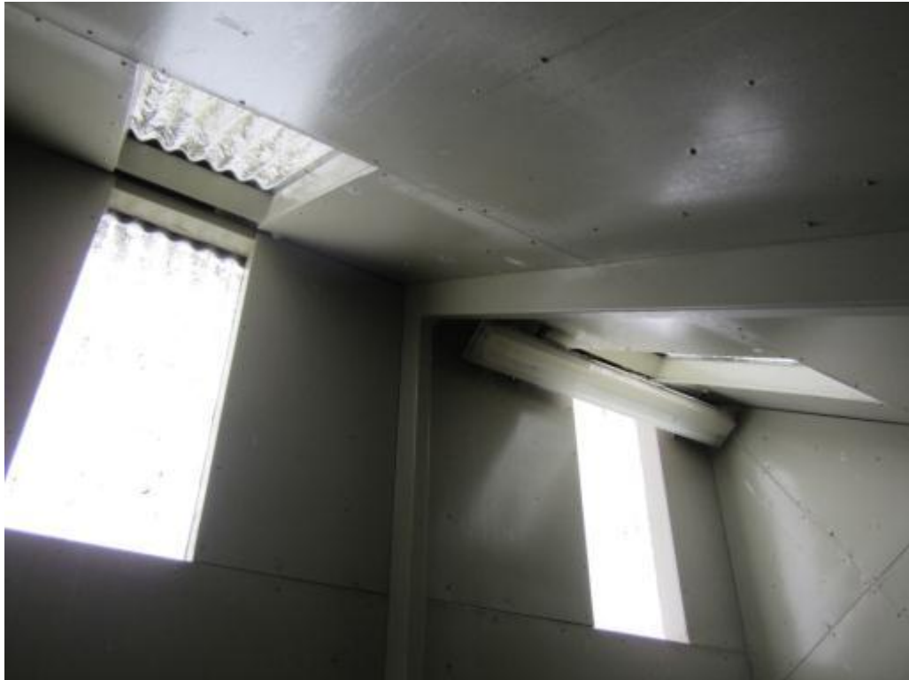
Photo 8. Internal view of ceiling lining, window and A-frame.
