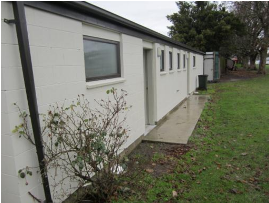
Photograph 2 View of the main Southwest wall.
