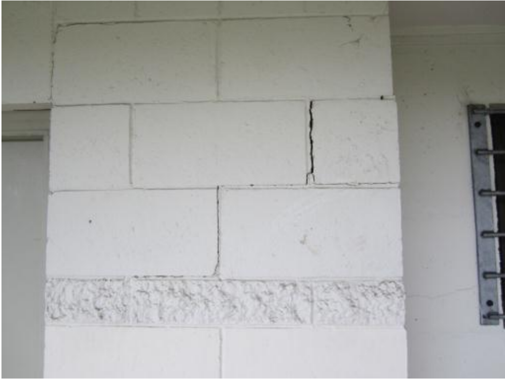
Photograph 7 Masonry pier containing diagonal crack.
