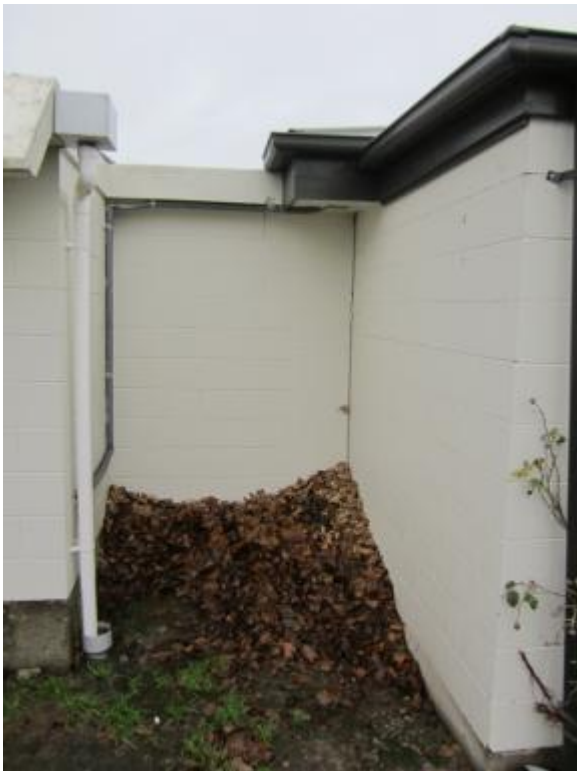
Photograph 4 Gap between building sections in back right corner.
