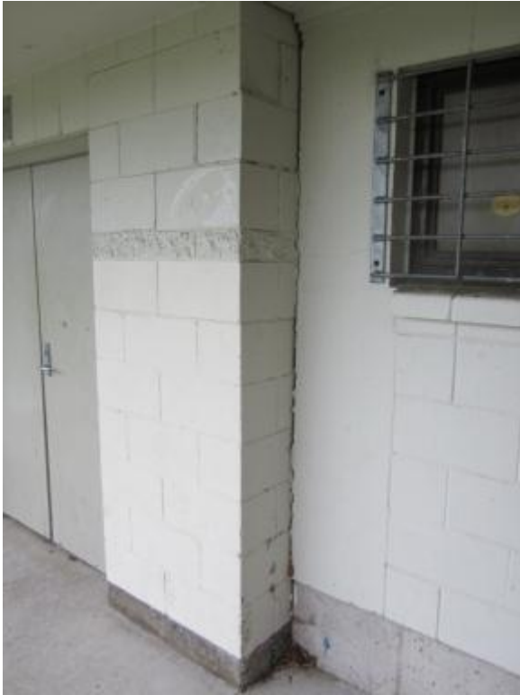
Photograph 3 Gap between two sections of structure, cracking to mortar top left.
