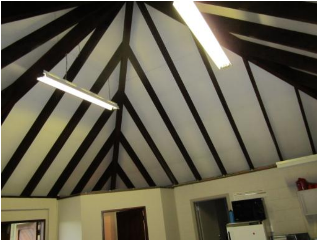
Photograph 6 Internal view of vaulted roof.
