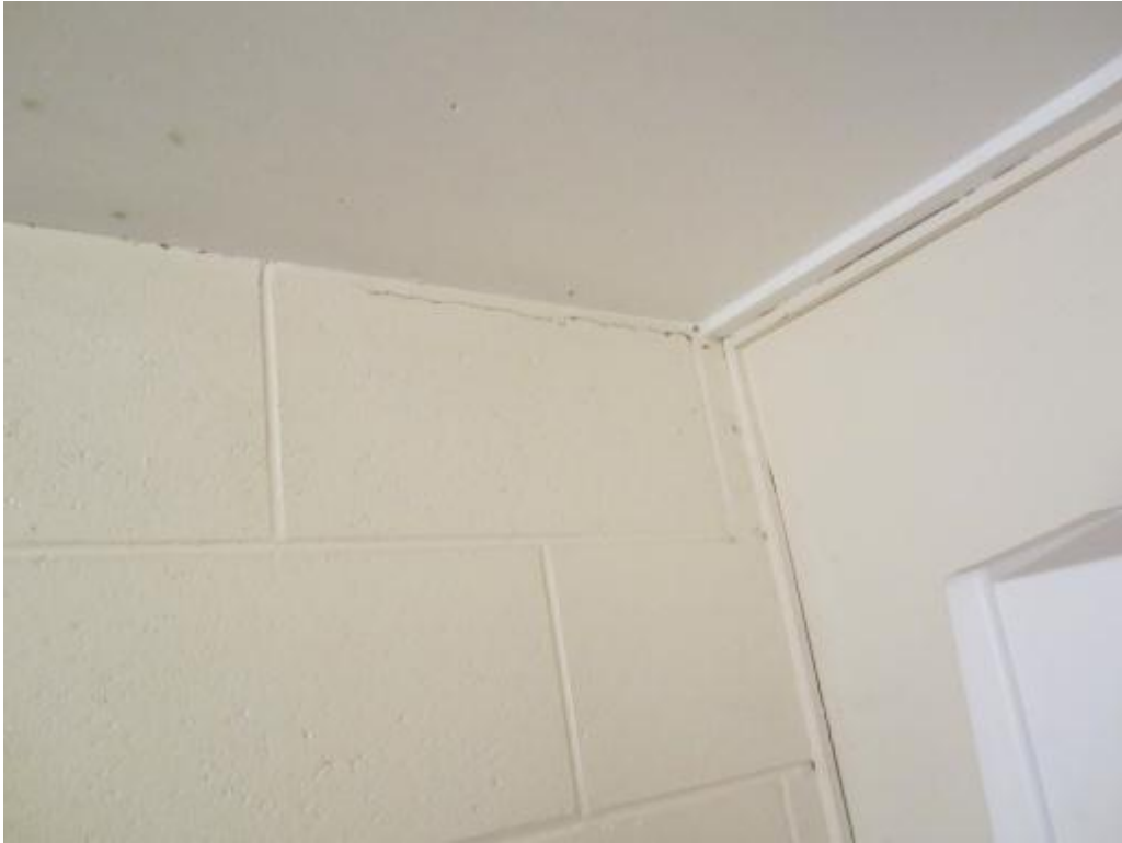
Photograph 5 Crack along bedding mortar of precast concrete roof slabs.
