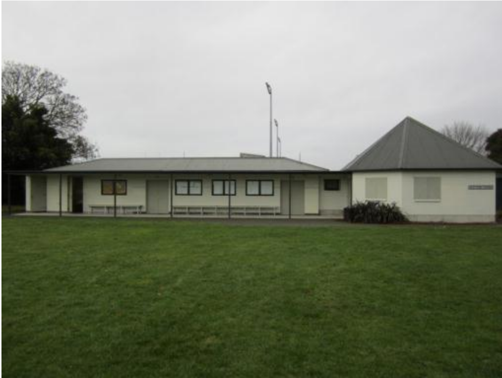
Photograph 1 View of building from the Northeast.
