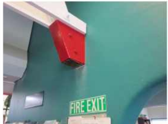
PHOTO 27: Dust coming out of the supporting bracket of roof truss T2
