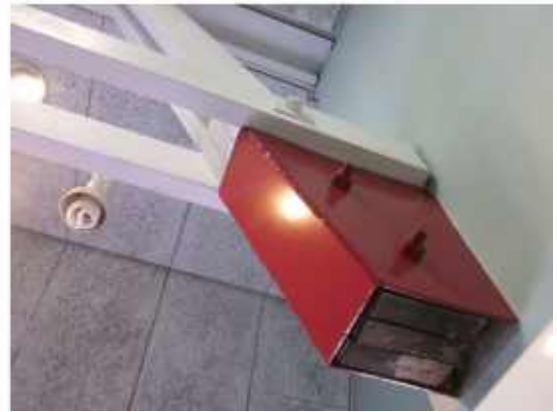
PHOTO 13: Roof trusses in the library – detail on supporting brackets
