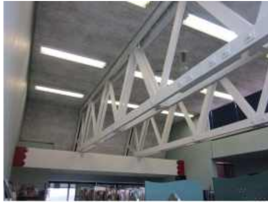
PHOTO 14: Roof trusses in the library – (T6 & T7)
