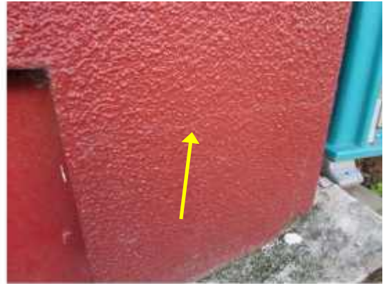
PHOTO 37: Typical external cracking of concrete shear walls
