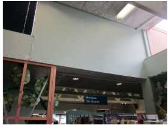
PHOTO 19: Temporary propping of the ceiling on grid line 4.
