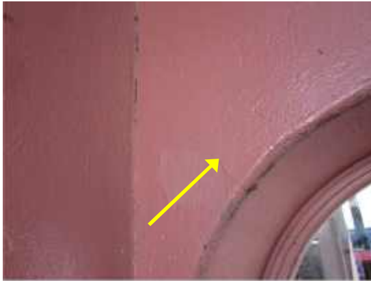
PHOTO 36: Typical external cracking of concrete shear walls
