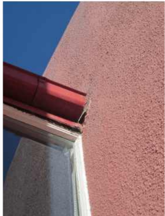
PHOTO 35: View of differential movement between adjacent roof structures.
