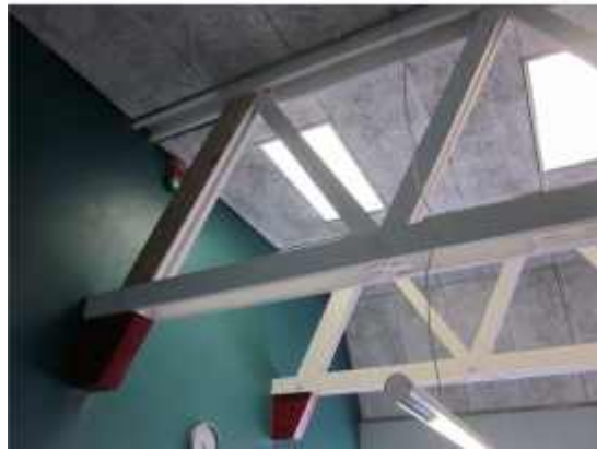
PHOTO 12: Roof trusses in the library (T1 & T2)
