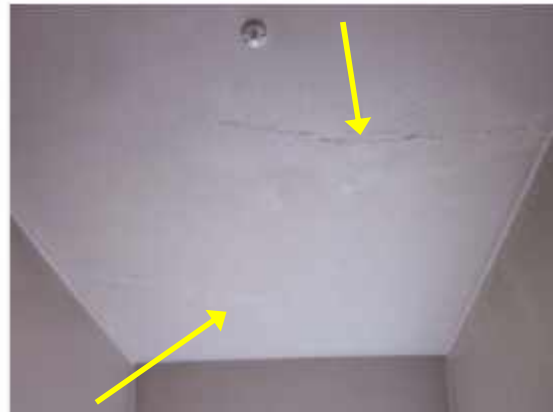
PHOTO 45: Cracking of concrete roof in stair core
