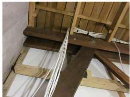
PHOTO 23: Roof Truss (T3)
