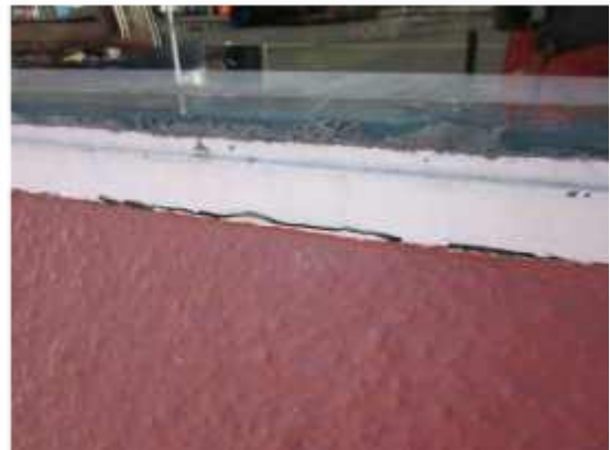
PHOTO 31: Separation of window frames from surrounding structure
