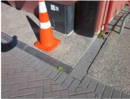
PHOTO 32: View of visible settlement between the structure and the adjacent paving
