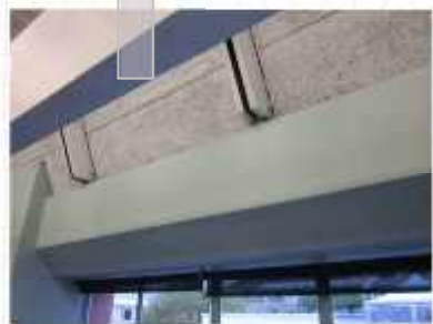
General view on concrete lintel
