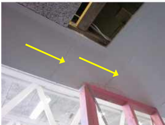
PHOTO 40: Typical plasterboard ceiling cracking
