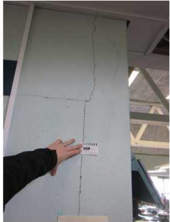
PHOTO 25: Cracking in concrete walls near D/5 (view from the library)
