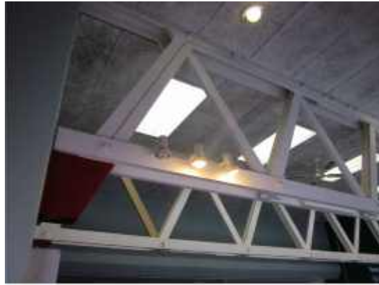
PHOTO 10: Roof trusses in the library (T1 & T2)
