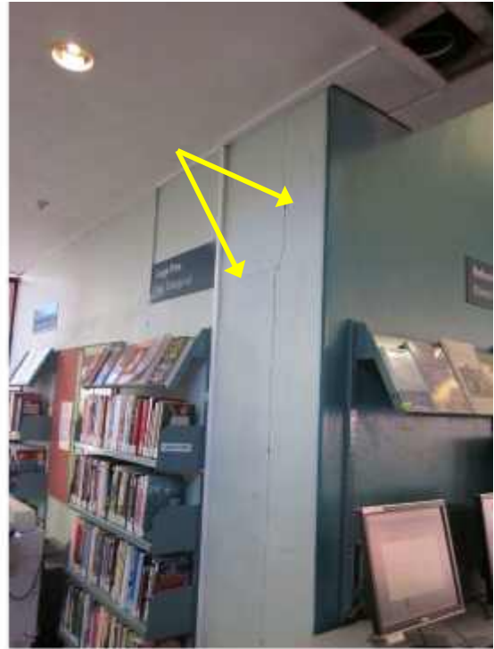
PHOTO 43: Typical plasterboard wall cracking adjacent to concrete wall
