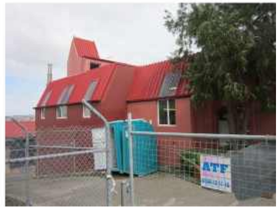
PHOTO 3: Exterior view of the property
