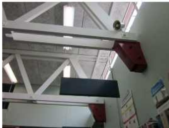
PHOTO 16: Roof trusses in the library – (T6 & T7)
