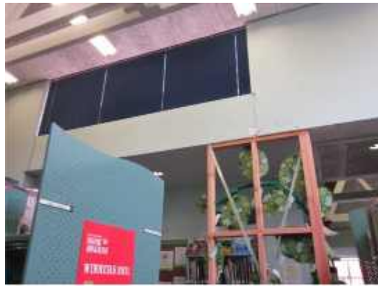
PHOTO 18: Temporary propping of the ceiling on grid line 4.
