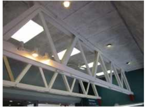
PHOTO 11: Roof trusses in the library (T1 & T2)
