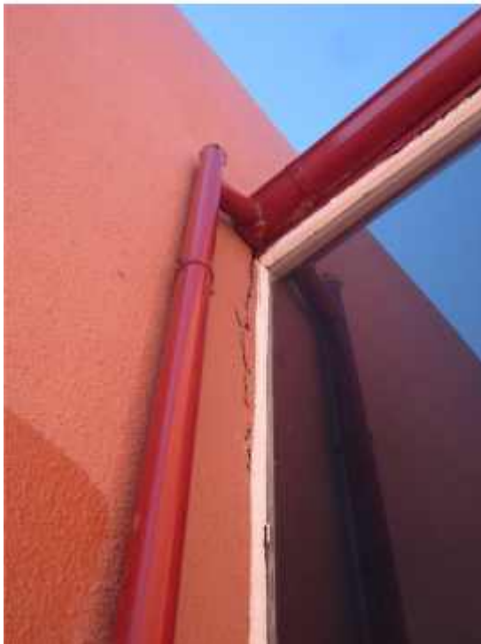
PHOTO 34: View of differential movement between adjacent roof structures.
