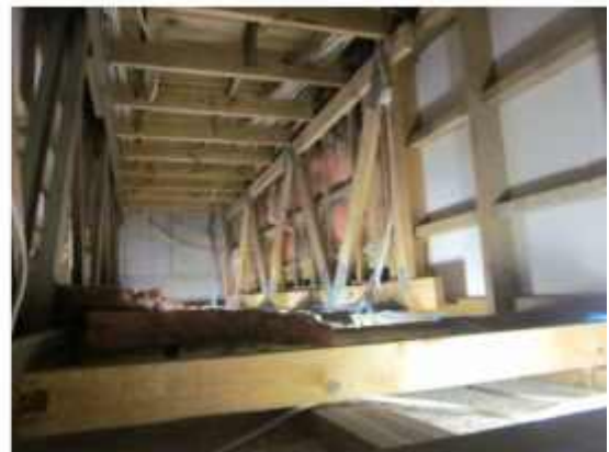
PHOTO 21: Roof Truss (T3) to the left
