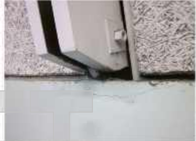
Photo of crack monitoring locations 34 & 35
