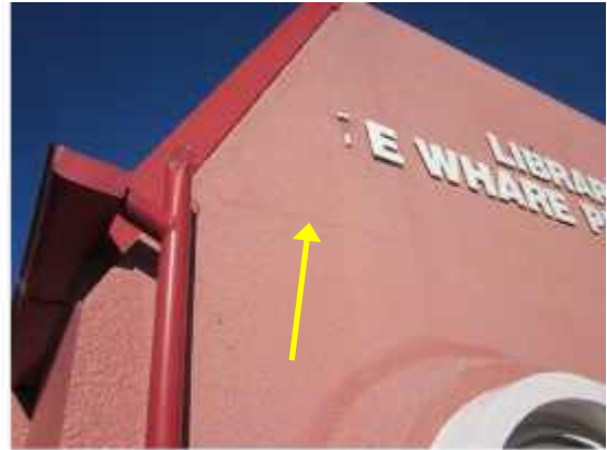
PHOTO 33: Typical external cracking of concrete shear walls
