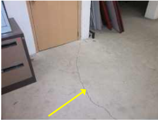
PHOTO 46: Typical cracking of concrete slab on grade
