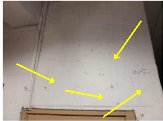
PHOTO 47: Typical internal cracking of concrete shear walls. Wide spread in this location.
