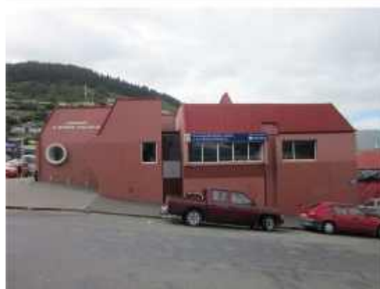
PHOTO 5: Exterior view of the property
