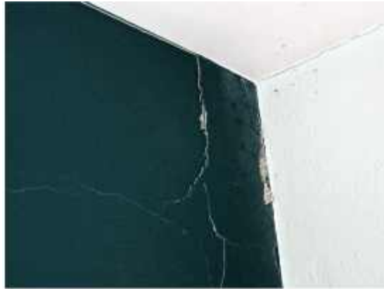
PHOTO 28: Cracking in concrete walls near D/5 (view from the office) – cracking appeared at the location of truss support attached from the other side of the wall)
