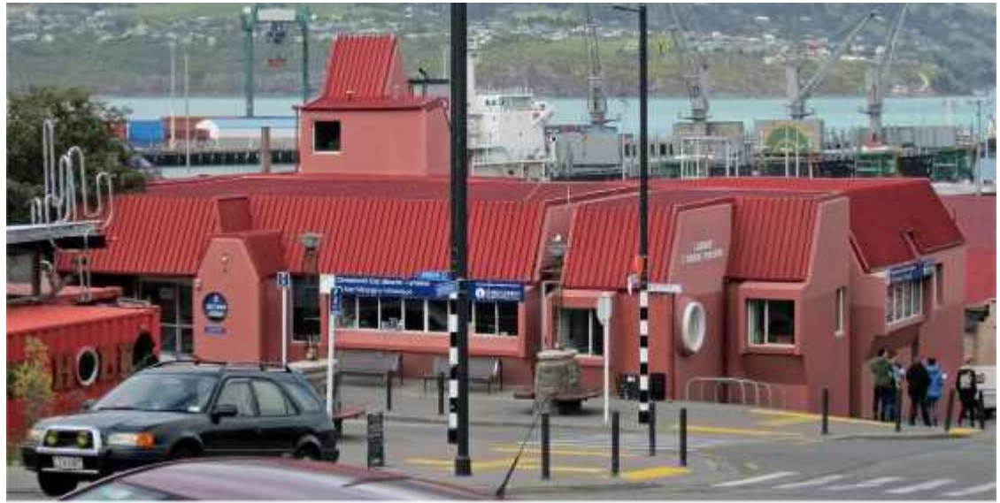
PHOTO 1: Exterior view of the property
