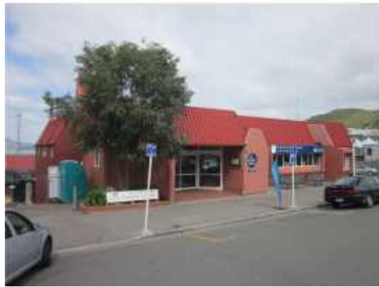
PHOTO 2: Exterior view of the property
