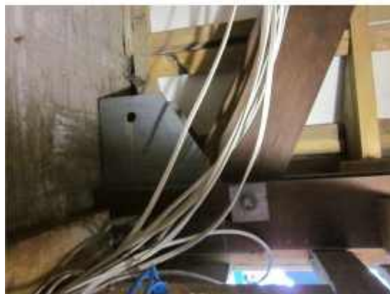
PHOTO 22: Supporting bracket to roof truss T3 – grid D/5
