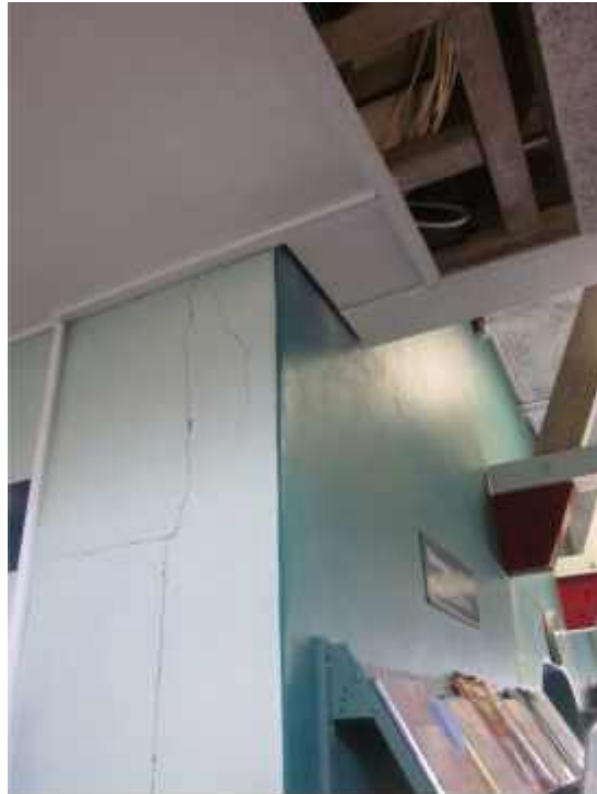
PHOTO 24: Cracking in concrete walls near D/5 (view from the library)
