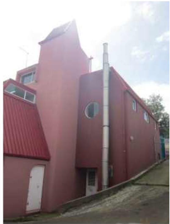
PHOTO 8: Exterior view of the property
