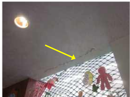
PHOTO 41: Typical plasterboard ceiling cracking
