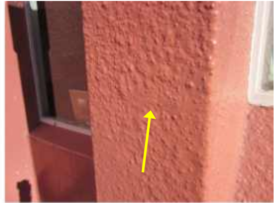
PHOTO 29: Typical external cracking of concrete shear walls
