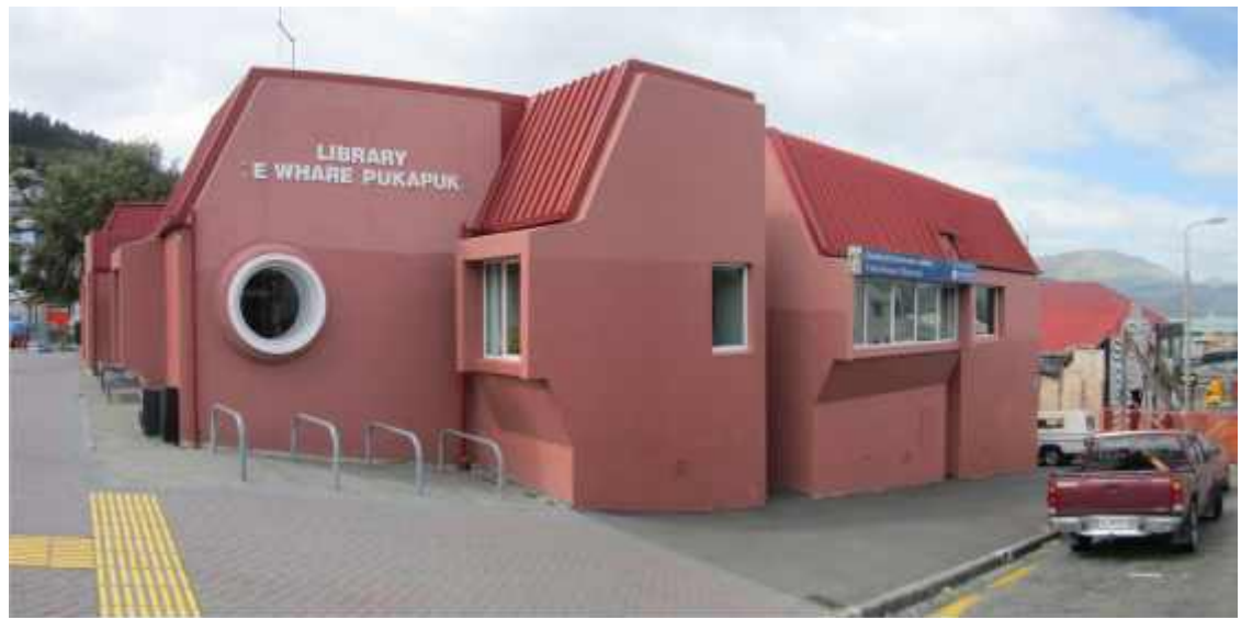
PHOTO 4: Exterior view of the property
