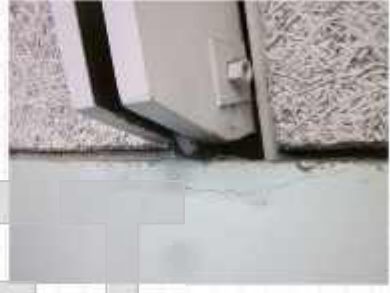
Photo of crack monitoring locations 34 & 35
