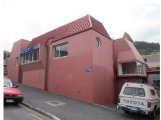
PHOTO 6: Exterior view of the property
