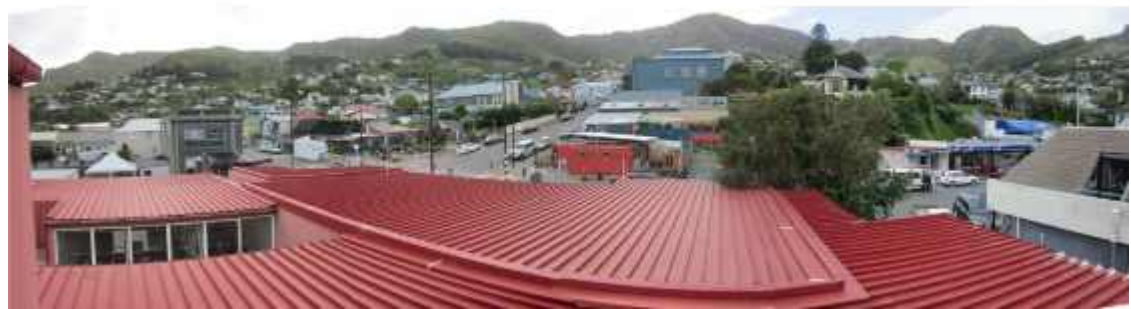
PHOTO 9: Exterior view of the property – roof from the top of the lift shaft
