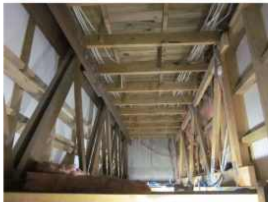
PHOTO 20: Roof Truss (T3) to the left
