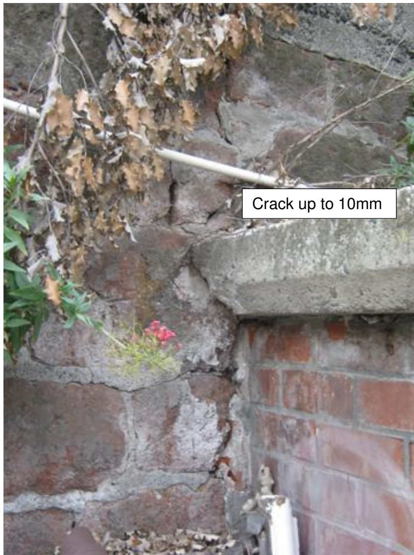
Photograph 7. Wall cracks
