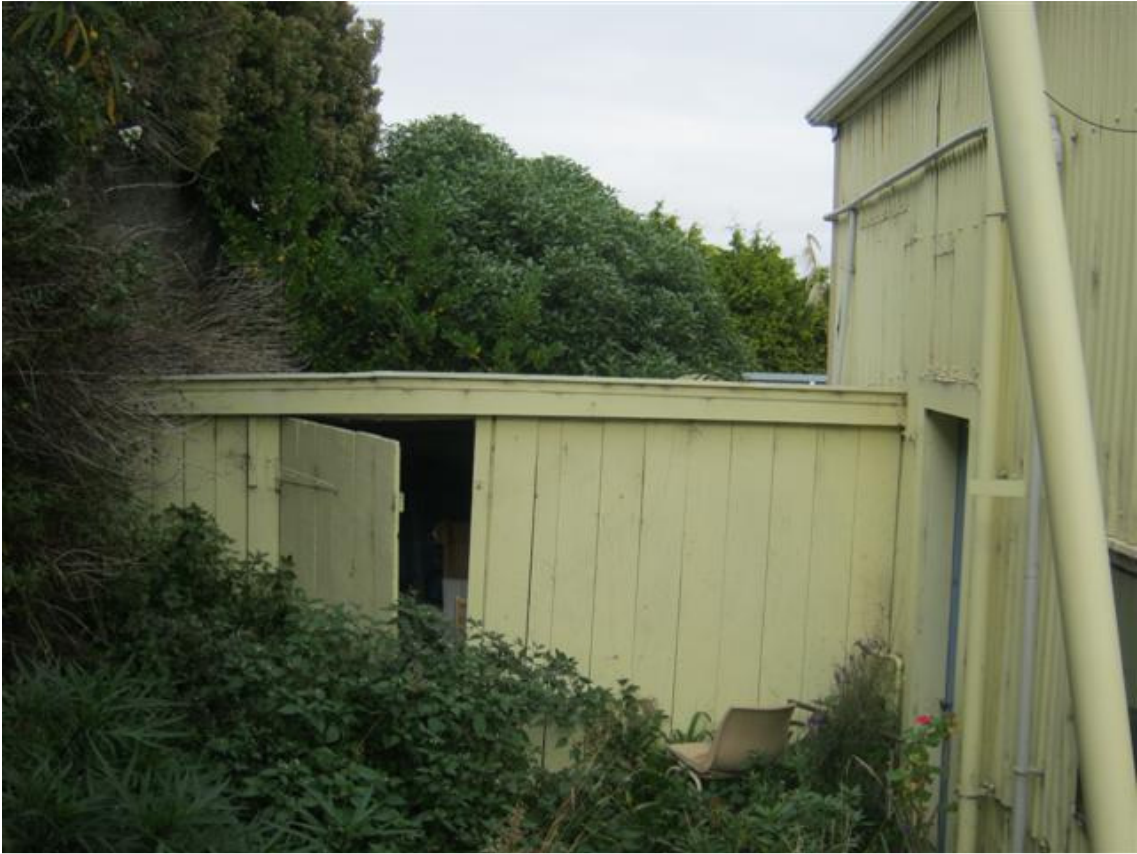
Photograph 1. Shed at the rear of the building
