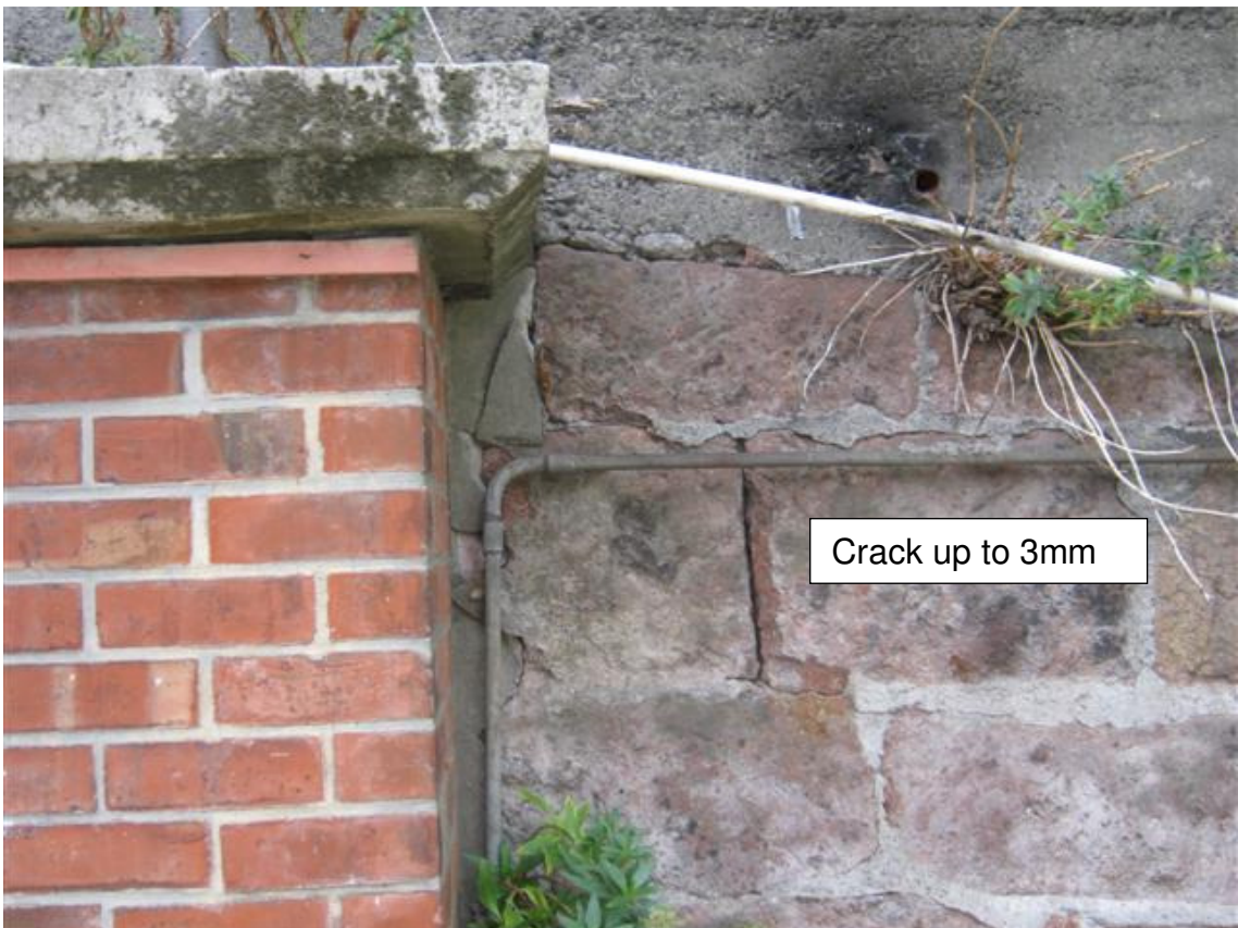
Photograph 6. Wall cracks
