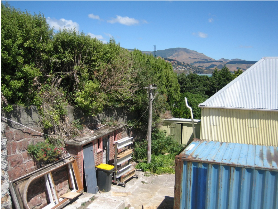
Photo 9: View of the retaining wall and shed at rear of the building
