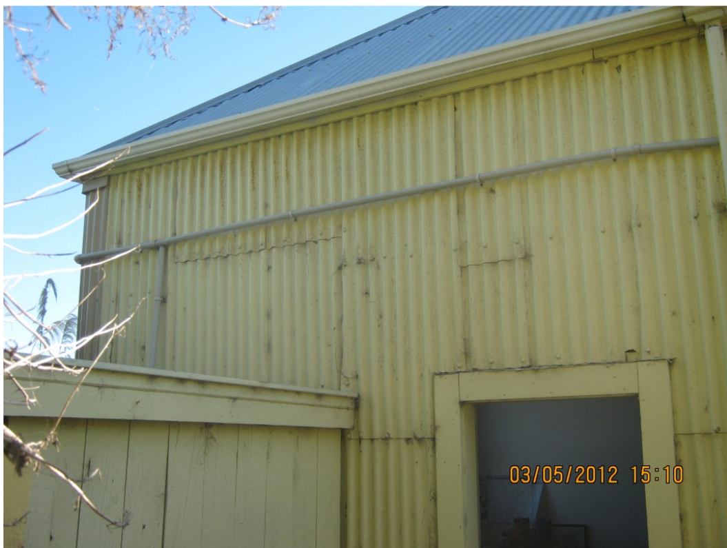
Photo 8: View of the back of the building and adjacent shed
