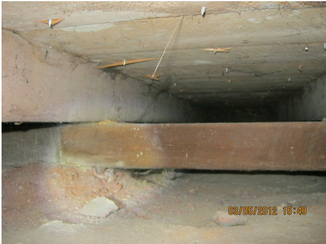
Photo 5: Subfloor bearers on rock piers
