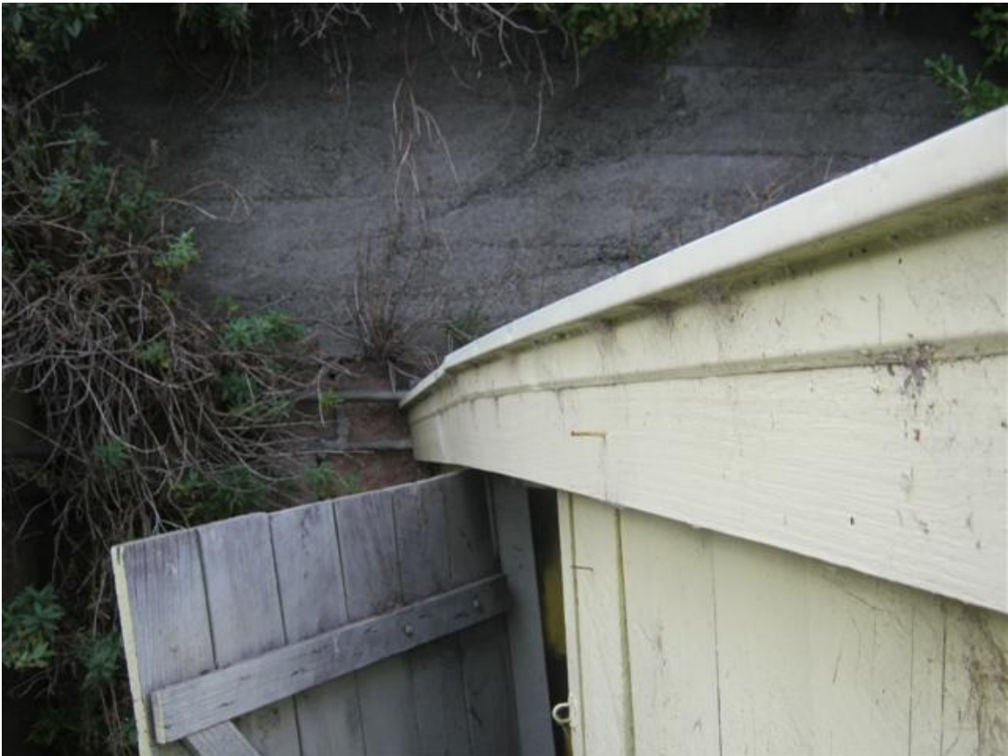
Photograph 2. Deformations along the roof of the shed
