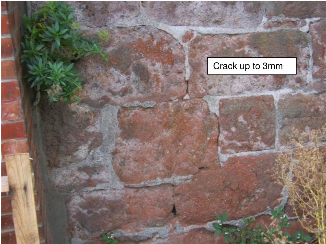
Photograph 5. Wall cracks
