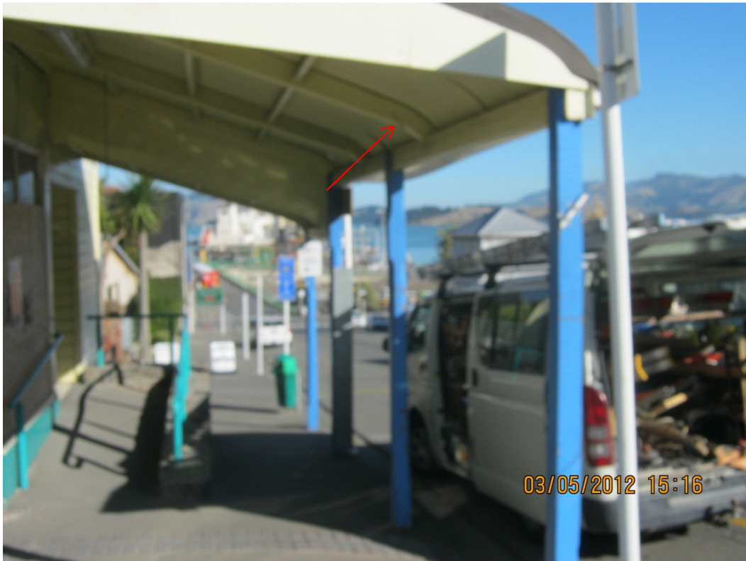
Photo 3: View of Front canopy – splice at curve of rafter
