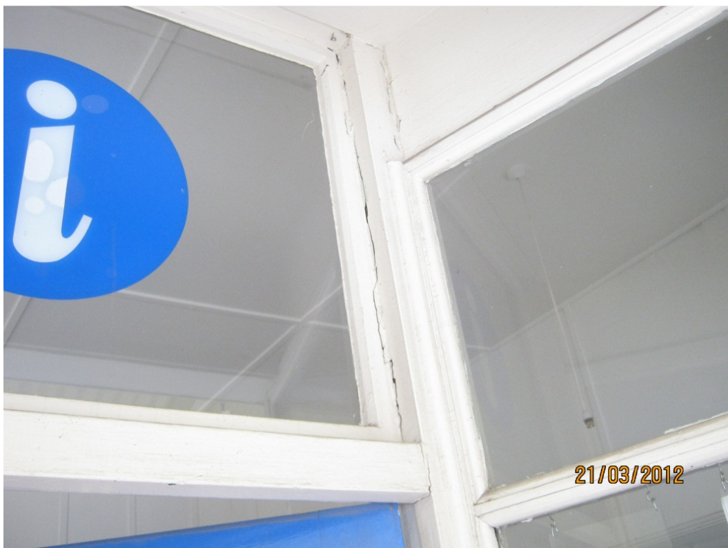
Photo 6: Crack in the window frame above the front door
