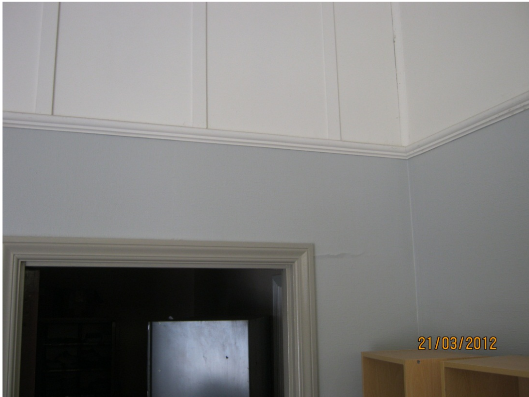
Photo 7: Horizontal crack in the internal wall
