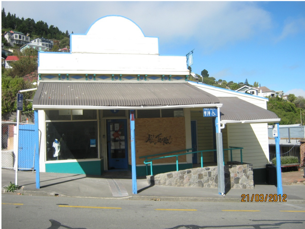
Photo 1: View of the building from the street. Broken window glass in the front
