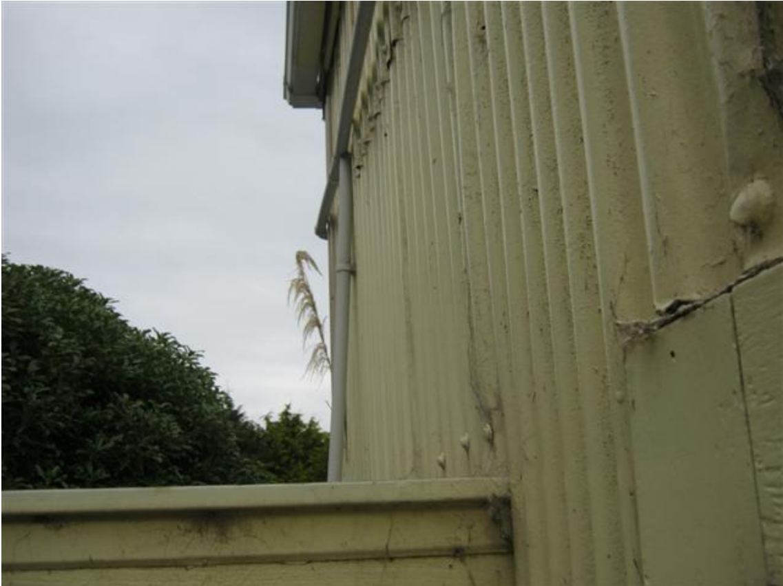
Photograph 3. Joint between the shed and building
