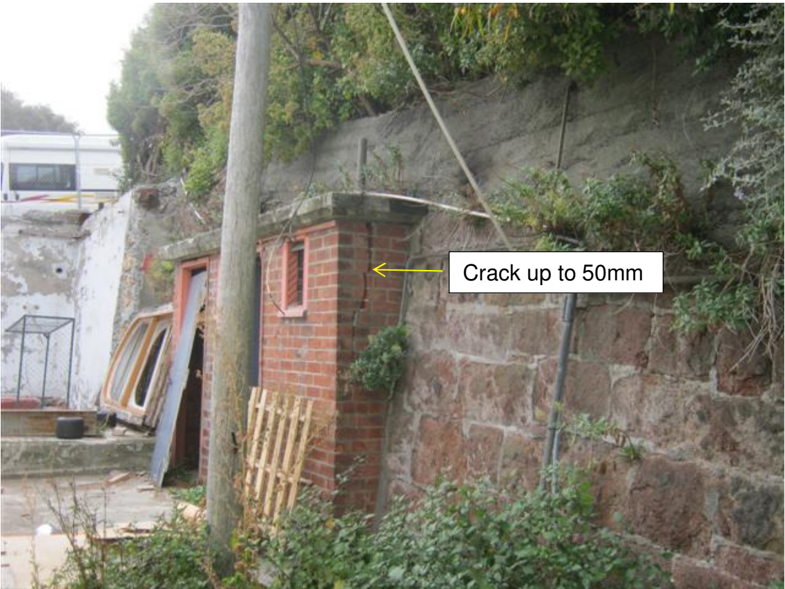
Photograph 4. Neighbouring structure cracks due to wall movement
