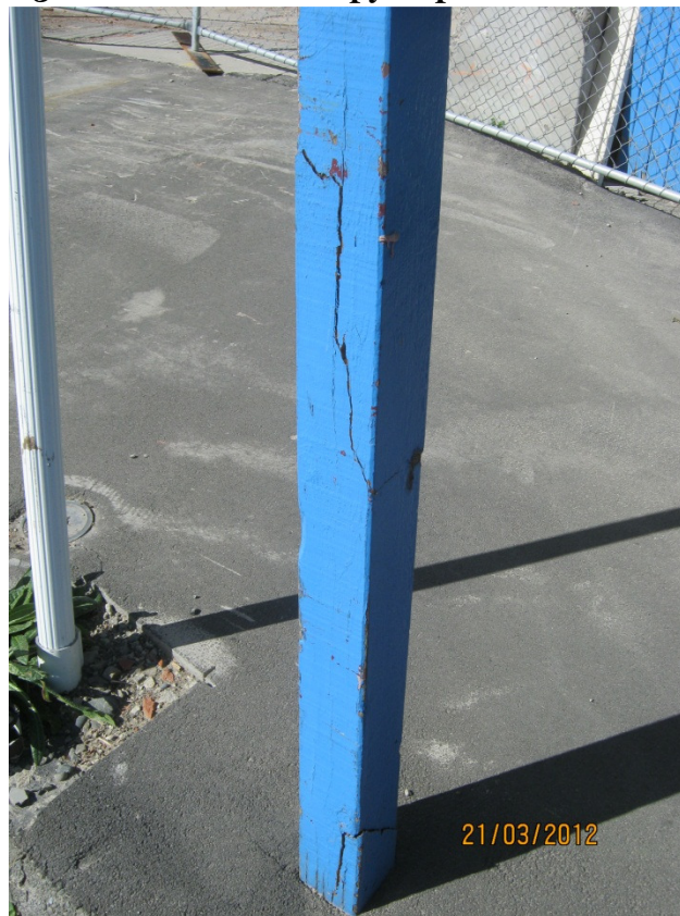
Photo 4: Cracked verandah post
