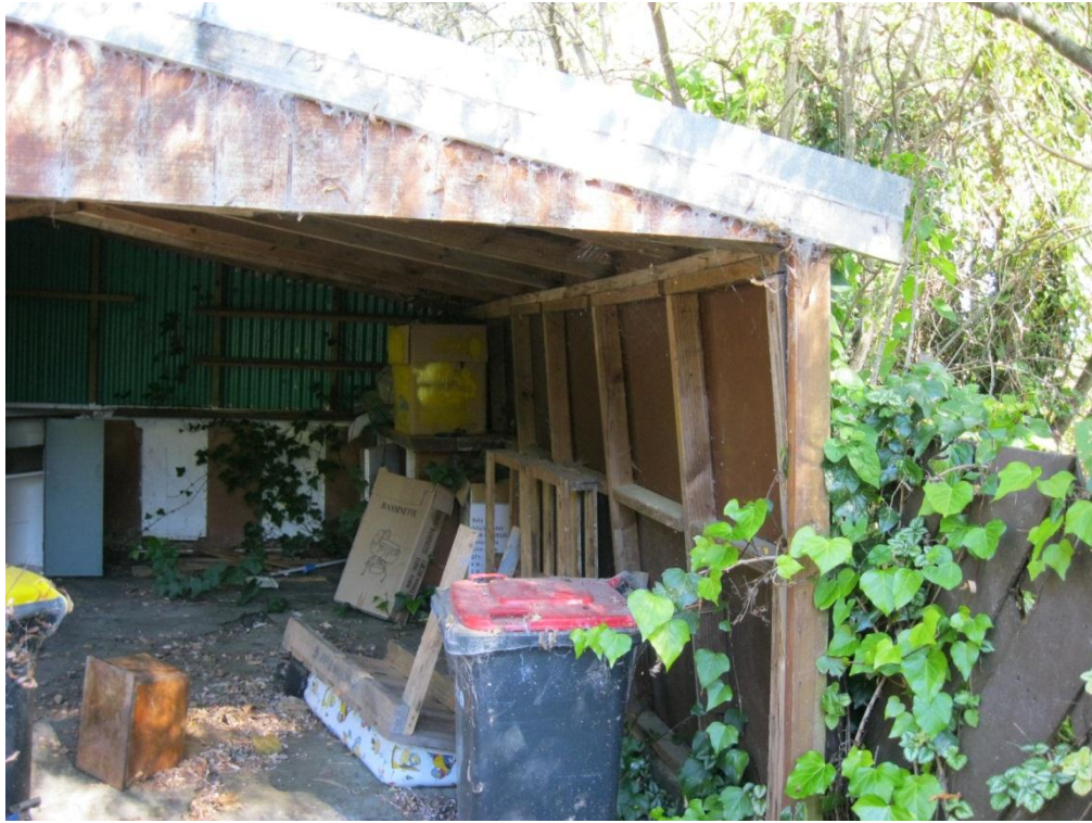
Photograph 5 View of the lateral wall- view from the north.
