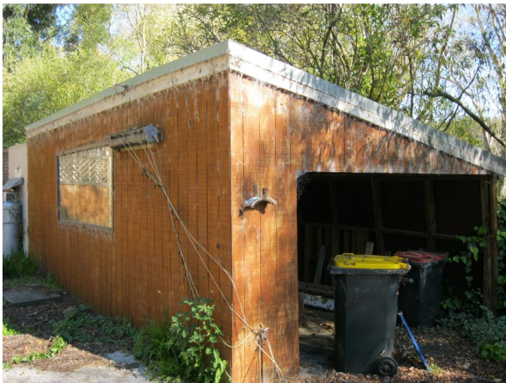
Photograph 3 View of the garage from the northeast.
