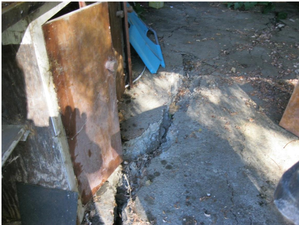
Photograph 6 Cracking of the slab on grade.
