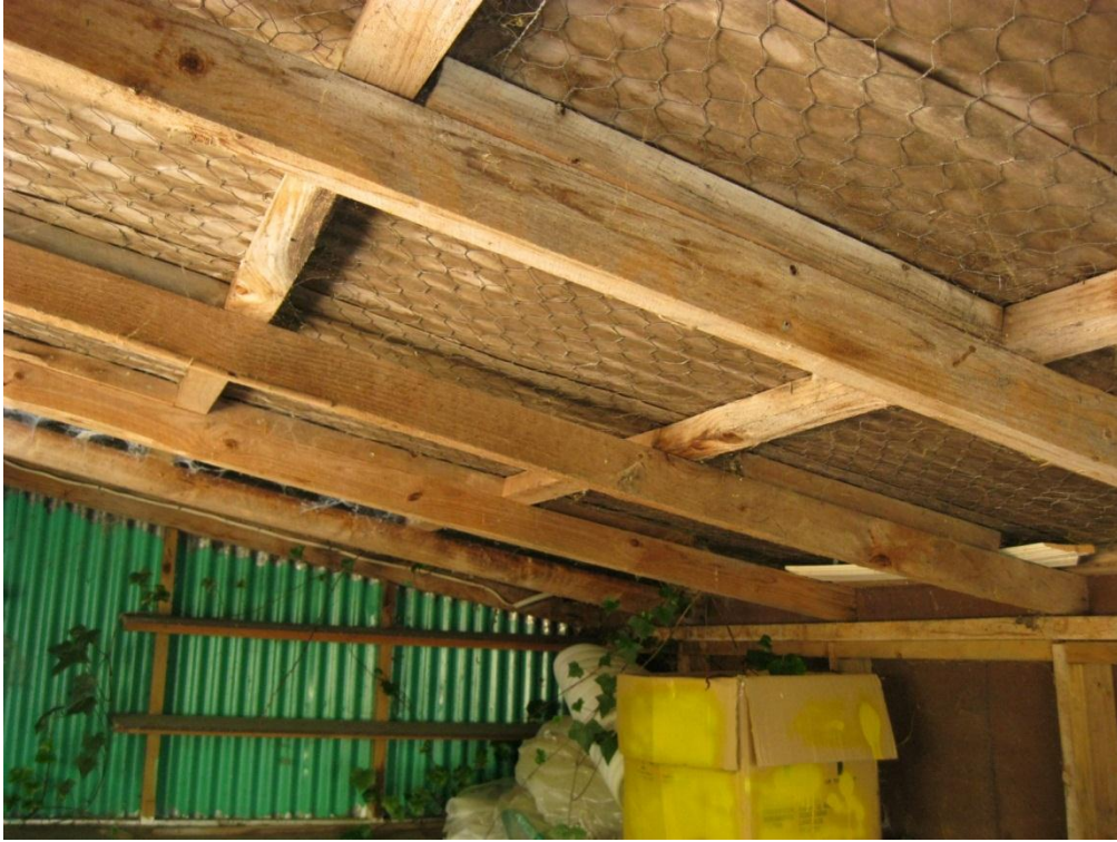
Photograph 7 Internal view of the southern corner of the building showing roof construction.
