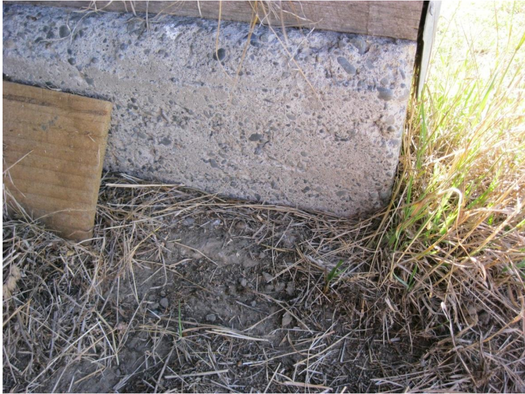
Photograph 7 Concrete strip footing foundations to the perimeter walls.
