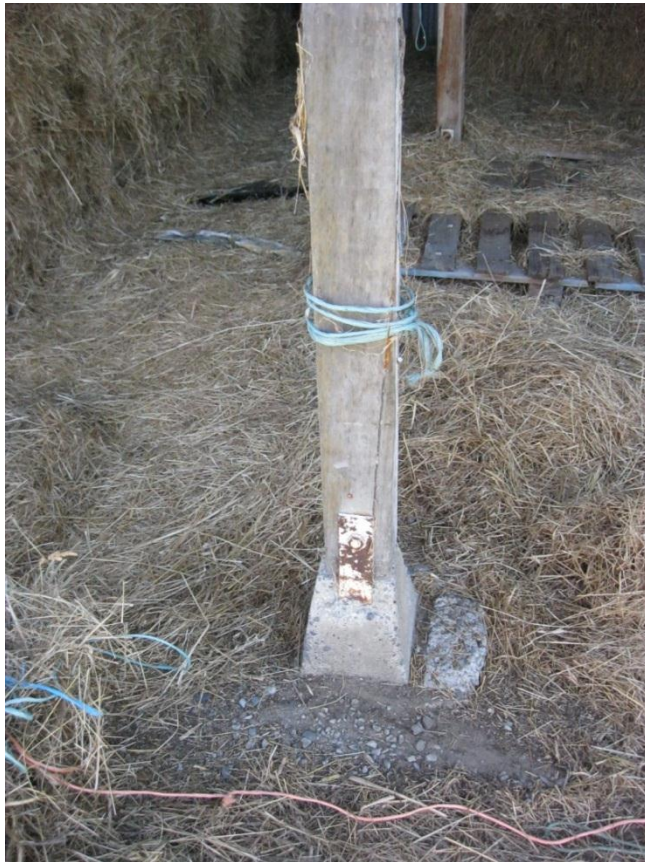
Photograph 8 Cracked timber support post.
