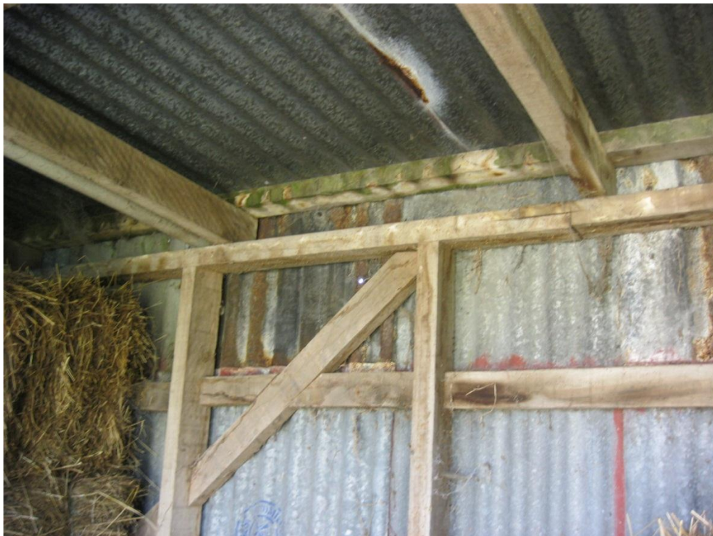
Photograph 6 Timber framed wall to the rear showing timber cross bracing.
