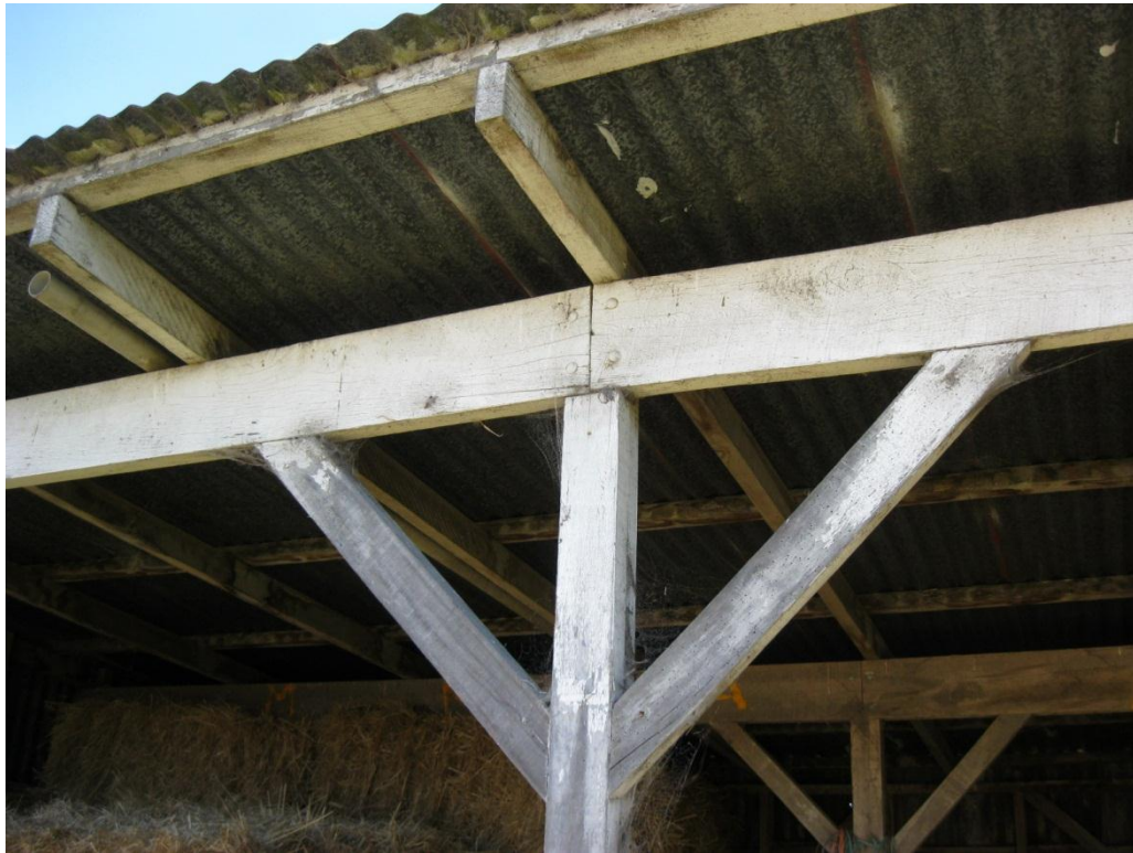
Photograph 5 Timber beam and post system on the front and centre of the building showing the knee connection. Lack of roof sarking is clearly visible.
