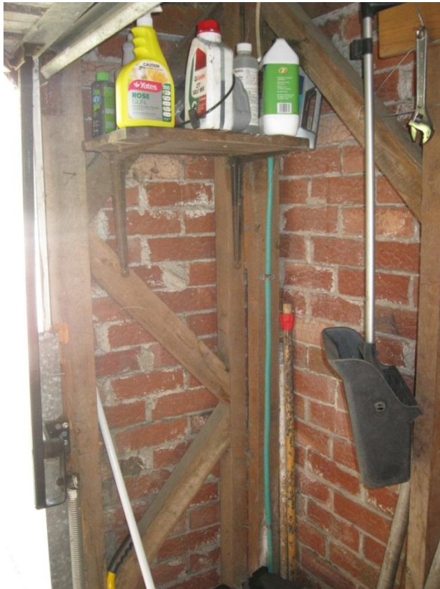
Photograph 6 Internal view of the southern corner of the building showing wall bracing.
