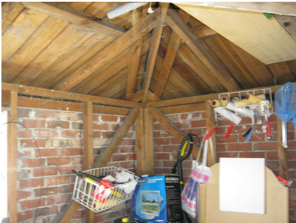
Photograph 7 Timber roof bracing and roof trusses visible.
