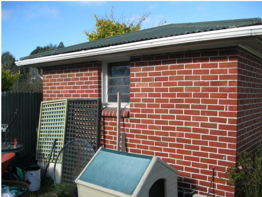
Photograph 4 View of the garage from the northwest.
