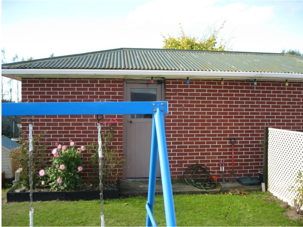
Photograph 3 View of the garage from the southwest.
