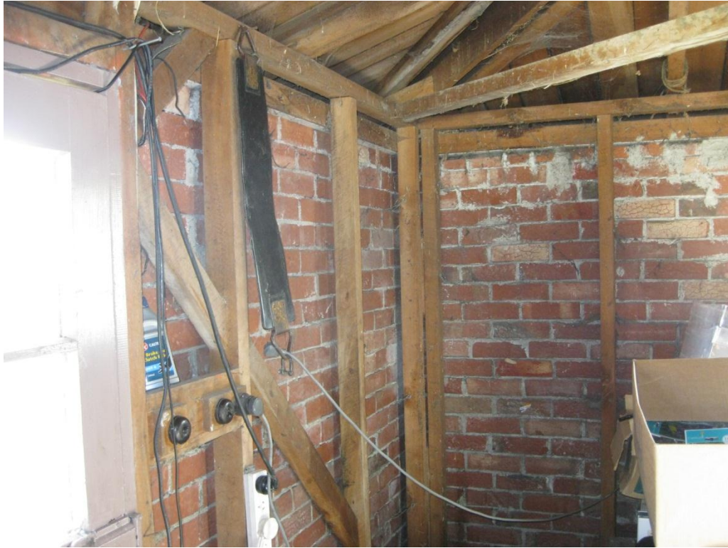
Photograph 5 View of the interior at the western corner of the building. No internal wall linings. Roof and wall bracing is clearly visible.
