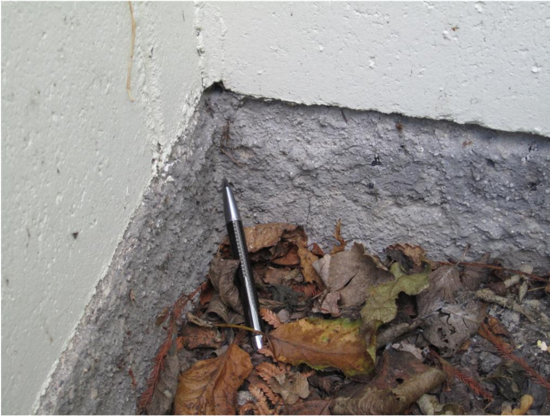
Photo 1: Hairline crack in foundation on south side of Unit 1 to 2
