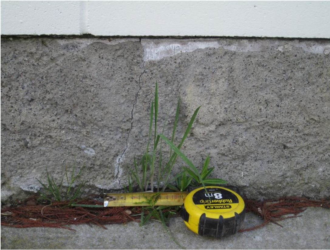
Photo 9: 1mm wide crack in foundation on southern end of Units 3 to 8
