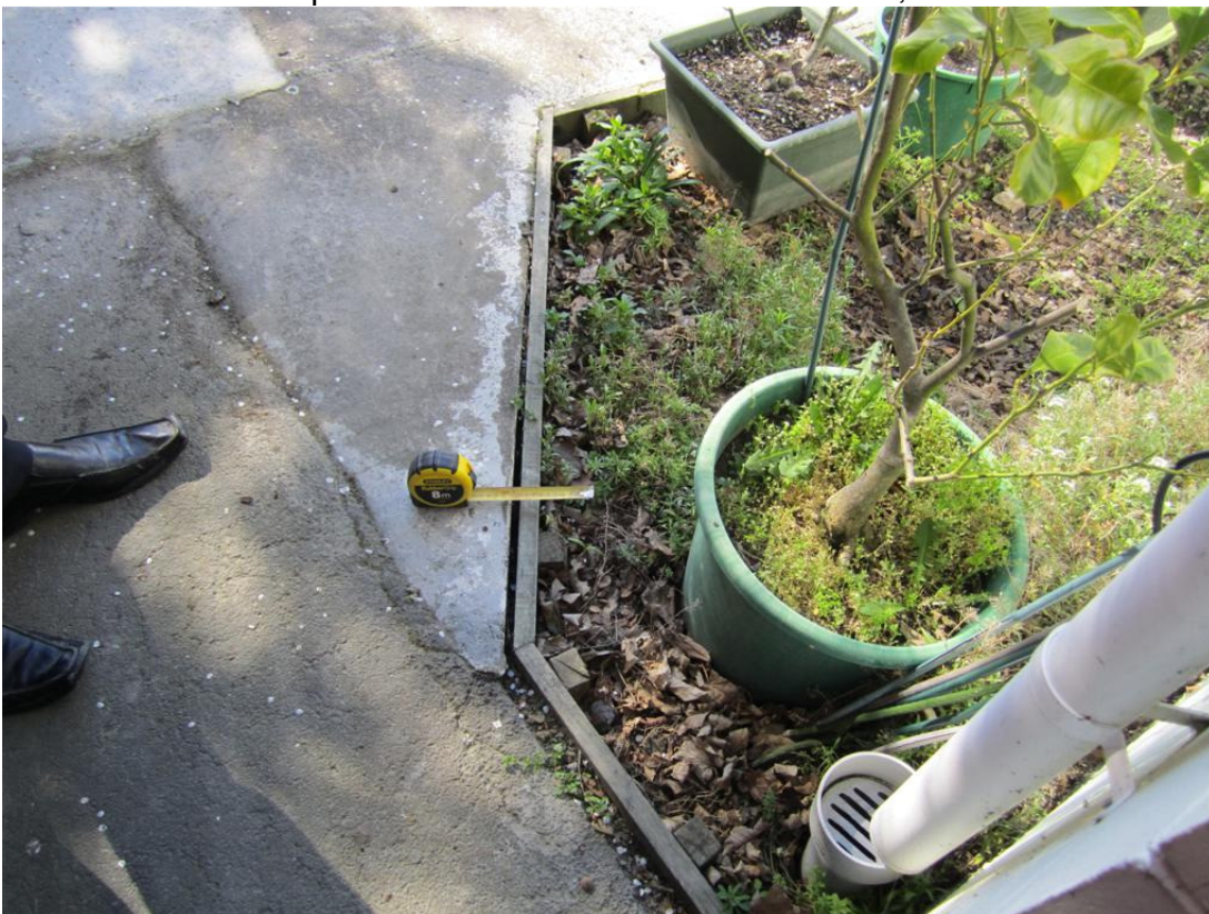
Photo 4: Crack (<1mm to 10mm wide) around path on north west end of Unit 1 to 2
