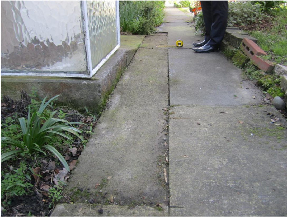
Photo 23: Distortion on path on south end of Units 9 to 13
