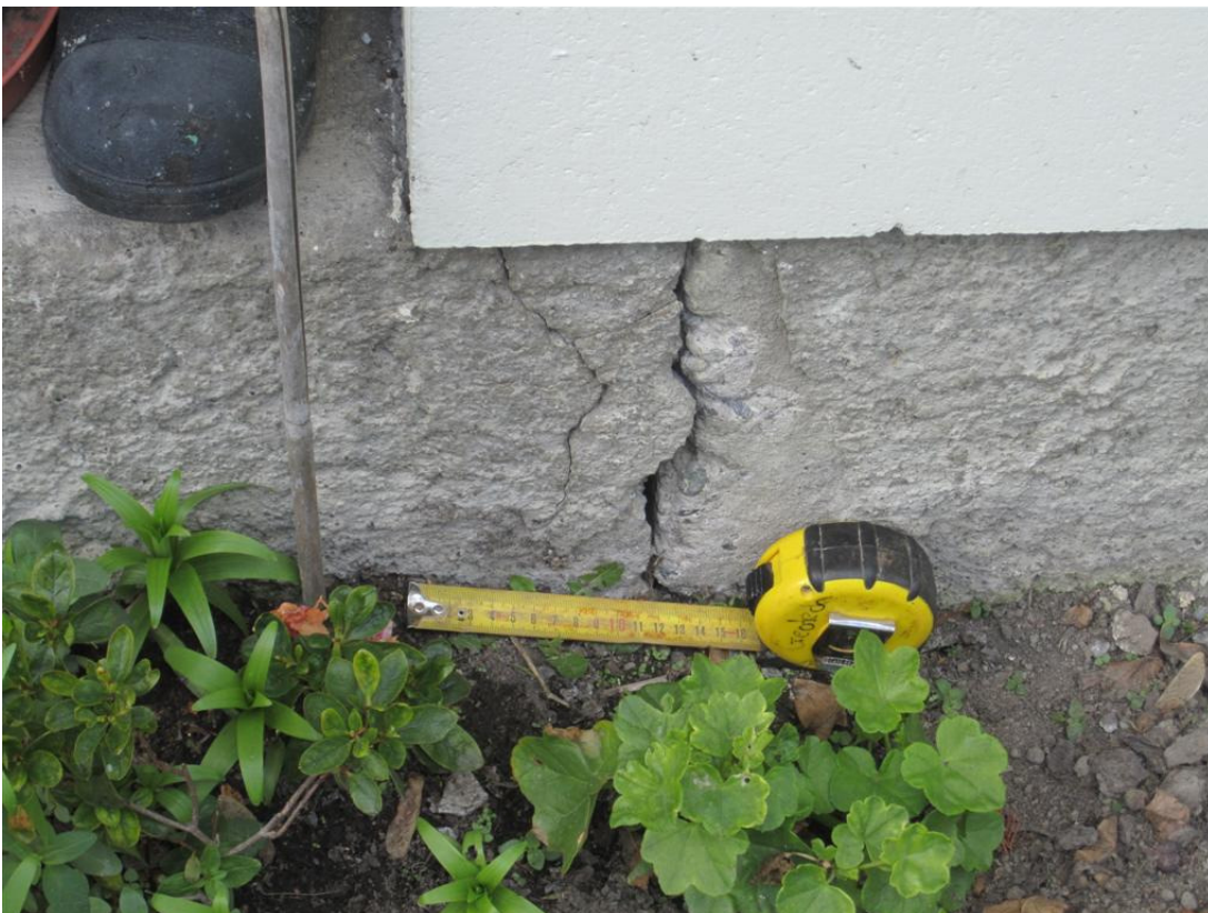
Photo 12: Cracks (up to 10mm wide) on west end of Units 3 to 8
