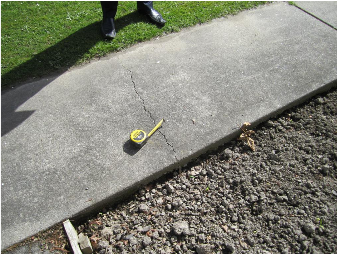
Photo 16: Crack (less than 5mm wide) in path close to south west part of Unit 3 to 8
