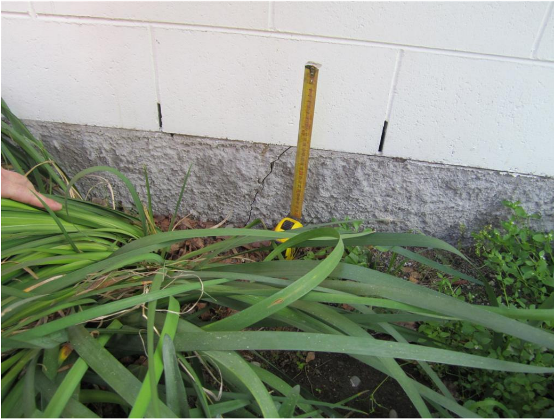
Photo 15: Crack (less than 5mm wide) on northern end of Units 3 to 8
