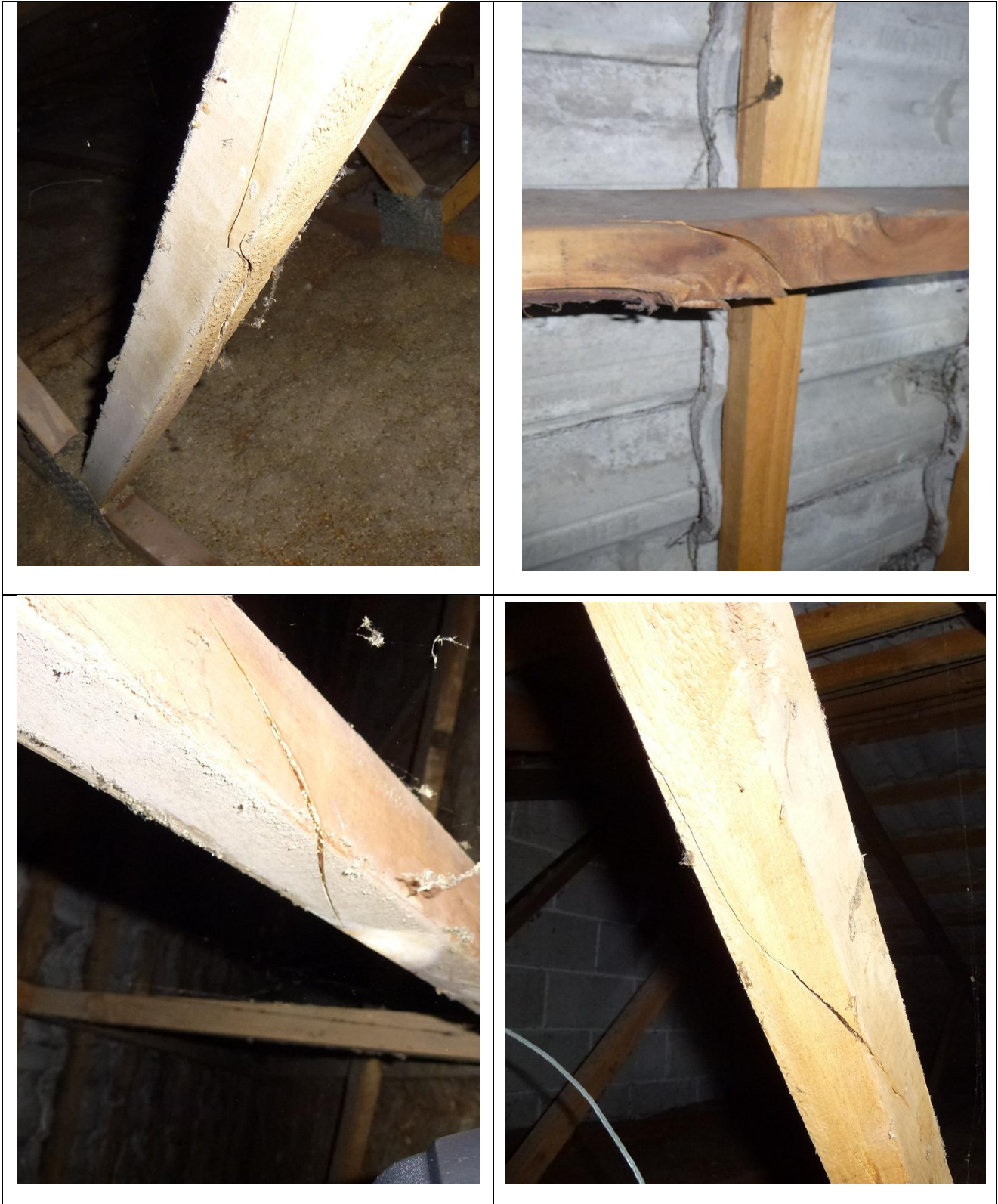
Photos 12 – 15: Breaking of roof trusses
