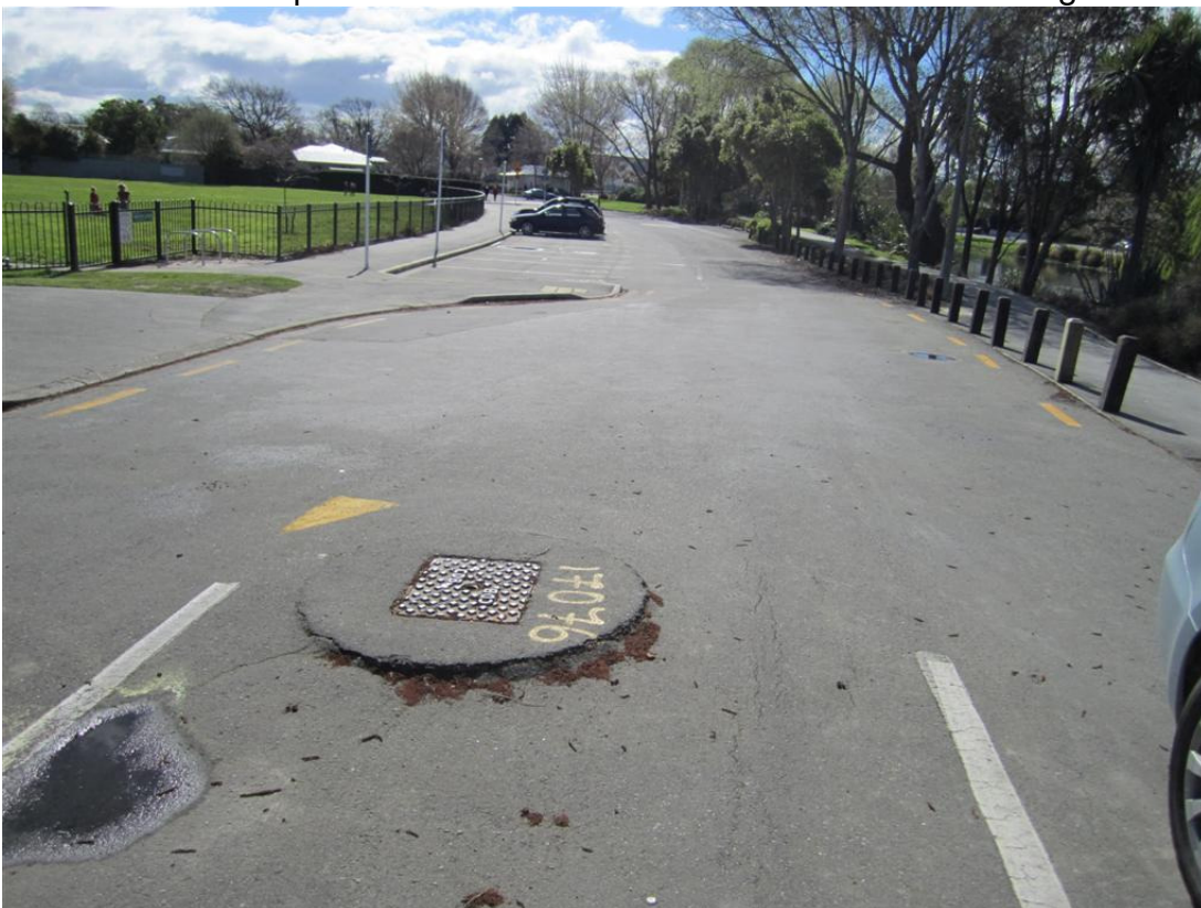
Photo 26: Manhole cover and chamber that has heaved 25mm-30mm.
