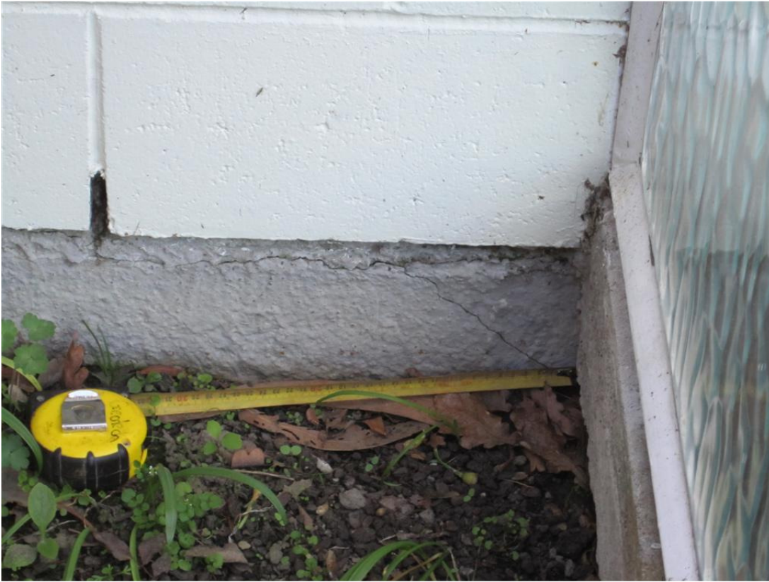
Photo 21: Crack (1mm wide) on south end of Units 9 to 13
