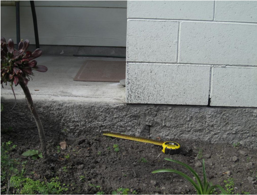
Photo 13: Hairline cracks on west end of Units 3 to 8
