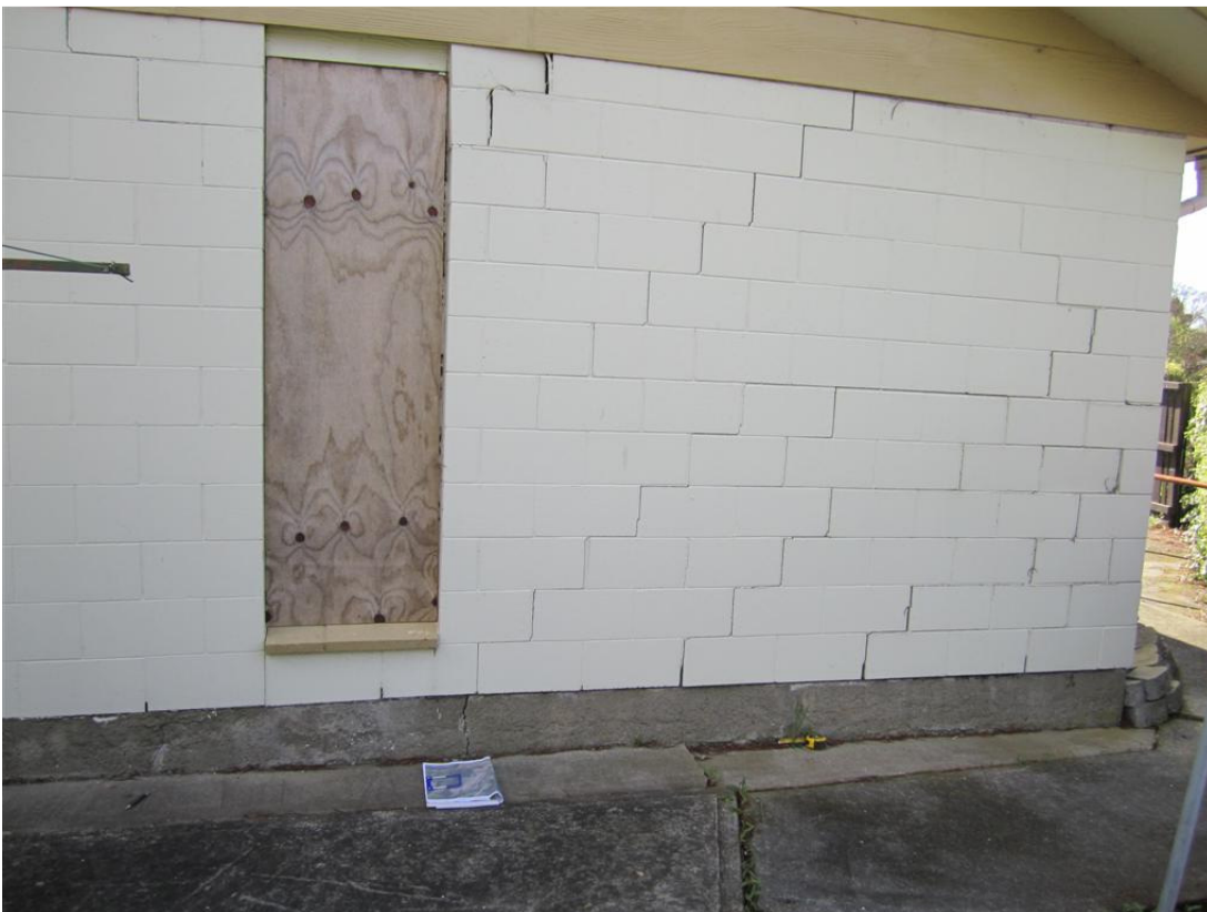
Photo 10: Step cracks on south side of Units 3 to 8
