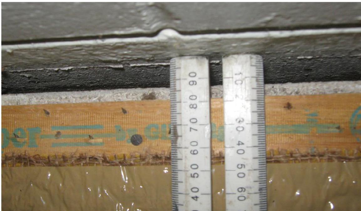
Photo 6: Ground slab separation from the foundation beam
