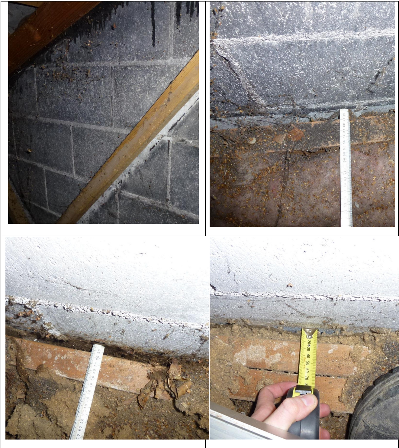
Photos 19 – 22: Blockwall separation
