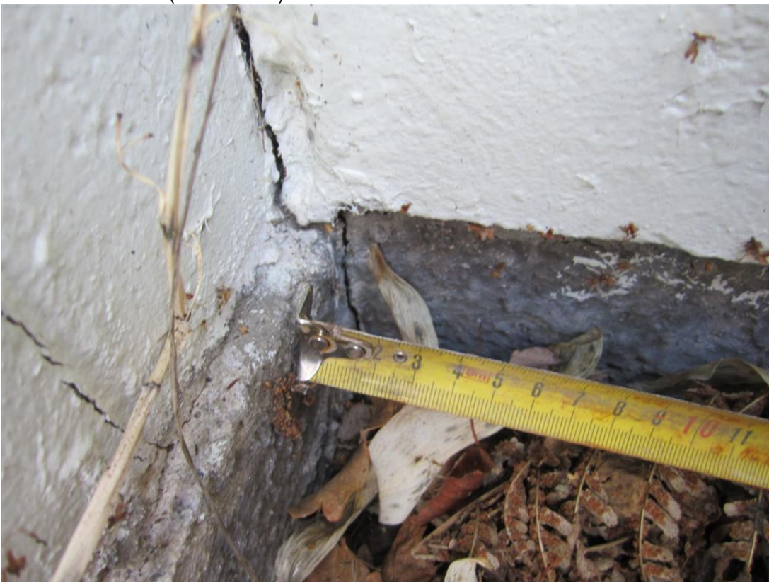
Photo 22: Crack (2mm wide) on south end of Units 9 to 13
