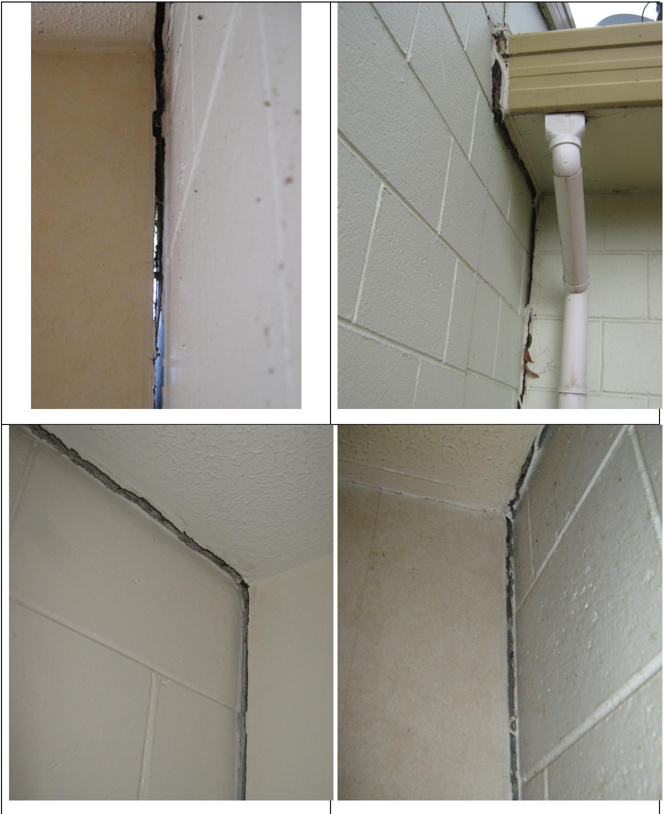
Photos 8 – 11: Blockwall separation
