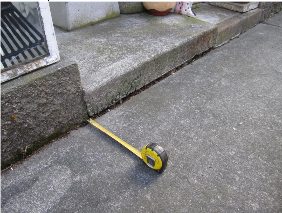
Photo 18: Slab separations on east end of Units 3 to 8
