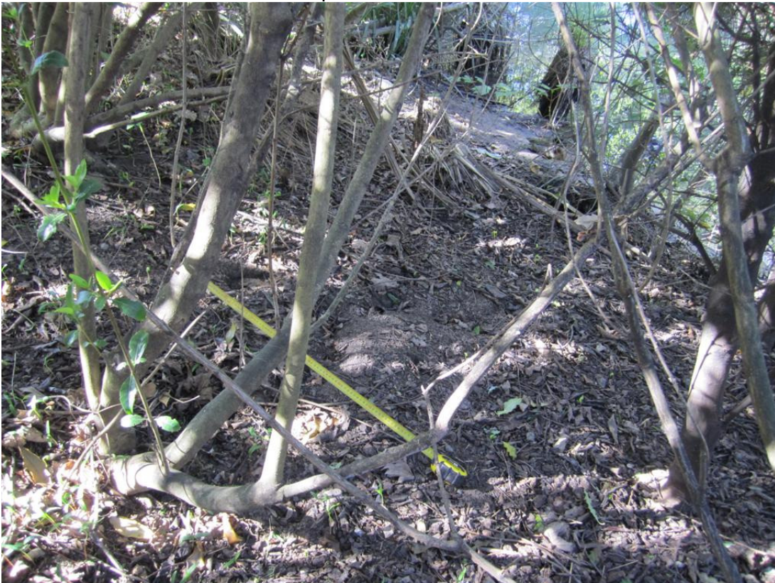
Photo 6: Suspected scarps / cracks on slope close to stream south of Units 1 and 2.
