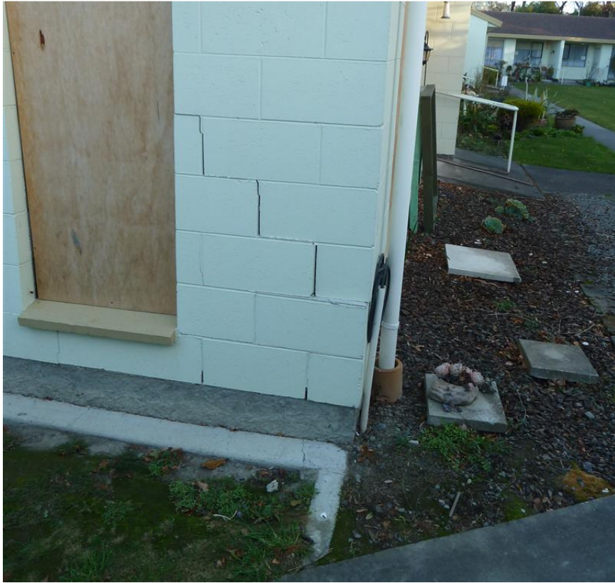
Photo 3: Cracking to block veneer
