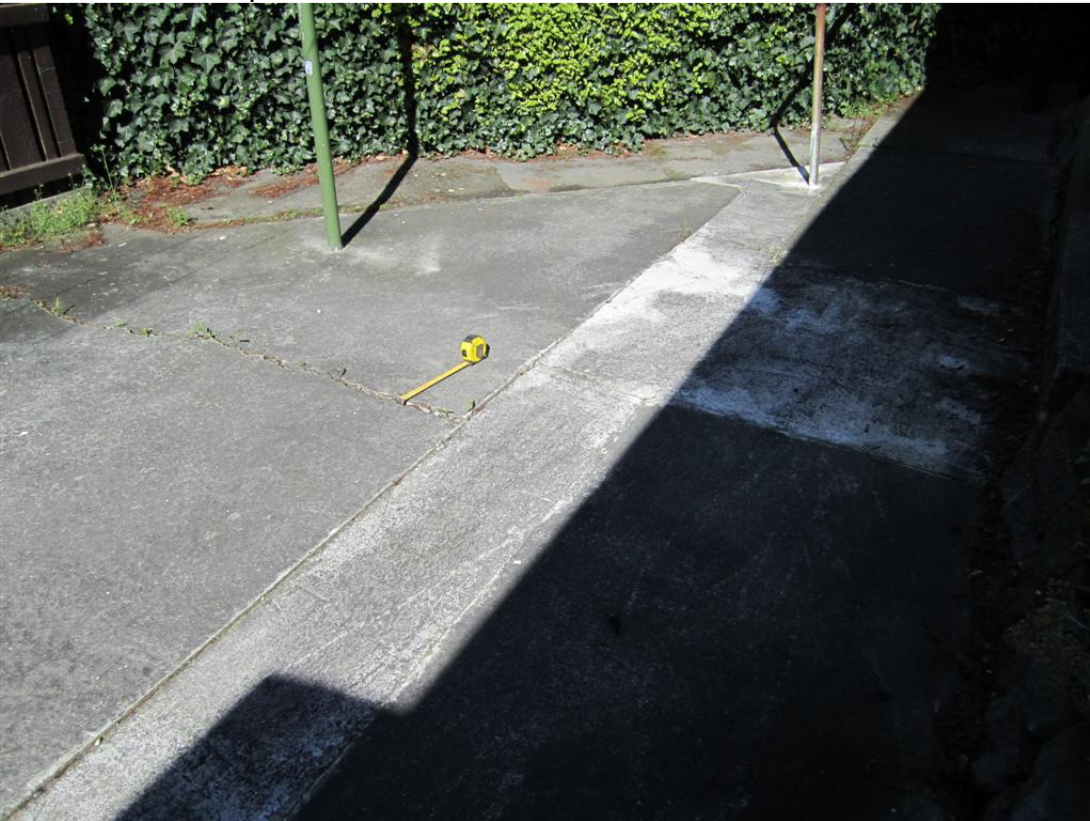
Photo 20: Paving slab distortion east of Units 3 to 8
