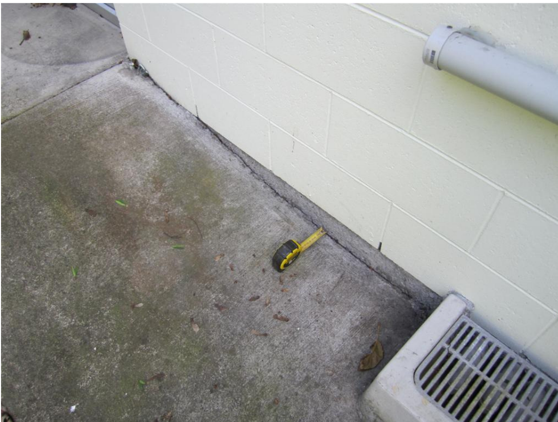
Photo 2: Slight separation (<math><5\text{mm}</math>) between foundation and concrete path
