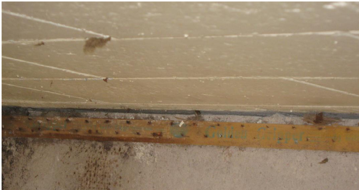
Photo 4: Ground slab separation from the foundation beam
