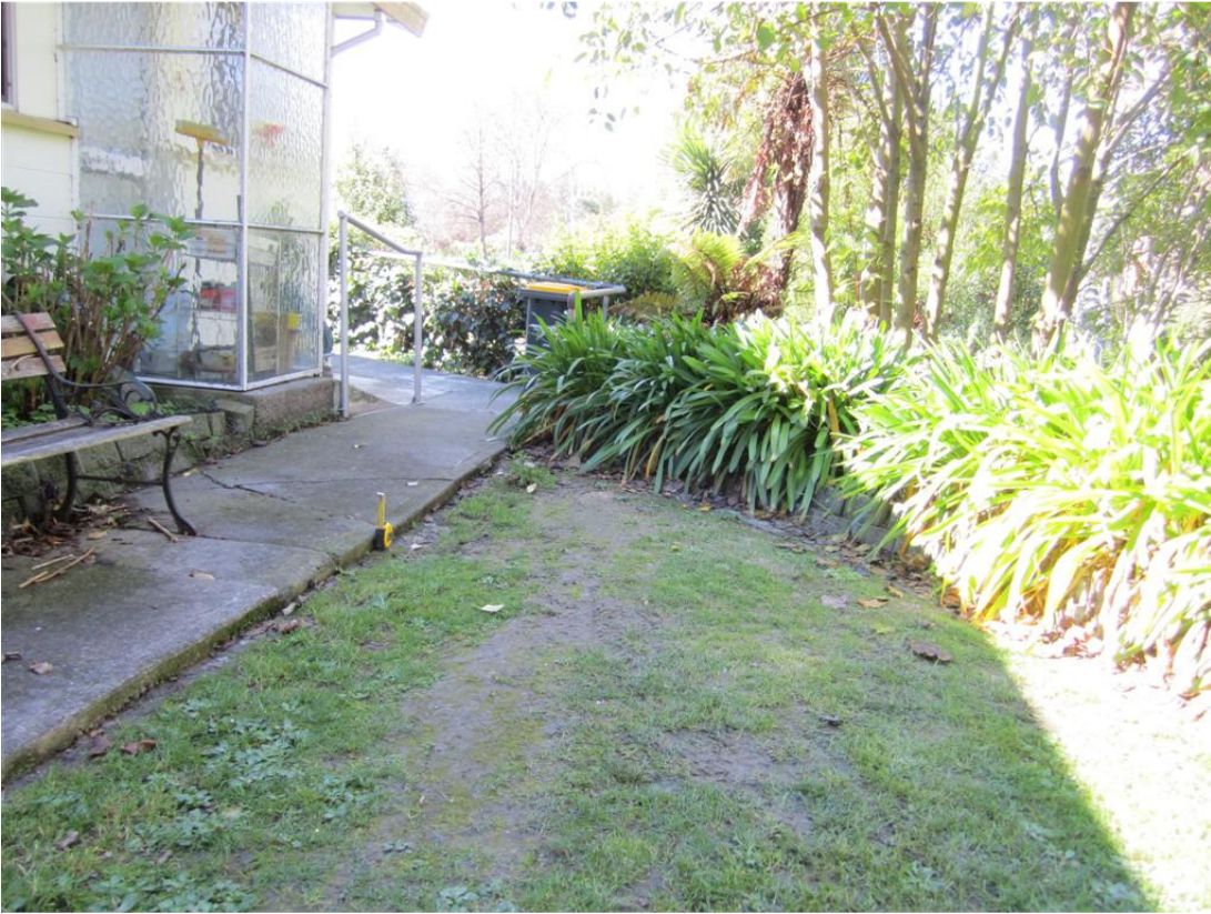
Photo 5: Difference in lawn and path levels on south side of unit 1 and 2
