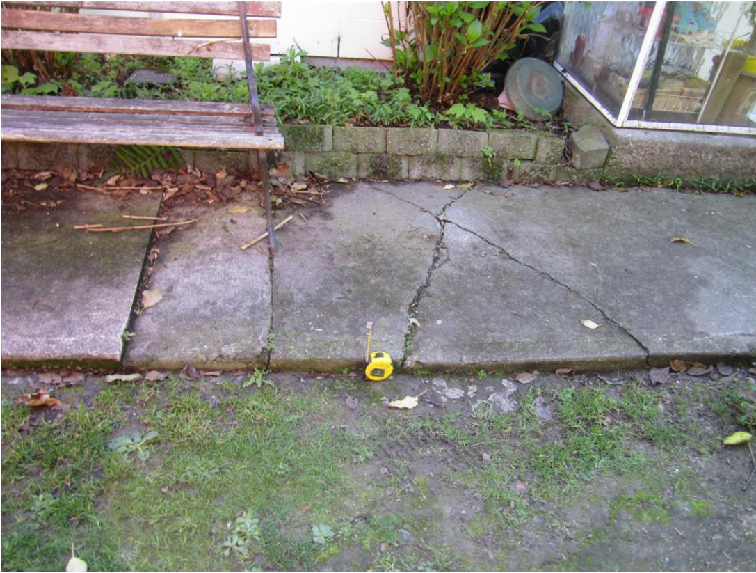
Photo 3: Cracks on path around south end of Units 1 to 2, with tilted blocks lining path.
