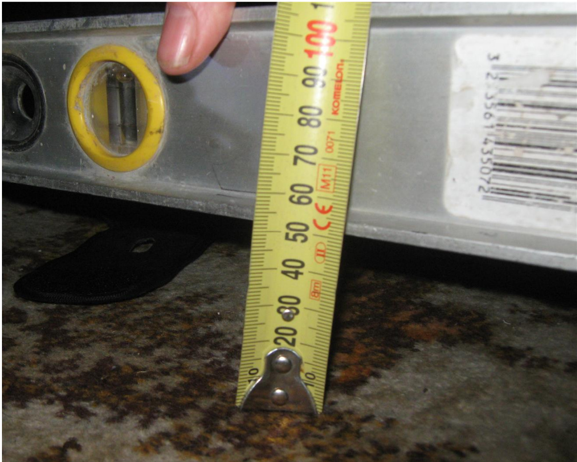
Photo 7: Ground floor settlement
