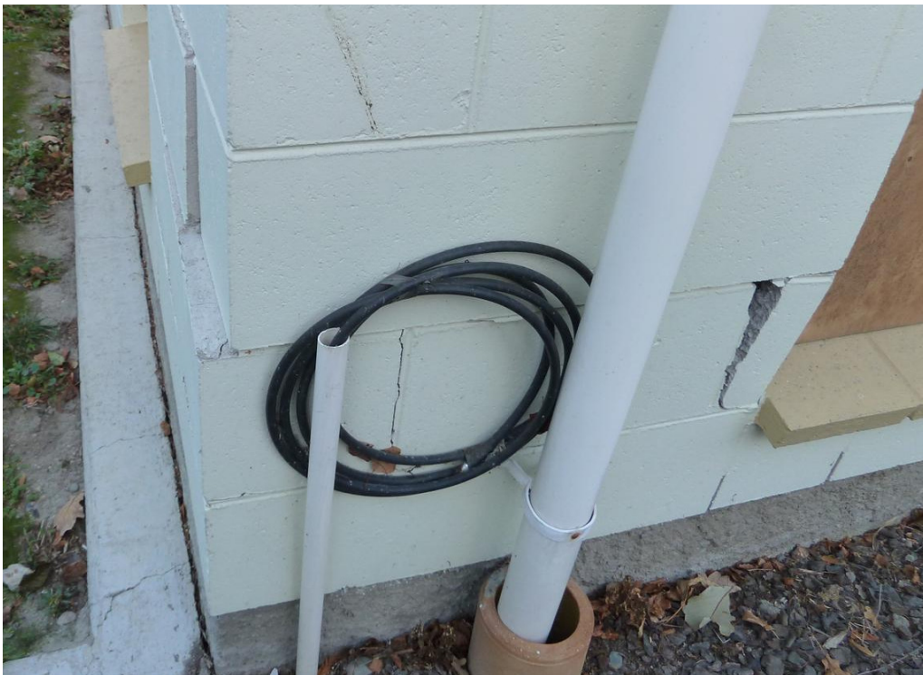
Photo 2: Cracking to block veneer
