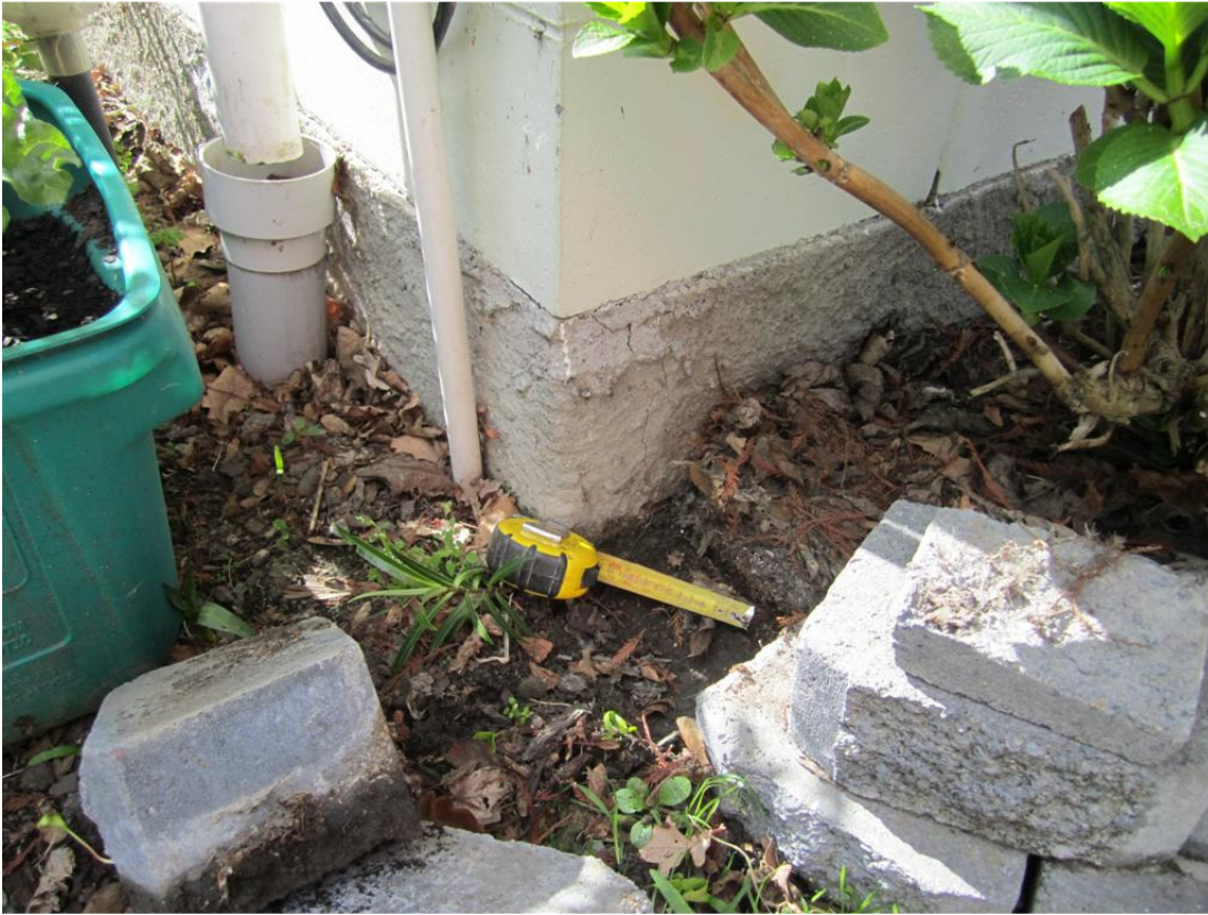
Photo 11: Hairline crack on south west corner of Units 3 to 8
