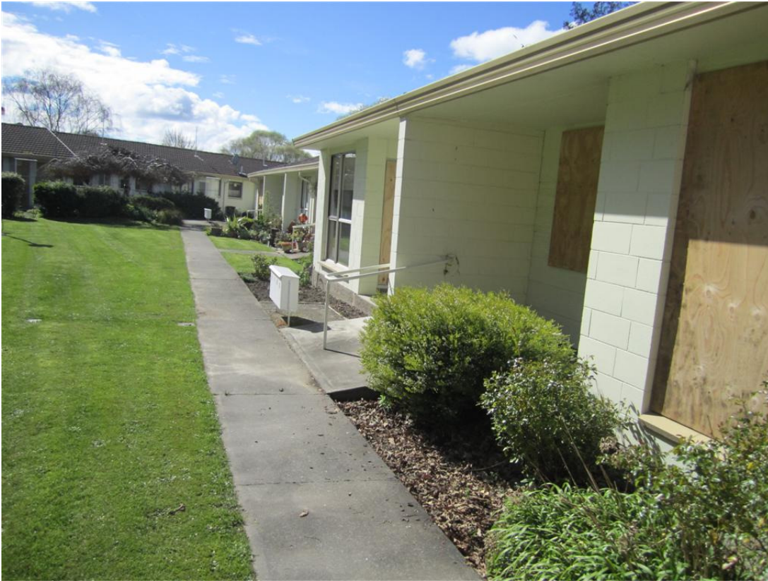
Photo 27: Lawn area on west of units 3-8, view to north. Units 3-8 on right of photo.
