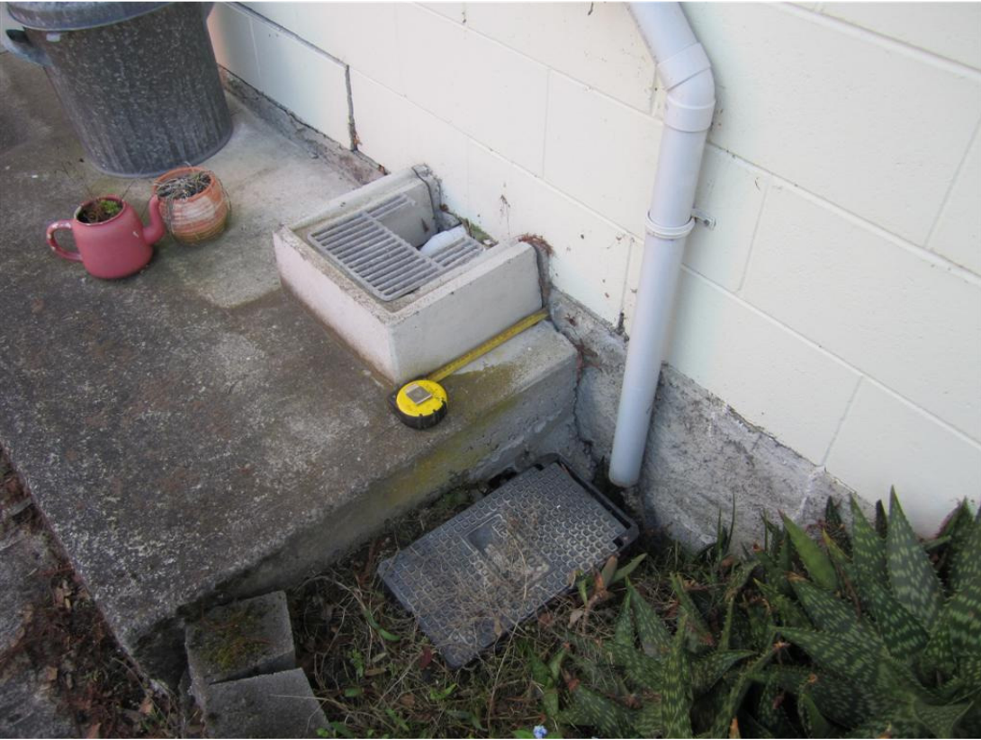
Photo 19: Slab separations on east end of Units 3 to 8
