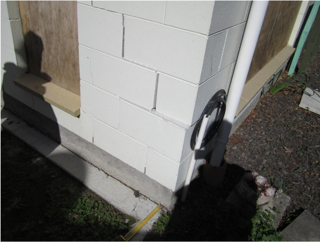
Photo 17: Separation on north west corner of unit 3 to 8
