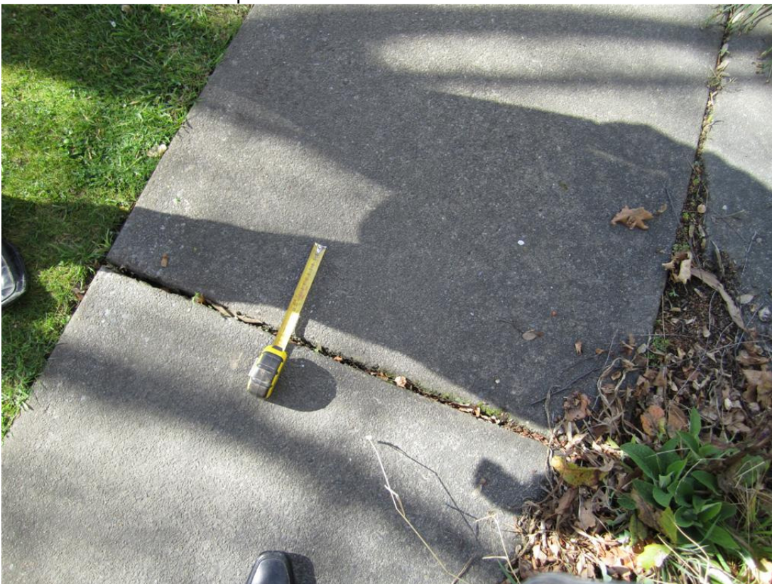
Photo 24: Separation of path slabs on north east end of Units 9 to 13
