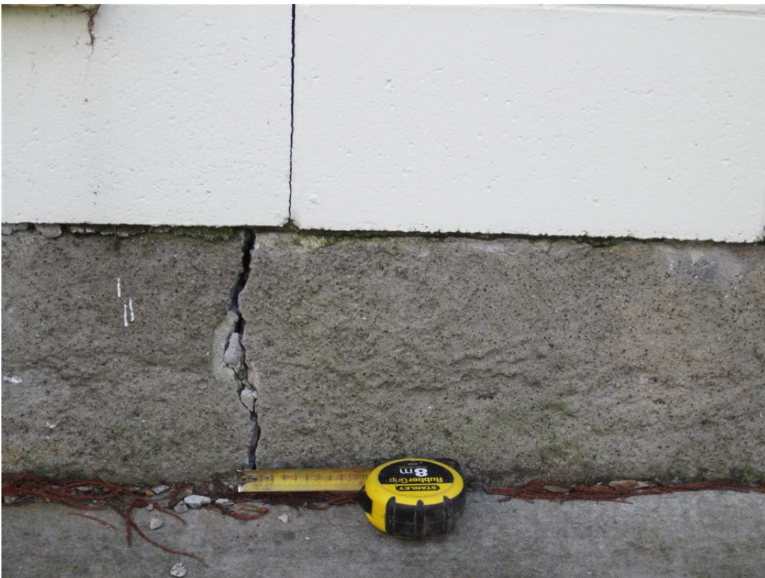
Photo 8: 6mm wide crack in foundation on southern end of Units 3 to 8
