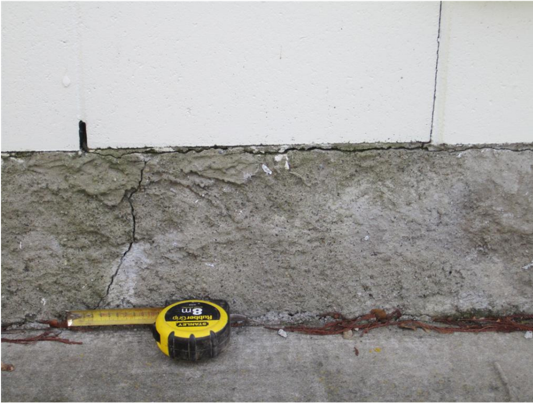
Photo 7: 2mm wide crack in foundation on southern end of Units 3 to 8
