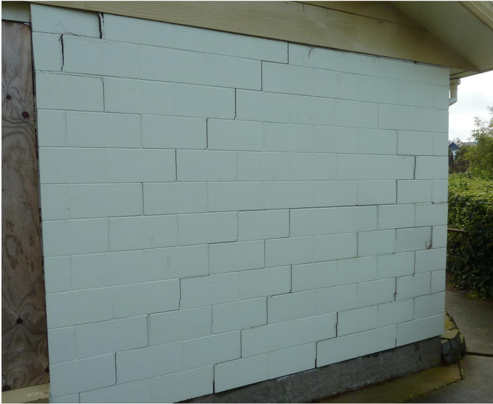
Photo 1: Cracking to block veneer
