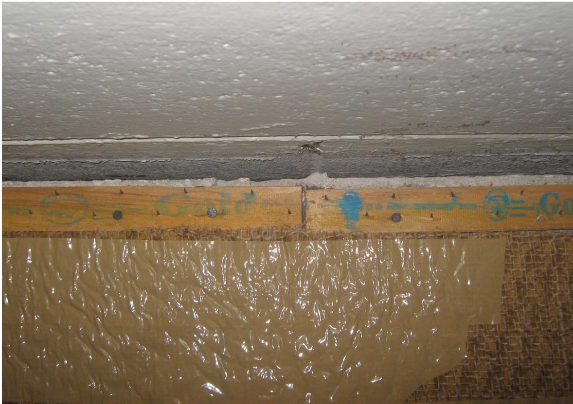
Photo 5: Ground slab separation from the foundation beam
