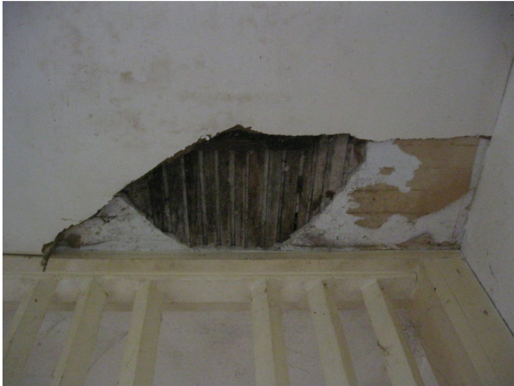
Photograph 5 Dilapidation in ceiling plaster and sarking .
