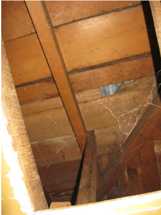
Photograph 3 Timber boards at roof level.
