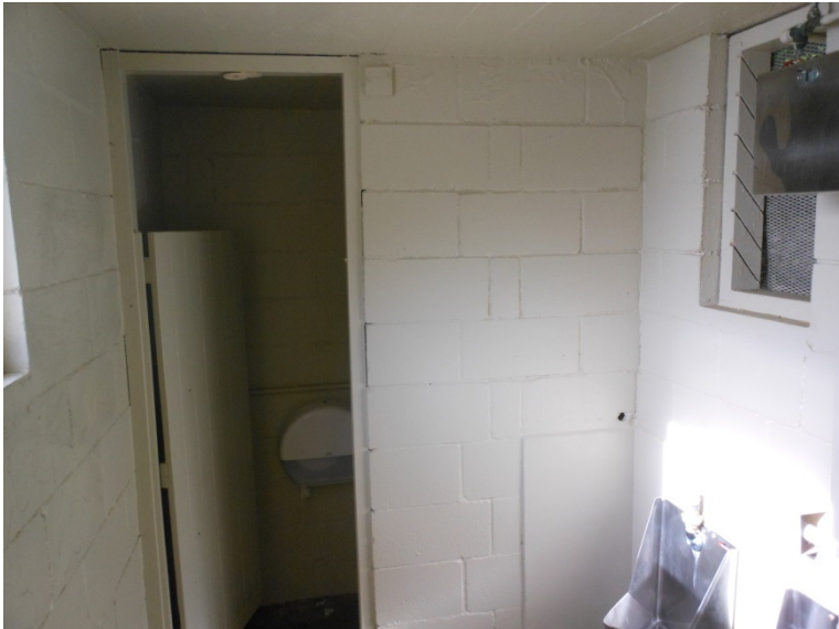
General view from inside the building.
