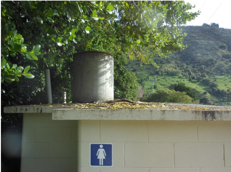
View on top of concrete roof showing water tank from southern side of building.
