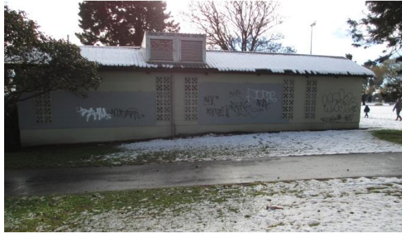
Southern elevation Linwood Park Pavilion and Toilets.
