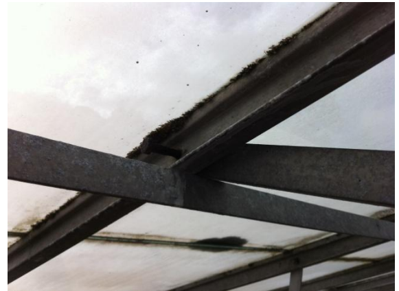
Photo 18: A loose bolt at an aluminium frame connection, mid-way along the west side of Glasshouse C
