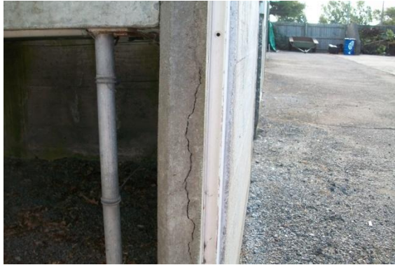
Photo 13: Typical spalling found on the vertical edge of the northern wall, adjacent to the door in Glasshouse B, C and E
