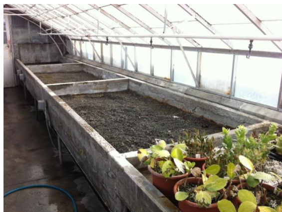
Photo 21: Concrete troughs at the south end of Glasshouse C
