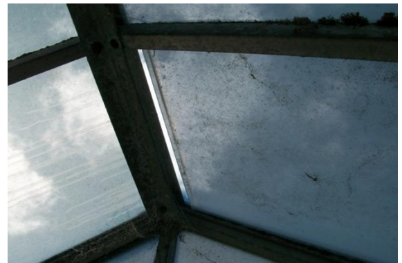
Photo 20: Glass pane which has shifted in Glasshouse A
