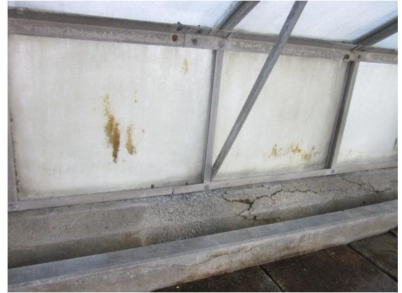
Photo 14: Fixings between sections of the aluminium frame structure
