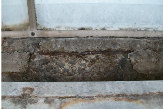
Photo 5: Typical spalling found at the top of the longitudinal concrete walls
