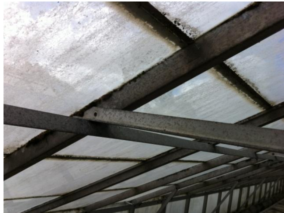
Photo 17: Bolt missing at an aluminium frame connection, mid-way along the east side of Glasshouse D
