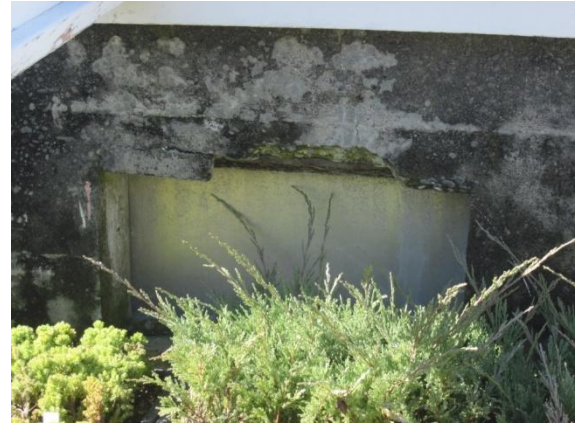
Photo 6: Spalling found adjacent to a vent, half way along the western wall of Glasshouse A
