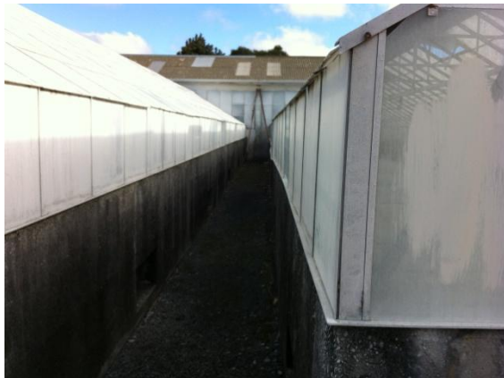
Photo 15: Lateral displacement mid-way along the east side of Glasshouse C
