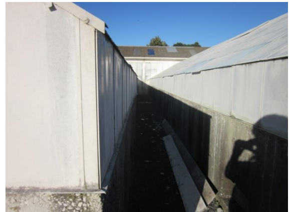
Photo 16: Lateral displacement mid-way along the west side of Glasshouse E
