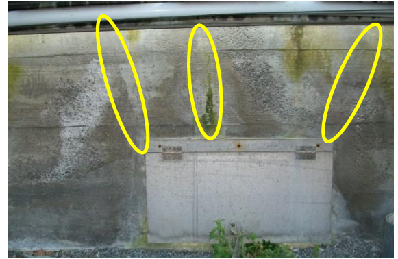
Photo 10: Typical vertical cracking found adjacent to vents in the longitudinal walls of Glasshouses A, C and E
