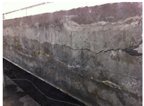
Photo 22: Detail of cracking to the sides of the concrete troughs in Glasshouse C
