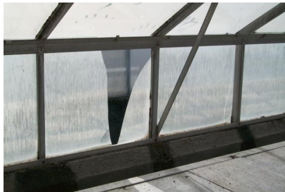
Photo 19: Broken glass pane at the south end of Glasshouse B
