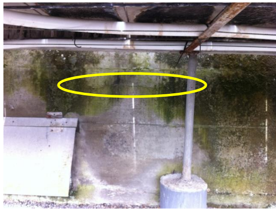
Photo 11: Horizontal cracking located approximately 350mm from the top of the eastern wall of Glasshouse B
