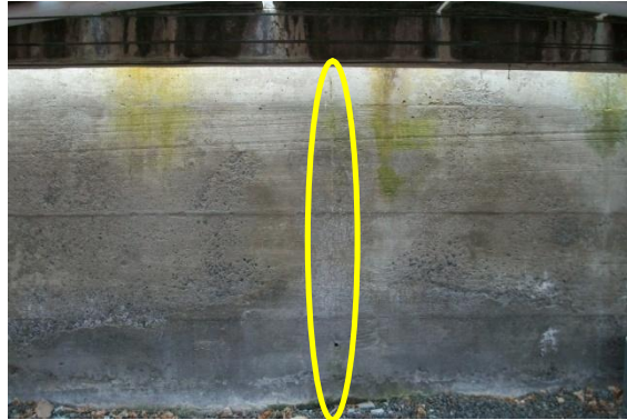
Photo 9: Typical vertical cracking found in the longitudinal walls of Glasshouses A, C and E
