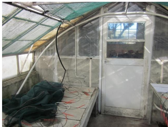
Photo 3: The south end of a glasshouse structure showing the connection to the wall of the Potting Shed (Building 4)
