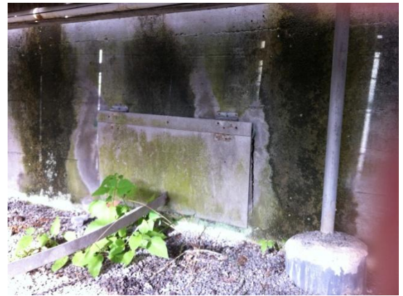
Photo 8: Spalling found adjacent to a vent half way along the eastern wall of Glasshouse C
