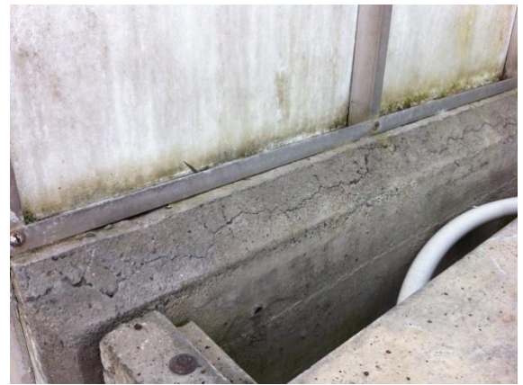
Photo 12: Typical cracking and spalling found at the top of the northern wall of Glasshouse A and D
