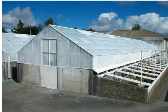
Photo 1: Exterior of a glasshouse structure
