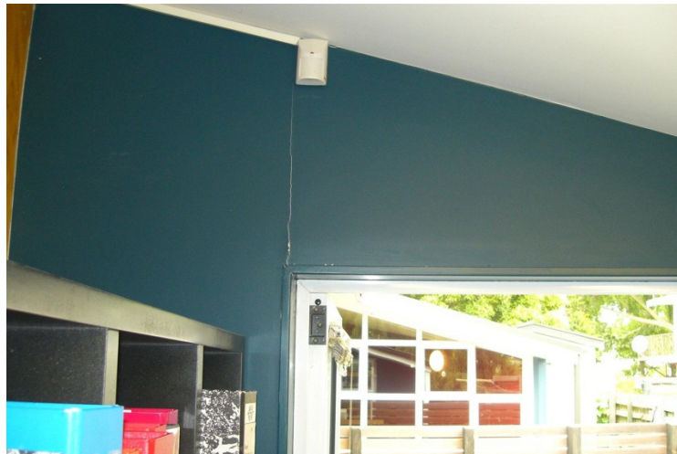
Photo 4 - Cracking to GIB lining in the staff room where the slab extension has moved
