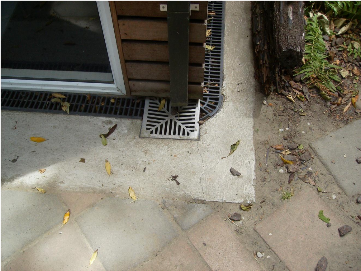
Photograph 3. Hairline crack in concrete encasement to slotted perimeter drain
