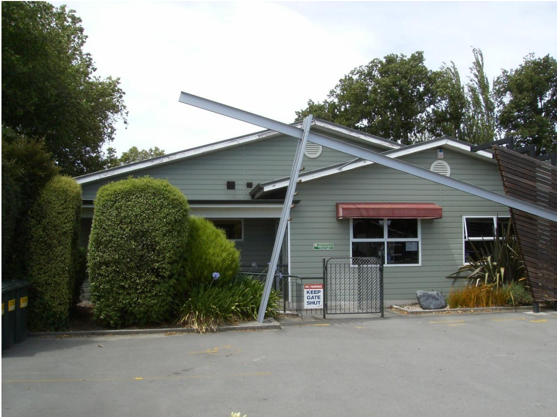
Photograph 1. Northern Elevation (Main entrance to building)
