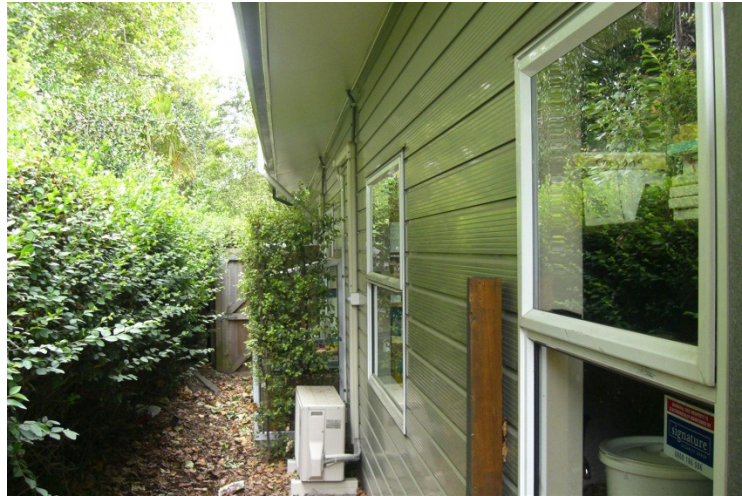
Photo 3 – Northern perimeter wall
