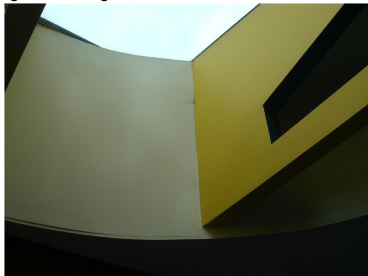
Photo 5 – Paint cracking in the circular skylight
