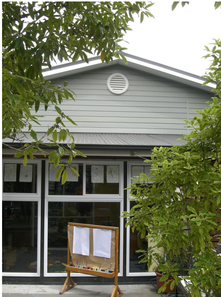
Photo 2 – Eastern perimeter wall
