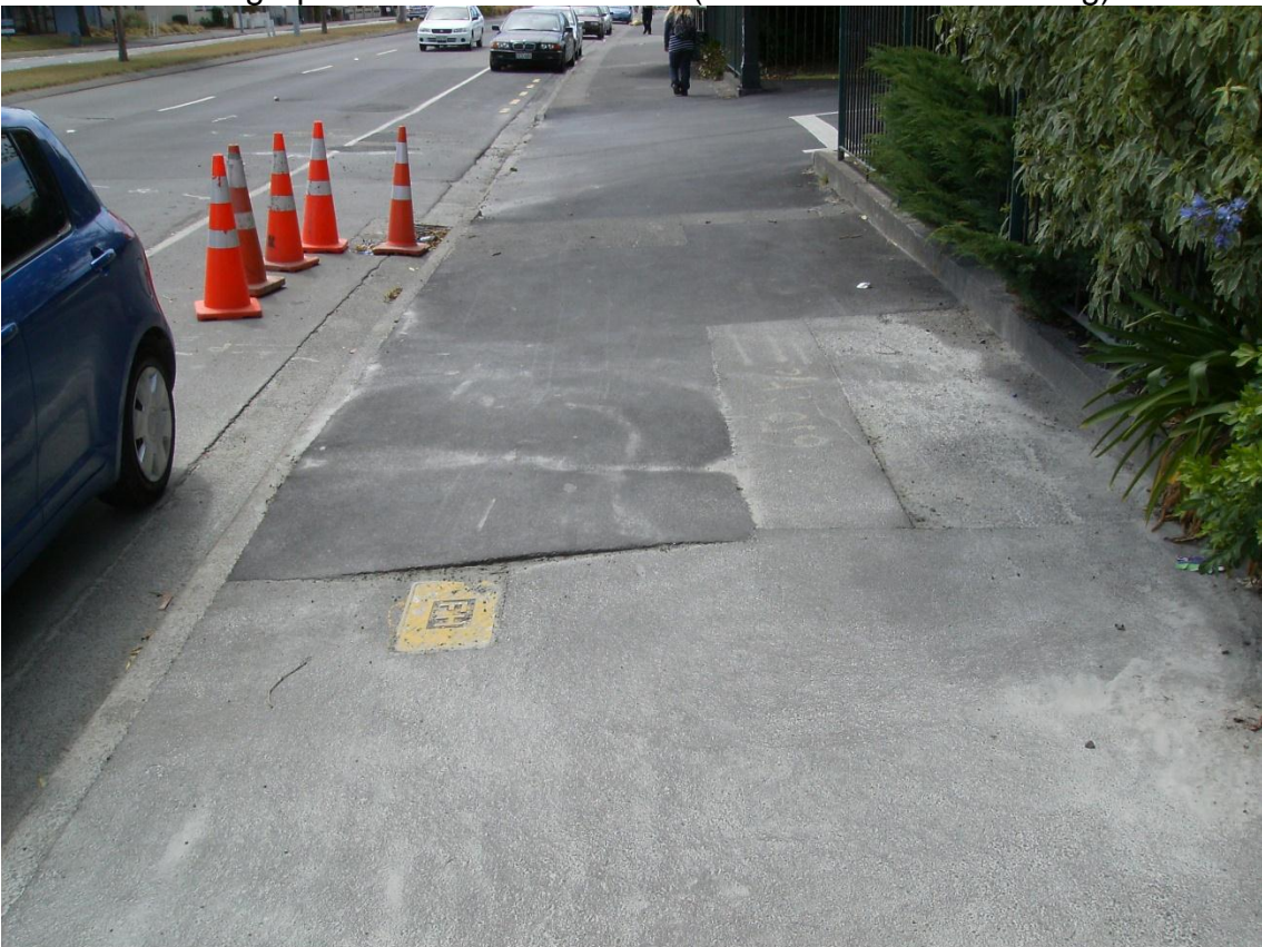
Photograph 2. 50mm undulations in asphalt footpath adjacent site on Aldwins Road
