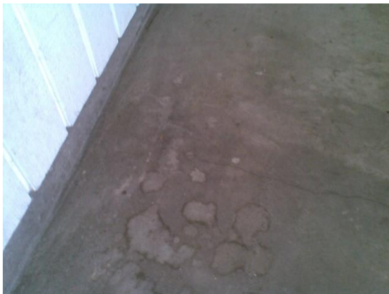
Photo 11: Floor slab cracking in the toilets
