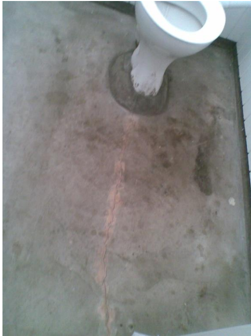
Photo 9: Typical cracking to slab foundation extending from floor penetration
