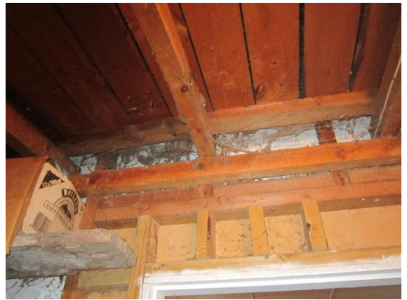
Photo 32: Timber framing of rear storage area of the hall
