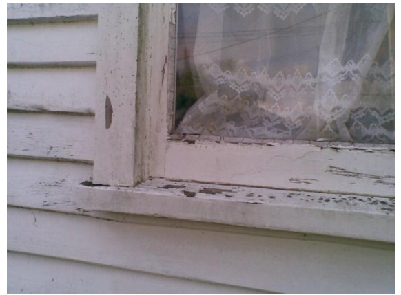
Photo 26: Timber rot around the window framing
