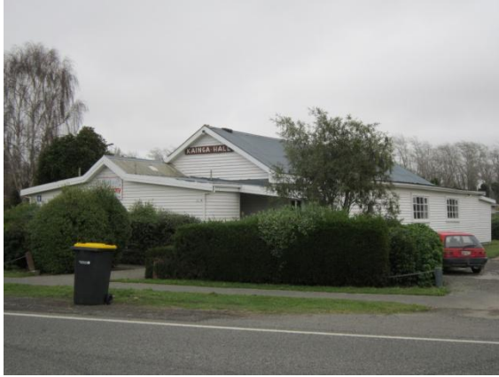
Photo 1: Photo looking south west at structure showing step between toilets front and Hall rear
