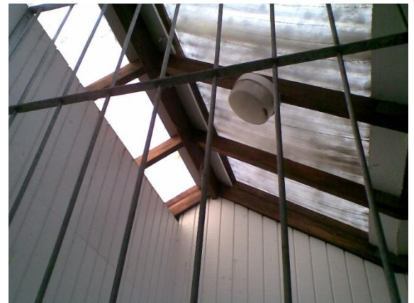
Photo 8: View of rafters and support beam at apex
