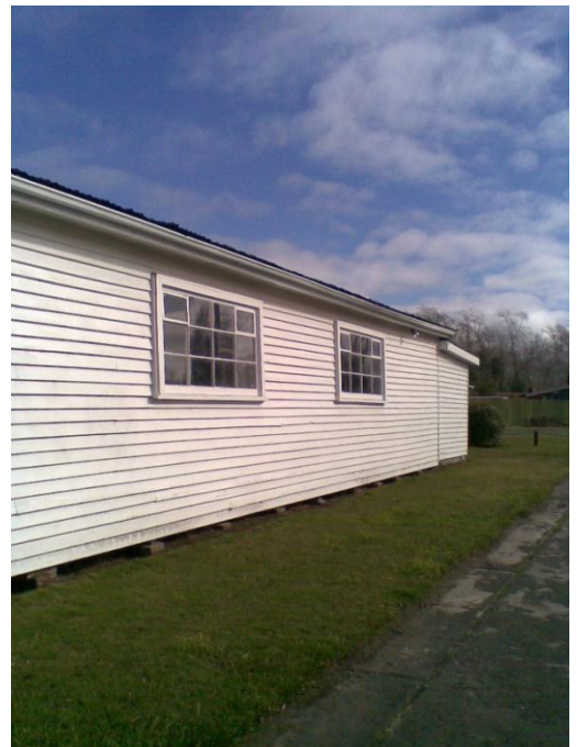
Photo 16: View west along the North wall of the building
