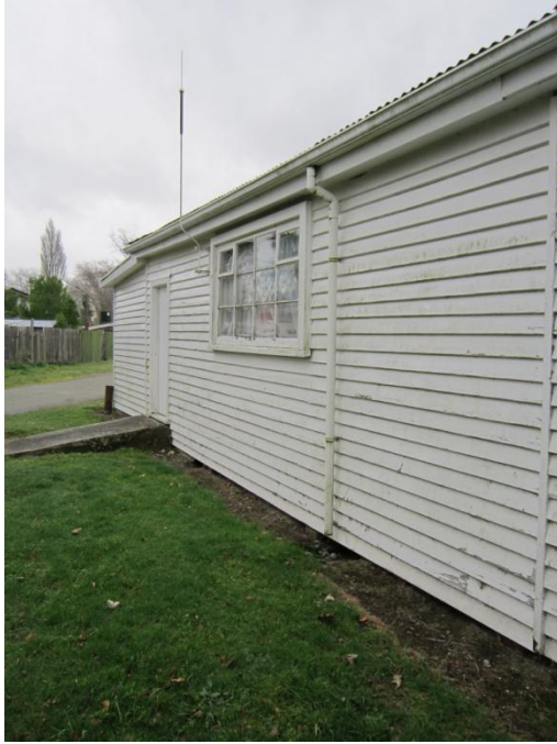
Photo 17: View west along the south wall of the building
