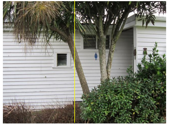
Photo 14: Building transition from hall to toilets
