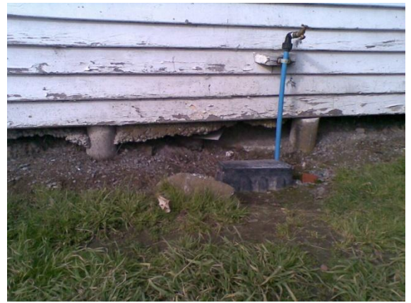
Photo 22: Slab on grade with perimeter concrete piles
