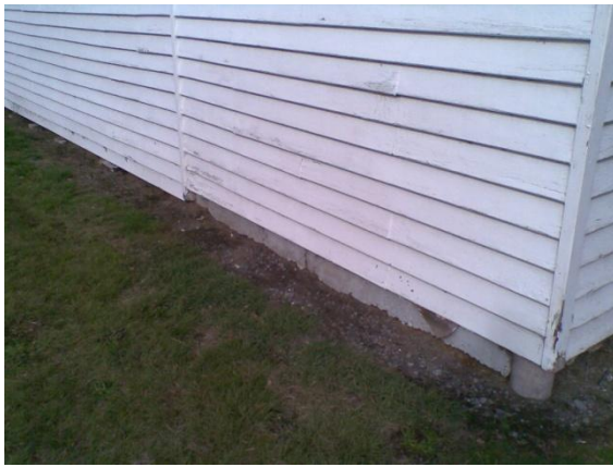
Photo 21: North west corner of the building addition where foundation transitions to slab on grade with perimeter concrete piles
