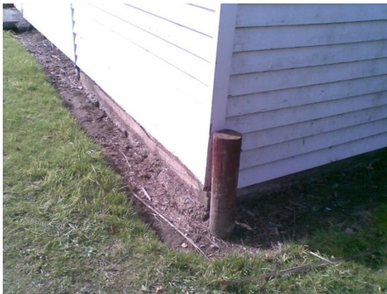
Photo 21: North west corner of the building addition where foundation transitions to slab on grade with perimeter concrete piles
