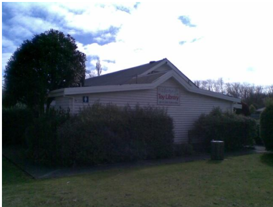
Photo 3: Roof extends at same level as the hall on south side of building
