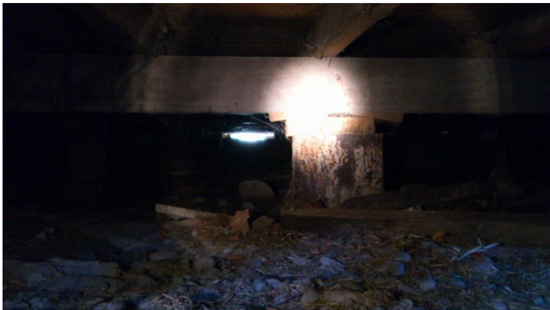
Photo 38: Shallow concrete pile encased with steel tin as formwork
