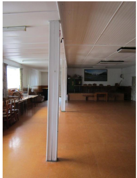
Photo 28: Internal timber columns noticeably out of plumb
