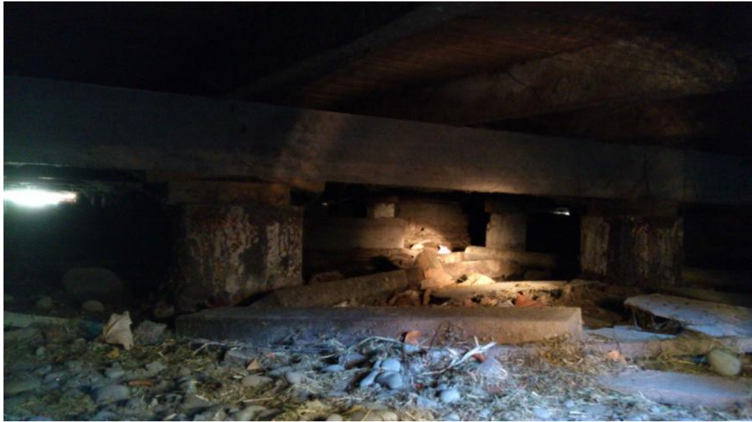
Photo 39: Foreground concrete piles, background piles and concrete pads
