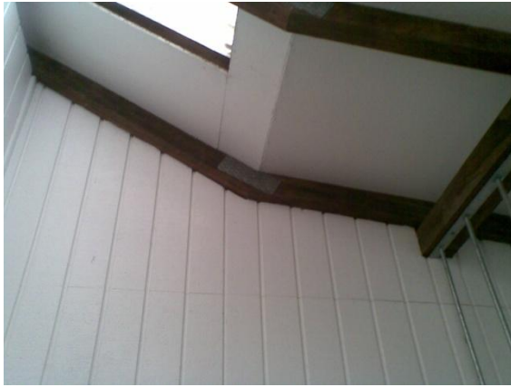
Photo 5: Support beam pictured (right) beneath light timber framed rafters
