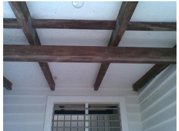
Photo 4: Timber framing of timber eave typical of roof framing within the public toilets. 100mm x 50mm beams on timber bearing beams at eaves roof pitch transition and apex
