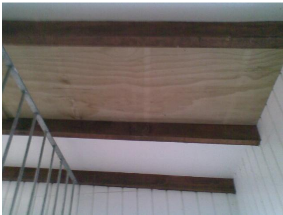
Photo 7: Replacement of roof panel or skylight with plywood
