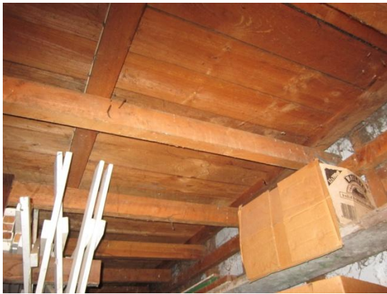
Photo 31: Timber framing of rear storage area of the hall
