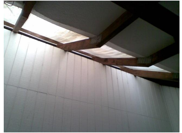
Photo 6: View looking at toilet apex
