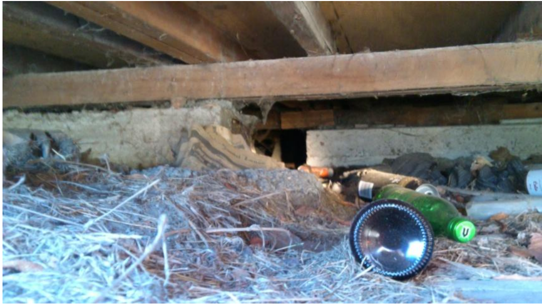
Photo 35: Pad foundation rows along the lines of the bearers
