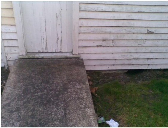
Photo 25: South west corner of the original hall perimeter foundations are concrete pad
