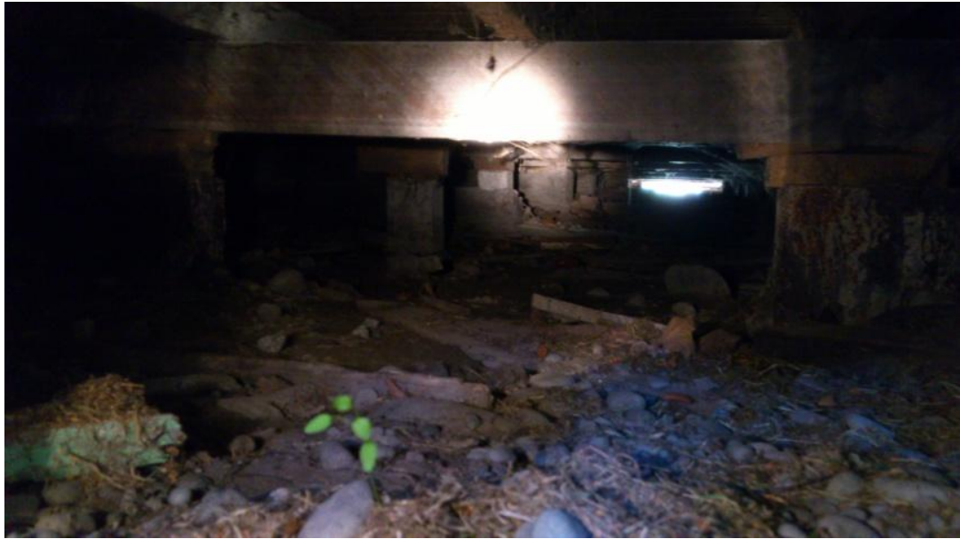
Photo 37: Subfloor looking north beneath the building. Combination of discrete piles and concrete pads
