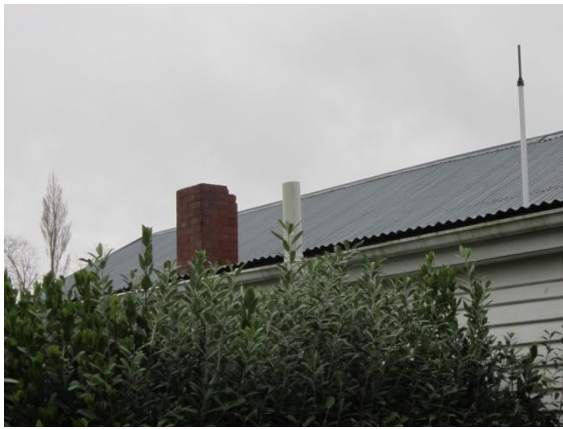
Photo 13: Chimney over the Kainga hall which lost an estimated 400mm of height
