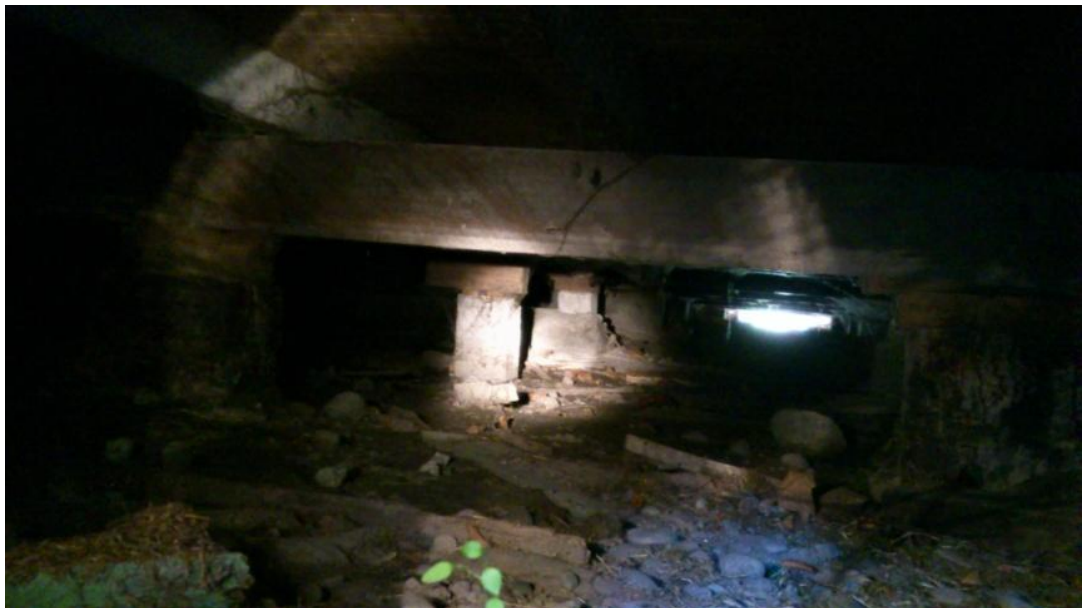
Photo 36: Subfloor looking north beneath the building. Combination of discrete piles and concrete pads
