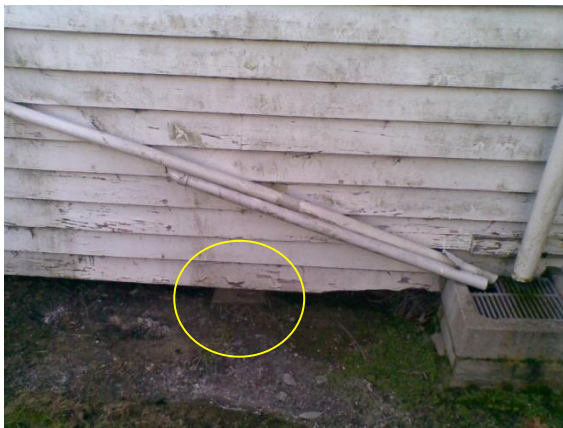
Photo 25: South west corner of the original hall perimeter foundations are concrete pad
