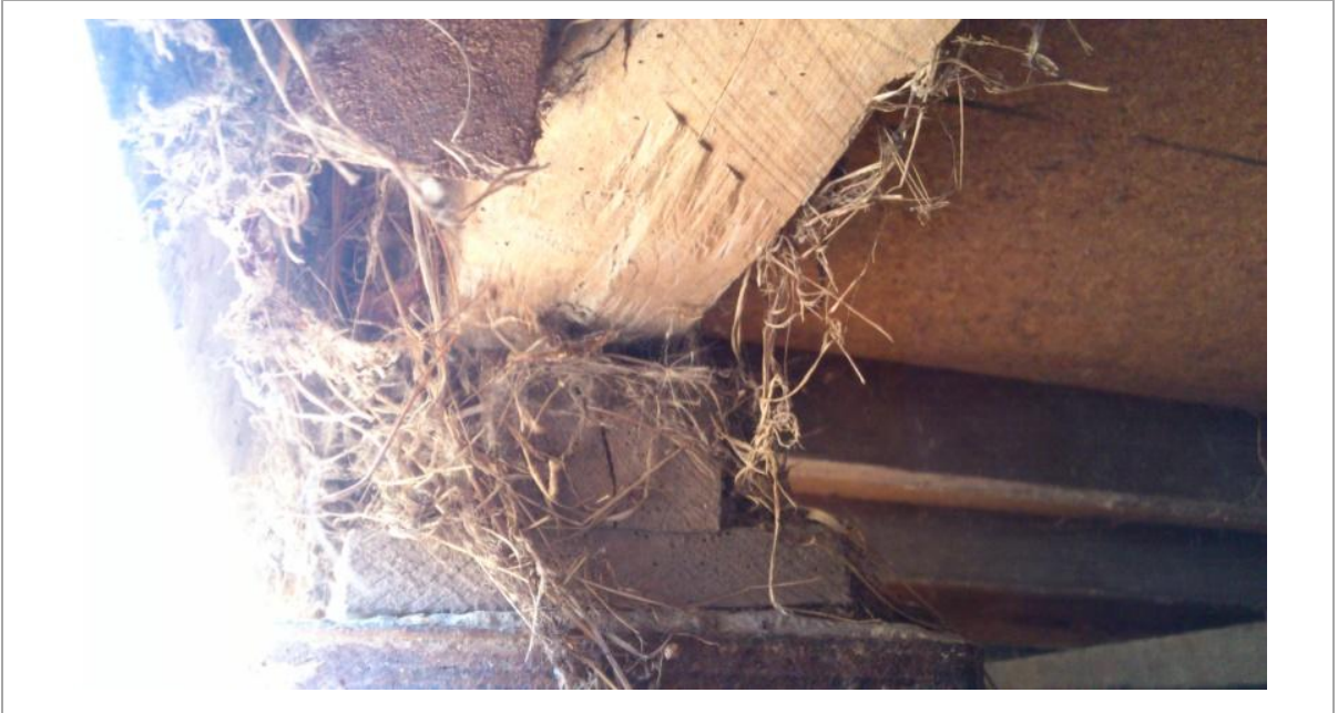
Photo 33: Timber connection between bearer and top of concrete pile
