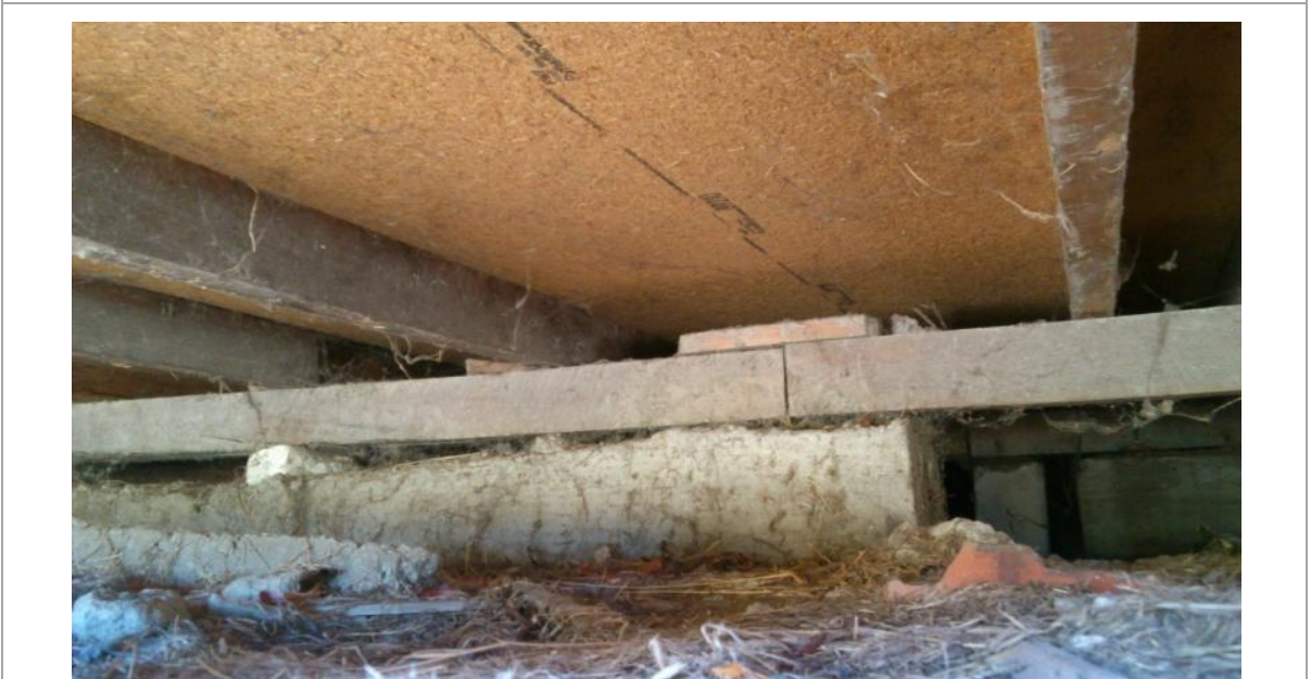
Photo 34: Particle board floor on timber joists and bearers supported by concrete pad foundations. Connection between bearer and pad could not be verified. Background - internal discrete pile supporting bearer and pad foundations
