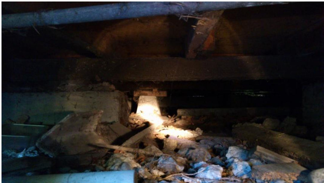
Photo 40: 200x200mm square concrete piles beneath the south east of the building
