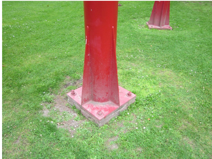
Figure 9 – Typical Column Base at Hydroslide Columns
