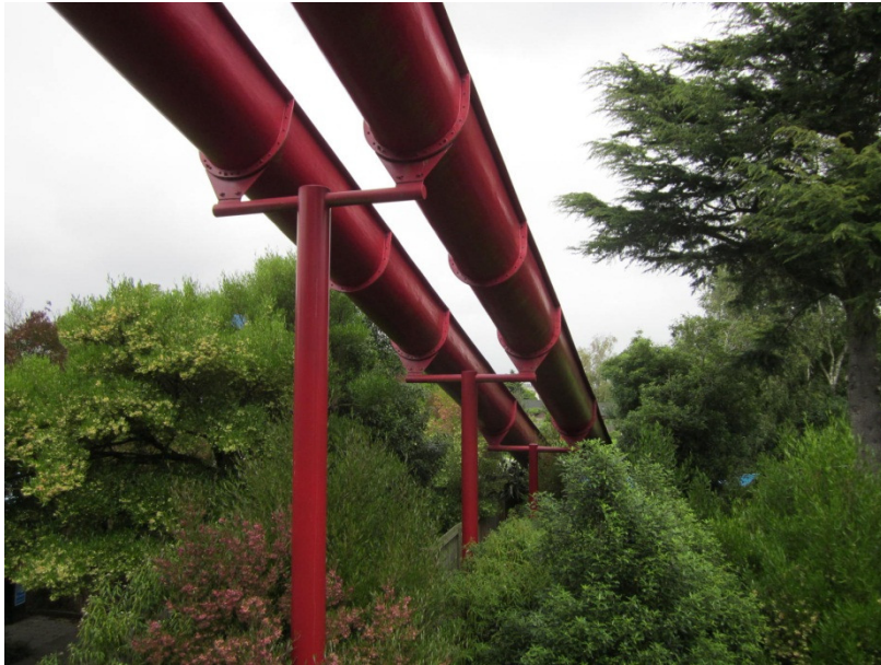
Figure 7 – Typical Column, Slide Fixing and Slide at Straight Hydroslides
