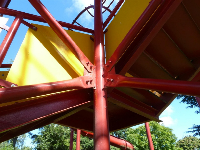
Figure 4 – Typical Mid-Column Height Pipe Brace-to-Column Connection
