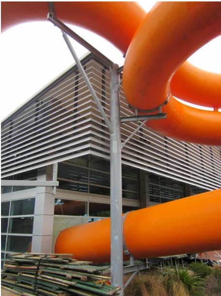
Figure 16 – Column, Slide Fixing and Slide at Indoor Hydroslide
