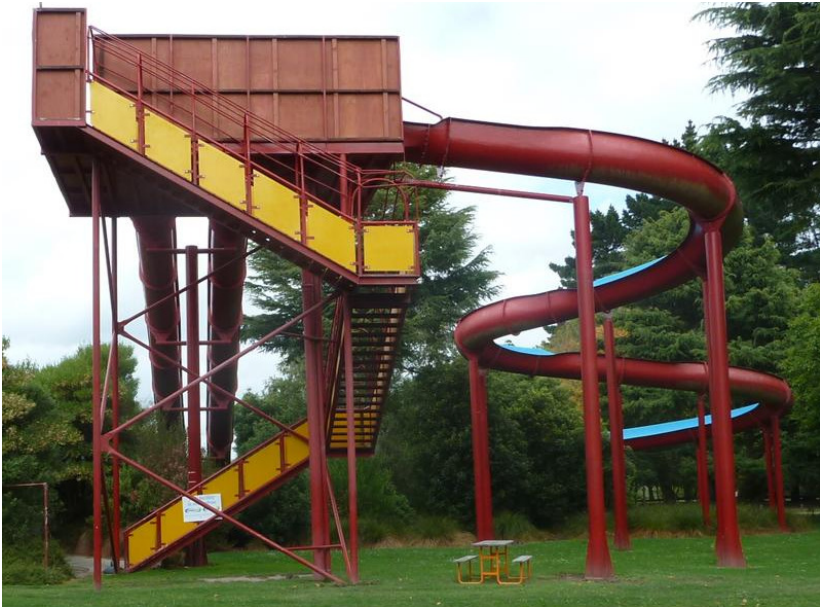
Figure 2 – Outdoor Hydroslide Platform Structure – Looking South
