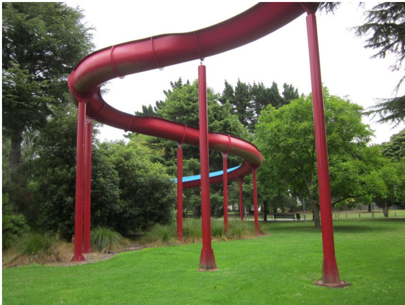
Figure 8 – Typical Column, Slide Fixing and Slide at Curved Hydroslide
