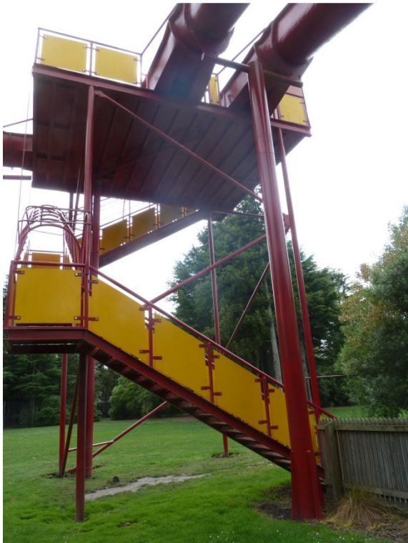
Figure 1 – Outdoor Hydroslide Platform Structure – Looking North
