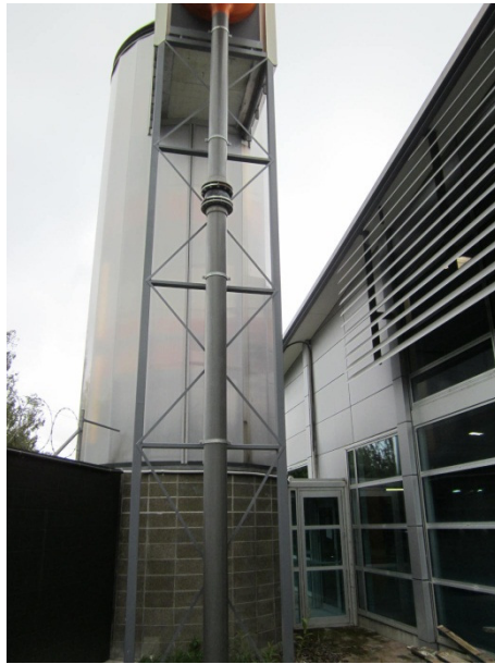
Figure 13 – Indoor Hydroslide Stair Tower and Braced Frame at Mouth of Slide
