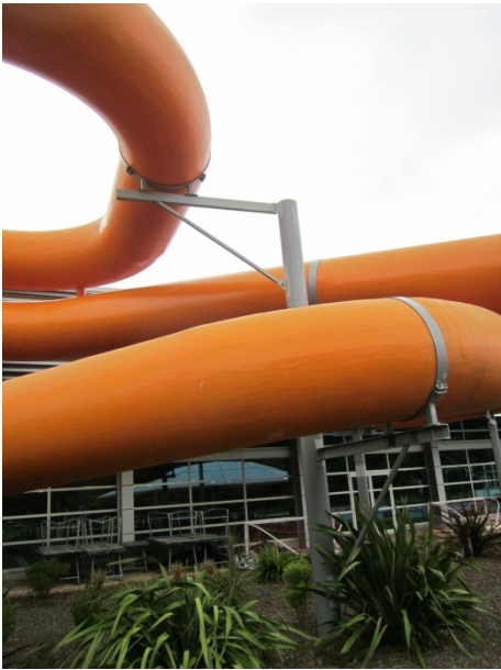
Figure 17 – Column, Slide Fixing and Slide at Indoor Hydroslide
