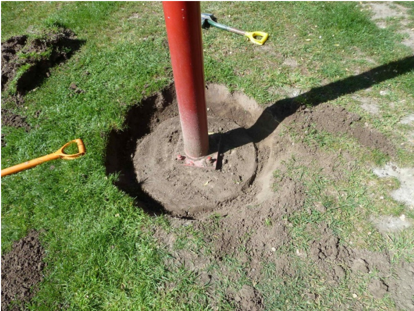
Figure 6 – Platform Column Base Connection
