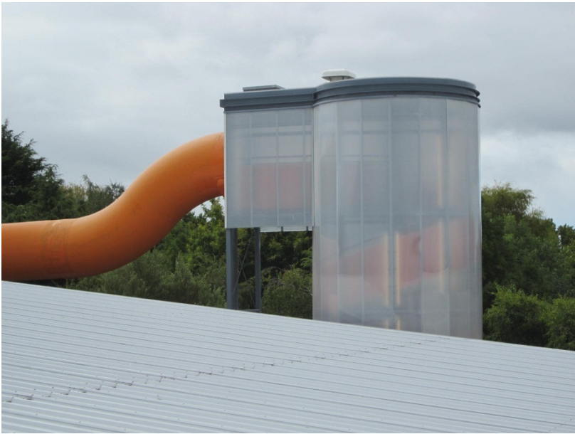
Figure 15 – Top of Stair Tower and Mouth of Hydroslide
