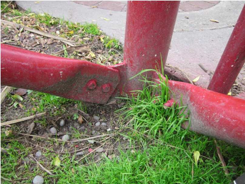
Figure 5 – Typical Pipe Brace-to-Column Connection at Platform Column Base
