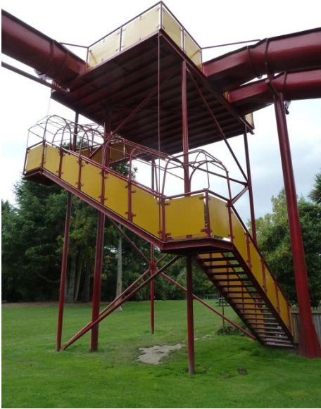
Figure 3 – Outdoor Hydroslide Platform Structure – Looking Northeast
