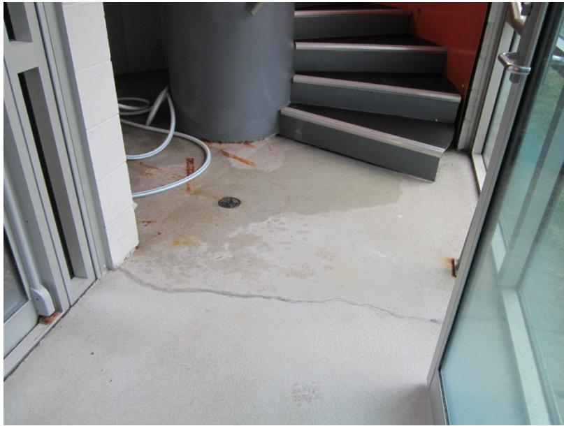
Figure 19 – Interior View of Stair Tower Base with Cracked Slab-on-grade (Evidence of Foundation Rocking)
