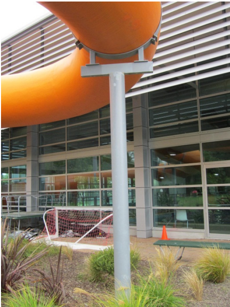
Figure 18 – Column, Slide Fixing and Slide at Indoor Hydroslide
