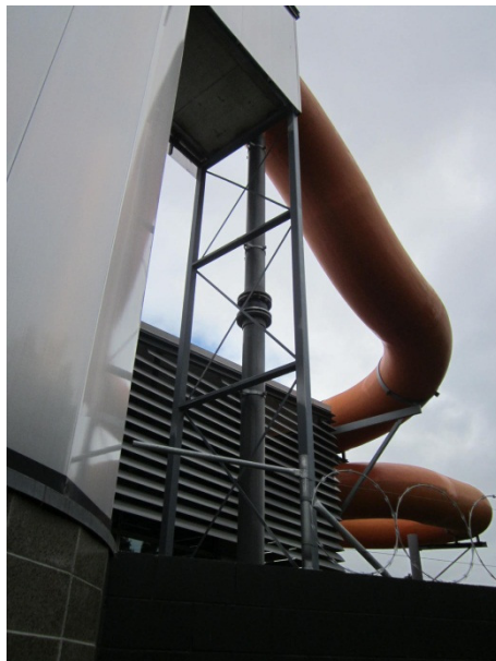
Figure 14 – Braced Frame Supporting Mouth of Slide and Stair Landing
