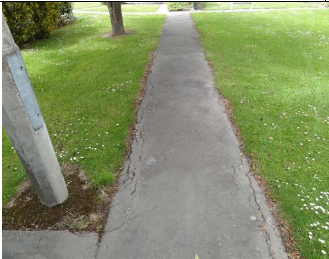
Figure 7 Cracking in footpath through the lawn
