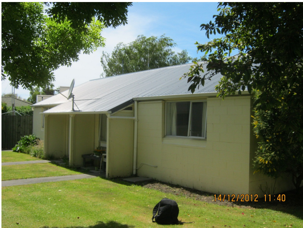
Photo 2: General configuration of the single storey buildings
