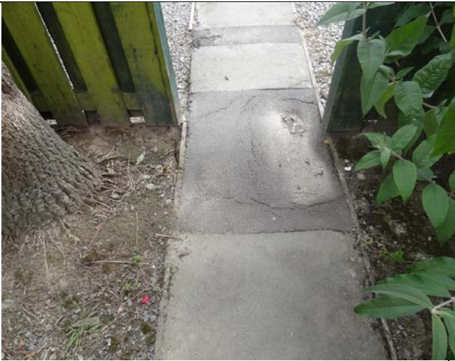
Figure 9 Local depression in footpath
