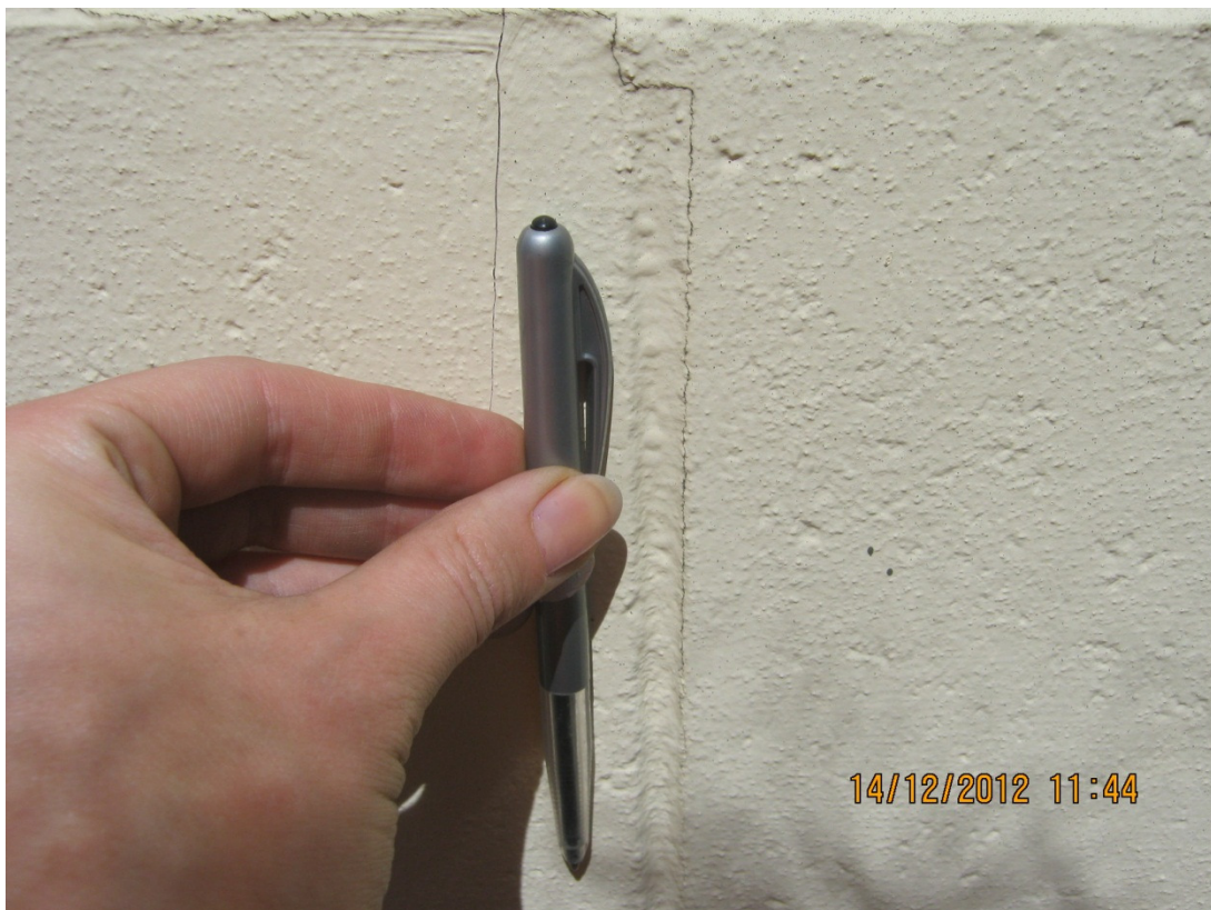
Photo 4: Cracking of the block veneer
