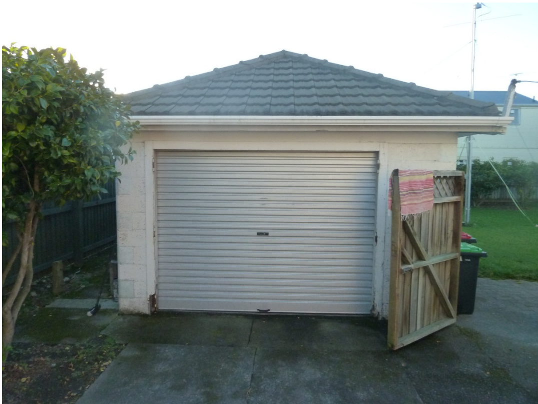
Photo 12: General configuration of the garage at 407 Innes Road
