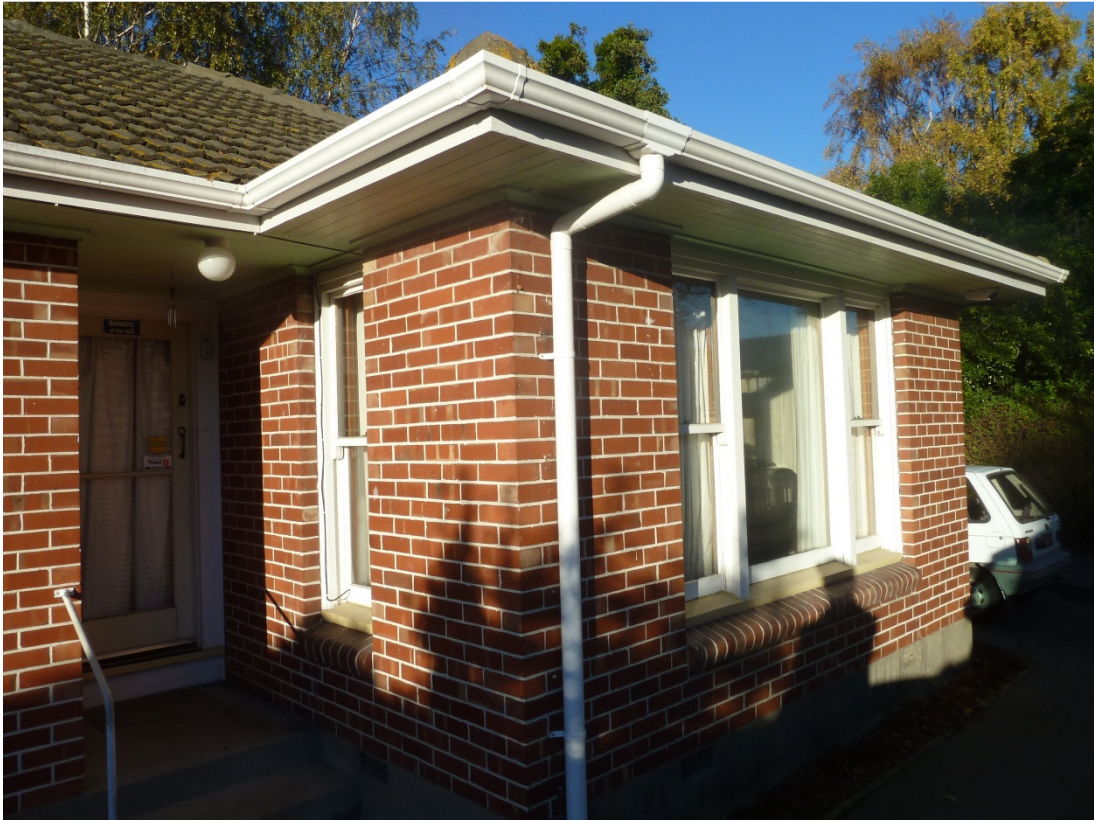
Photo 9: General configuration of the house at 407 Innes Road
