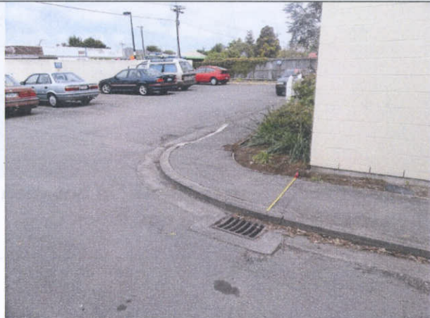
Figure 3 Cracks in footpath, same location as figure 3
