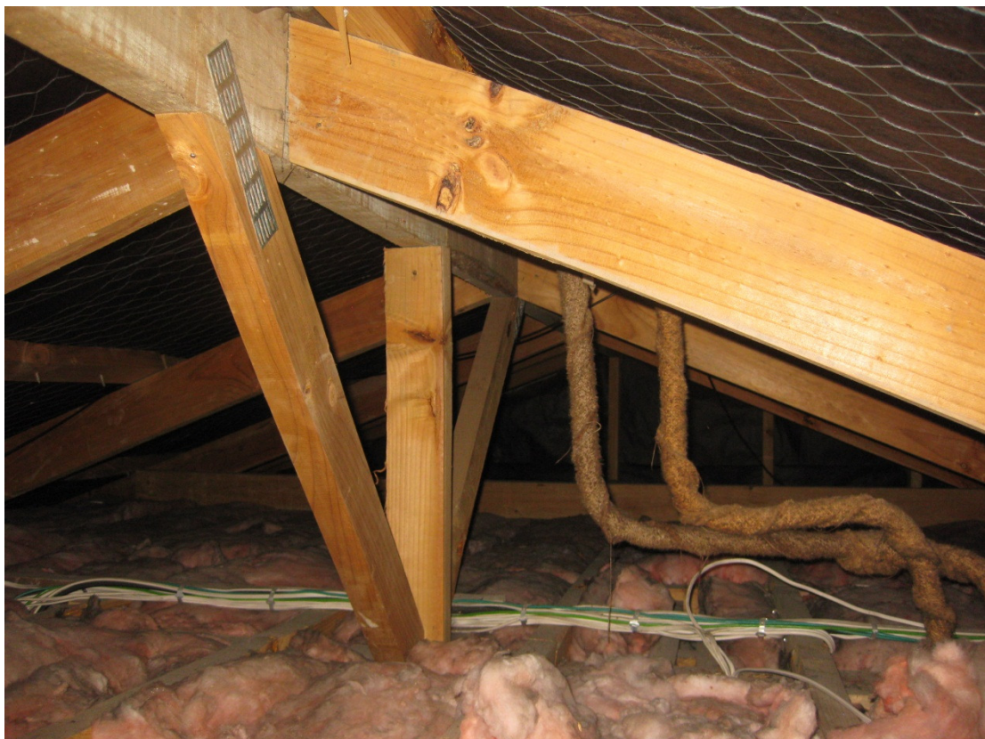
Photo 6: Roof structure without bracings
