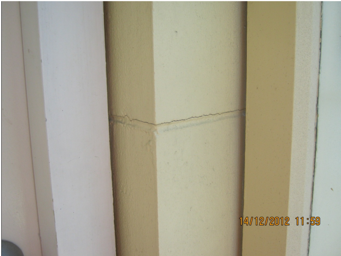
Photo 5: Cracking of the block veneer
