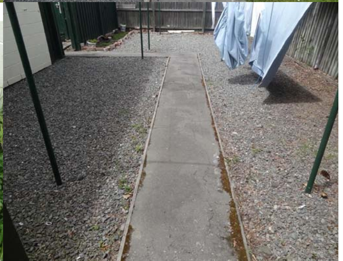
Figure 13 Cracks in footpath, through the drying area, next to unit 23/30 block E
