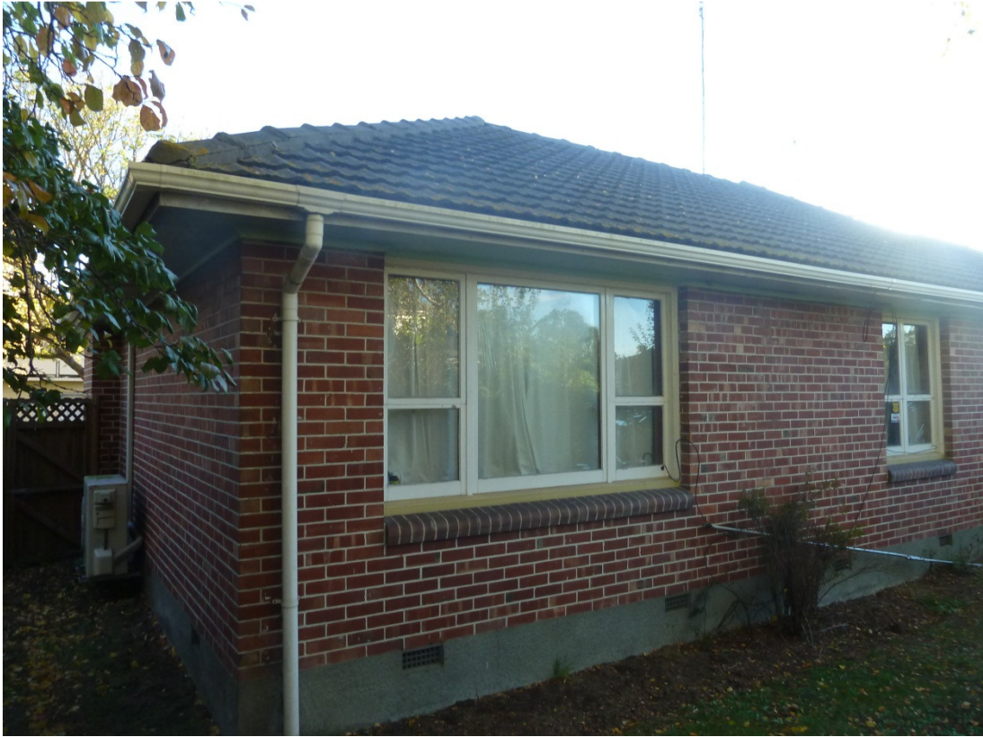
Photo 11: General configuration of the house at 407 Innes Road
