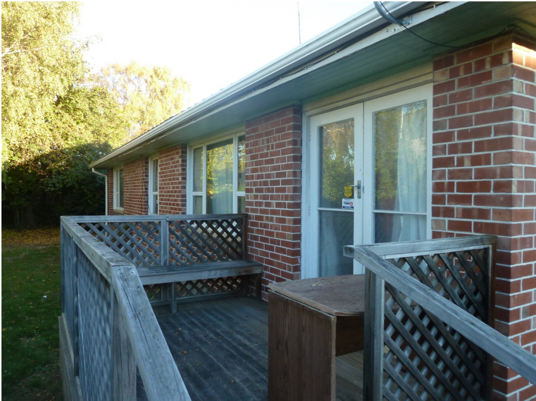
Photo 10: General configuration of the house at 407 Innes Road
