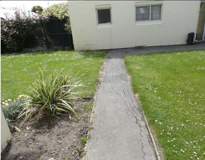
Figure 11 Typical cracking in footpaths
