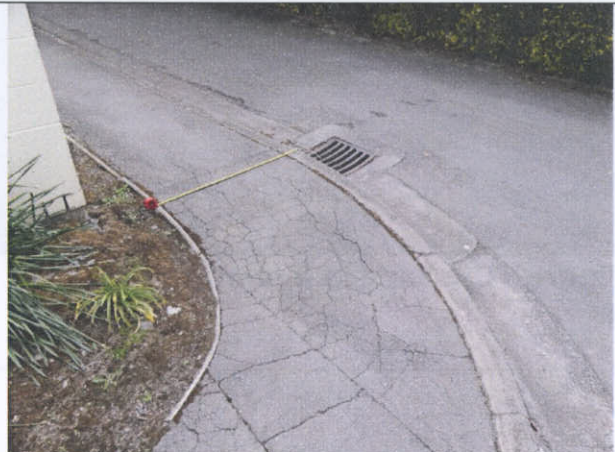
Figure 4 Detail of various cracks and settlement near gully pot, same location as (figure 3)
