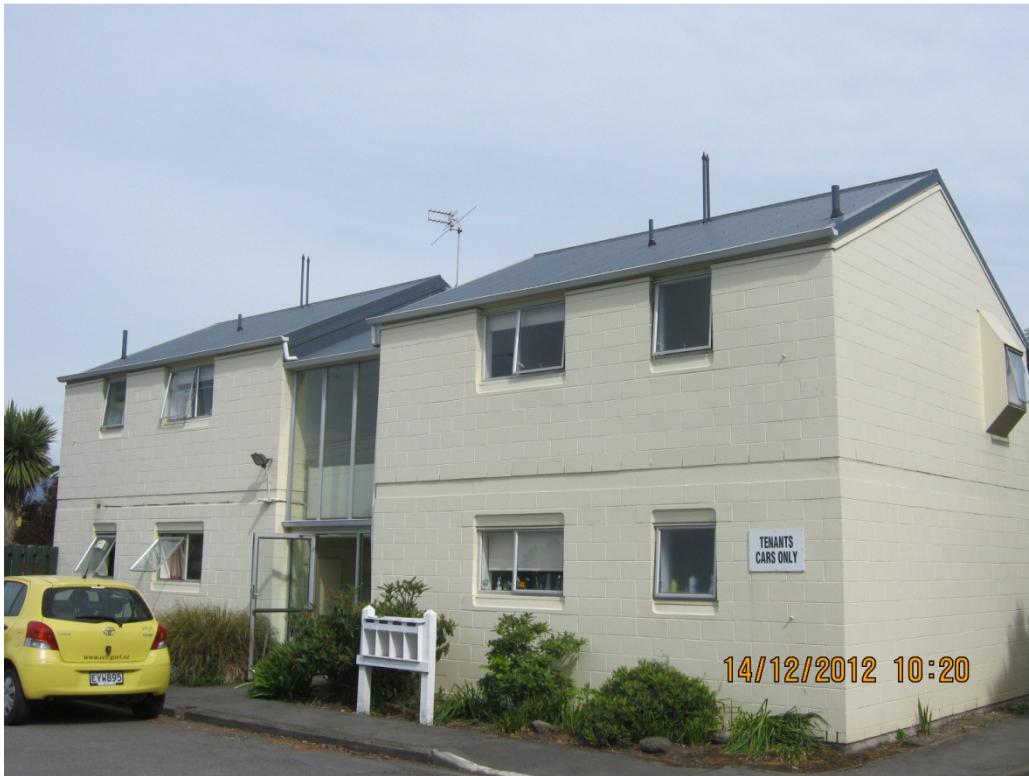
Photo 1: General configuration of the two storey buildings
