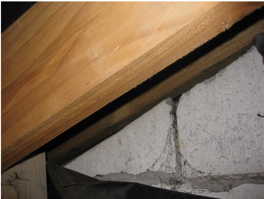
Photo 8: Roof structure without bracings
