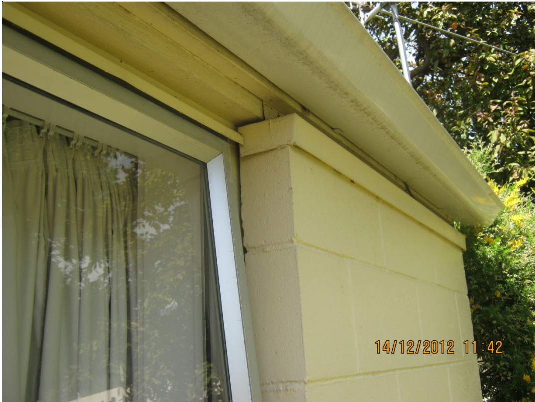
Photo 3: Connection of the block veneer to the roof structure
