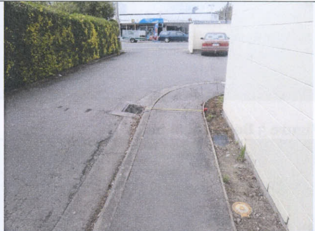
Figure 2 Footpath next to unit 2/7 Block A
