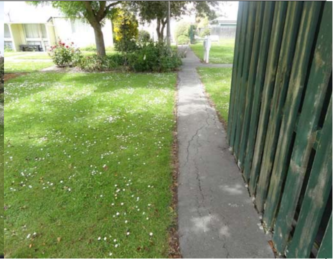
Figure 6 Cracking in footpath next to block E.
