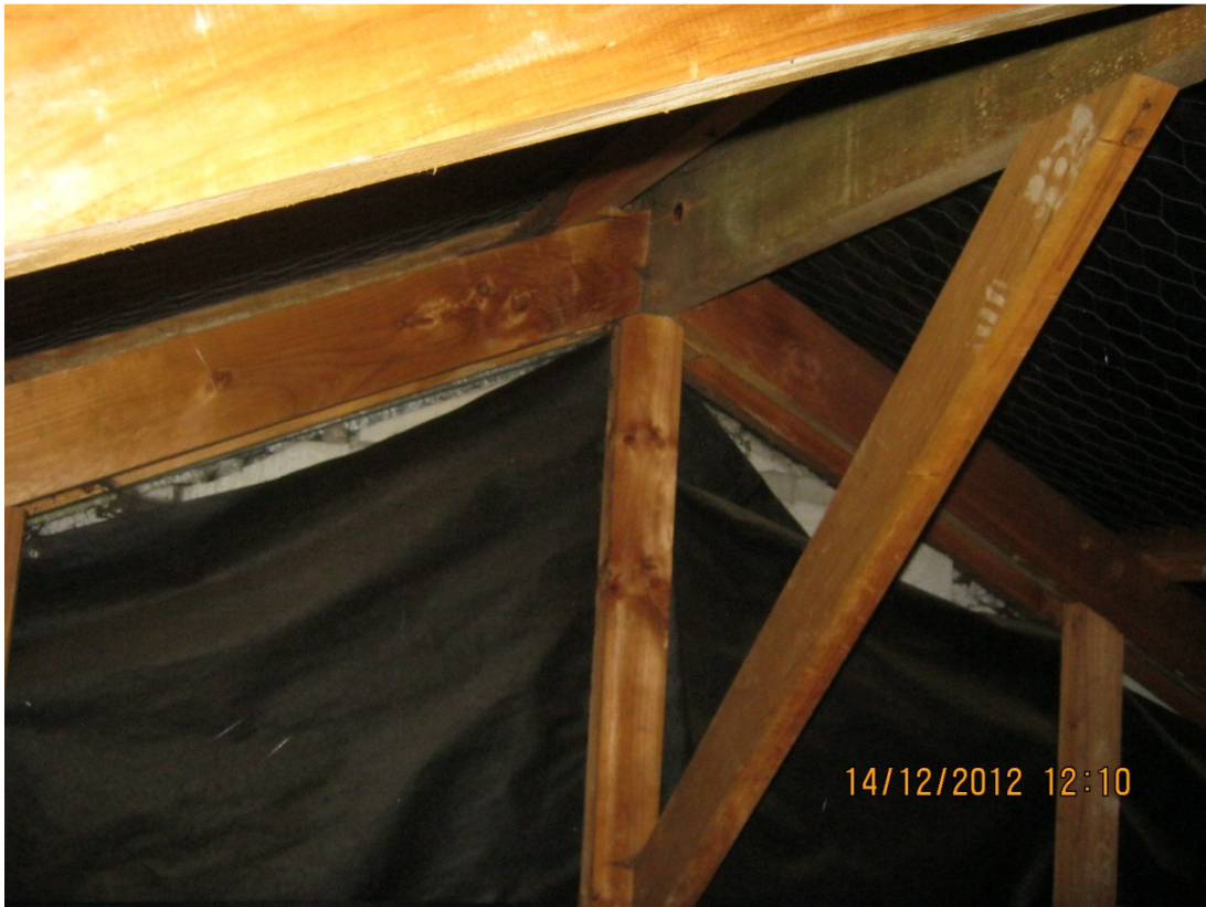
Photo 7: Roof structure without bracings
