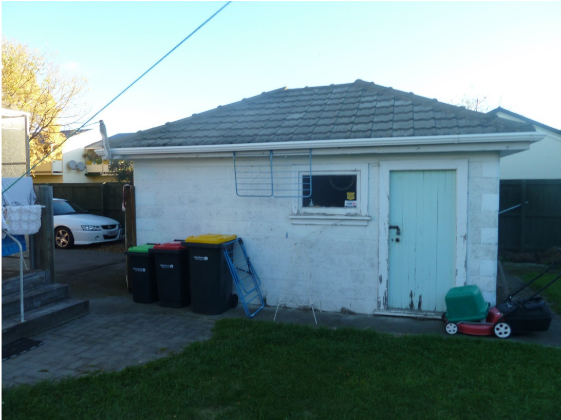
Photo 13: General configuration of the garage at 407 Innes Road
