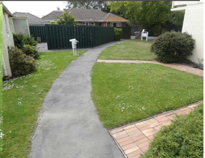
Figure 8 Cracking in footpath, in between block B unit 11/12 (right) and block C, unit 13/14 (left)
