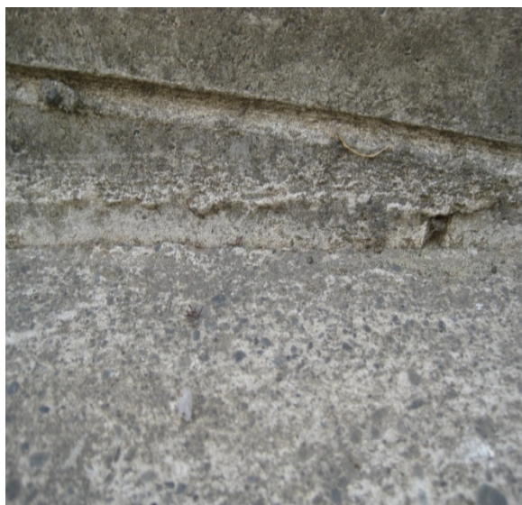
Photo 8: View as pointed by the arrow in photo 7 showing the concrete ramp and masonry wall interface where apparent settlement is observed.
