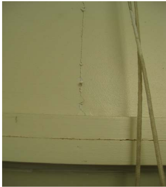
Photo 17: Plaster board cracks found on toilet walls.
