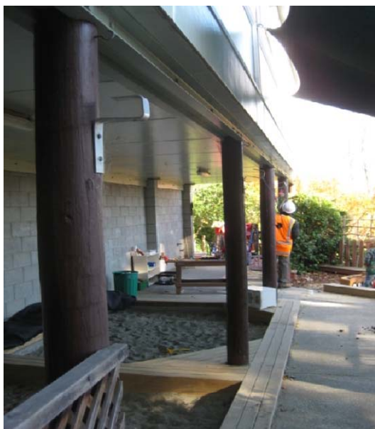
Photo 5: View on the northern side of the building showing the basement walls and timber piles supporting the timber flooring on the ground floor.
