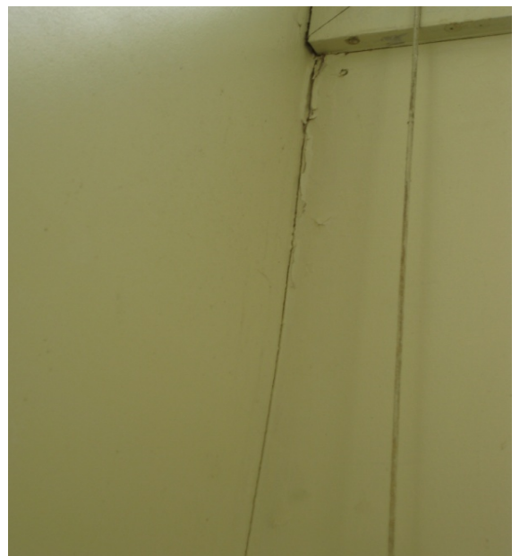
Photo 16: Plaster board cracks found on toilet walls.
