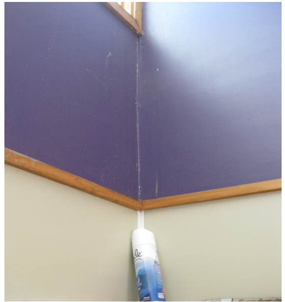
Photo 14: Plaster board cracks found on toilet walls.
