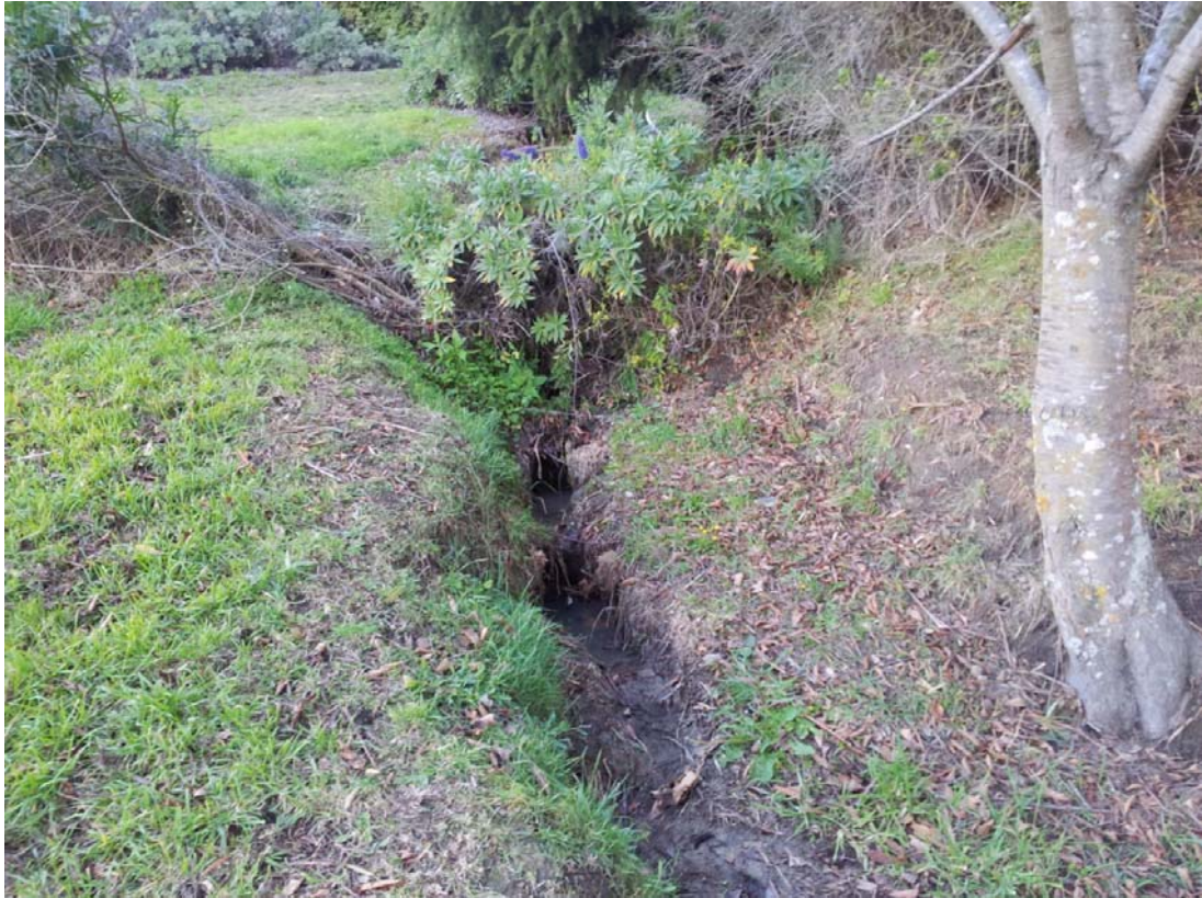
■ Figure 7 Observed tunnel gully
