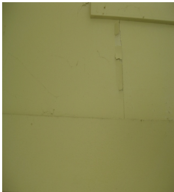
Photo 15: Plaster board cracks found on toilet walls.
