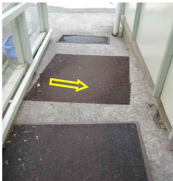
Photo 7: Photo of the building access on the south side of building.
