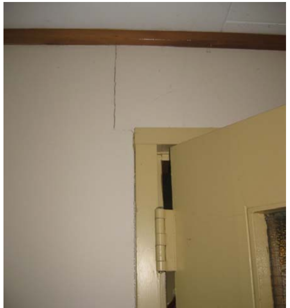
Photo 18: Plaster board cracks found on toilet walls.
