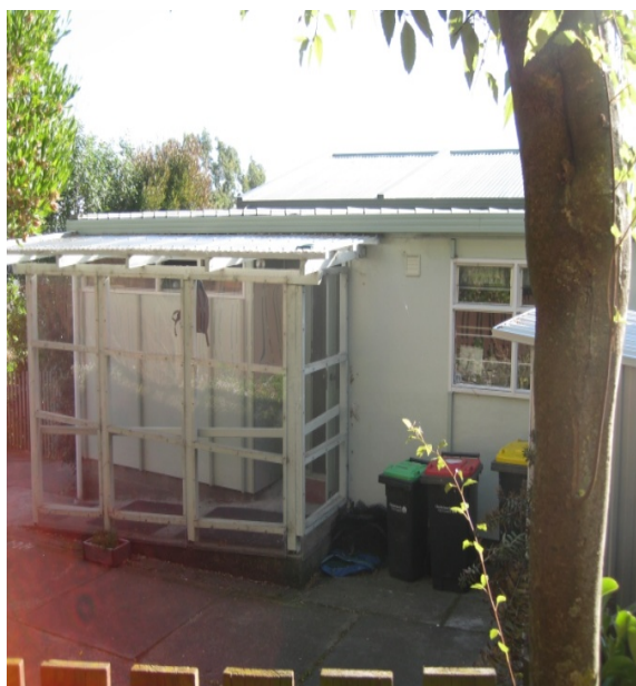
Photo 2: View of the building from south showing alternate access.
