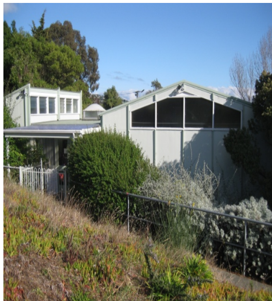
Photo 1: View of the building looking west.
