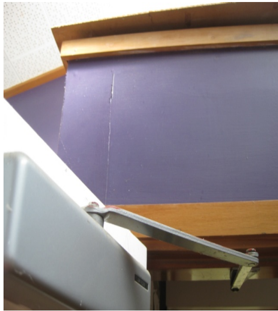
Photo 13: Plaster board cracks found on toilet walls.
