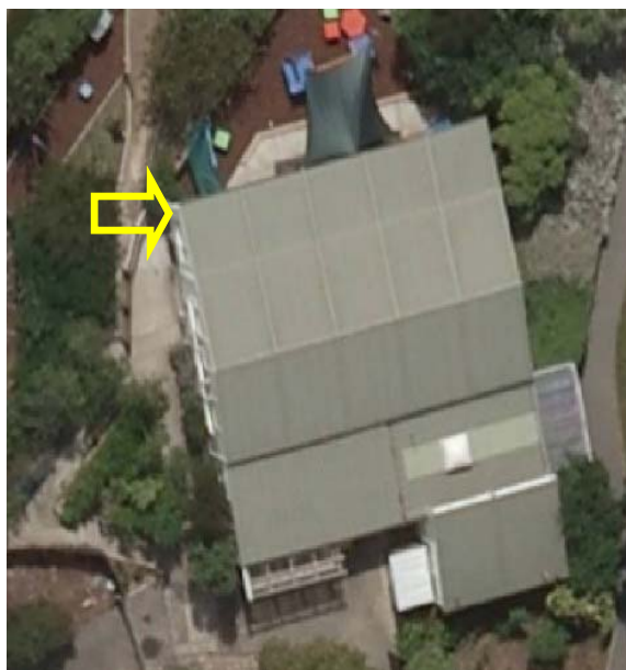
Photo 4: Aerial photo showing location of cracks in Photo 3.
