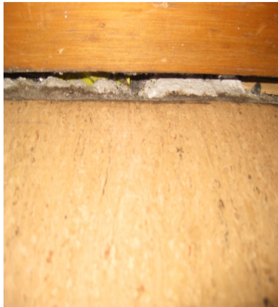
Photo 9: Photo showing increased gap between floor and wall base on the along the corridor of the building access on its south.
