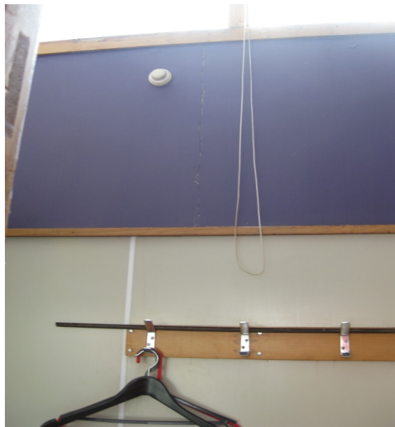
Photo 11: Plaster board cracks found on toilet walls.
