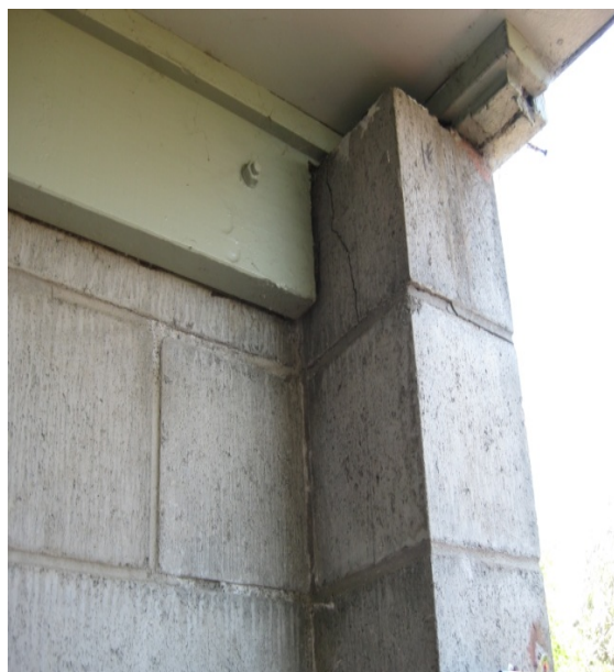
Photo 3: Photo showing cracks on the masonry column on the north west side corner of the retaining wall.
