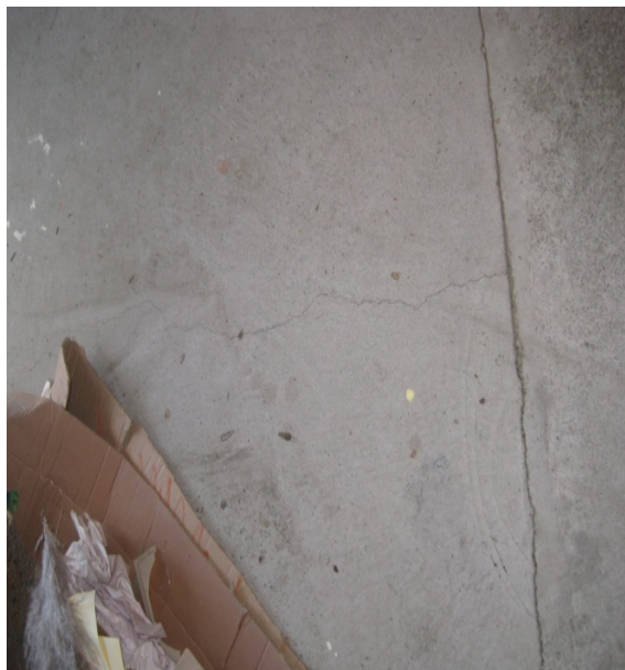
Photo 6: Construction joint on the basement floor opening slightly by about 0.8mm.
