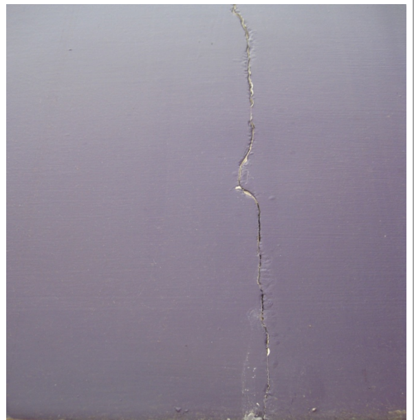
Photo 12: Plaster board cracks found on toilet walls.
