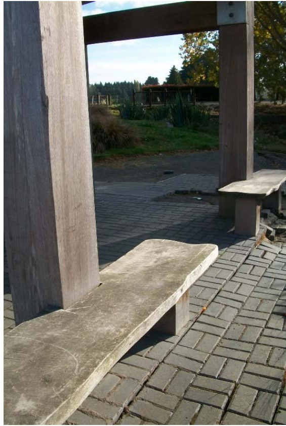
Photo 13: Ground movement in front of the East side of the building.
