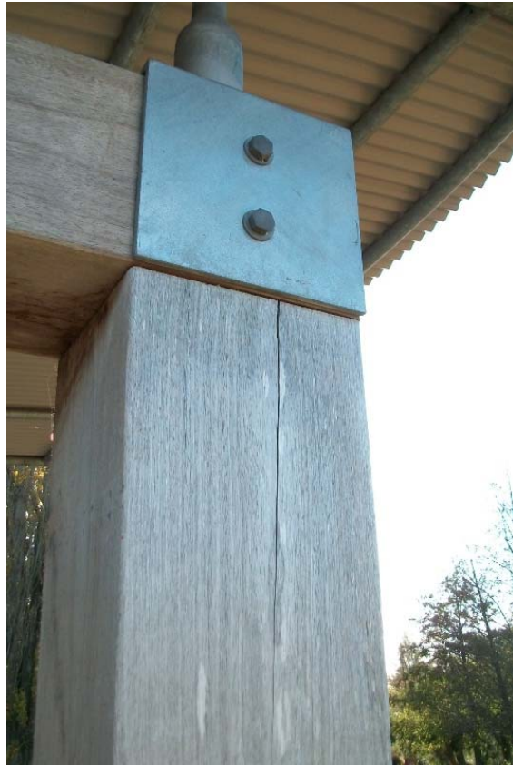
Photo 5: Cracking along the grain of one of the South timber columns (typical).
