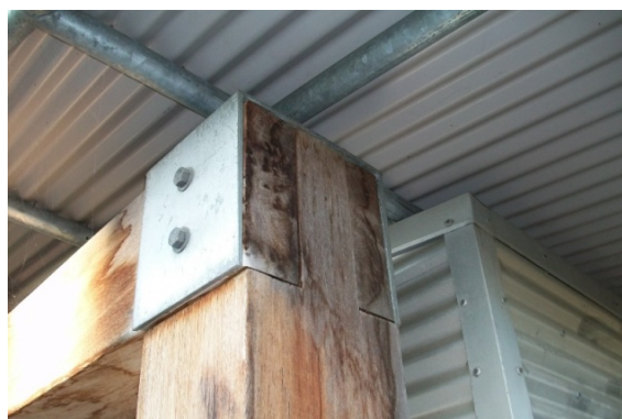
Photo 7: Beam-column connection detail of timber portal frame on West side of building (typical).
