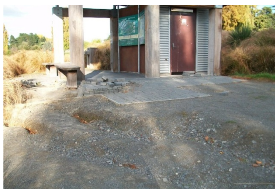
Photo 15: Ground movement around the building.
