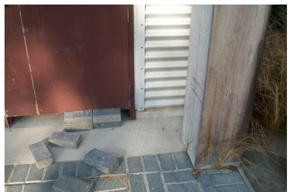
Photo 8: No damage to foundation slab (North side of building shown, typical).
