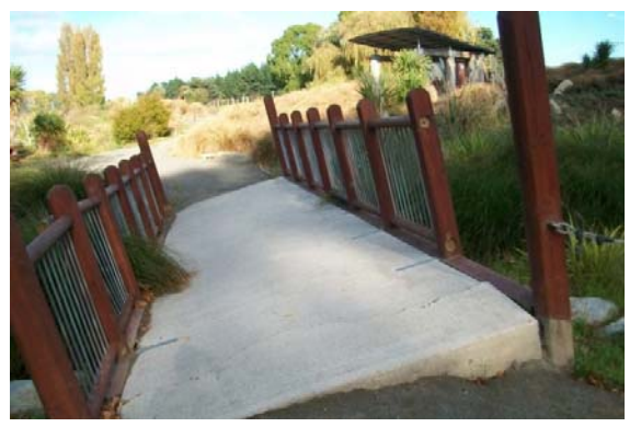
Photo 16: Ramp angled and cracked showing evidence of ground movement Northeast of the building.
