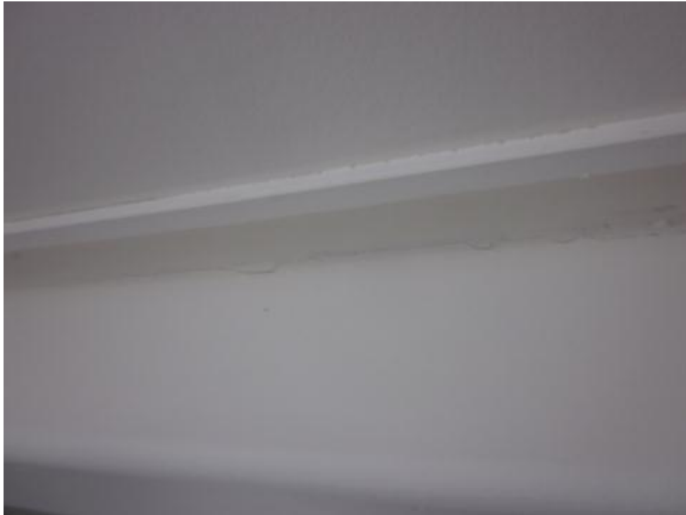
Photograph 5 Minor cracking to internal plasterboard lining.
