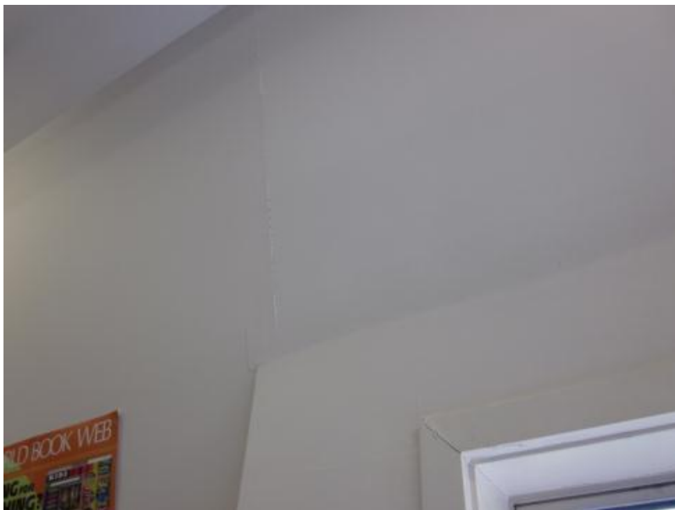
Photograph 8 Minor cracking to internal plasterboard lining.
