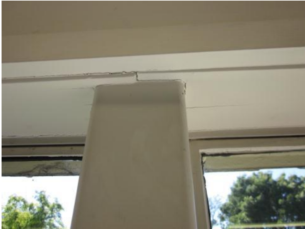
Photograph 7 Minor cracking to internal plasterboard lining around steel portal frame.
