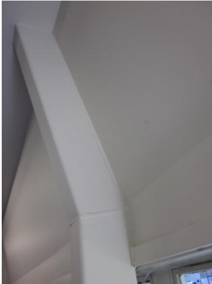
Photograph 9 View of steel portal frame.
