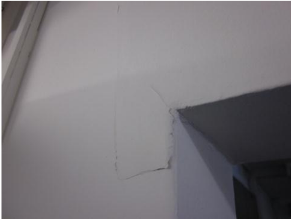
Photograph 10 Minor cracking to internal plasterboard lining.
