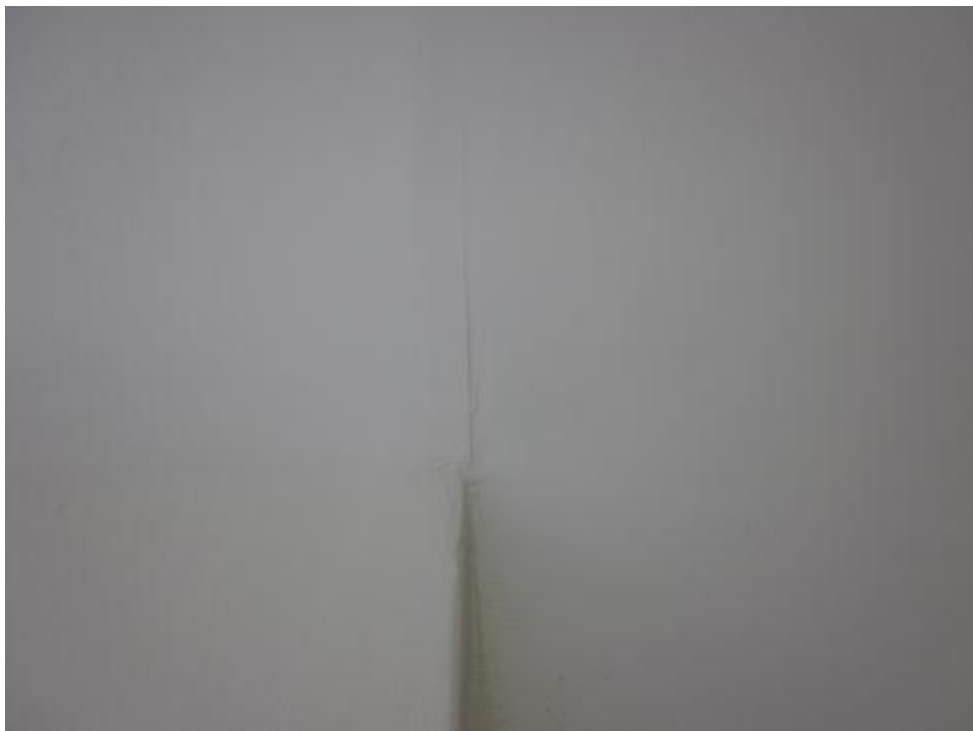
Photograph 6 Minor cracking to internal plasterboard lining.
