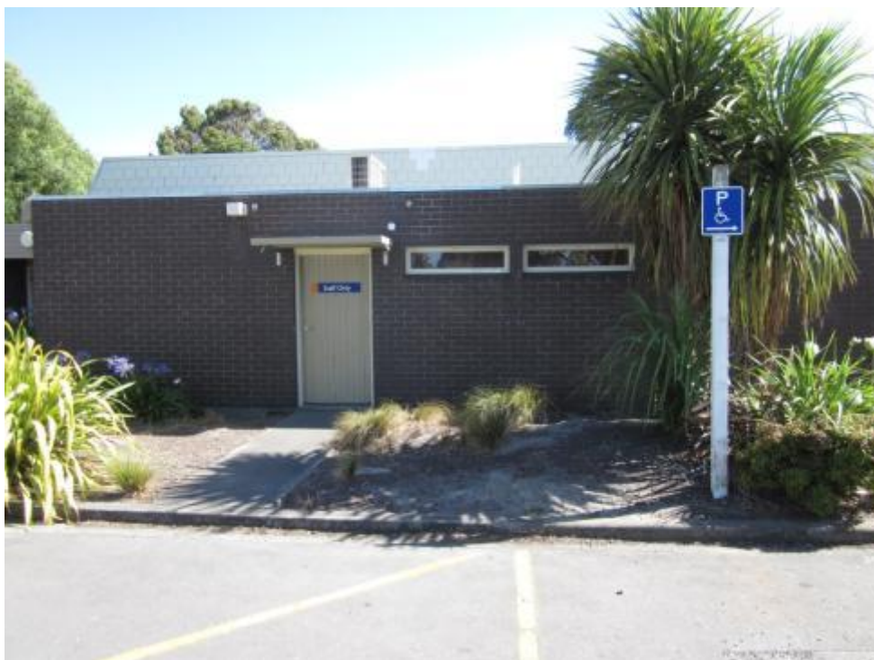
Photograph 3 Brick clad, timber framed section of the building.
