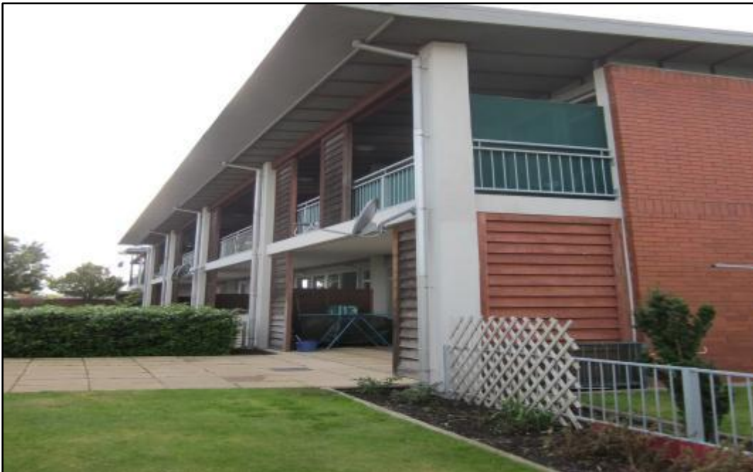
Photo 2. Hornby Courts Block B (Front, southwest of the building).
