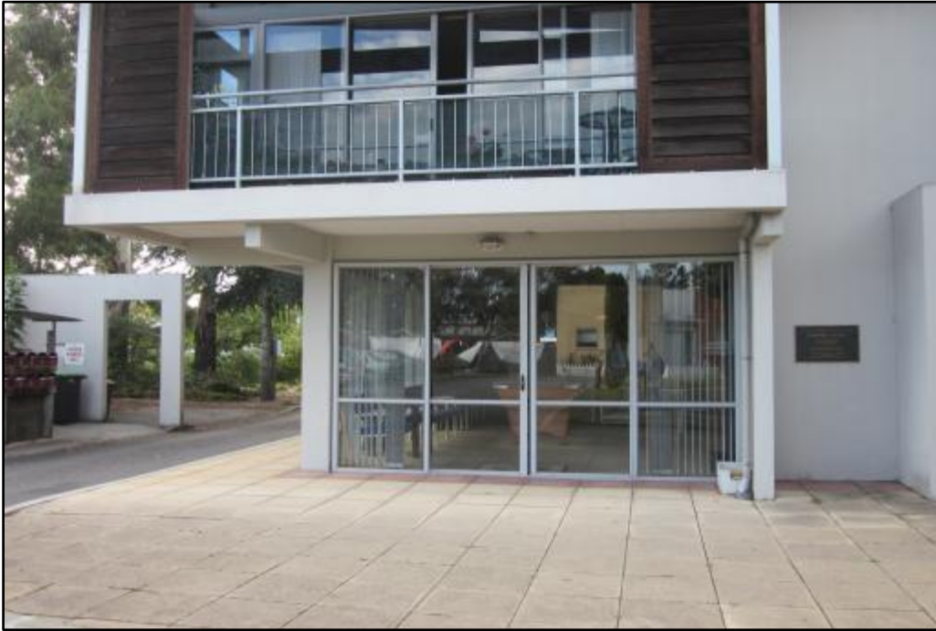
Photo 17. Reinforced cantilevered slab, front view of Communal Block.
