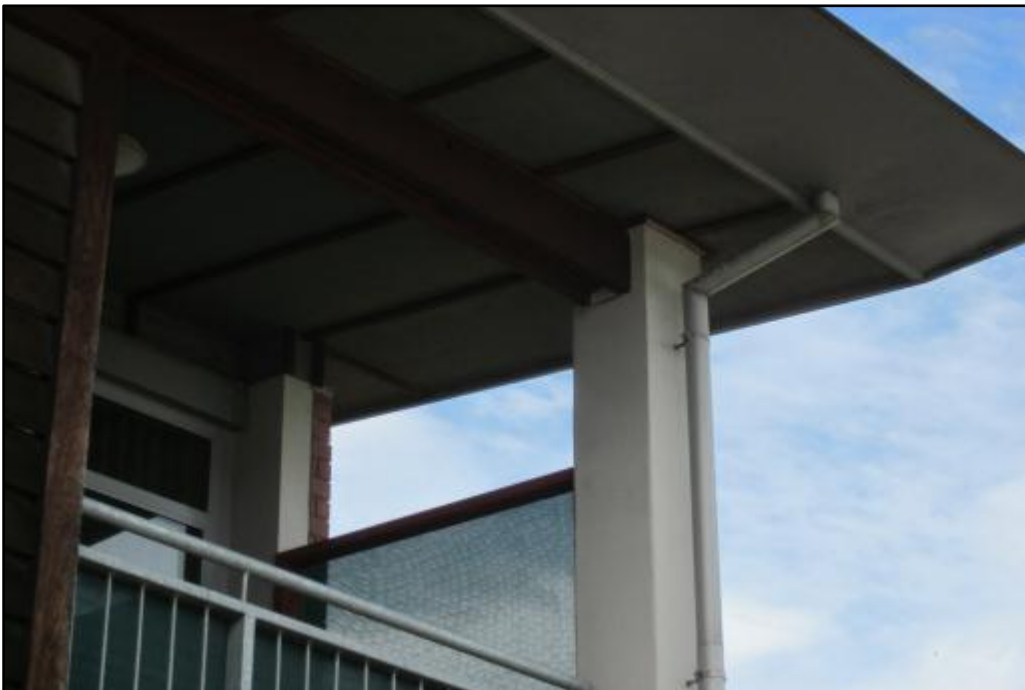
Photo 6. RC column supporting the roof (front view of building).
