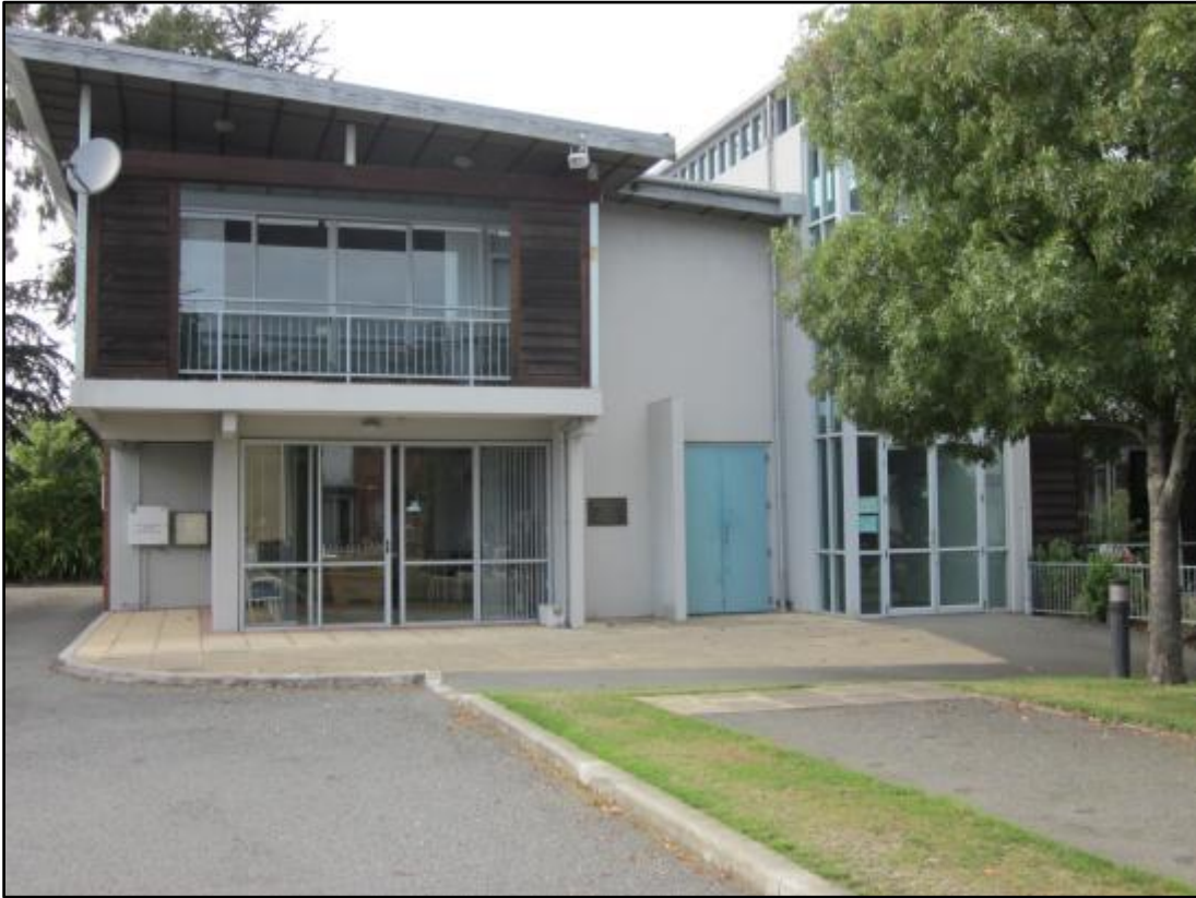
Photo 5. Hornby Courts Block A Communal Block (Front, northeast of the building).
