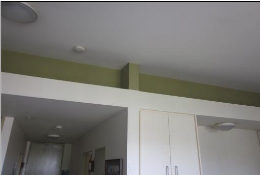
Photo 10. Interior of building.
