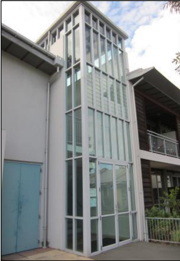
Photo 11. Door entrance toward staircase (communal block to the left and residential block to the right).
