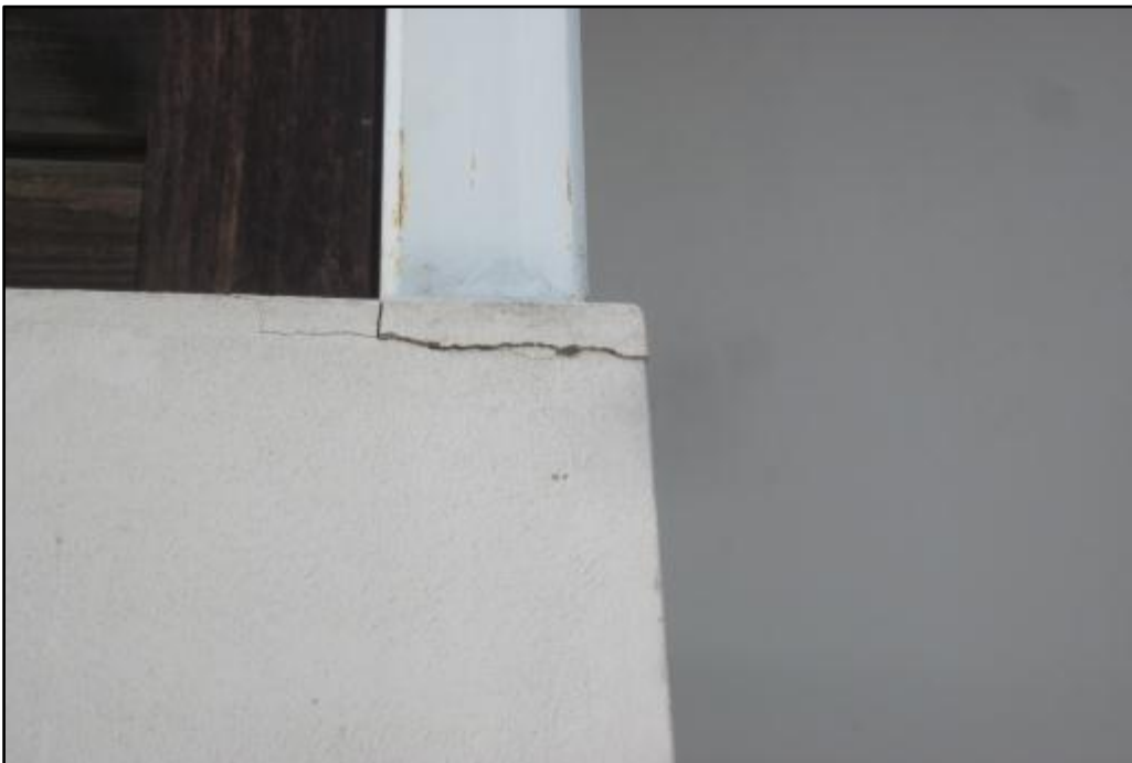
Photo 14. Cracking at slab bearing the loads from the steel column (front view).
