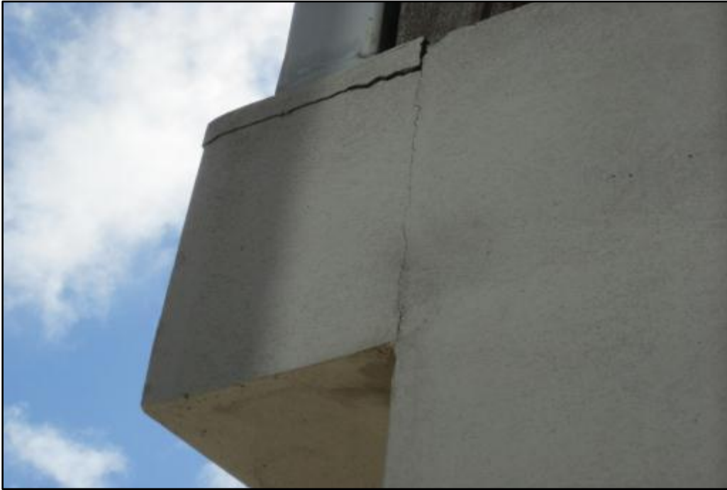
Photo 15. Cracking at slab bearing the loads from the steel column (side view).
