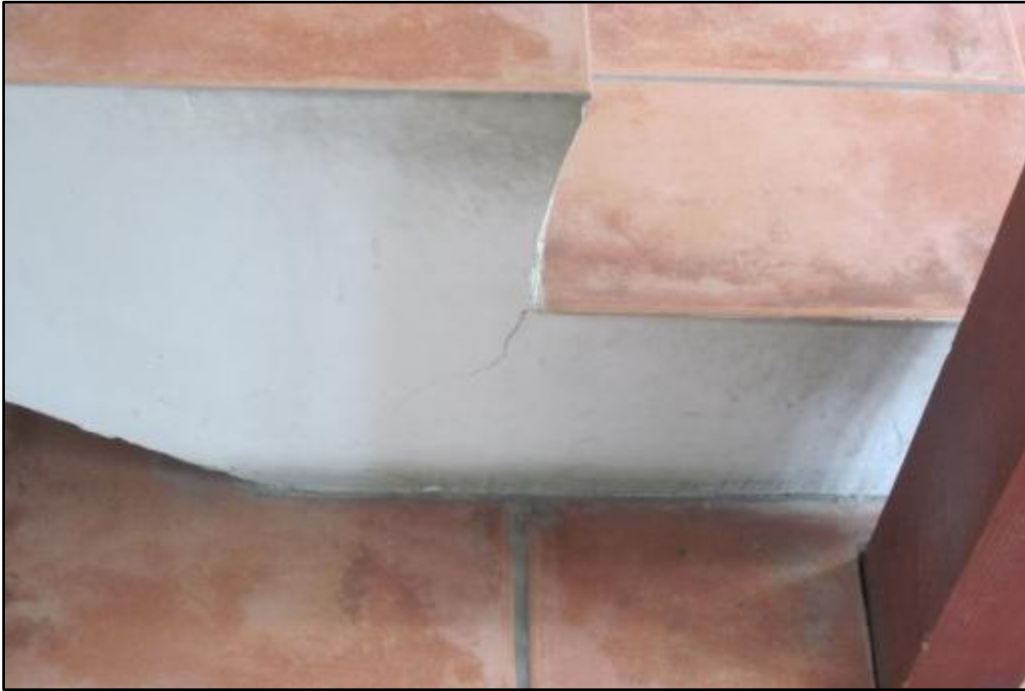
Photo 13. Minor cracks at concrete staircase.
