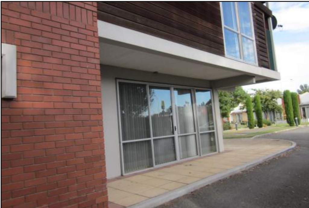
Photo 16. Reinforced cantilevered slab at front; brick wall cladding at rear (photo taken at side view of communal block).
