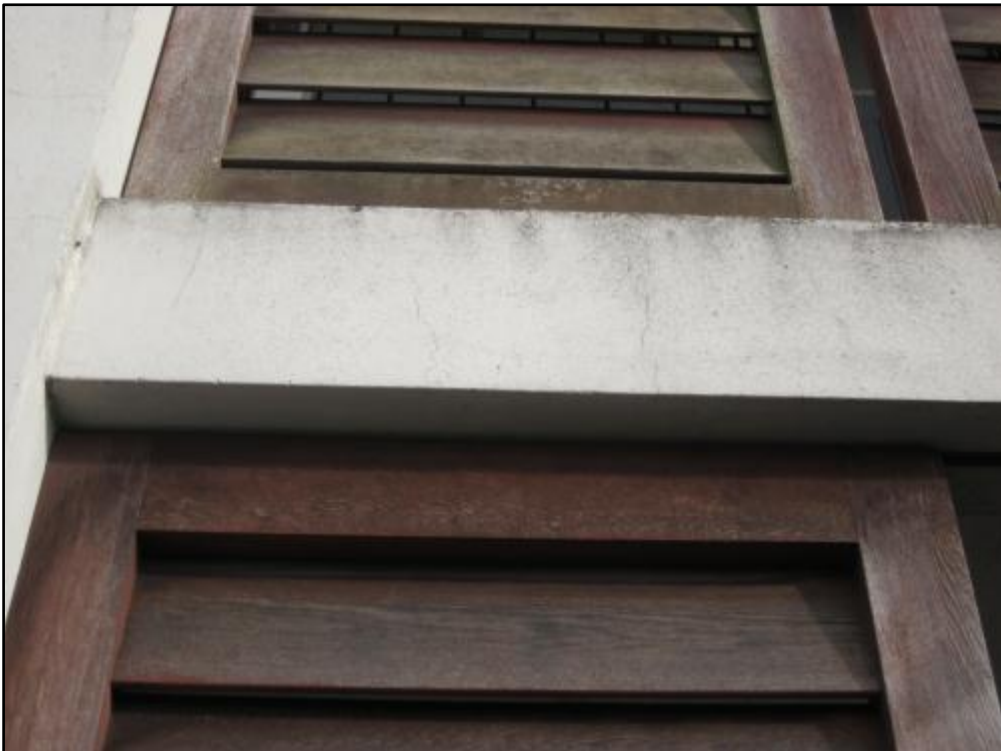
Photo 18. Cracking found at external beam.
