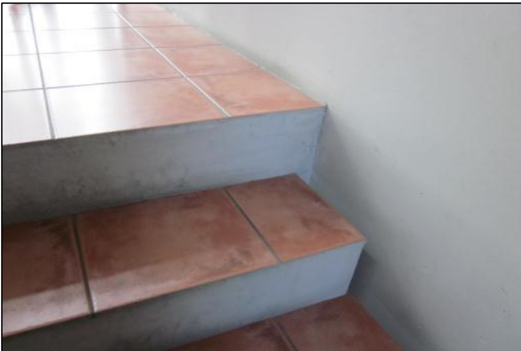
Photo 12. Minor cracks at concrete staircase.
