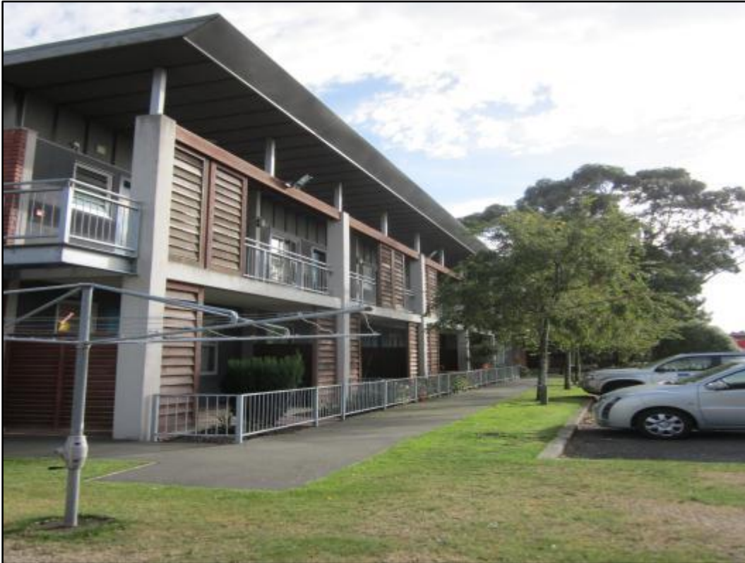
Photo 1. Hornby Courts Block A (Rear, southwest of the building).
