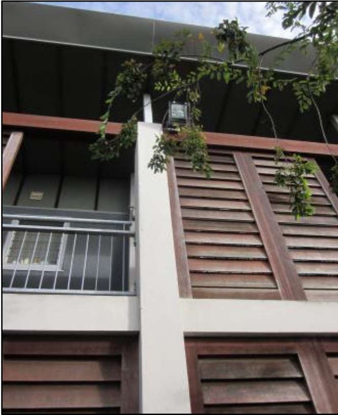
Photo 7. RC columns connected to steel columns supporting the roof (rear view of building).
