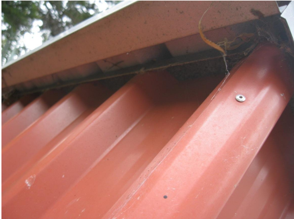
Photograph 3 Wall at eaves with gutter above.
