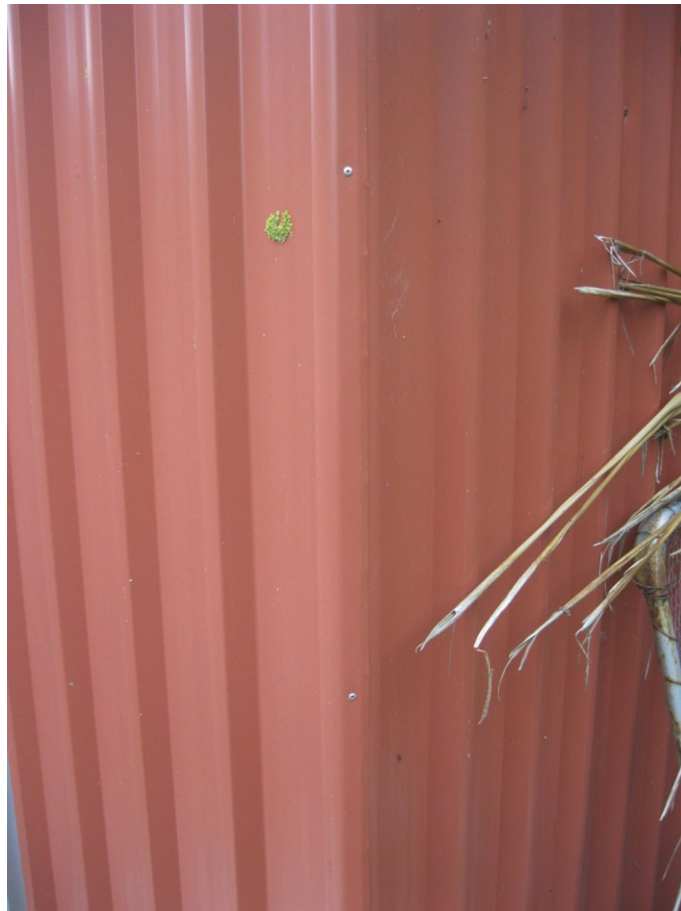
Photograph 2 Rivet connections of steel sheets at corners.
