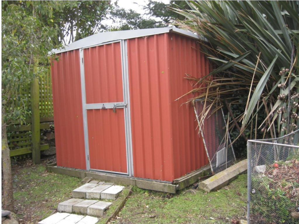
Photograph 1 View of shed from the north.
