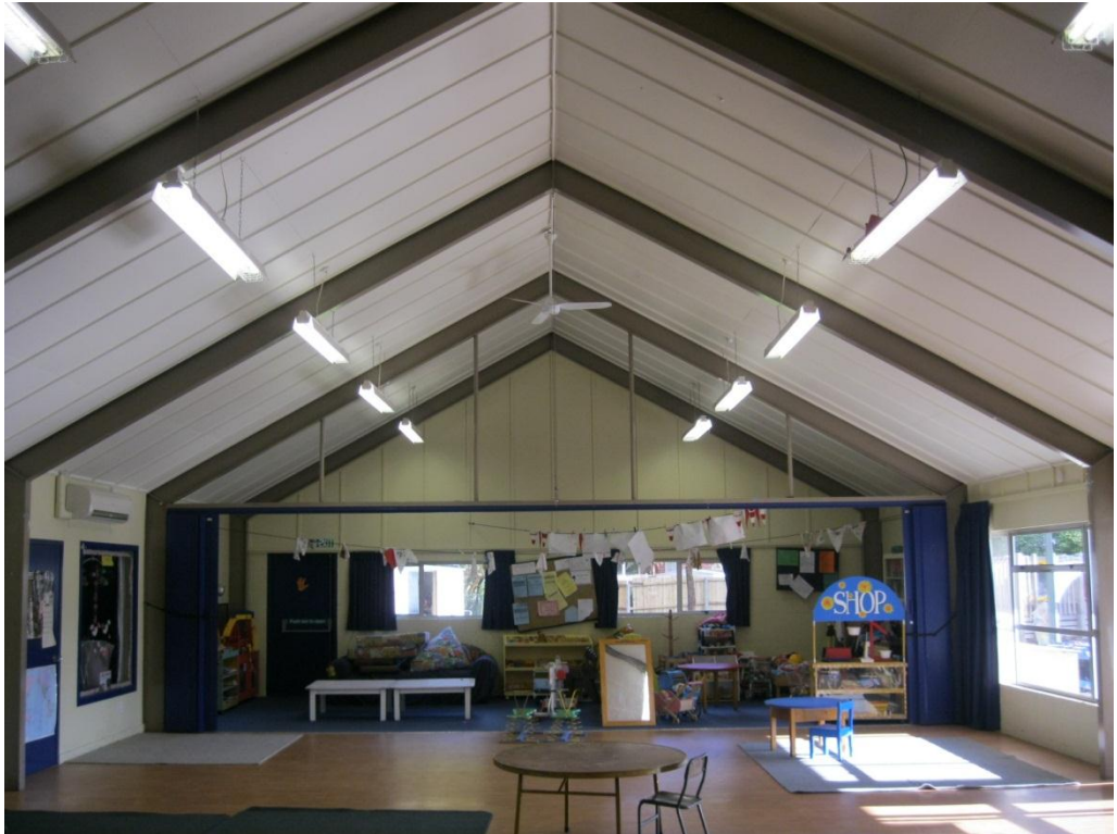
Photograph 3: Steel portal frame to hall structure
