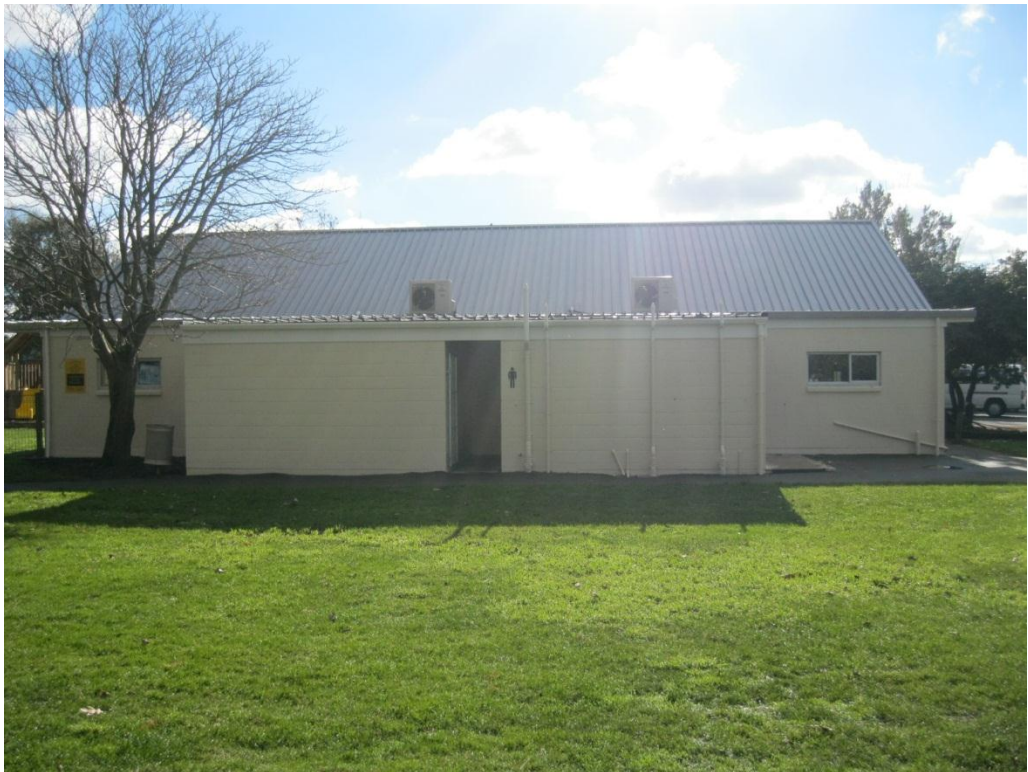
Photograph 2: Toilet block to west of the structure
