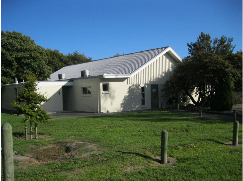
Photograph 1: Western and southern facing elevations showing hall and toilet block
