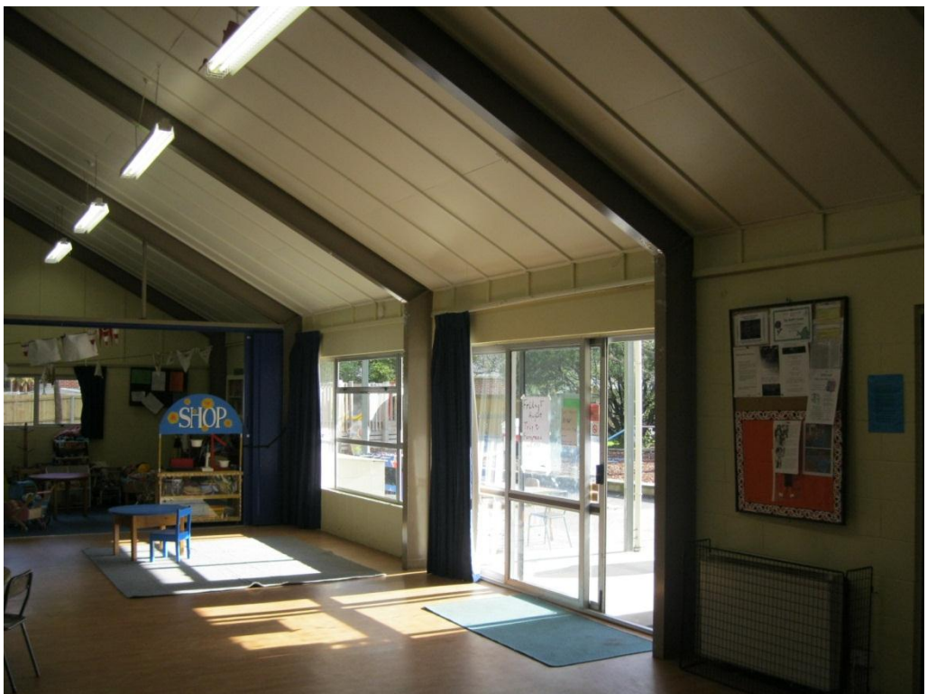
Photograph 4: Concrete columns and beams to right of portal frame to offer support for openings
