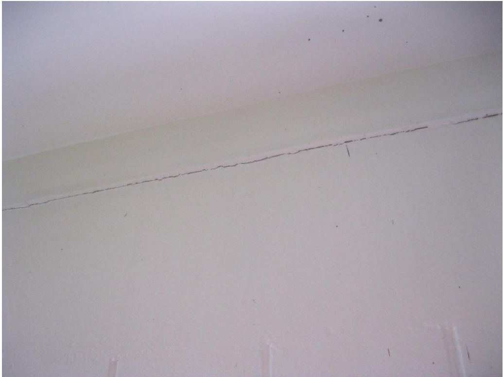
Photograph 5: Minor separation between plasterboard ceiling and blockwork masonry
