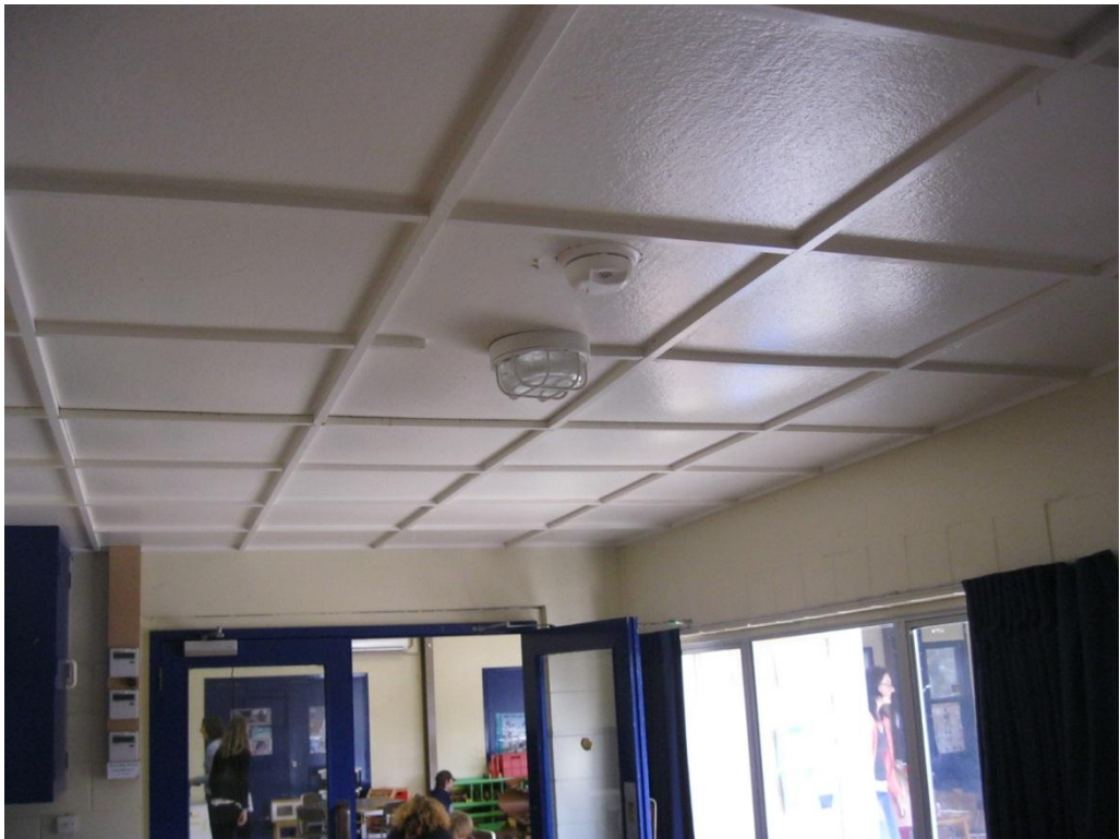
Photograph 6: Fibreboard ceiling to kitchen/toilet block to eastern side of the structure
