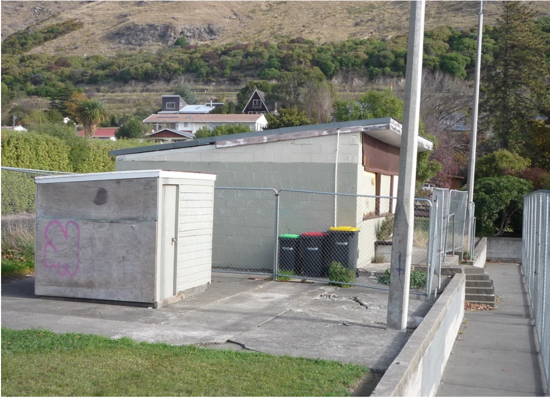
Photograph 1: General view of the north facing side of the shed.
