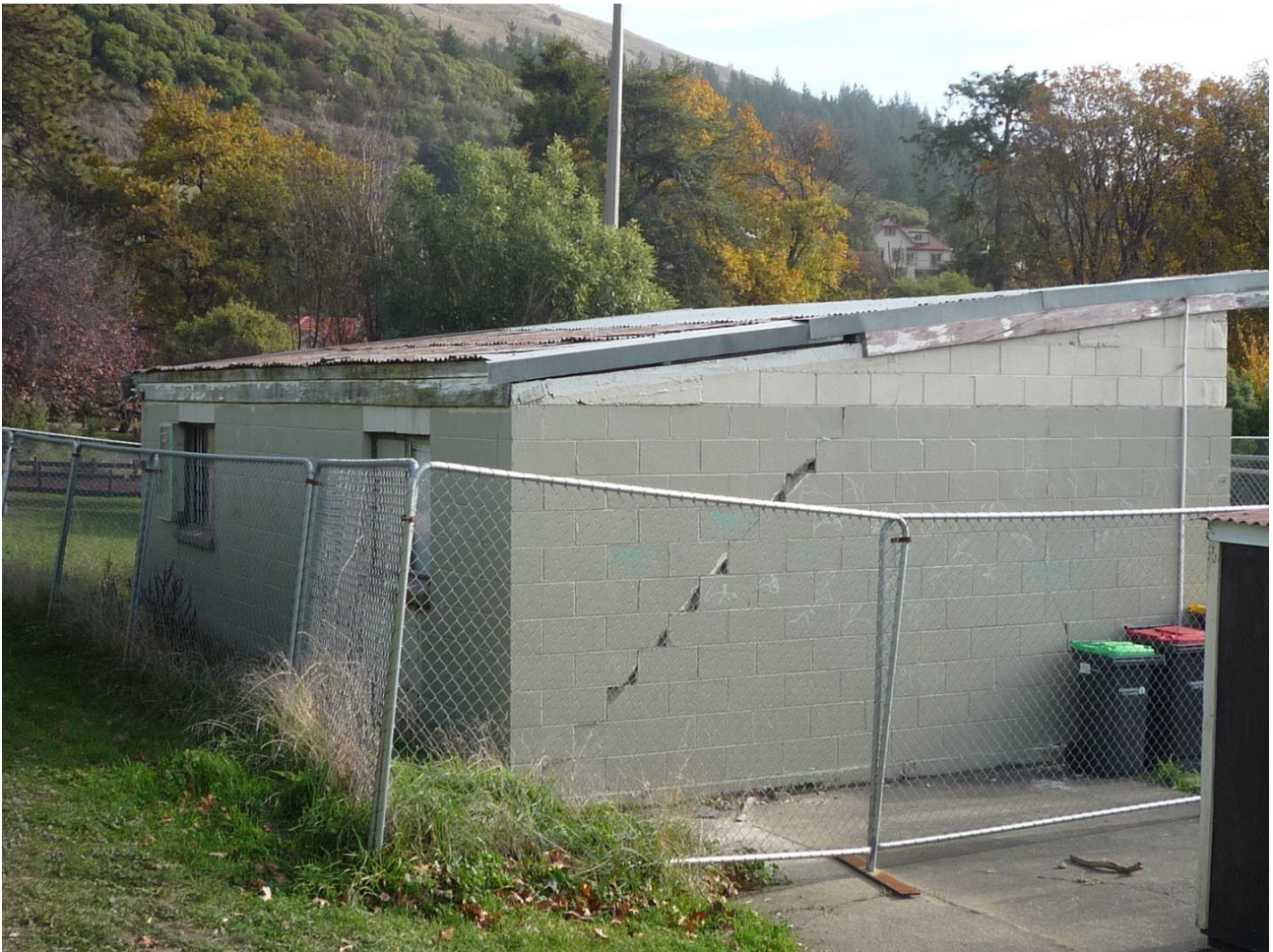
Photo 2: View of the large crack on the east wall
