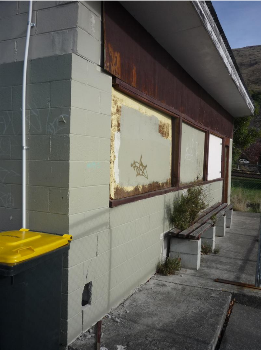
Photo 1: View of the north wall of the building
