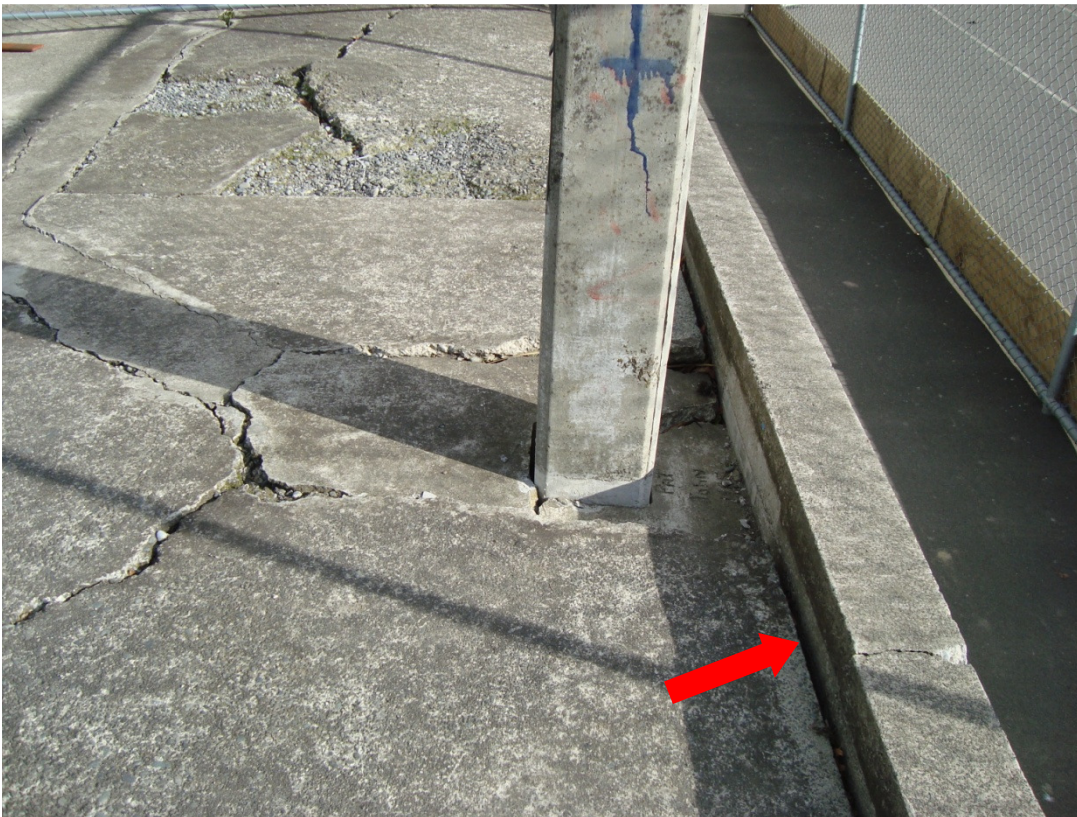
Photograph 4: View of the 20mm lateral movement of the retaining wall.
