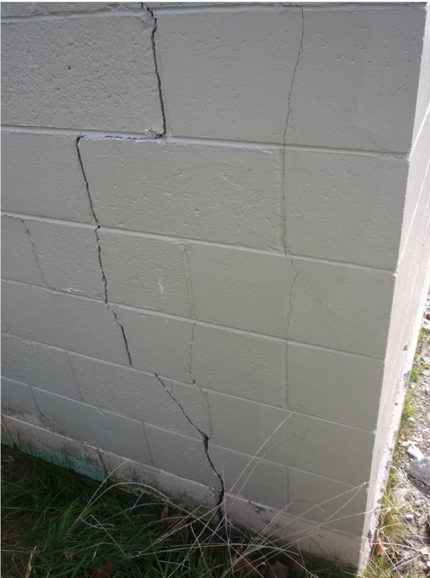
Photo 4: View of the south wall showing the crack caused by the east wall leaning out of plane
