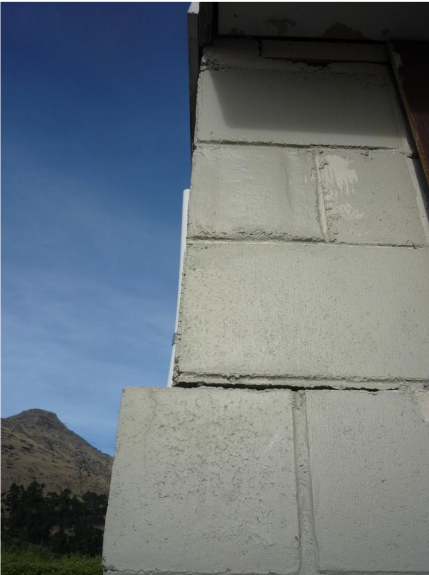
Photo 3: View of the wall lateral displacement near the top of the east wall
