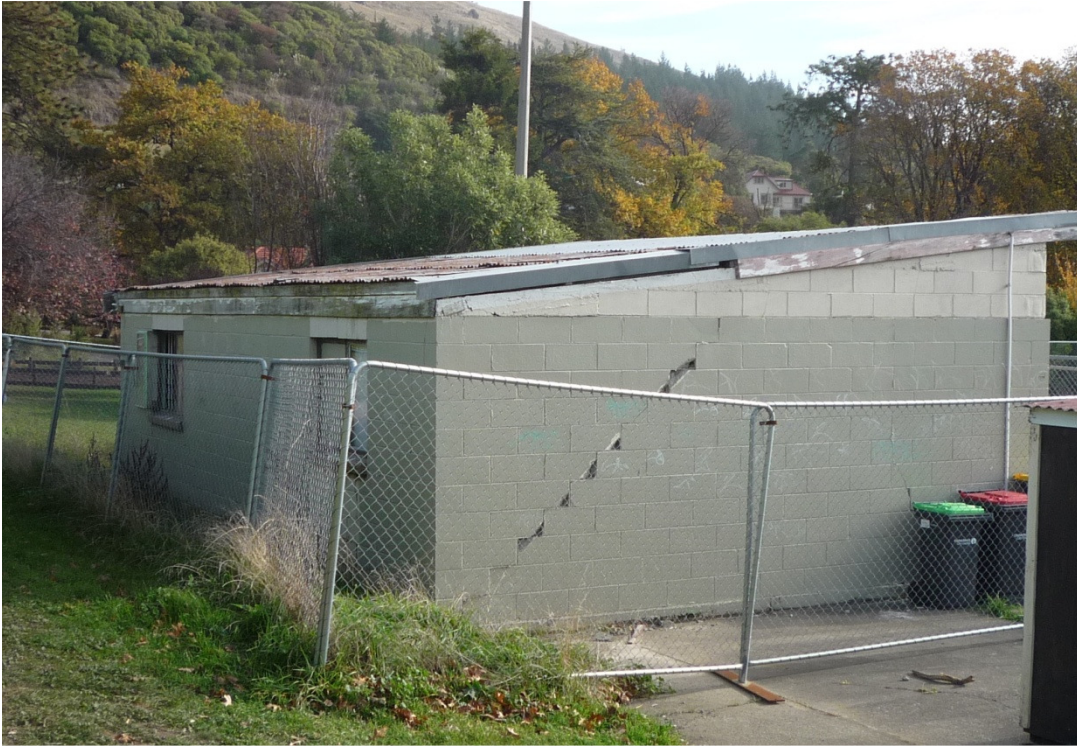
Photograph 5: General view of the east and south elevations of the shed.
