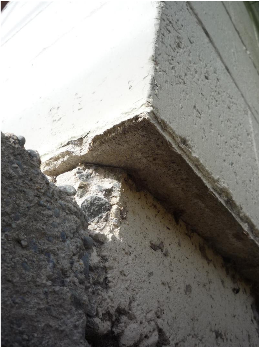
Photo 5: View of the west wall displacing laterally at the foundations
