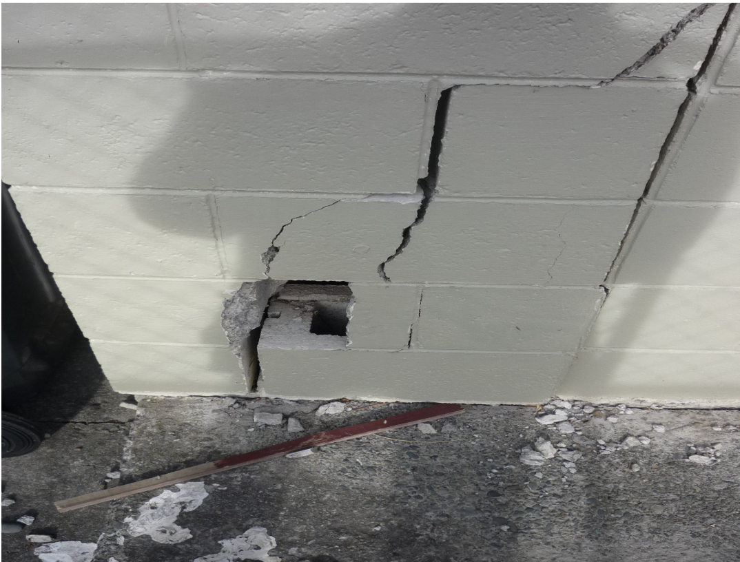
Photograph 2: View of the 10mm wide separation between the perimeter wall and the concrete slab.
