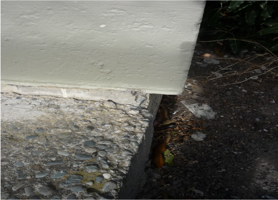
Photograph 3: View of the 20mm subsidence of the concrete slab from perimeter wall. (Located far west corner of the north elevation of the shed)
