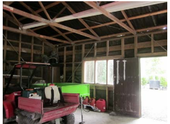
Photo 4: North Wall Bracing
