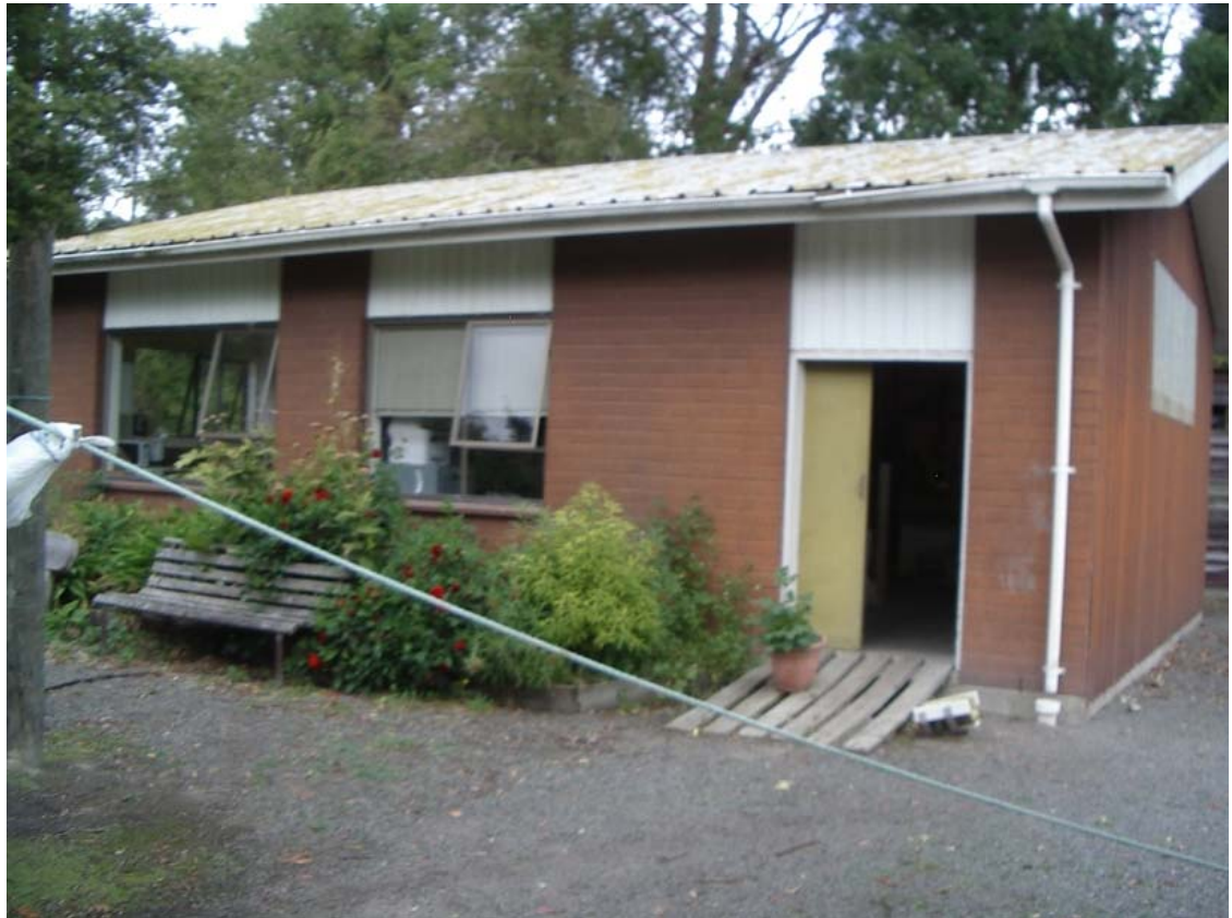
■ Figure 7 No visible damage to the structure
