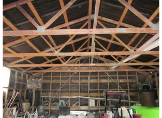
Photo 2: Internal Structure of Building
