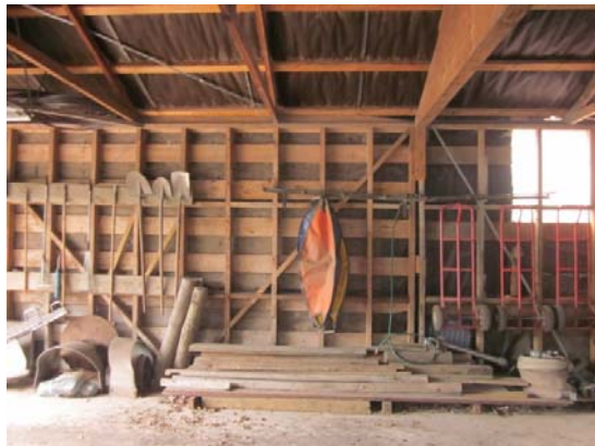
Photo 3: South Wall Bracing
