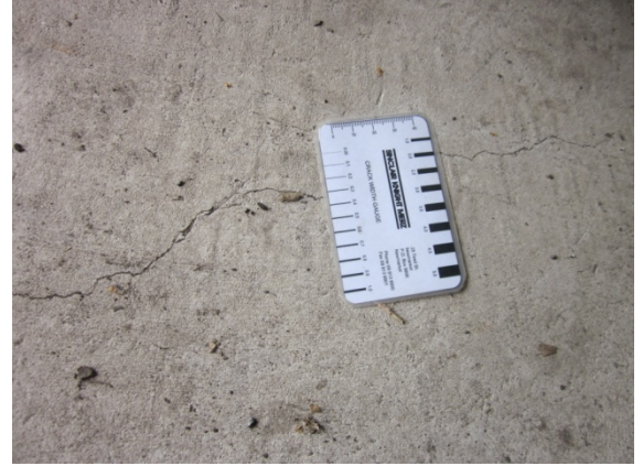
Photo 8: Close up of Photo 8
