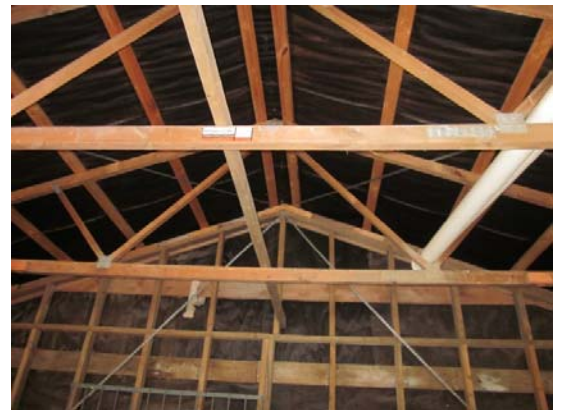
Photo 6: West Wall & Roof Bracing
