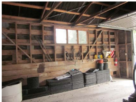
Photo 5: North Wall Bracing Continued
