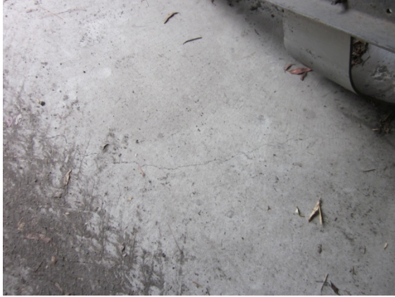
Photo 7: Hairline Cracking to Floor Slab – Near Main Entrance
