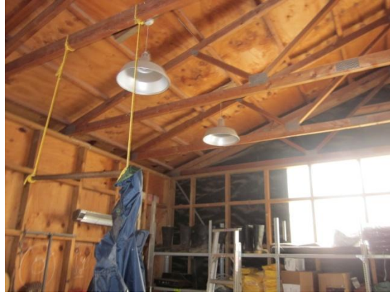
Photo 5: Internal View – Plywood Linings
