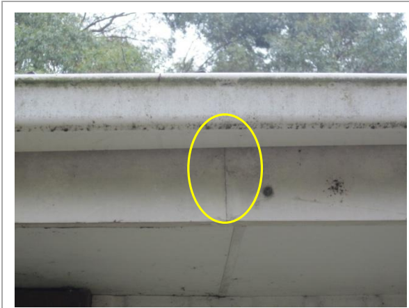
Photo 9: Close up of Photo 9
