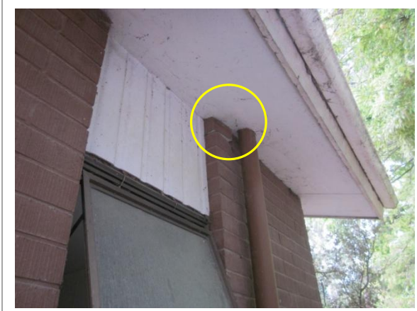
Photo 11: Loose Brick above Toilet Window
