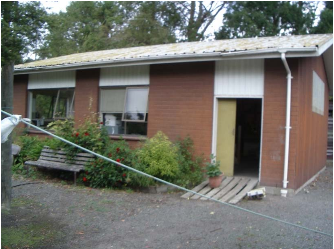
■ Figure 7 No visible damage to the structure
