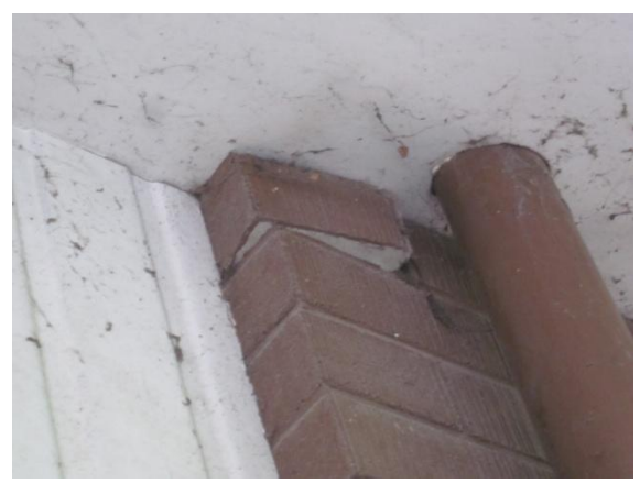
Photo 12: Close up of Photo 11
