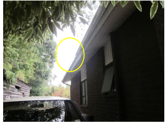
Photo 10: Damaged Guttering along West Wall
