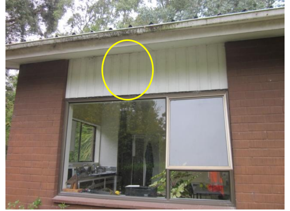
Photo 6: Hairline Cracking at Hardiboard Vertical Joints
