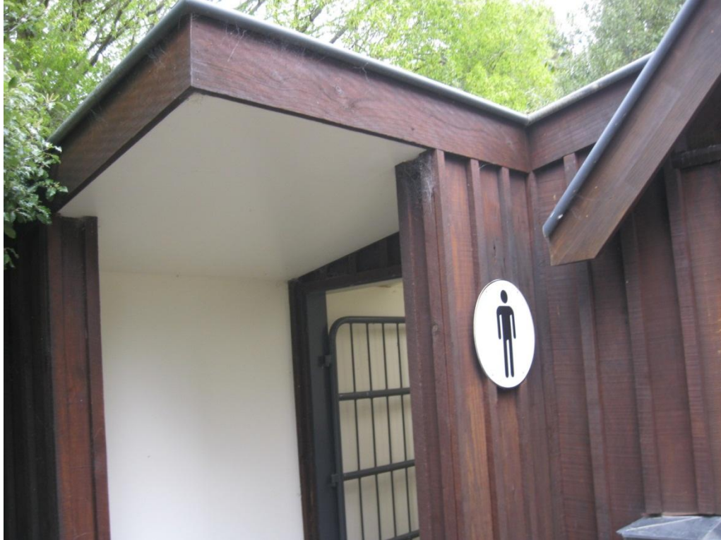
Photograph 3 Cantilevered Roof over entrance to the addition (section not shown in plans)
