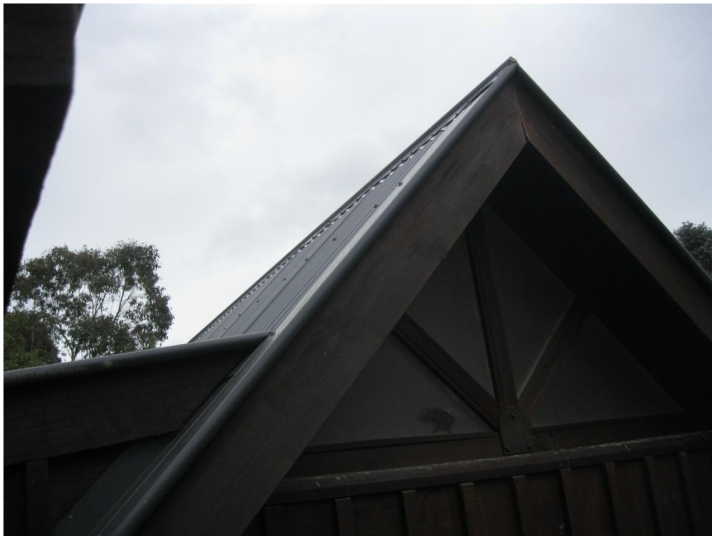
Photograph 8 Additional roof section meeting original section.
