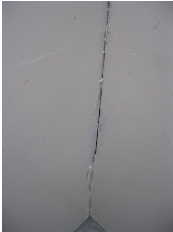
Photograph 6 Vertical crack in paint finish between adjacent walls.
