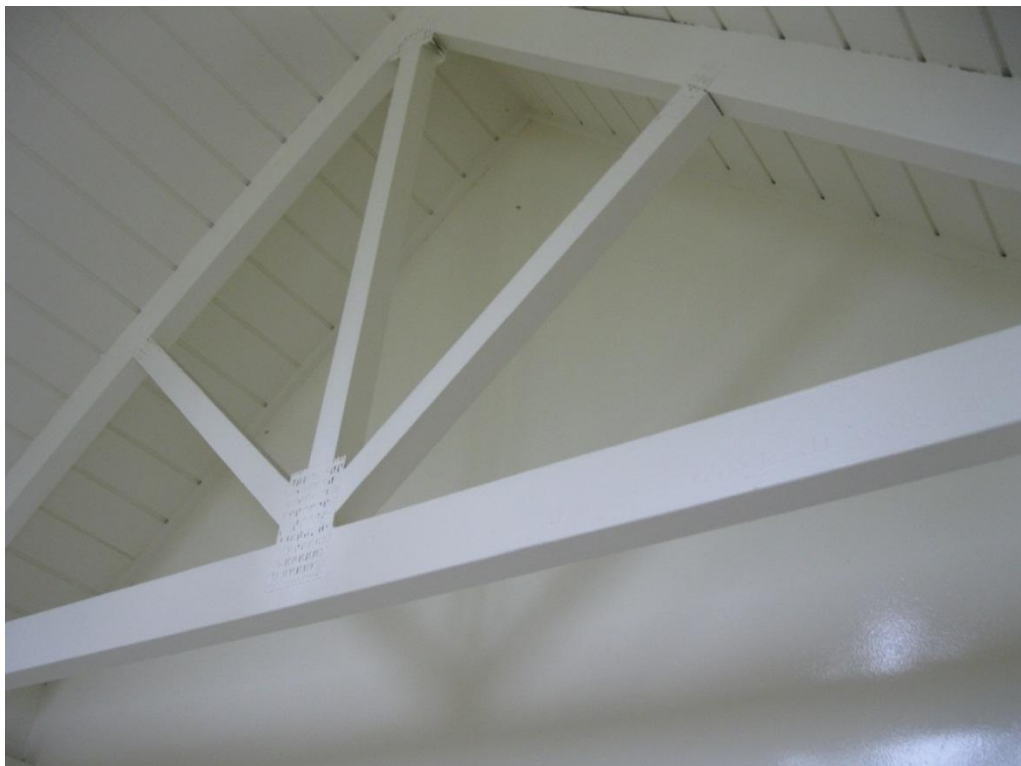
Photograph 4 Timber truss and boards inside original structure.
