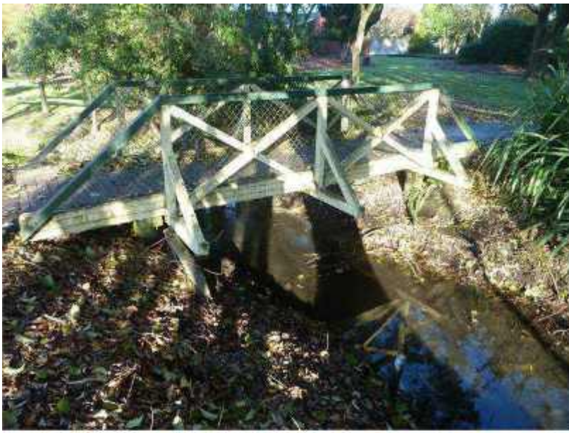
Photo 9: View of Stream alongside Halswell Road, Looking Southwest
