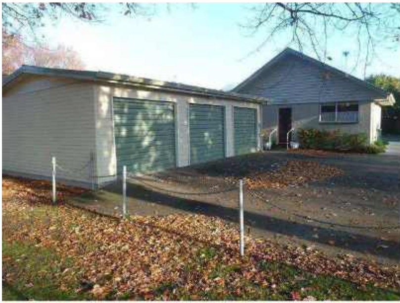
Photo 5: View behind Flat 11, Looking West (Garages in Foreground)
