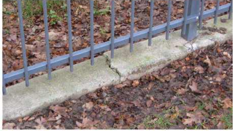
Photo 10: View Cracked Southern Fence Foundation, Looking Southwest
