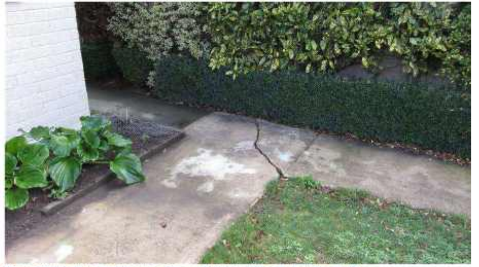
Photo 30: Cracking of Concrete Footpath behind Flat 1, Looking North
