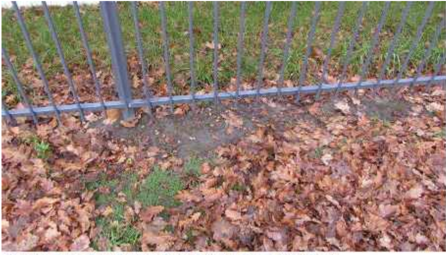
Photo 13: Ejecta along Southern Fence Behind Flat 15, Looking South
