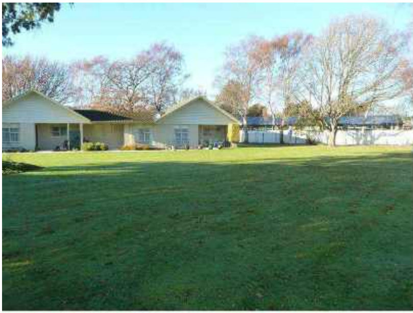
Photo 1: View Behind Flats 3-5, Looking Southeast
