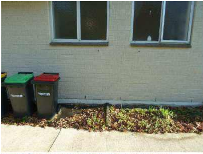
Photo 21: Minor Stepping Crack at Back of Flat 6, Looking Northwest
