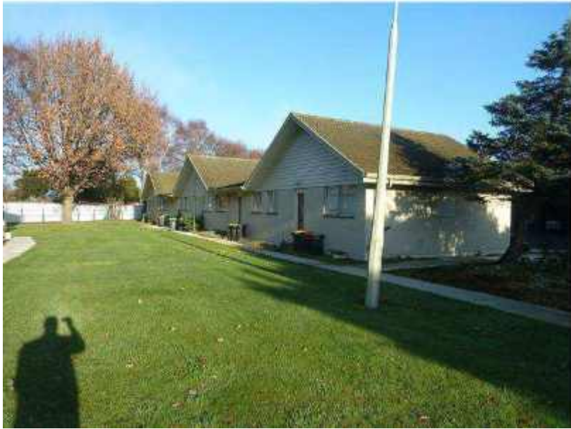
Photo 7: View Behind Flats 6-14, Looking South
