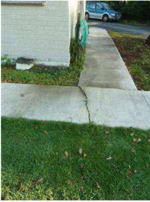
Photo 29: Cracking of Concrete Footpath Behind Flat 6, Looking Northwest
