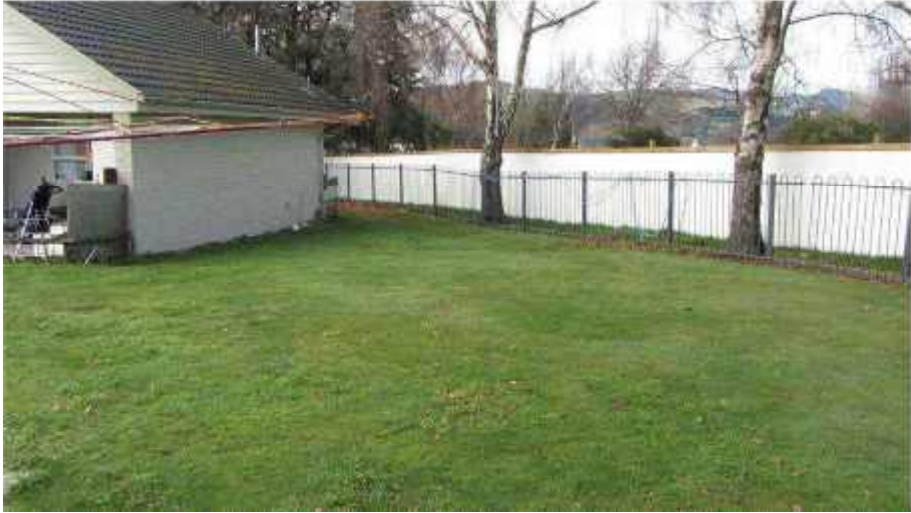
Photo 15: View of Ground Settlement behind Flat 15, Looking Southeast
