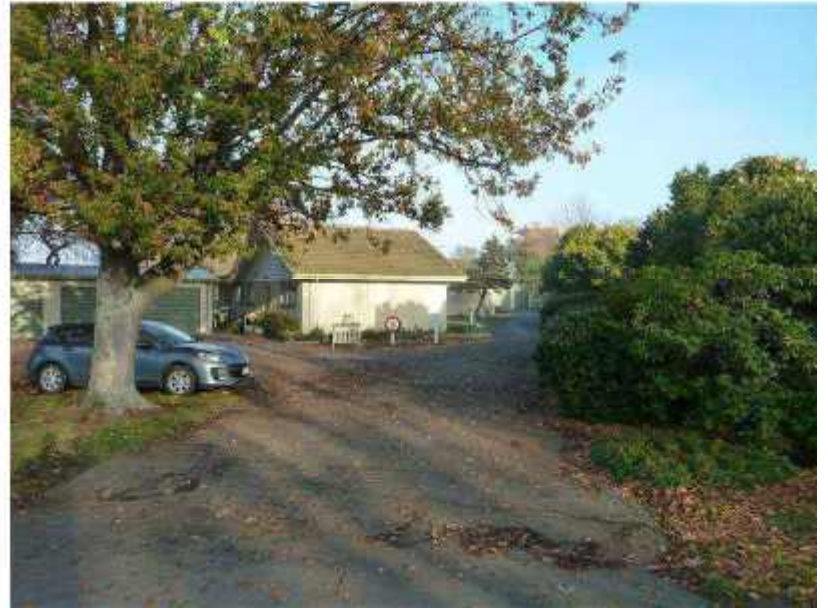
Photo 4: View of Driveway, Flat 11 and Garages, Looking West
