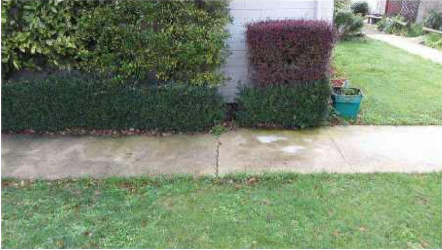
Photo 31: Cracking of Concrete Footpath behind Flat 1, Looking Northeast
