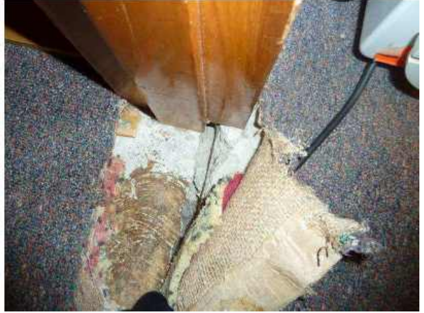
Photo 28: Cracking of Concrete Slab Floor in Flat 8
