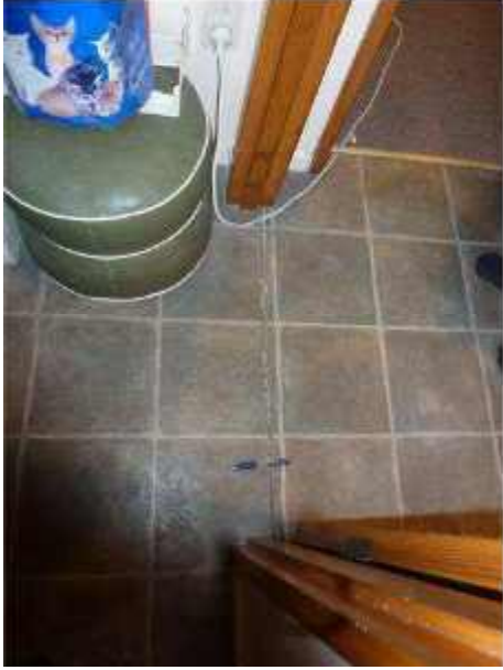
Photo 27: Cracking of Concrete Slab Floor in Flat 8
