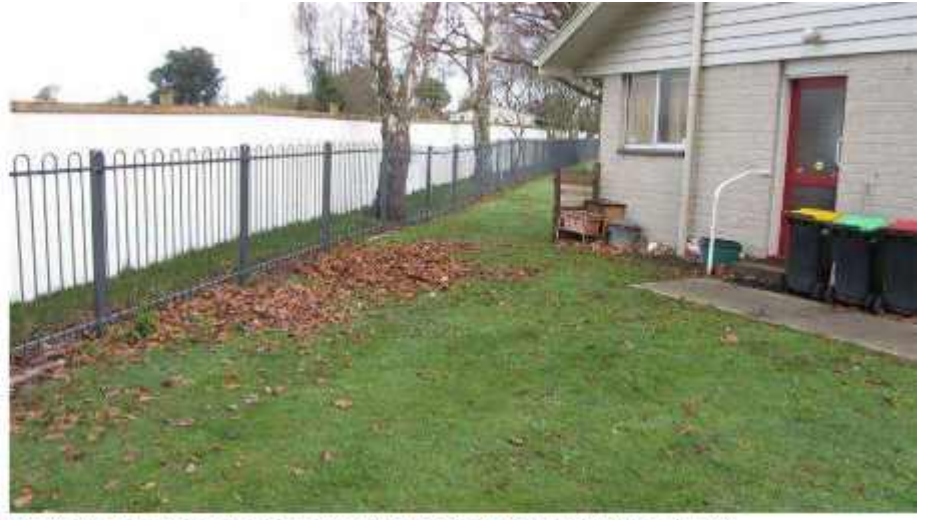
Photo 14: View of Ground Settlement behind Flat 15, Looking Southwest
