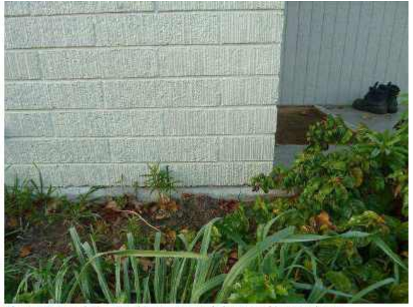
Photo 26: Foundation Cracking at Front of Flat 8, Looking Southeast
