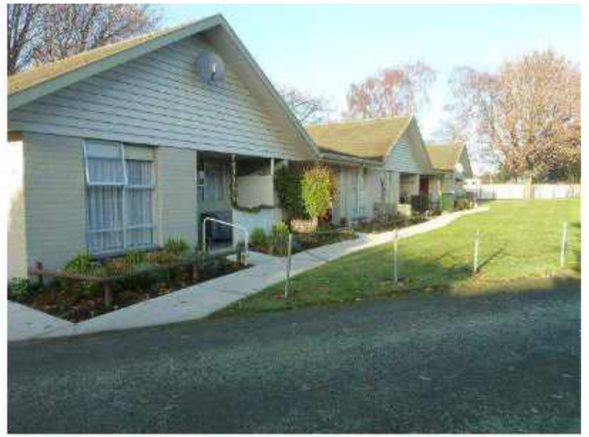
Photo 6: View of Front of Flats 11-15, Looking South
