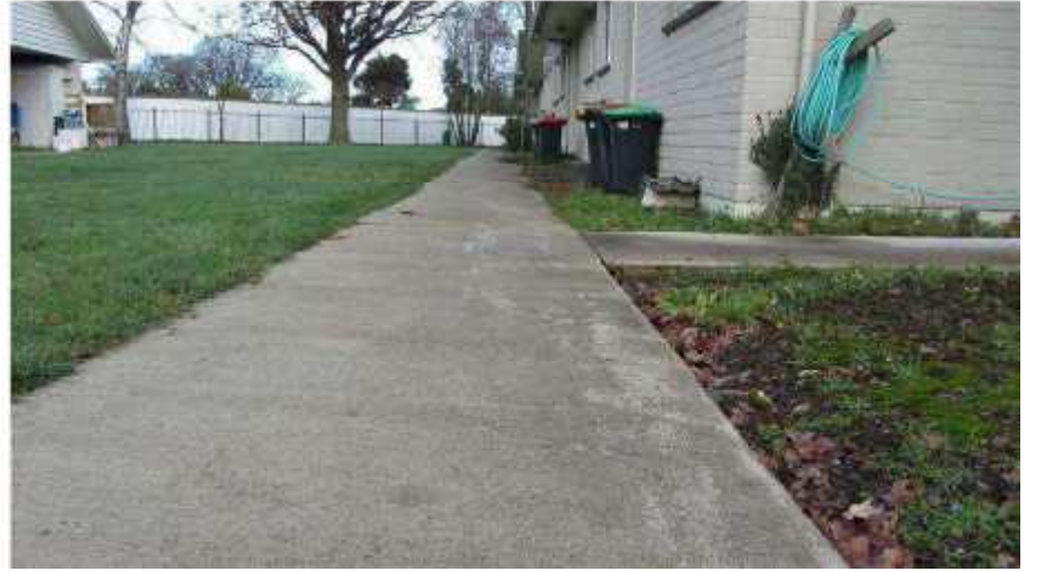
Photo 32: Subsidence Tilting of Concrete Footpath behind Flats 6-8, Looking Southwest
