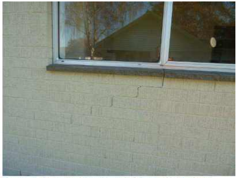
Photo 22: Moderate Stepping Crack at Back of Flat 7, Looking Northwest
