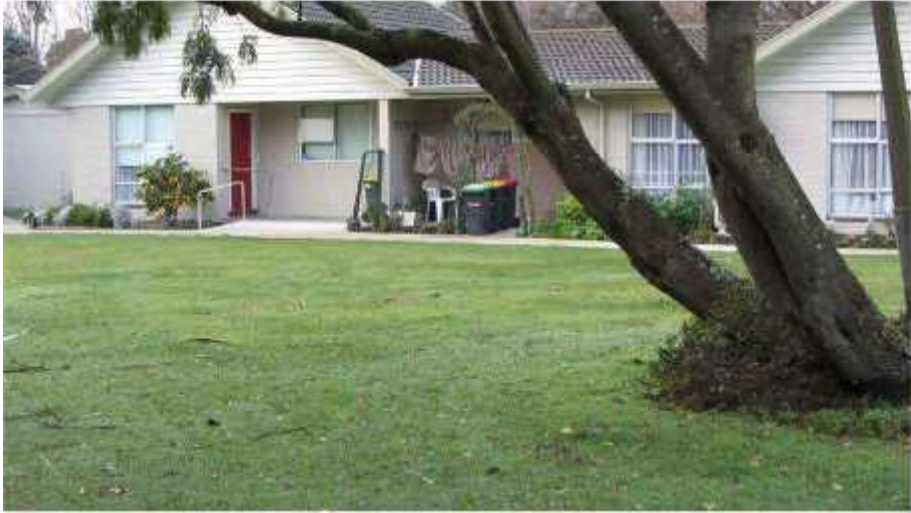
Photo 19: Shallow Depression in Front of Flats 1-3, Looking Northeast
