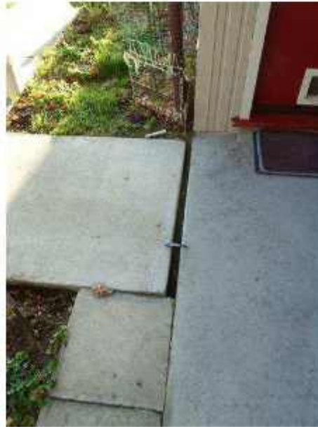
Photo 24: Displacement in Concrete Footpath at Front of Flat 15, Looking Northeast
