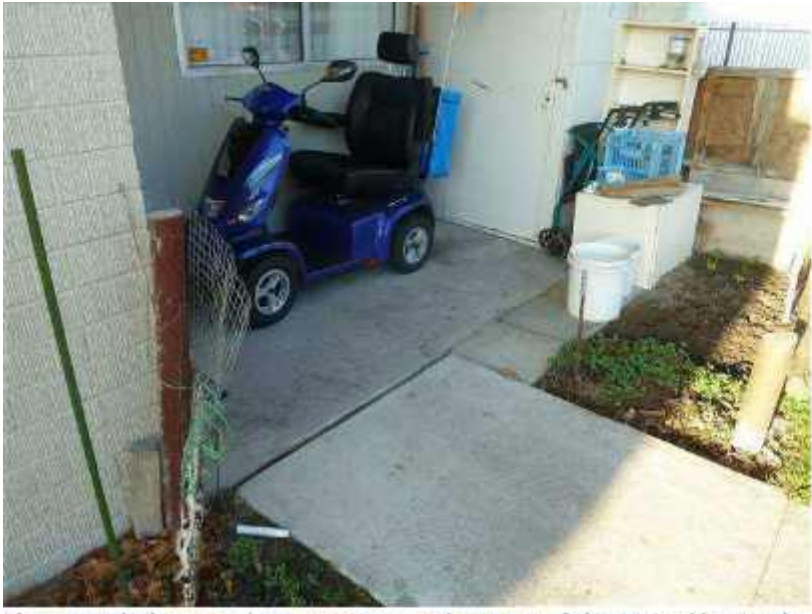
Photo 25: Displacement in Concrete Footpath at Front of Flat 15, Looking South
