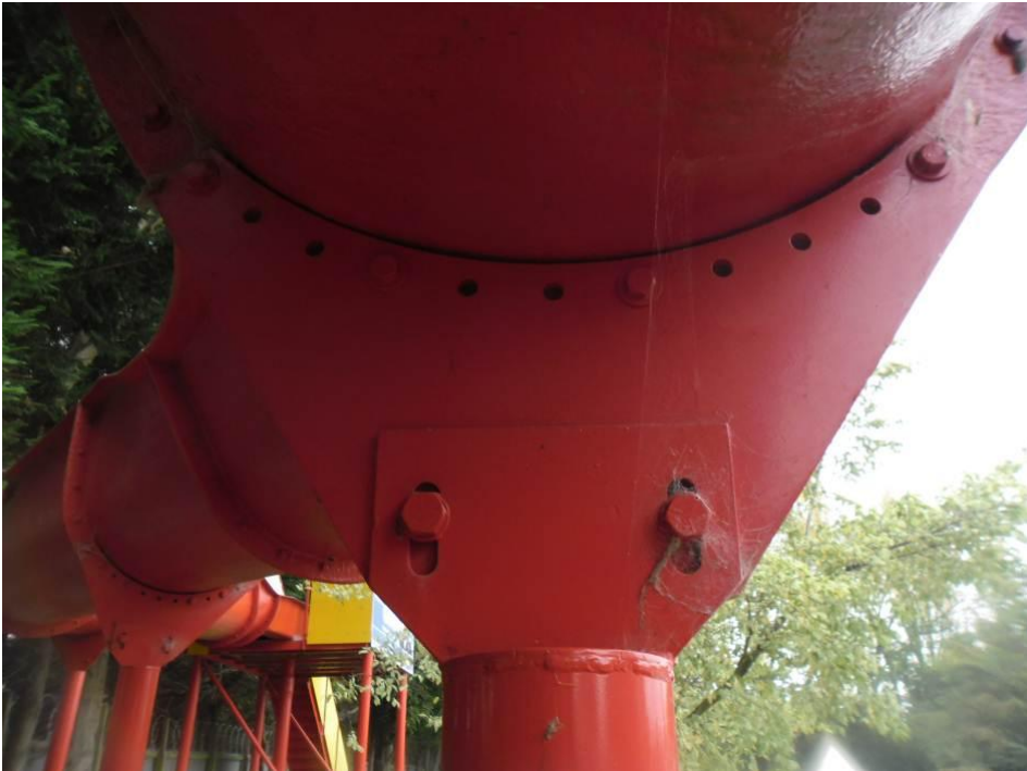
Photo 4: Connection between slide and cantilever support column
