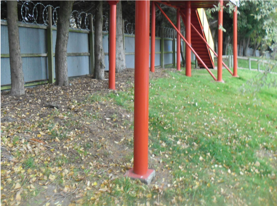
Photo 3: Exposed part of foundation
