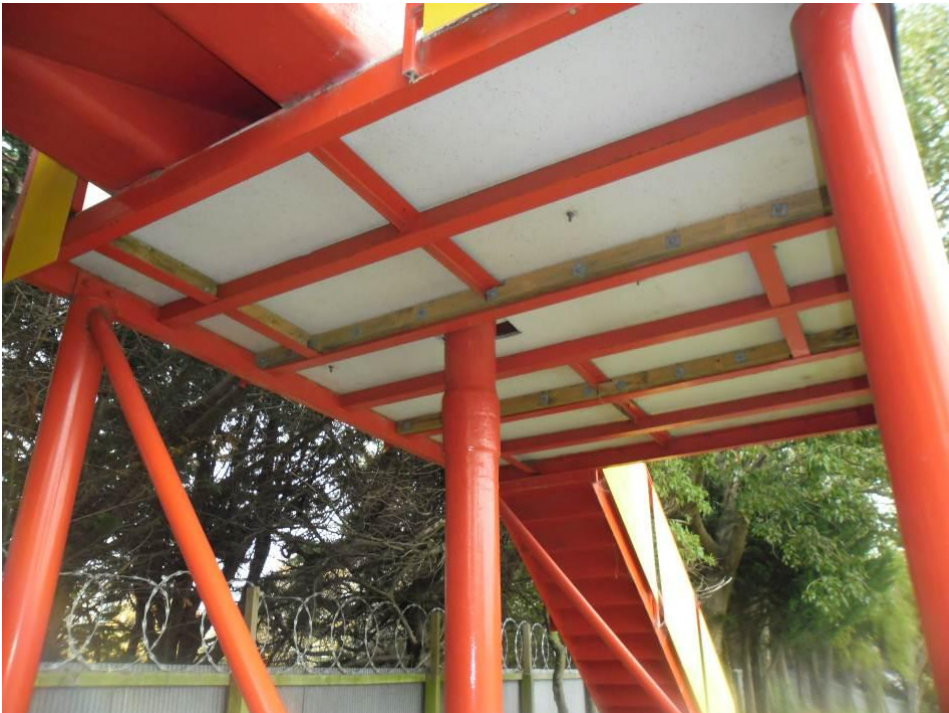
Photo 2: Underside of entrance platform
