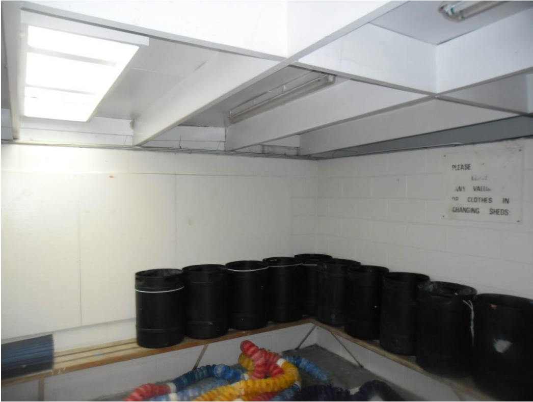
Photo 3: Internal view of changing room
