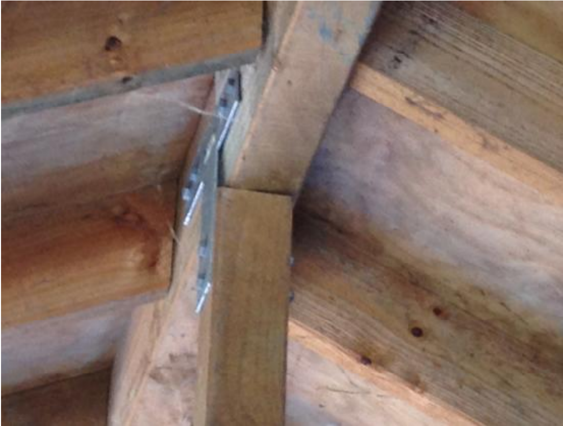
Photo 5: Ridge beam and rafter typical connection.
