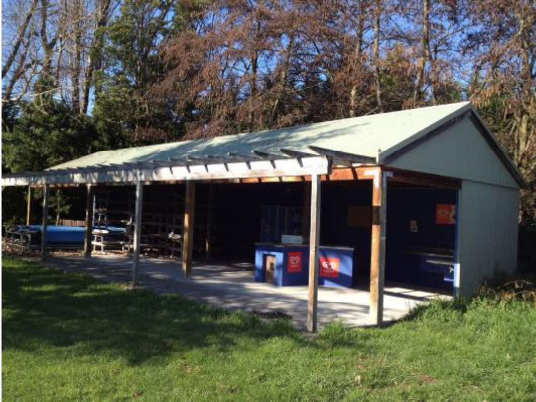
Photo 1: External view of the building with awning.
