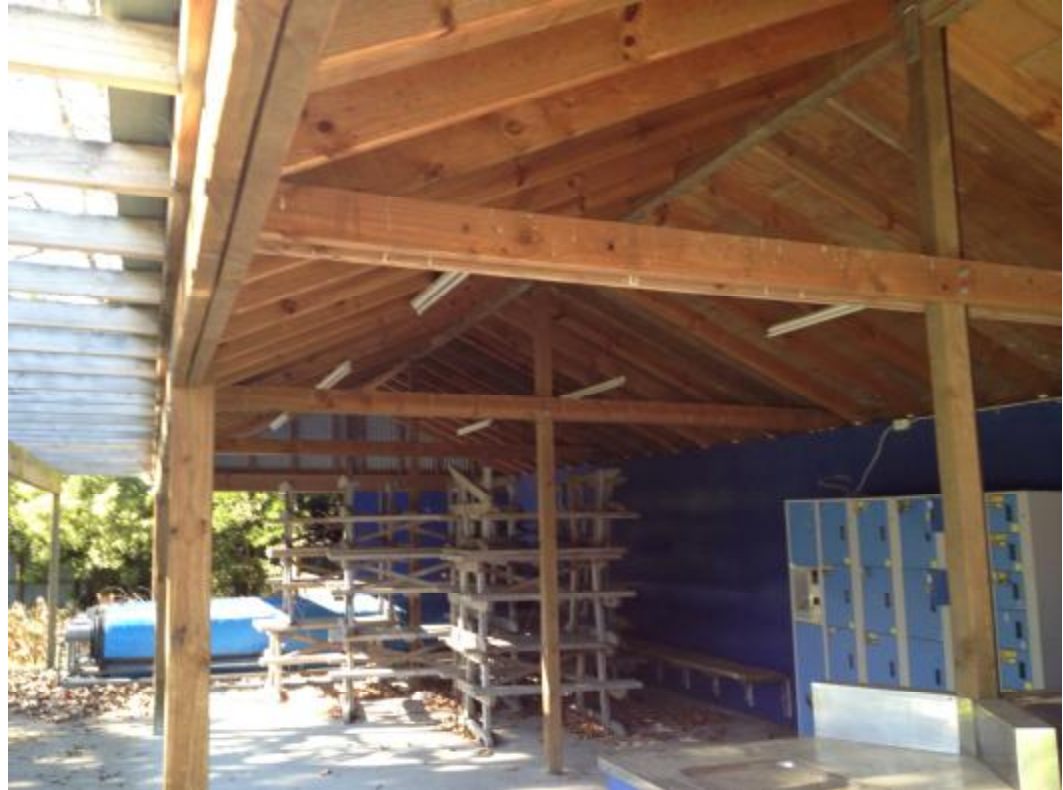
Photo 2: Internal view with the southern wall linings shown.
