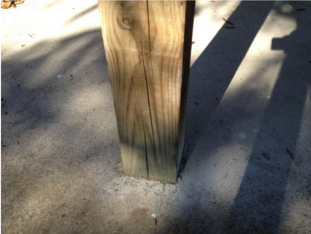
Photo 3: Timber column embedded into concrete slab.
