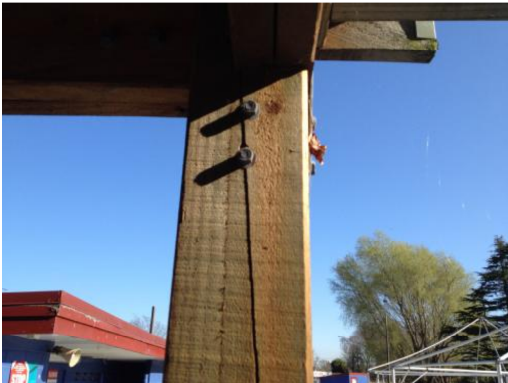
Photo 4: Typical column/beam connection
