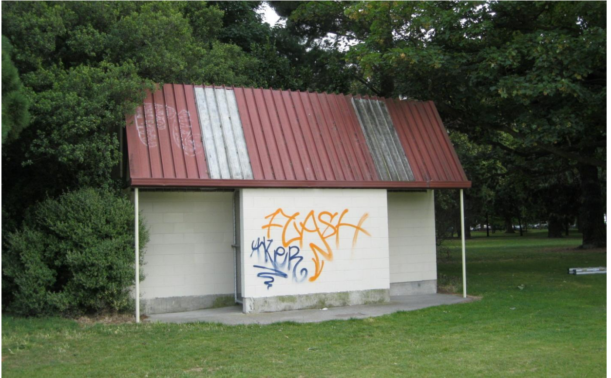
Photograph 1: Front (South) elevation of Hagley Park South Toilet Block
