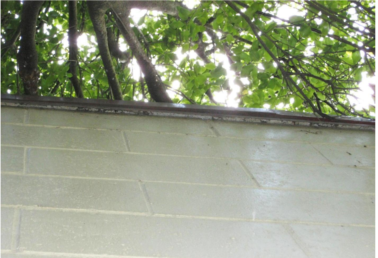
Photograph 27: Close-up view of gap between roof flashing and top of concrete masonry wall on West elevation
