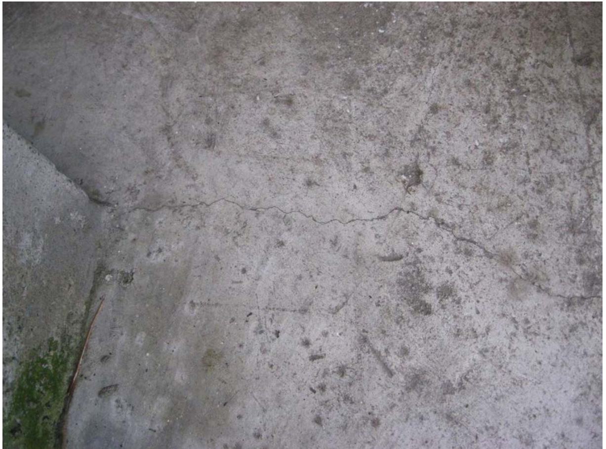
Photograph 16: Close-up view of crack in internal concrete floor slab
