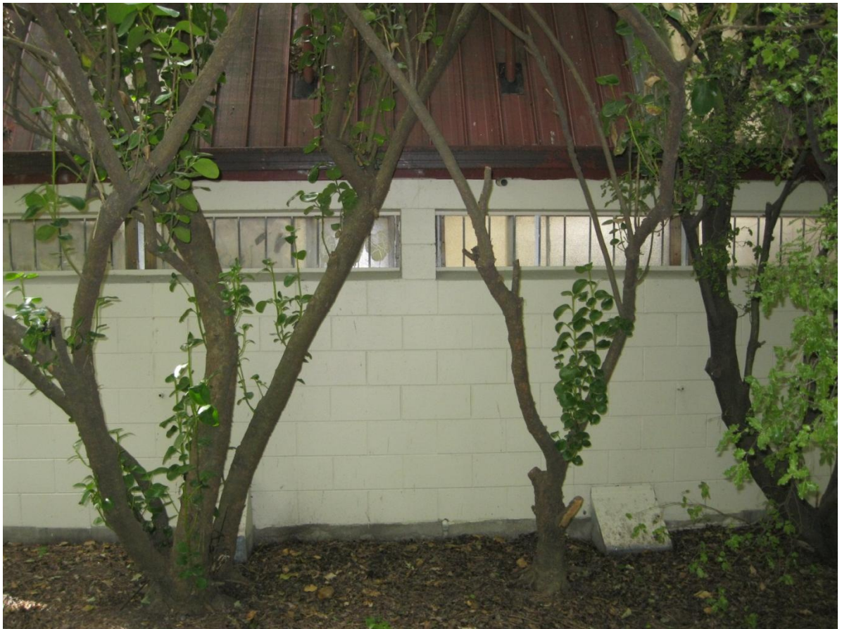
Photograph 3: Rear (North) elevation
