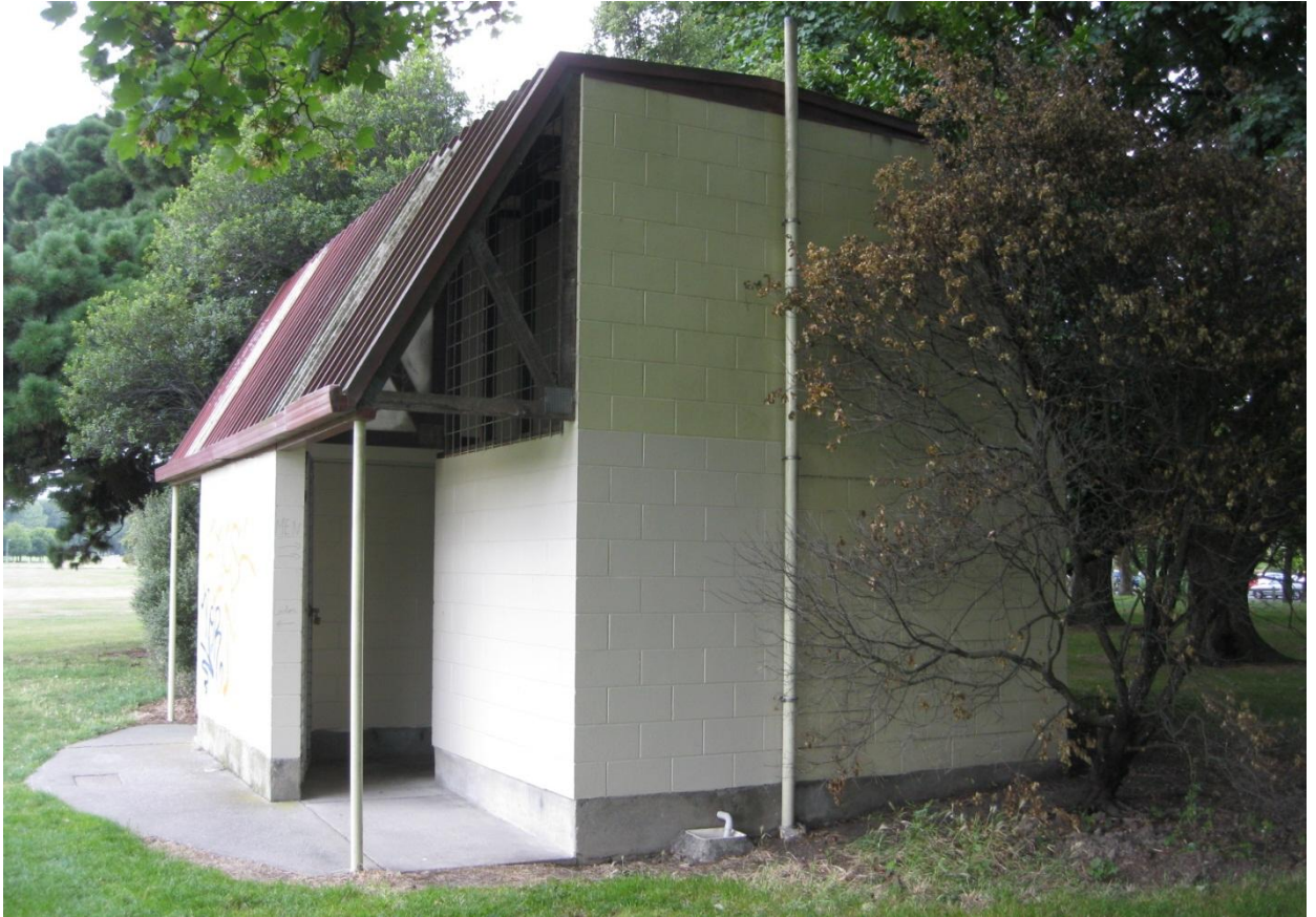
Photograph 5: East elevation with cantilevered concrete masonry wall
