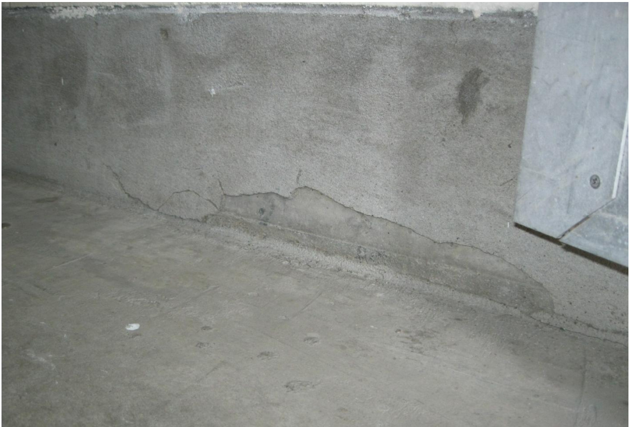
Photograph 19: Cracking and spalling of render on concrete footing to internal wall
