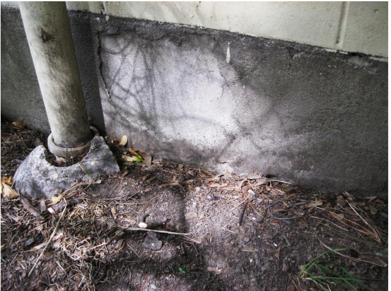
Photograph 26: Spalling of render on external concrete footing and movement of building shown by gap between concrete and drainpipe
