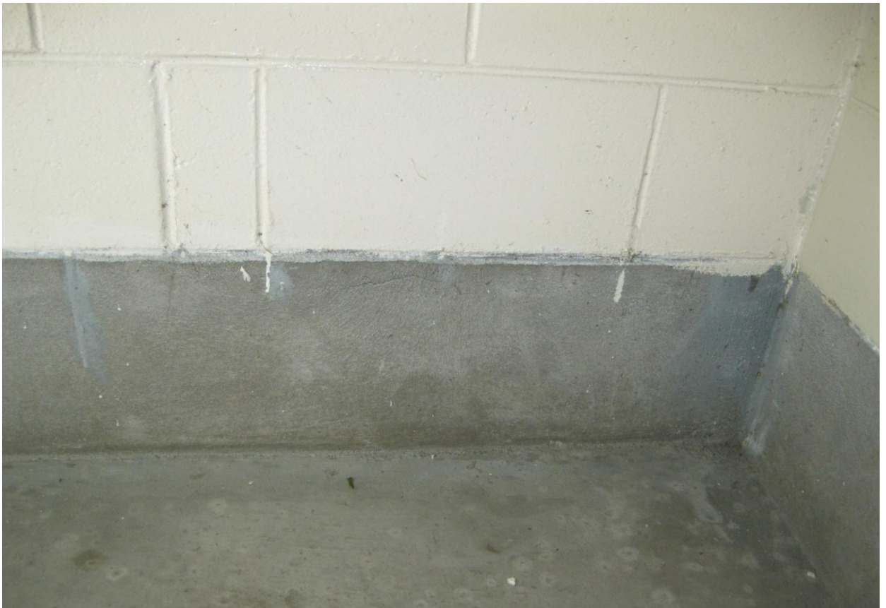
Photograph 21: Minor cracking in render on concrete footing to internal wall
