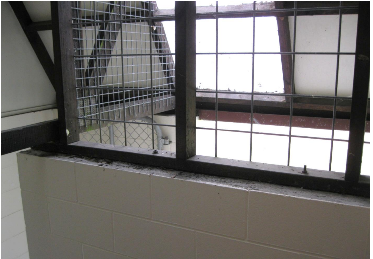
Photograph 9: Internal view showing timber roof framing fixed along top of fully filled concrete masonry walls
