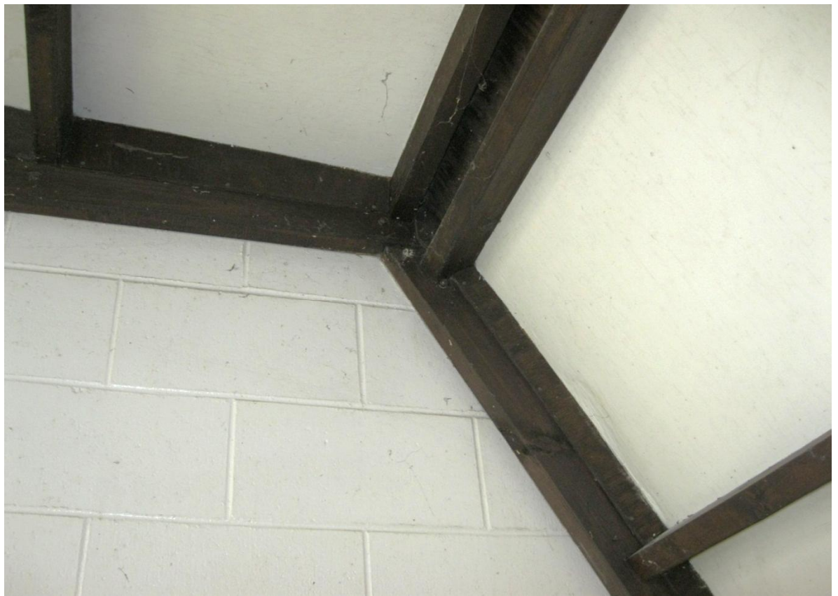
Photograph 12: Internal view showing fixing of timber roof framing to concrete masonry wall on western elevation
