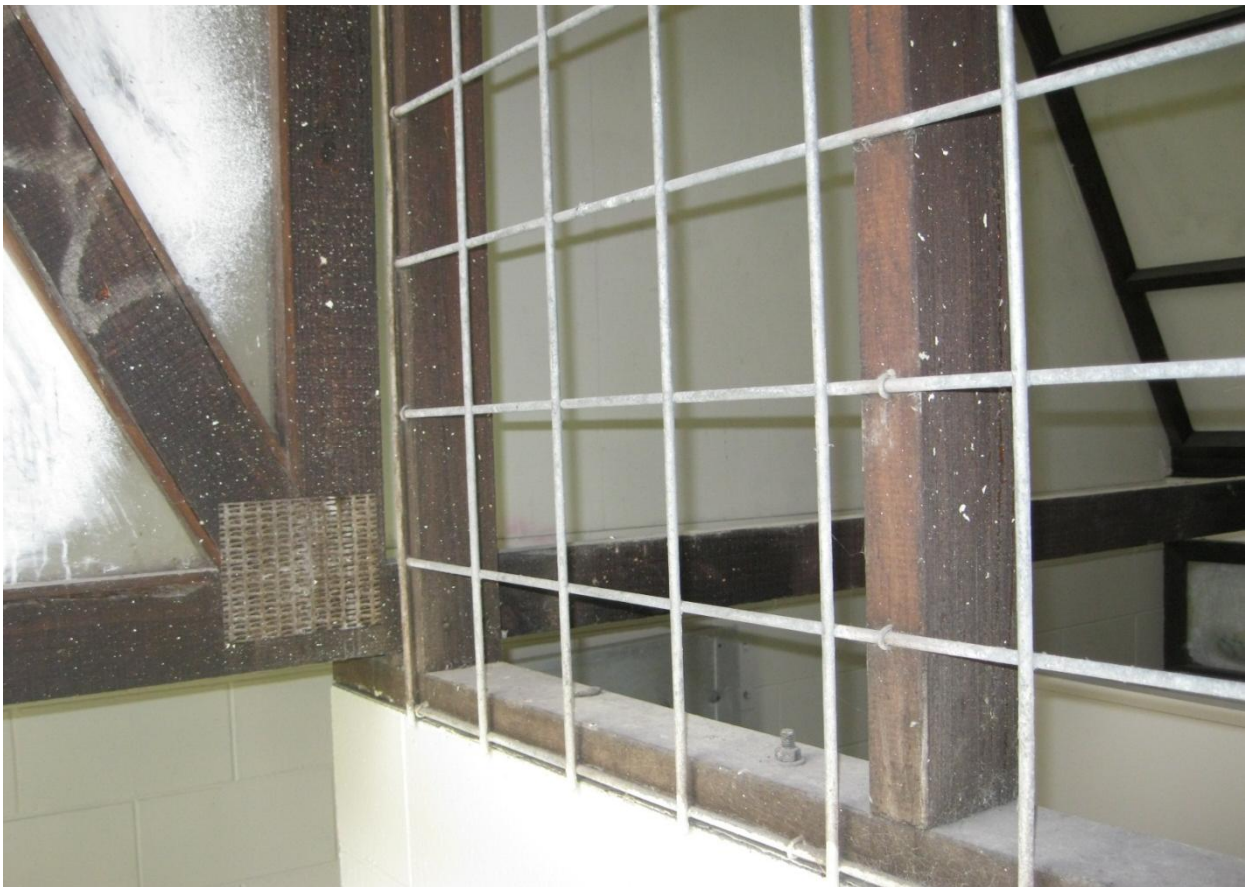
Photograph 10: Internal view showing nailplate connection detail of timber roof trusses
