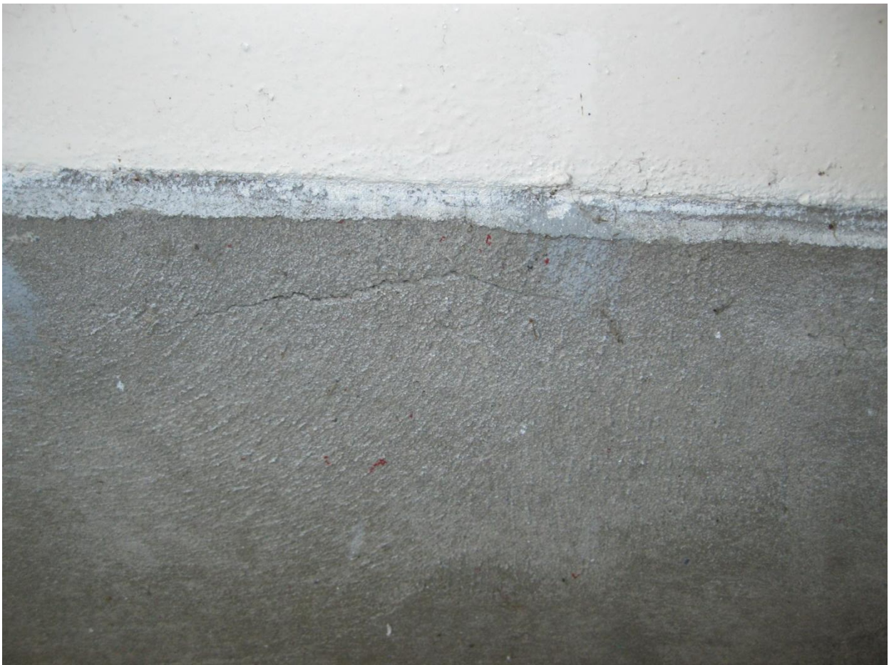
Photograph 22: Close-up view of minor cracking in render on concrete footing to internal wall
