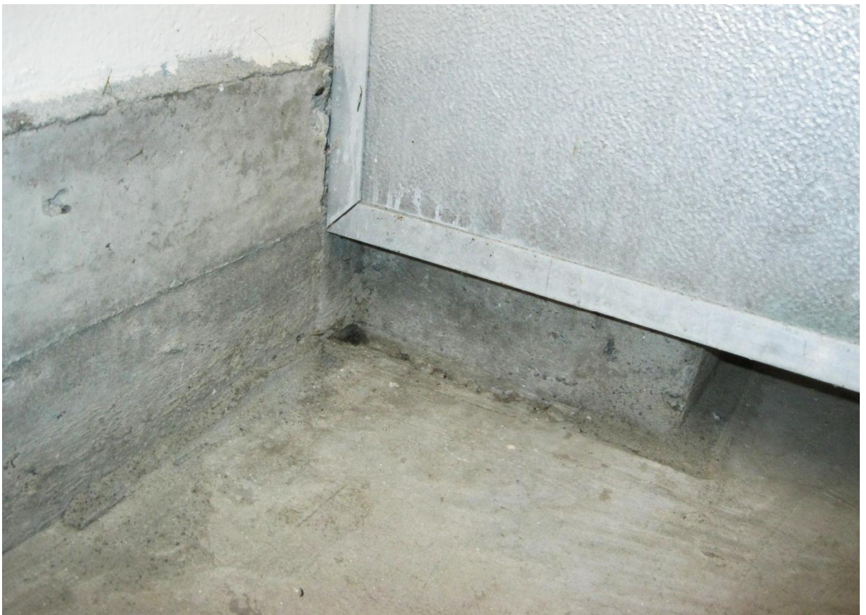
Photograph 24: Render spalled off concrete footing to internal wall
