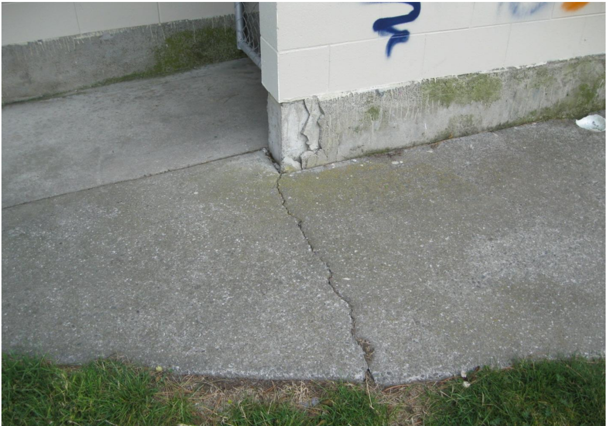
Photograph 13: Cracking in external slab and spalling of render on concrete footing to wall
