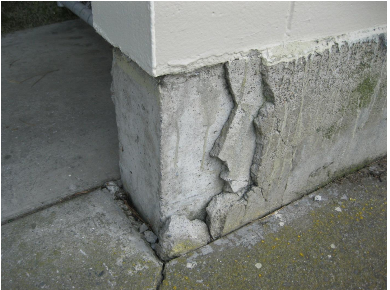
Photograph 14: Close-up view of spalling of render on concrete footing to wall
