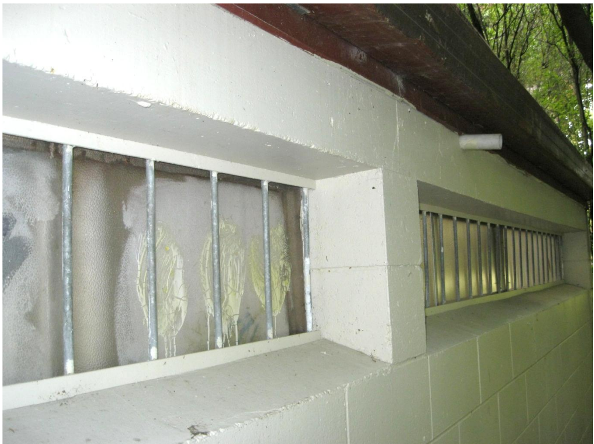
Photograph 4: Rear (North) elevation
