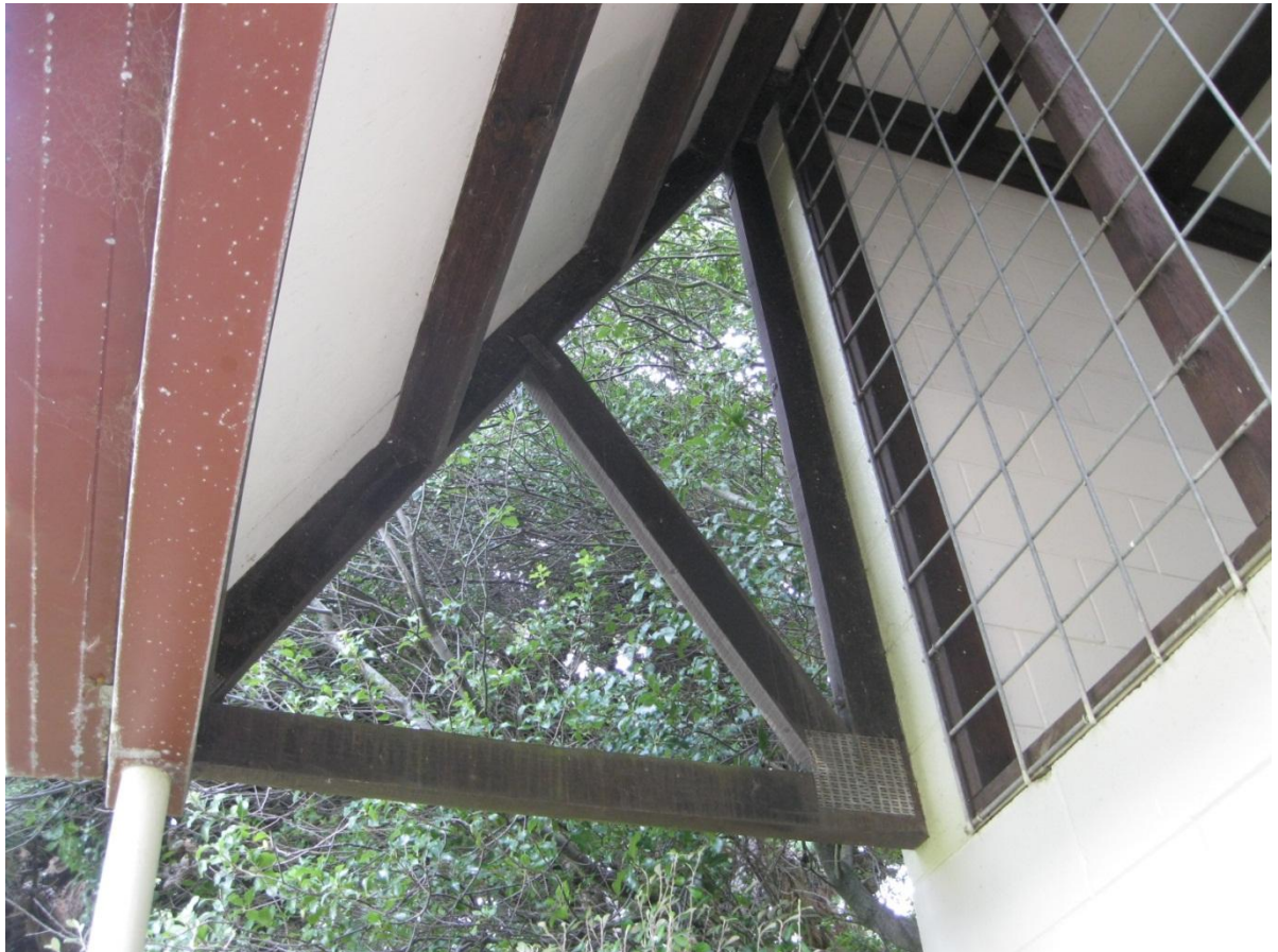
Photograph 7: View of timber truss supporting roof on West elevation at cantilevered wall
