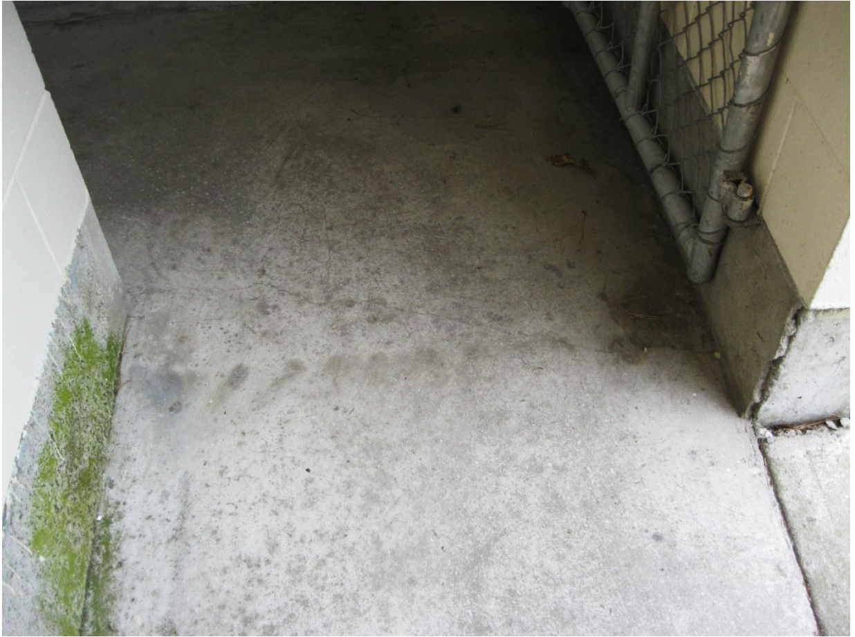
Photograph 15: View of crack in internal concrete floor slab
