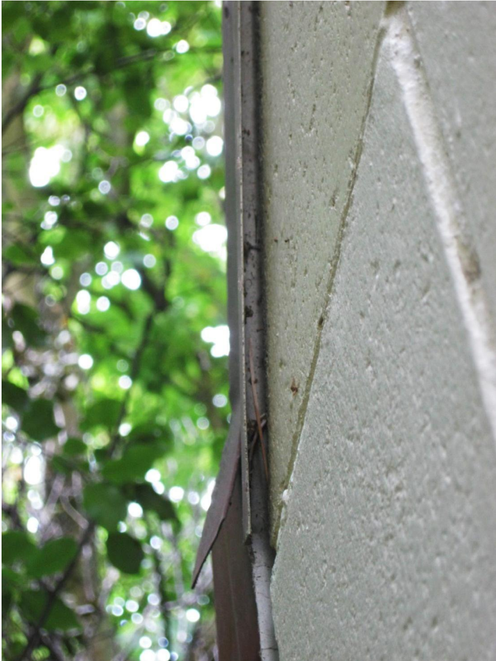
Photograph 29: Close-up view of gap between roof flashing and top of concrete masonry wall on West elevation
