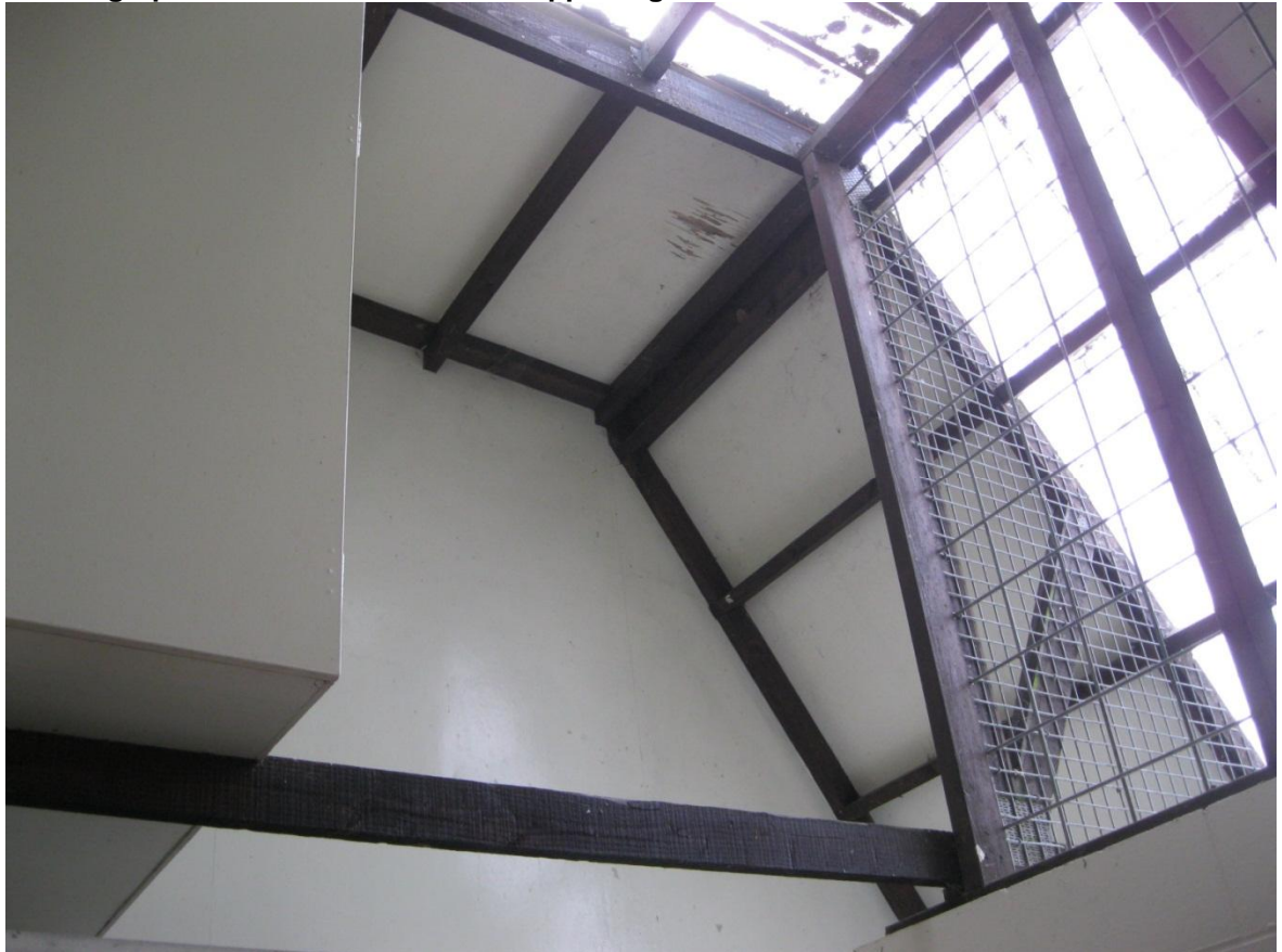
Photograph 8: Internal view with timber roof framing and plywood ceiling
