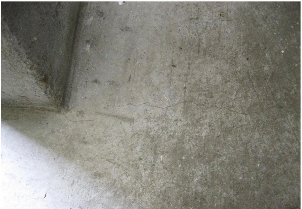
Photograph 18: View of crack in internal concrete floor slab
