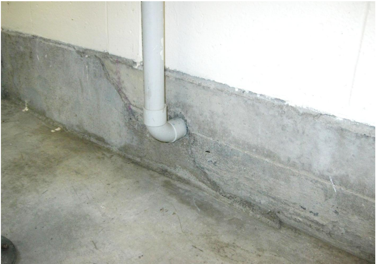
Photograph 23: Spalling of render on concrete footing to internal wall
