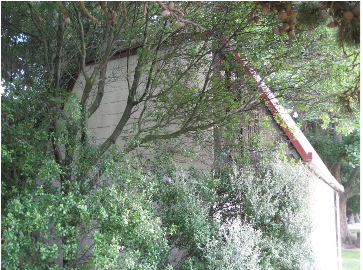
Photograph 6: West elevation with cantilevered concrete masonry wall
