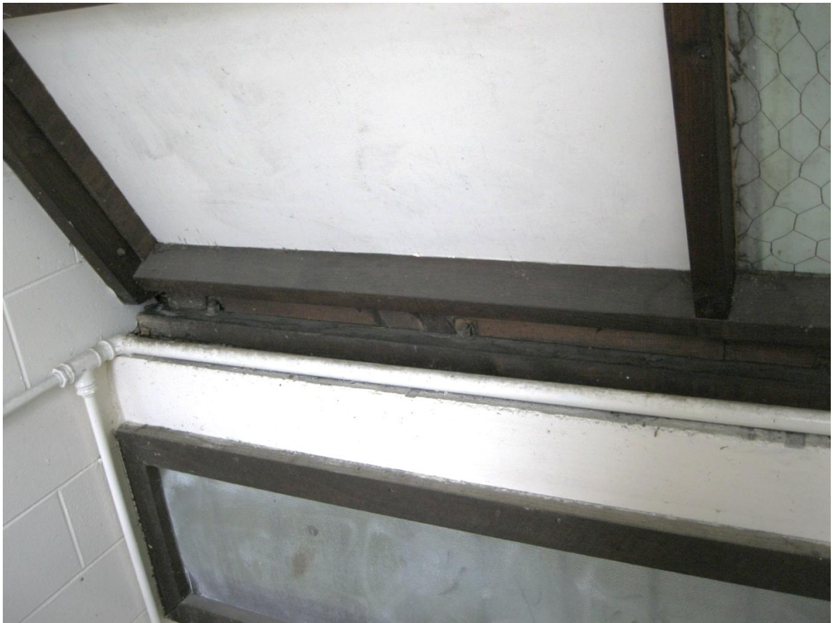
Photograph 11: Internal view showing fixing of timber roof framing to rear elevation concrete beam above window
