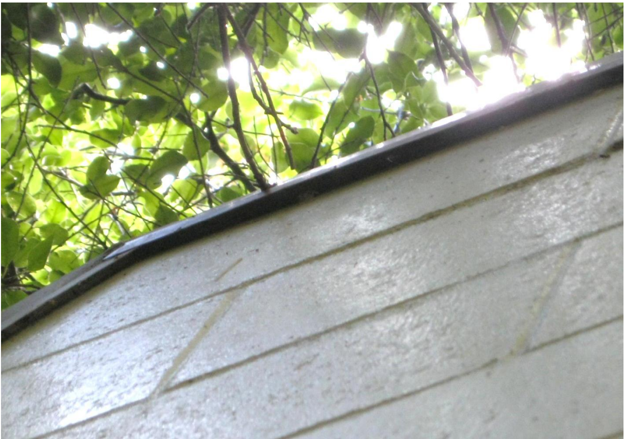
Photograph 28: Close-up view of gap between roof flashing and top of concrete masonry wall on West elevation
