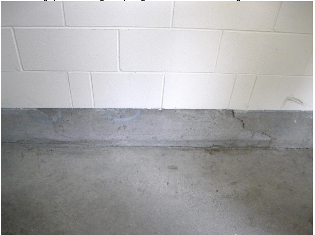
Photograph 20: Spalling of render on concrete footing to internal wall
