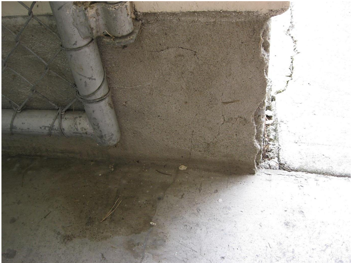
Photograph 17: Close-up view of crack in concrete floor slab and in render on footing to wall
