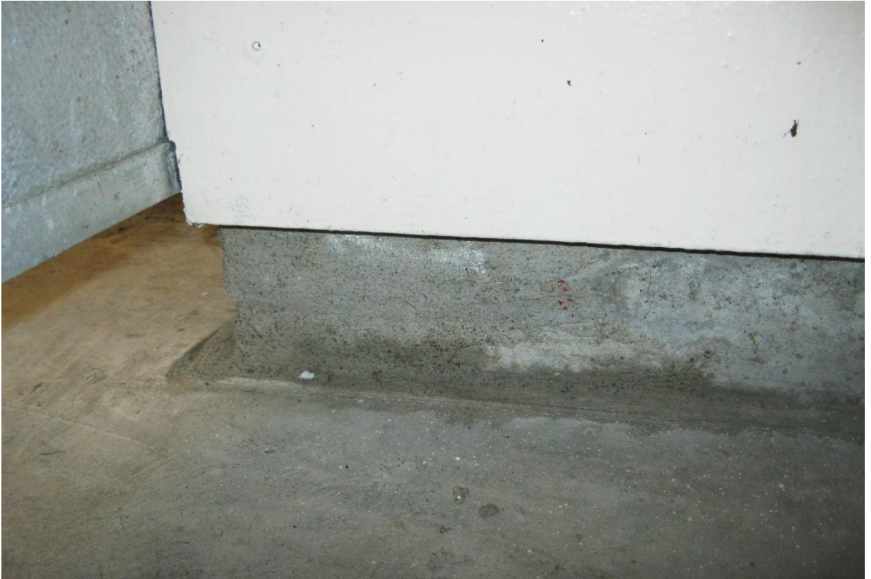
Photograph 25: Render spalled off concrete footing to internal wall
