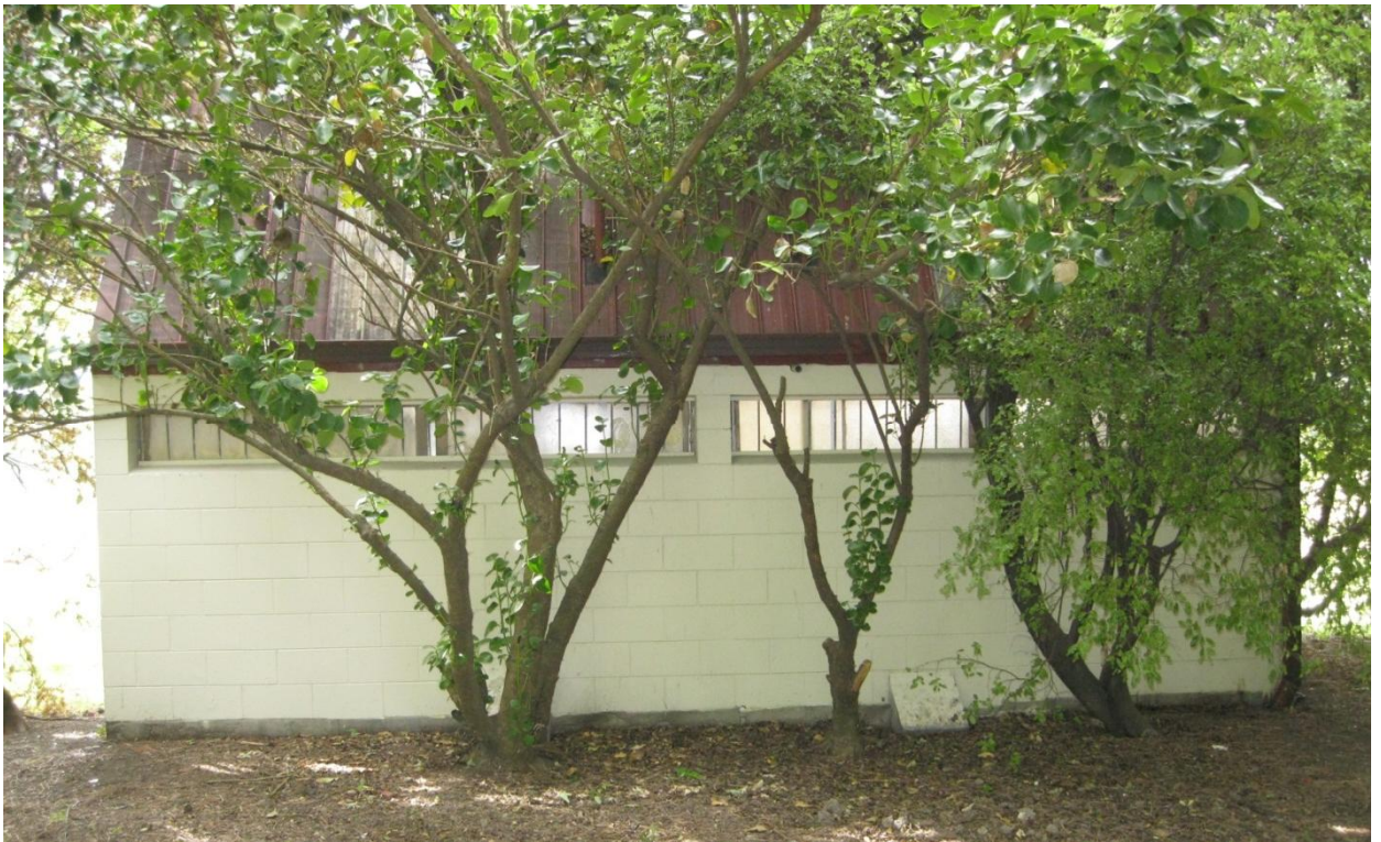
Photograph 2: Rear (North) elevation
