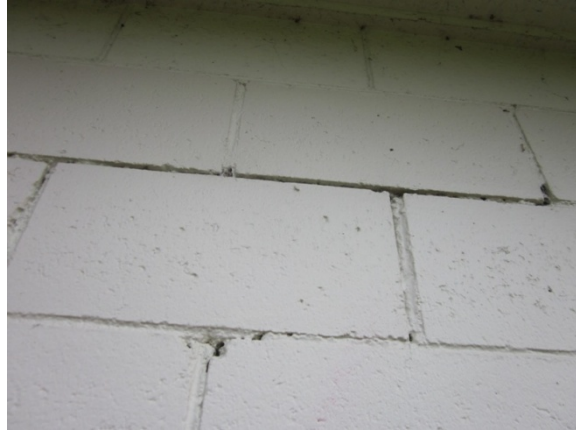
Photo 13: Existing low quality pointing of west masonry wall.
