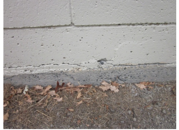
Photo 6: Hairline crack in concrete footing under west wall (typical).
