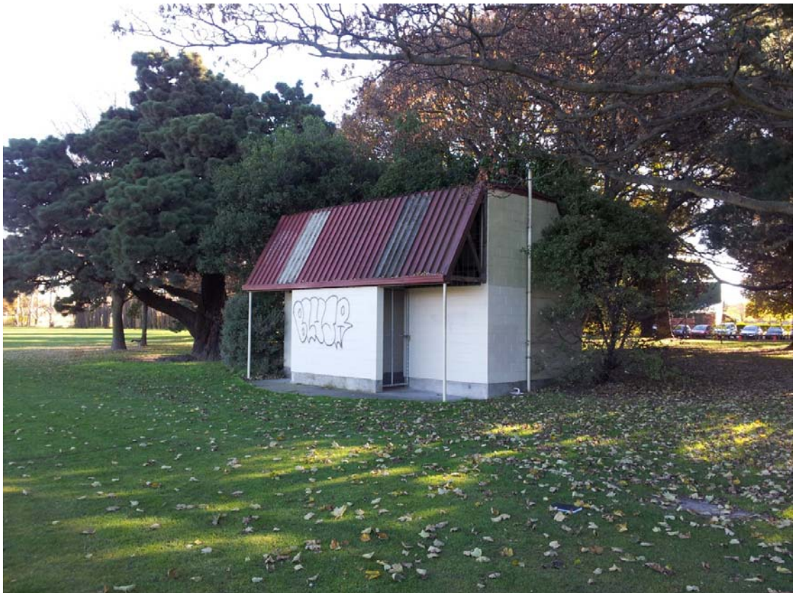
■ Figure 8 Overview of structures – Hospital toilet
