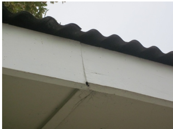
Photo 15: Existing warping of timber roof member on north side.
