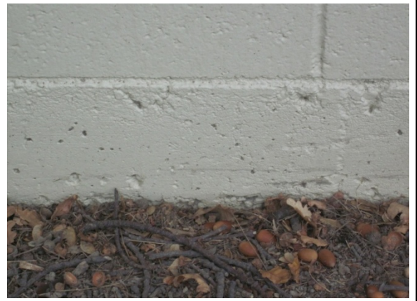
Photo 16: Existing spalling of concrete footing (typical).
