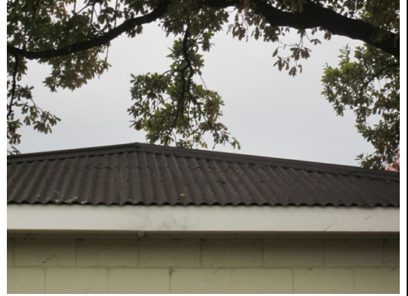
Photo 14: External roof cladding.
