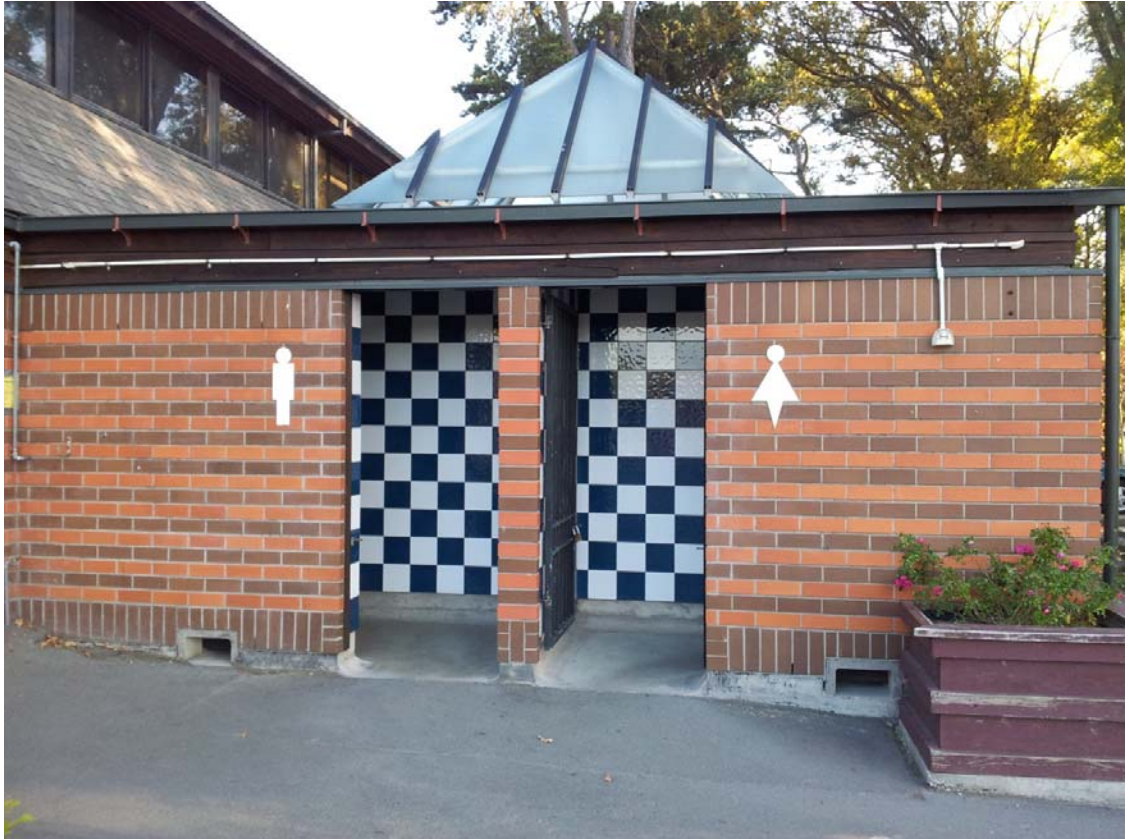
■ Figure 9 Overview of structures – Netball toilets
