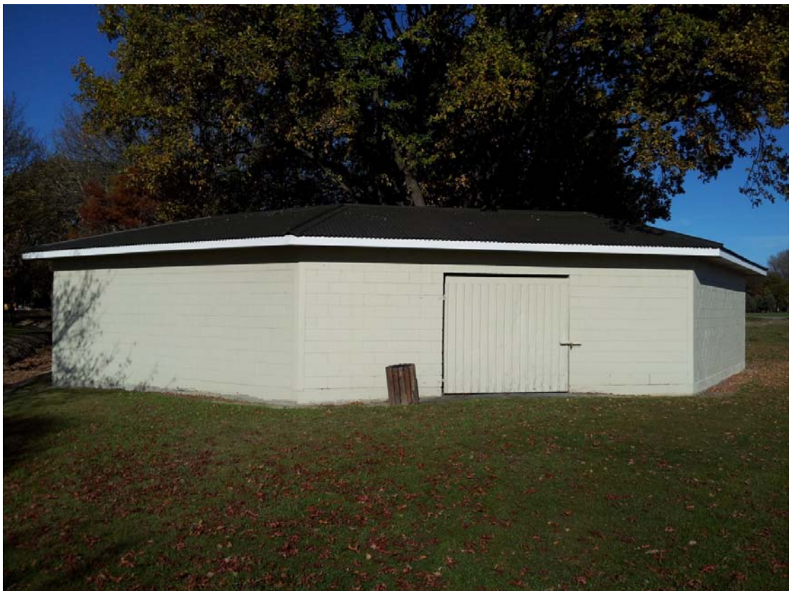
■ Figure 7 Overview of structures – Pavilion
