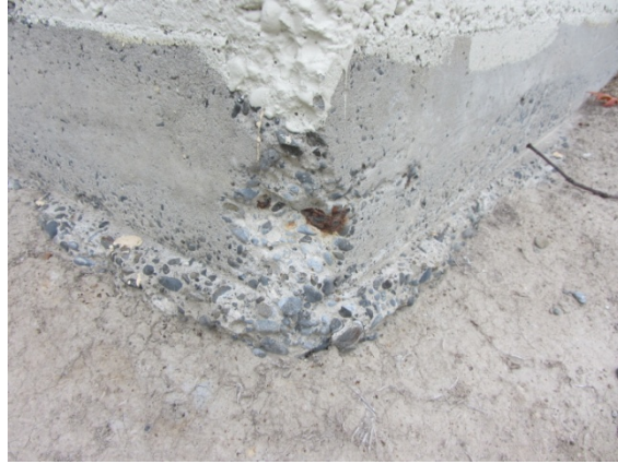
Photo 5: Existing impact damage to concrete footing on northwest corner, with rusted footing reinforcing exposed.
