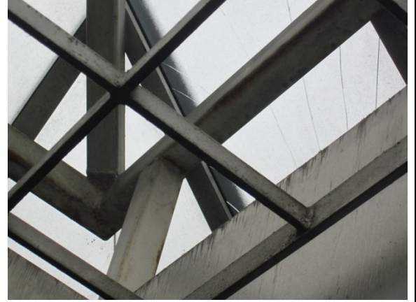
Photo 14: Cracked glass panel on west side of dome.
