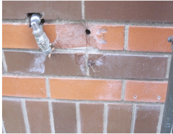
Photo 17: Existing damage to brickwork on west wall.
