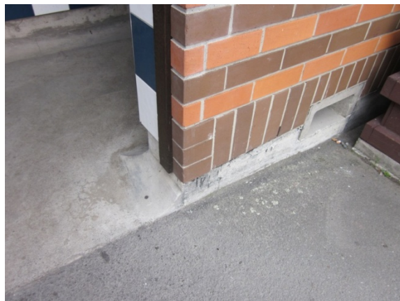
Photo 7: Concrete ground slab shown.
