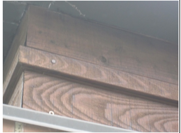
Photo 18: Crack in timber beam at roof level on southwest corner.
