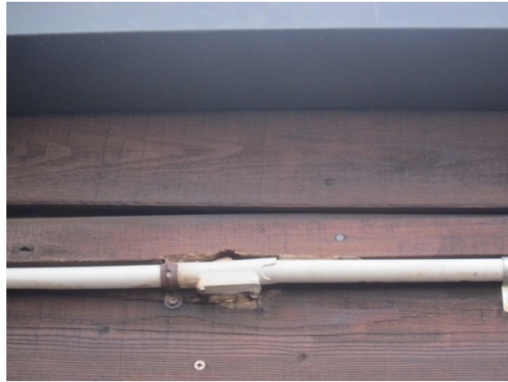
Photo 5: Existing damage to timber at cable level on north wall.
