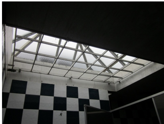
Photo 11: Ceiling under glass dome.
