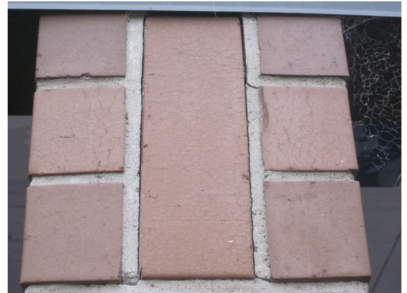
Photo 6: Gaps opening up between masonry and bricks at the top of the column on the north wall.
