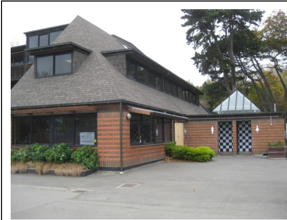
Photo 1: North elevation of Christchurch Netball Centre building and toilet block
