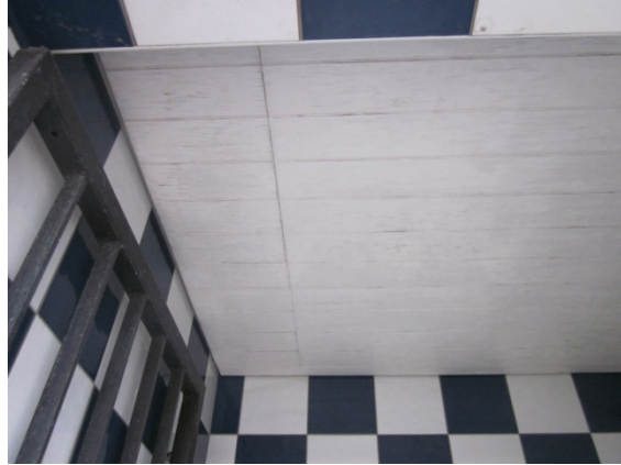
Photo 9: Timber ceiling cladding.
