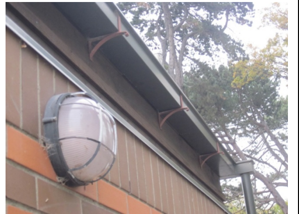
Photo 16: Timber beam and gutter running along building at roof level.
