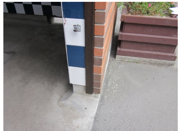
Photo 8: Concrete wall with external brick cladding and internal tile cladding.
