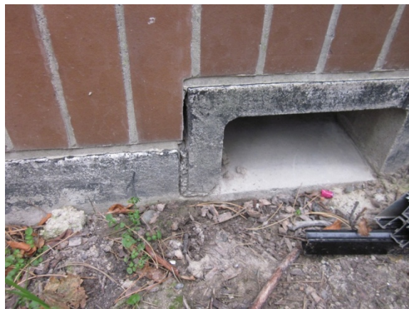
Photo 19: Existing mortar removal on south wall.
