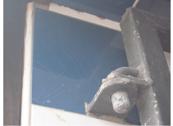
Photo 10: Cracks in the tile believed to have been caused by impact load on the door as it is connected to the concrete directly behind the tile, and no other tile was cracked.
