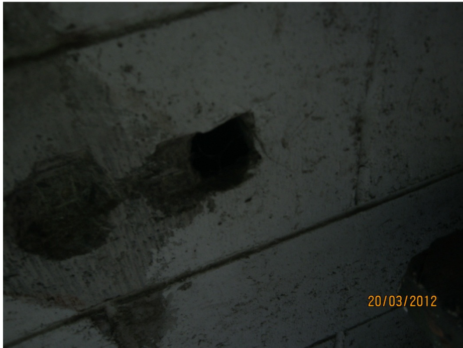
Photo 5: Existing hole in block wall – ungrouted
