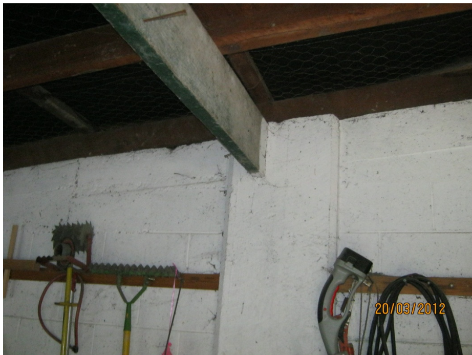
Photo 10: Roof framing of Implement Shed
