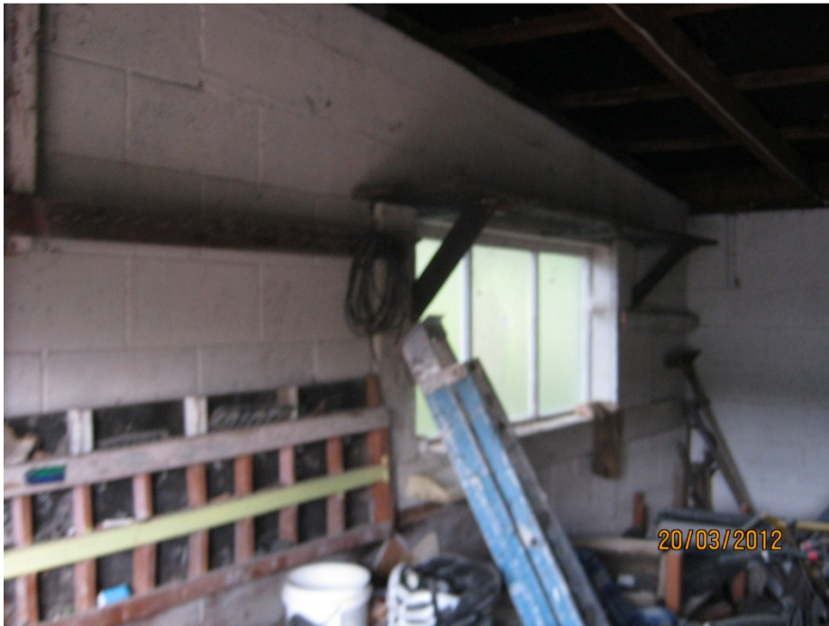
Photo 7: Interior of Implement Shed
