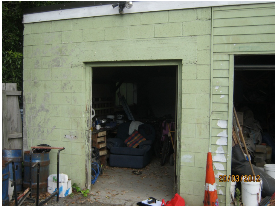
Photo 1: North elevation of the Implement Shed
