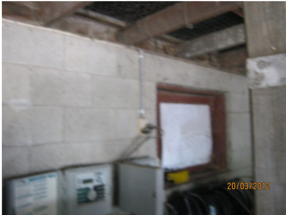
Photo 9: Roof supports of Implement Shed
