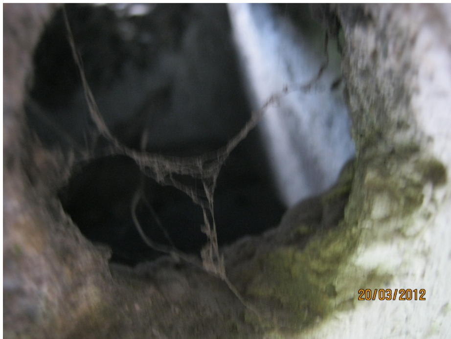
Photo 6: Existing hole in block wall – ungrouted (close-up)
