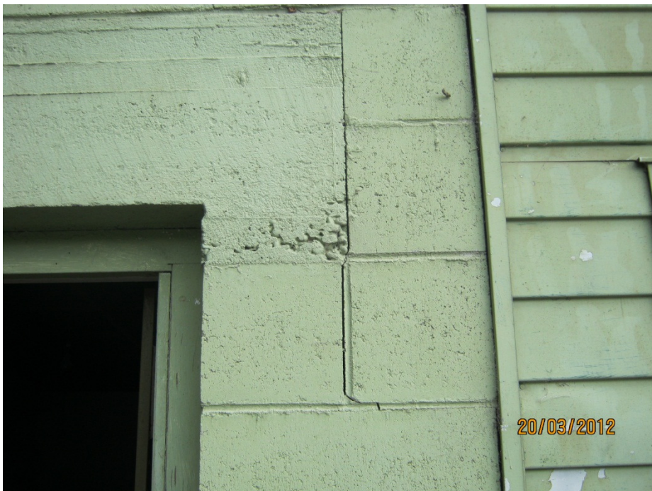
Photo 4: Crack at edge of concrete lintel
