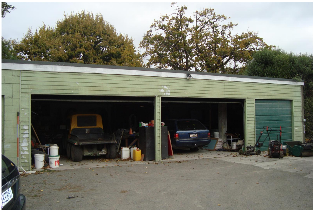
Photo 2: North elevation of the Implement Shed
