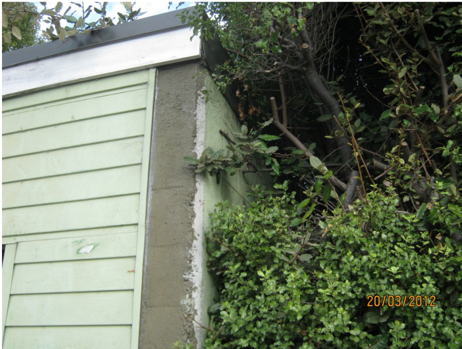
Photo 3: North-west corner of the Implement Shed
