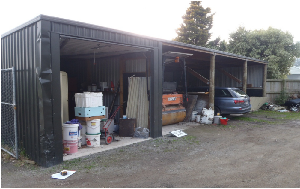
Photo 1: Front View of Building
