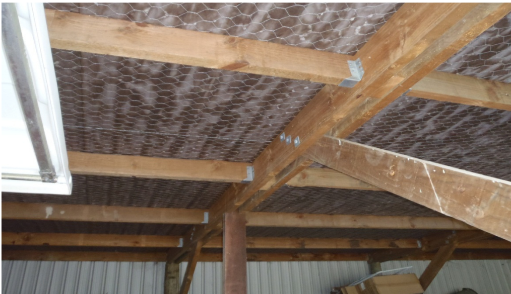
Photo 4: View of Roof Detail
