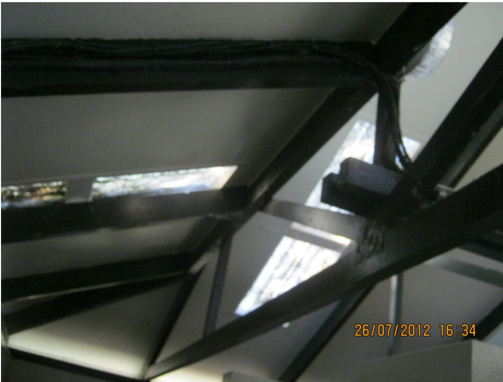
Photo 4: View of the roof of the east/west side joining to the main trusses
