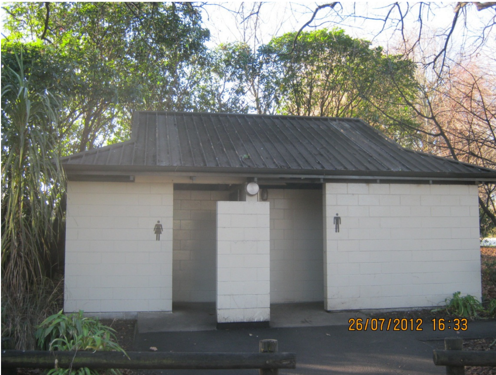
Photo 1: The north wall of the building
