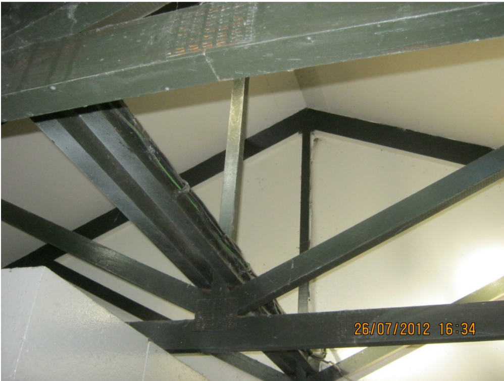
Photo 3: View of the roof truss
