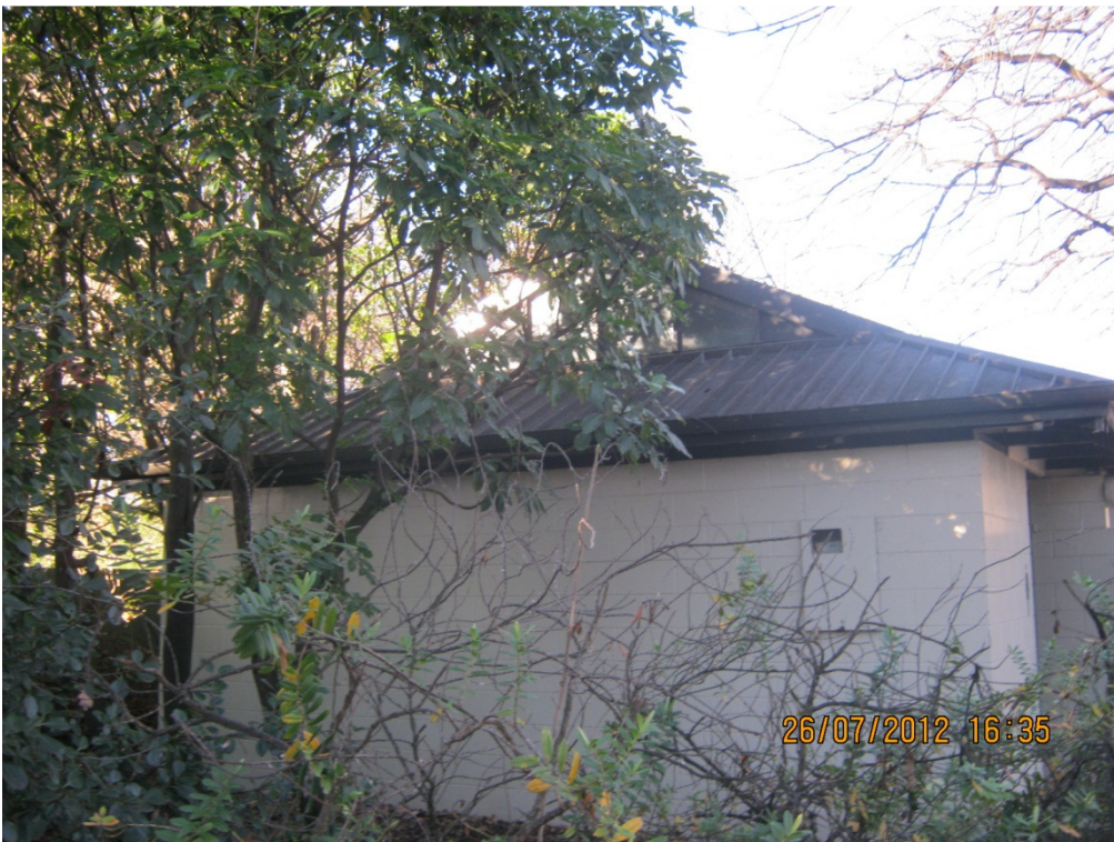
Photo 2: The east wall of the building
