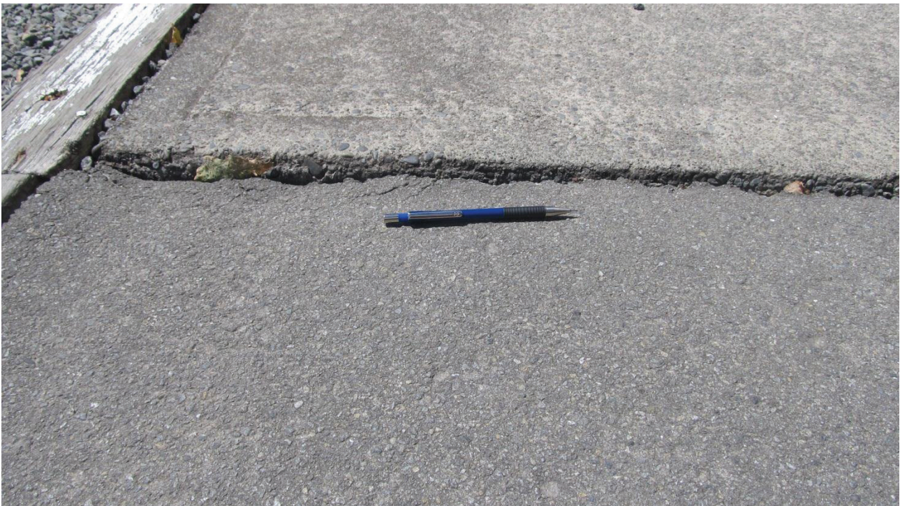
Photo 4: Upto 10mm of vertical and horizontal displacements of concrete paving.
