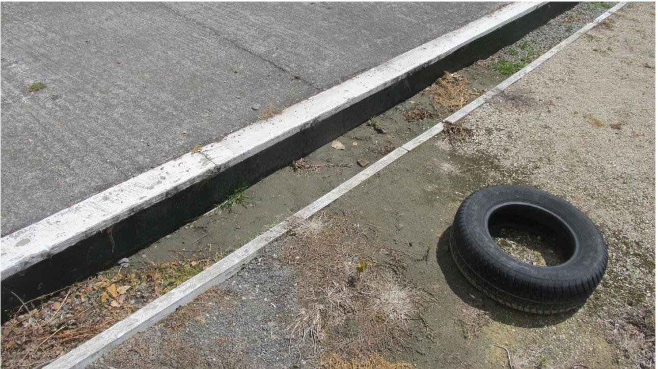
Photo 8: Approximately 1m 2 of liquefaction.
