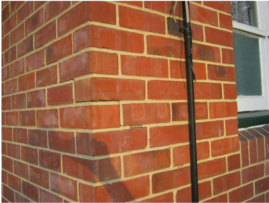
Step cracking on north west corner
