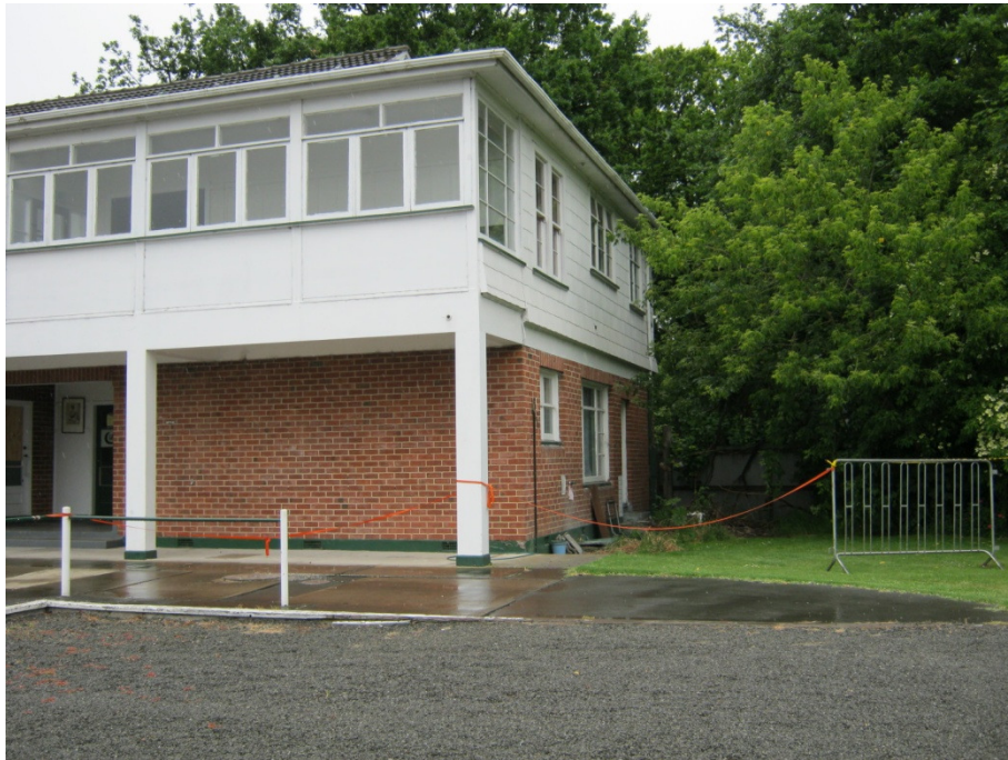
Western Side of Building
