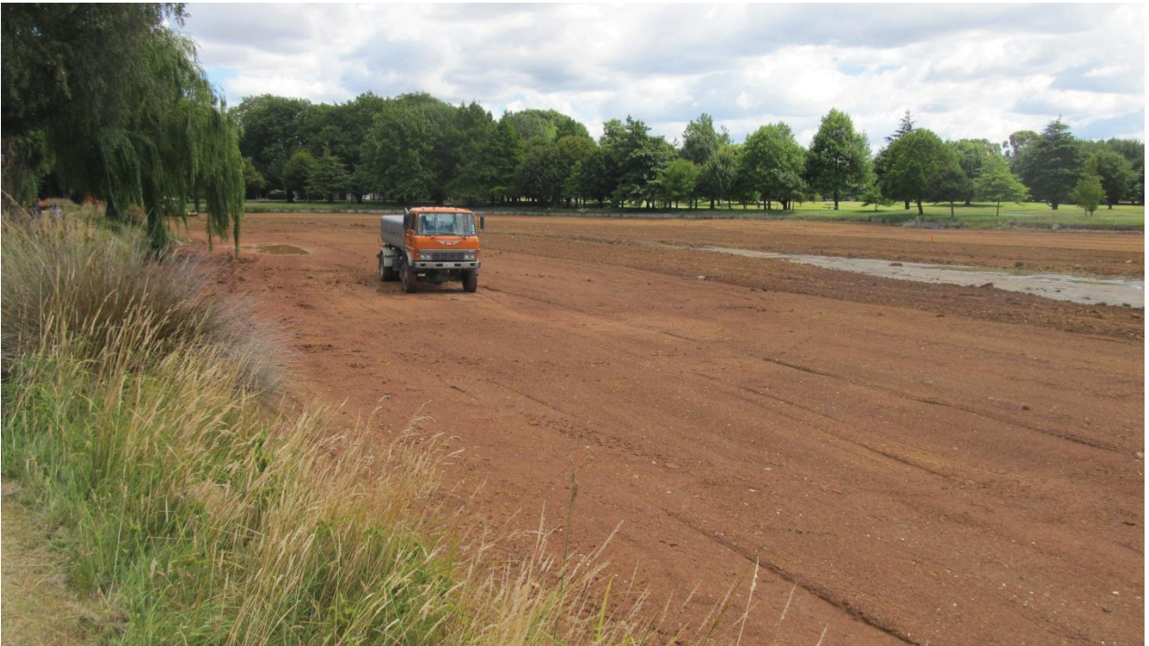
Photo 10: New liner in Victoria Lake.
