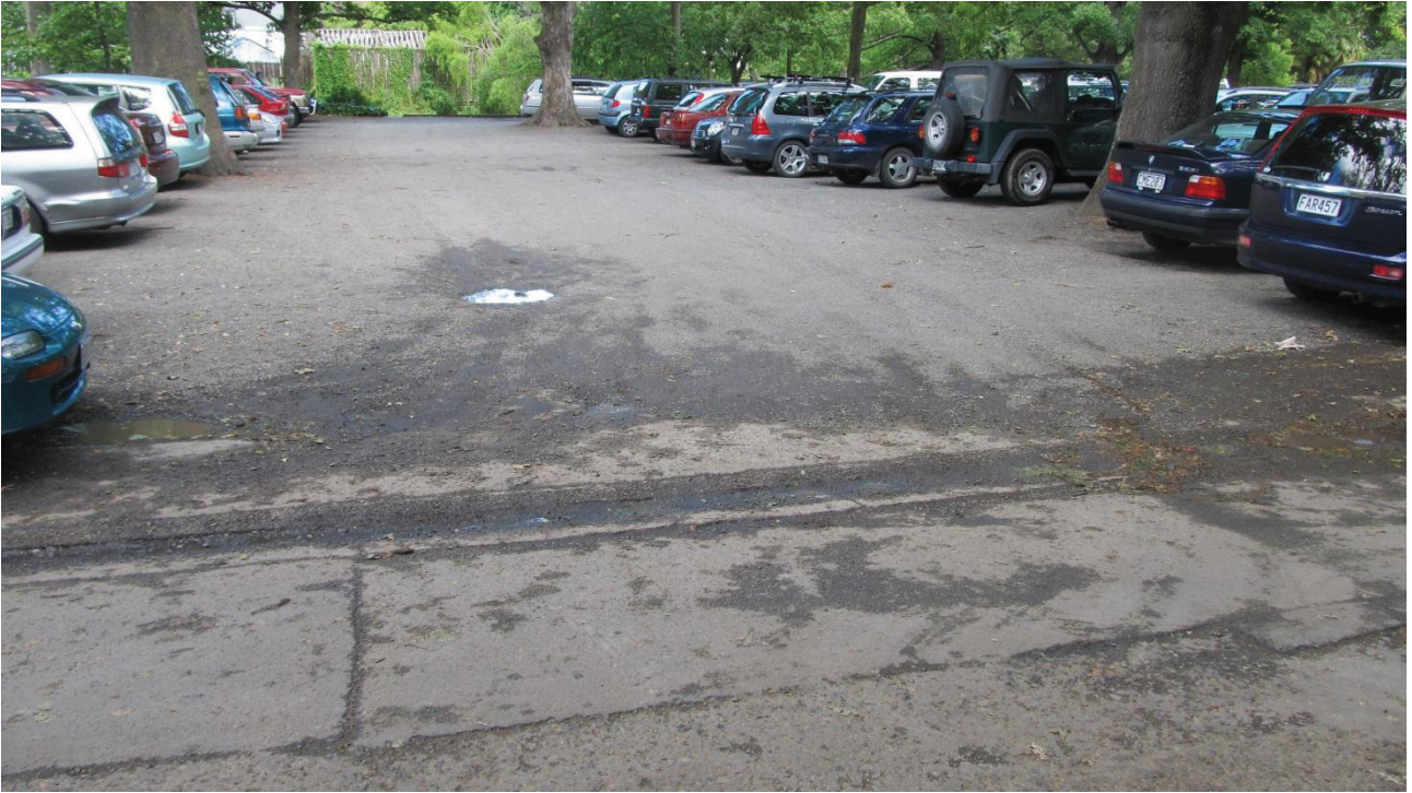
Photo 9: No evidence of cracking and heaving due to the earthquakes.
