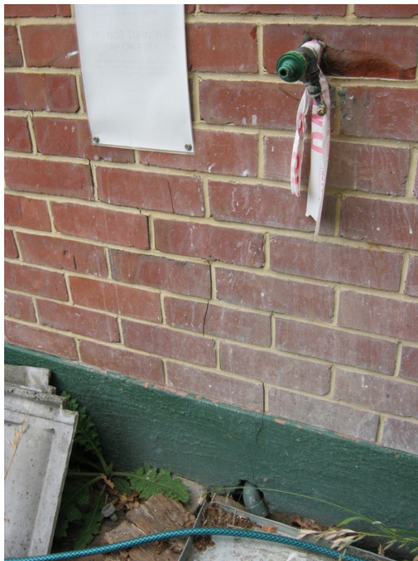
Foundation Damage
