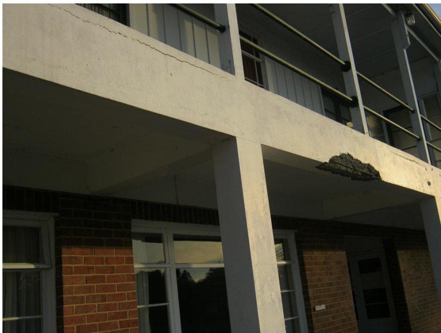
Spalled concrete on First Floor balcony
