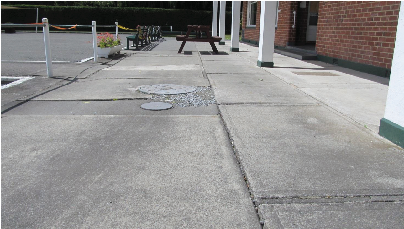
Photo 3: Localised settlement of footpath (10mm-50mm) and manhole uplift (10mm to 20mm).
