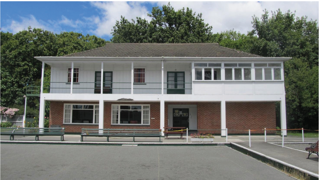
Photo 2: North elevation of the building.
