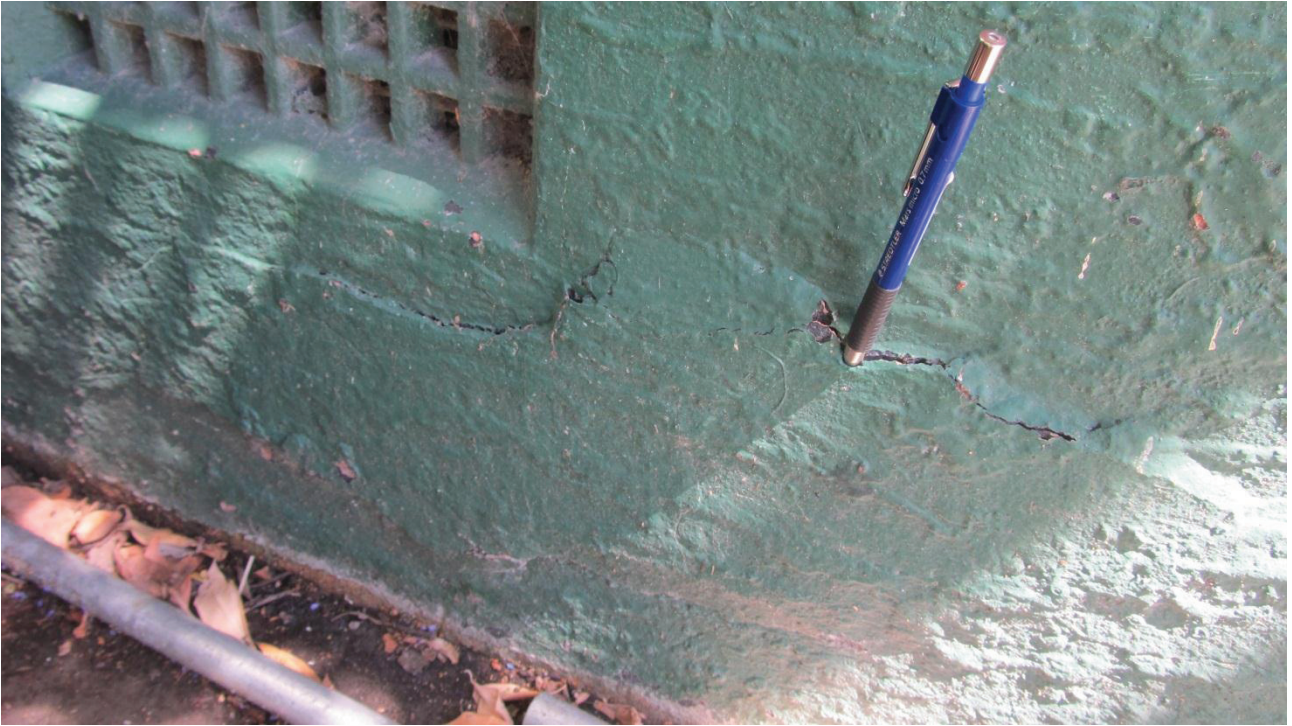
Photo 7: Possible superficial damage to east foundation.
