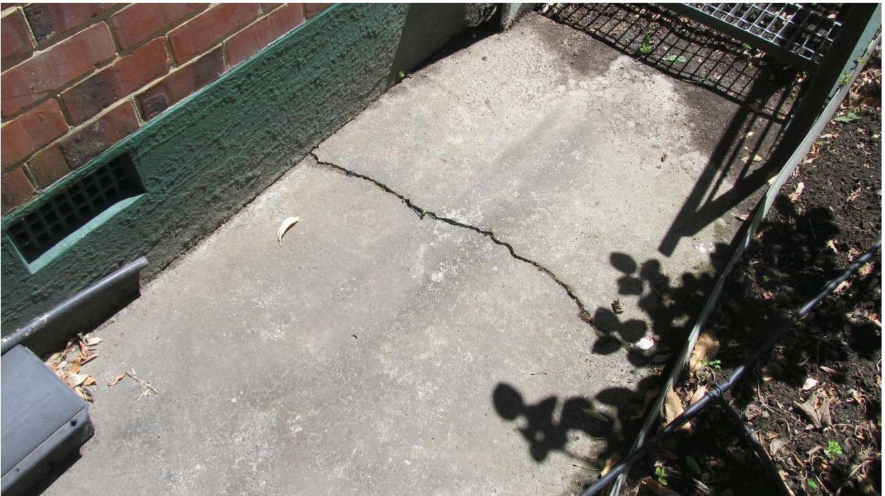
Photo 6: 10mm crack across footpath at east elevation.
