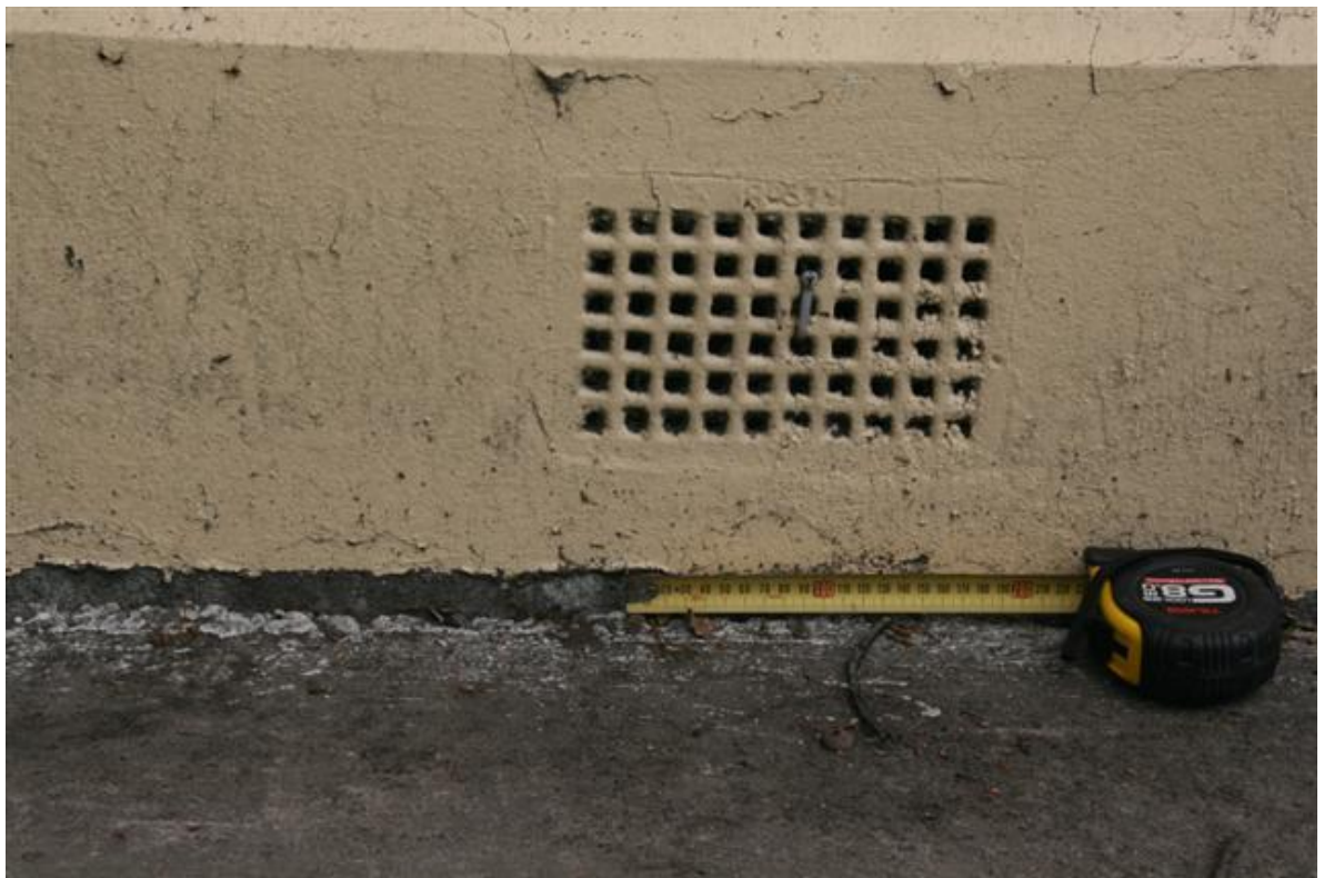
Photo 2: The concrete footpath on the east elevation has settled approximately 20mm.
