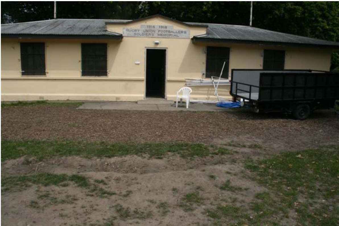
Photo 1: North elevation of the North Pavilion.
