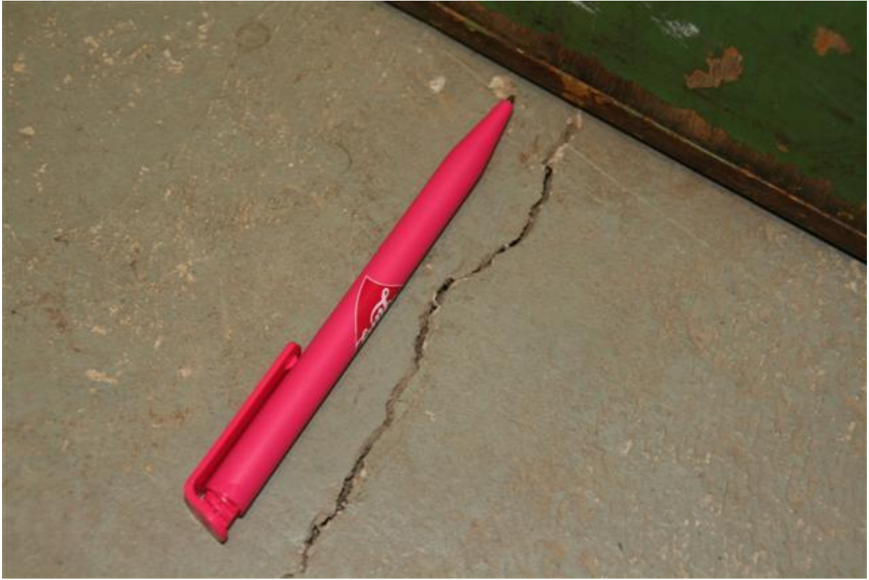
Photo 5: Internal floor crack that is approximately 2mm wide.
