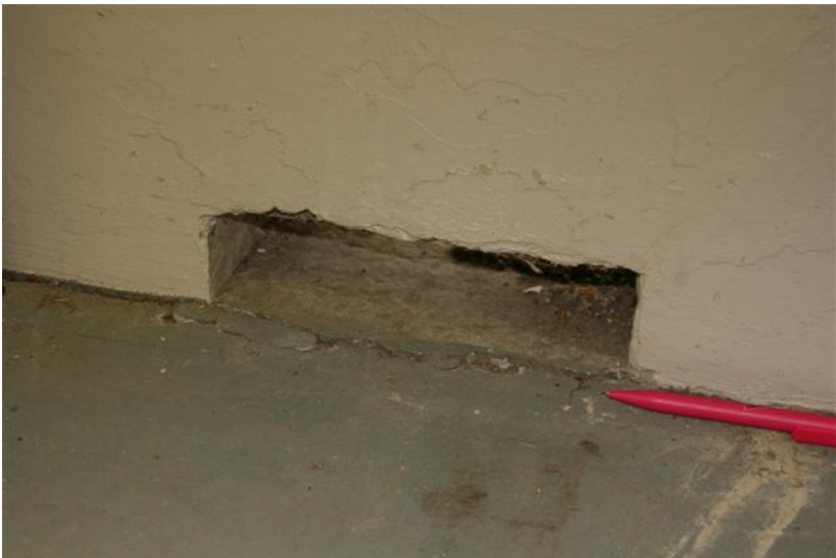
Photo 4 : The floor slab has settled approximately 5mm.
