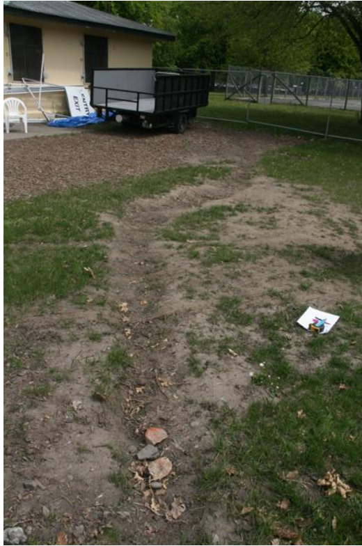
Photo 3: The ground surrounding the water pipe has settled by approximately 50mm.
