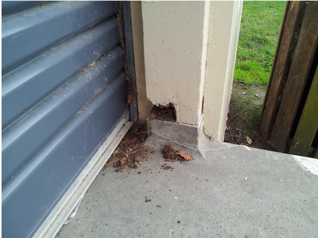
■ Figure 8 Observed impact damage to timber column on the northern side
