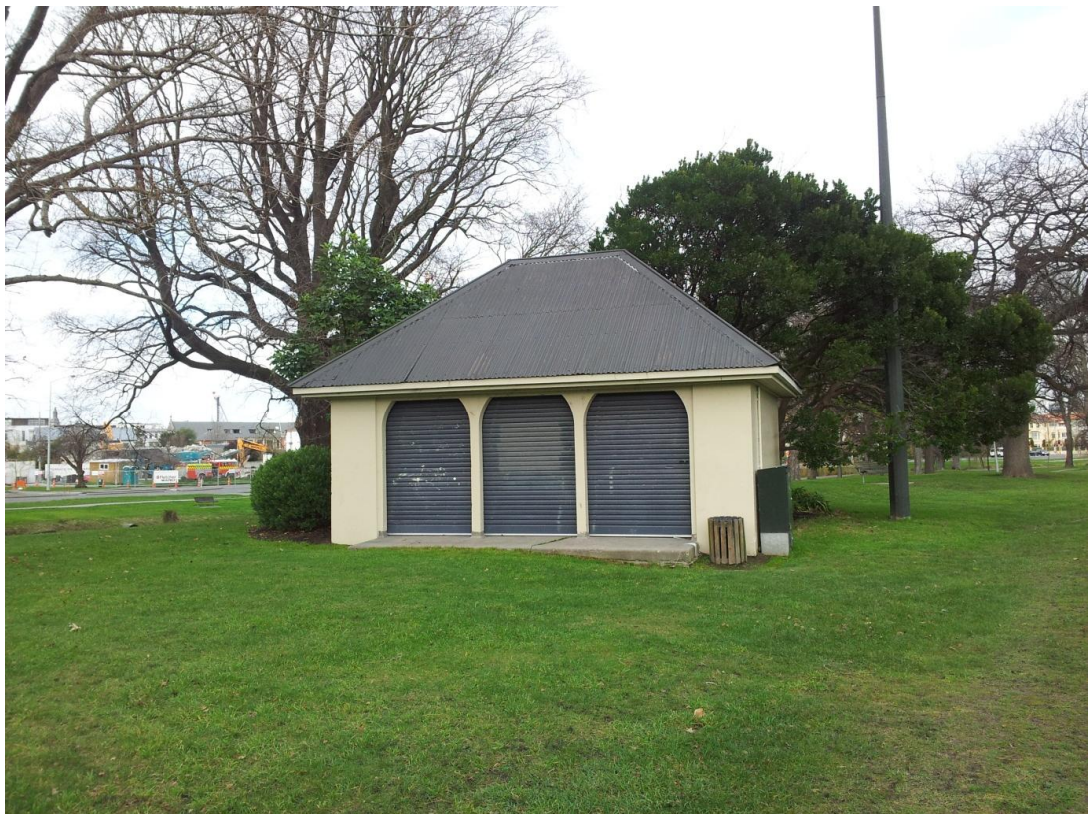
■ Figure 7 Overview of the building (Northern Elevation)
