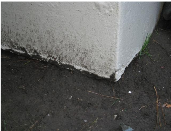
Photo 15: Underside of concrete footing exposed on northwest corner.
