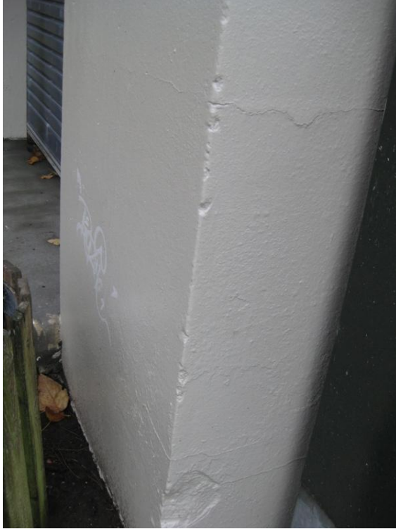
Photo 13: Hairline cracking in concrete wall on northwest corner (typical).
