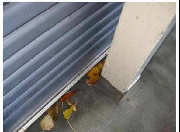
Photo 8: Timber column on north side in front of garage door.
