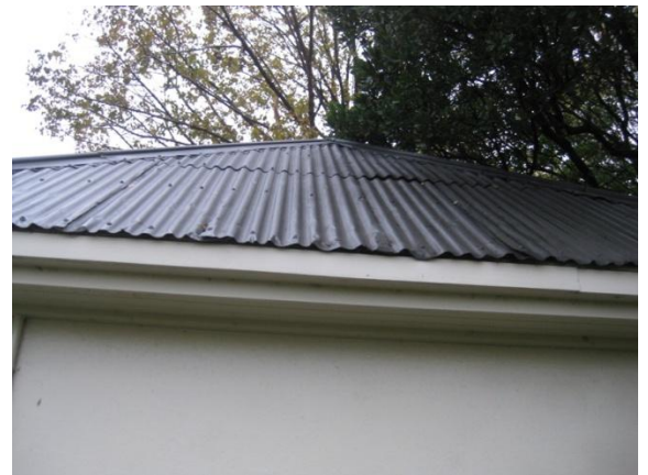
Photo 16: Corrugated metal roof cladding.
