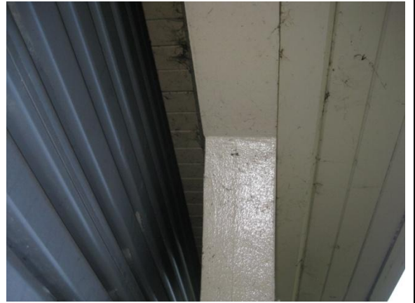
Photo 6: Timber column on north side in front of garage door.
