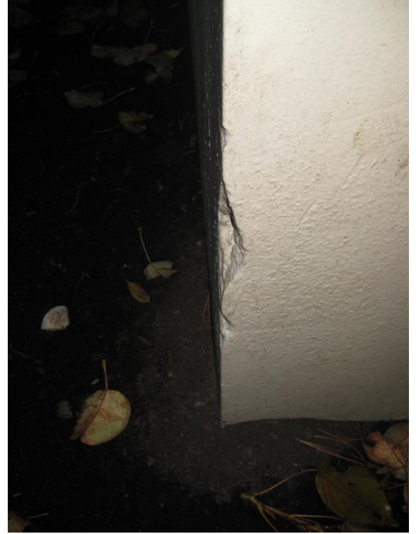
Photo 18: Existing impact damage on southeast corner (typical).
