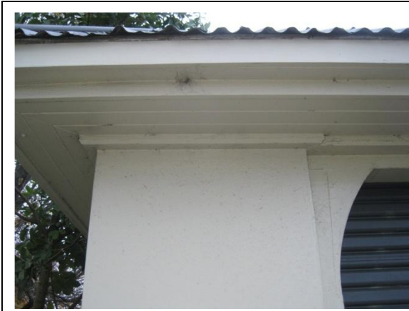
Photo 5: Timber roofing elements on the north side.
