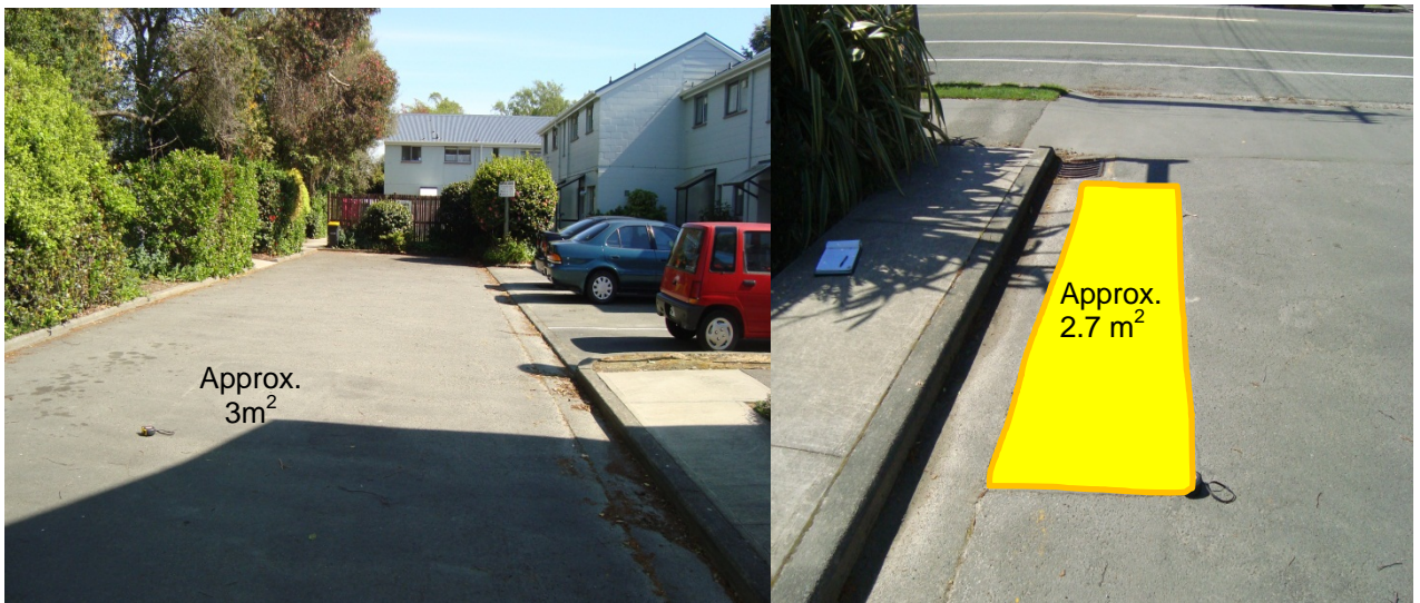
Photograph 10: Repaired liquefaction damaged asphalted ground by the driveway to Hadfield Courts
