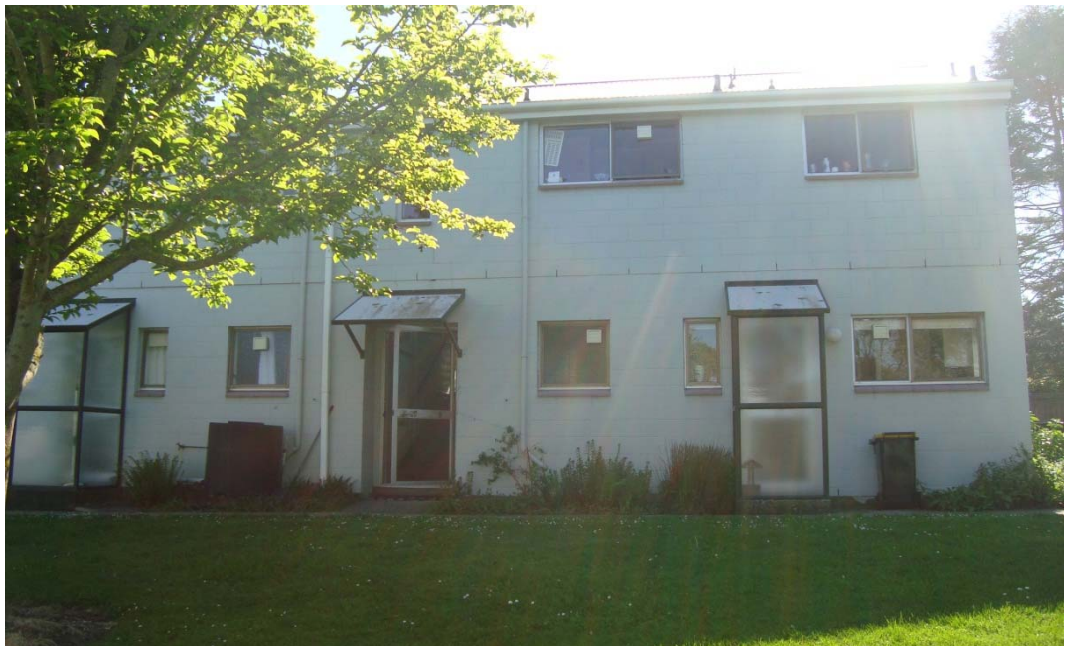
Photograph 8: Rear elevation of Block 4– Unit 17 to 20.
