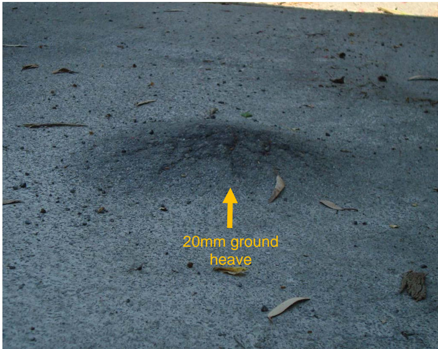
Photograph 16. 20mm ground heave on the asphalted car park in front of Unit 7
