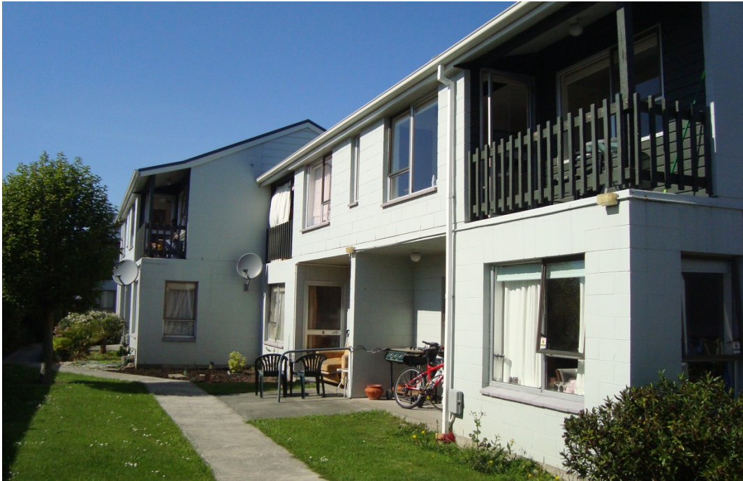
Photograph 5: Front Elevation of Block 2 – Units 5 to 12 with Unit 11 and 12 in the foreground.
