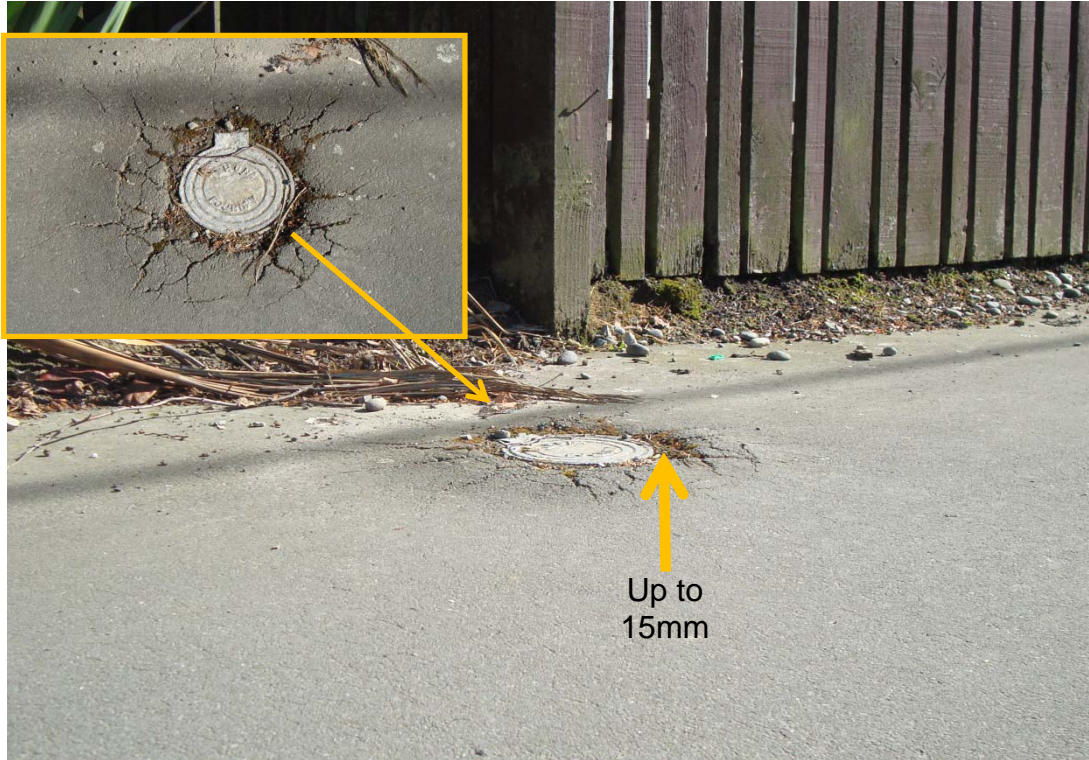
Photograph 11: Up to 15mm lift on the ground around buried services along Somerfield Street by the southern boundary of Hadfield Courts
