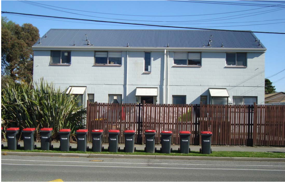
Photograph 1: Rear elevation of Block 1 – Unit 1 to 4
