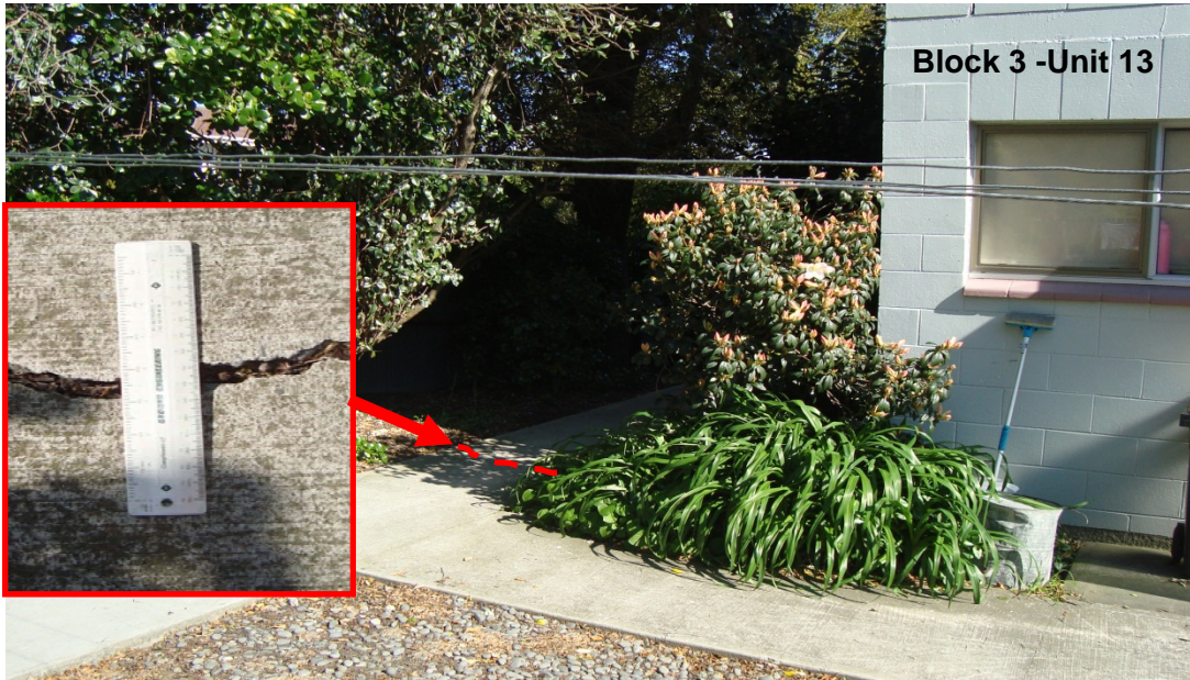
Photograph 17. Up to 15mm wide cracks on the concrete footpath east of Block 3-Unit 13
