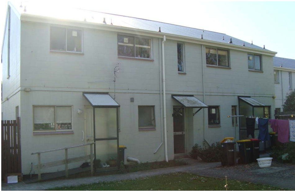
Photograph 3: Rear Elevation of Block 2 – Units 9 to 12.
