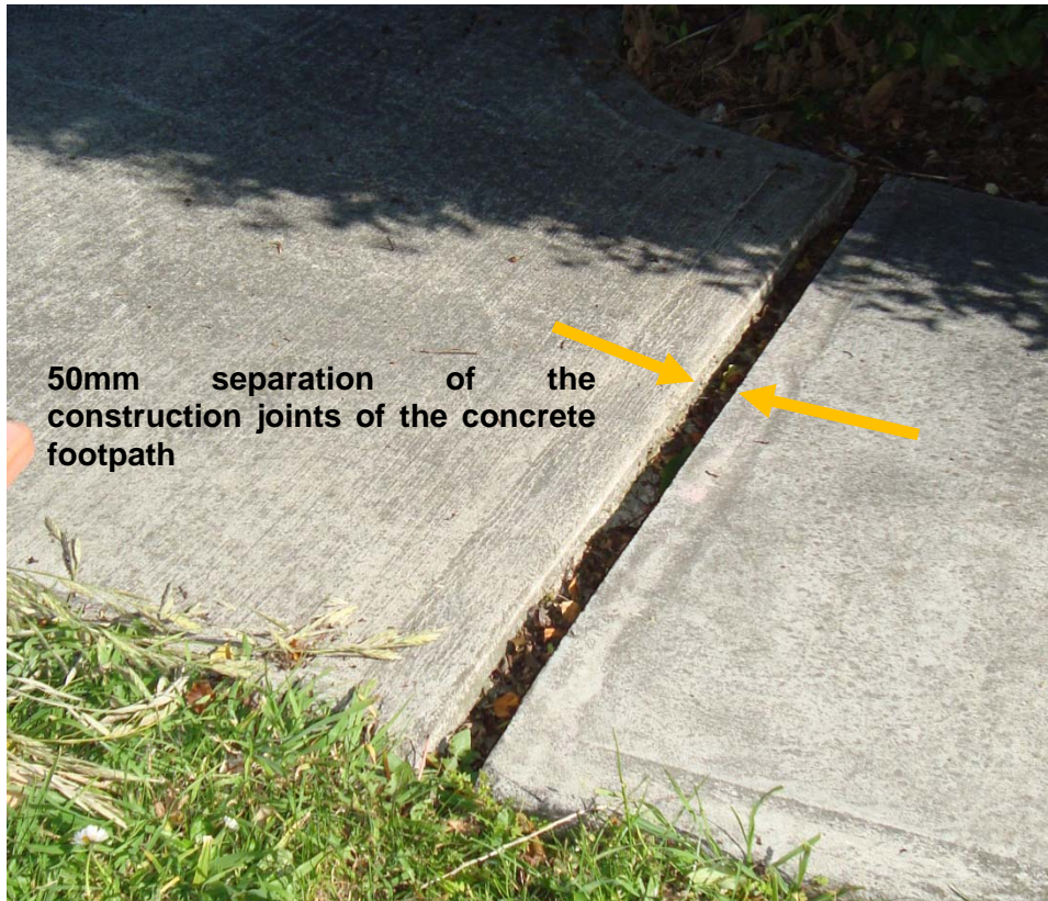
Photograph 17. Up to 15mm wide cracks on the concrete footpath east of Block 3-Unit 13
