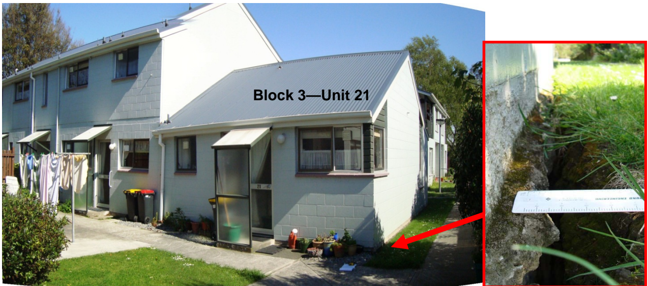
Photograph 6: Rear Elevation of Block 3 – Units 13 to 16, 21 (left photo). Up to 70mm gap between the ground and perimeter foundation at the end elevation of Unit 21 (right photo).
