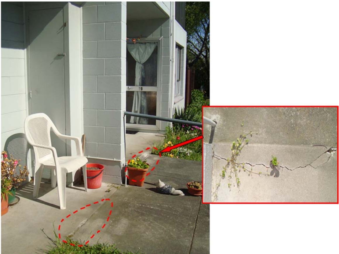
Photograph 20. Up to 10mm wide cracks and differential settlement of less than 10mm on the concrete patio by the lounge door entrance of Block 3 - Units 19 and 17
