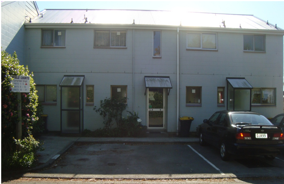
Photograph 4: Rear Elevation of Block 2 – Units 5 to 8
