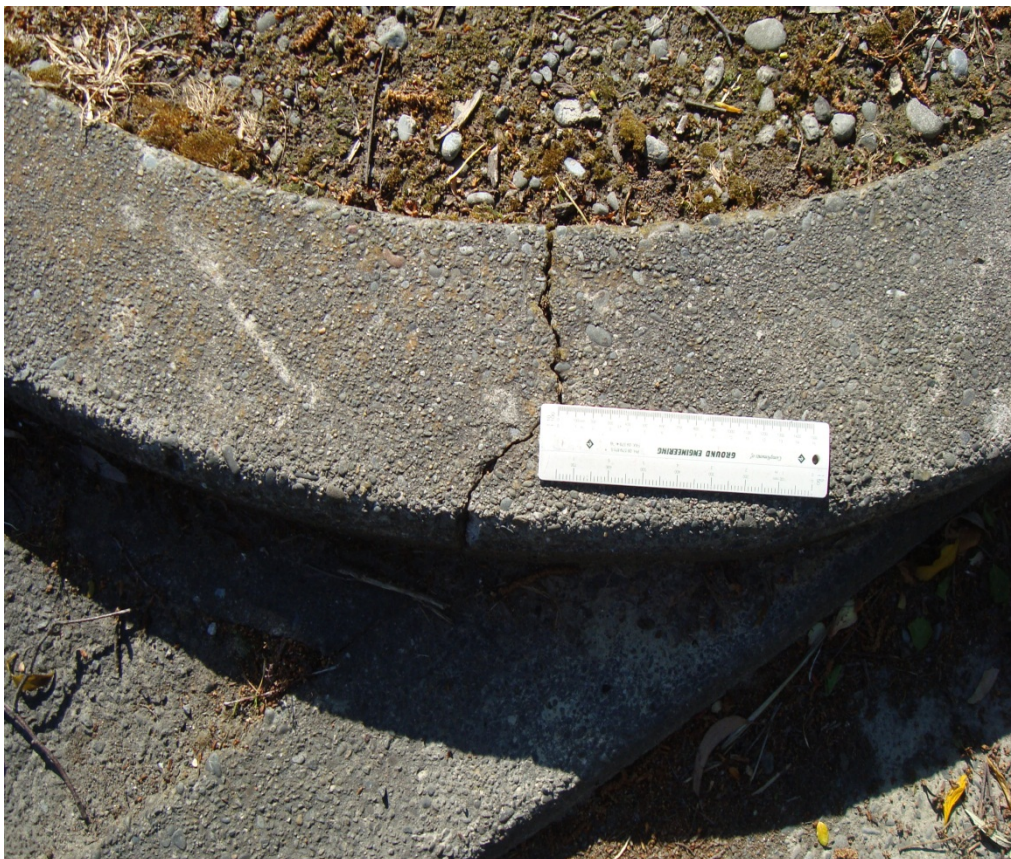
Photograph 14: Up to 4mm wide crack on the concrete kerb in various places within the car park area.
