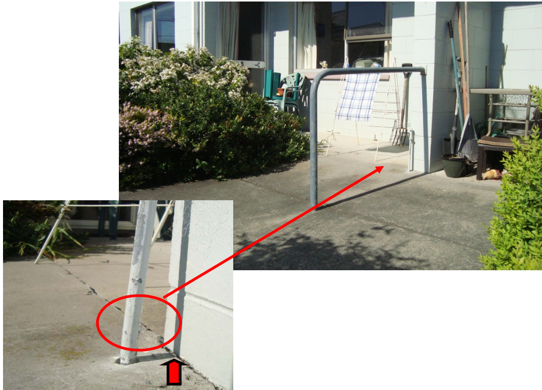
Photograph 21. Concrete slab by the lounge doors of Unit 5 and 7 lifted up to 9mm
