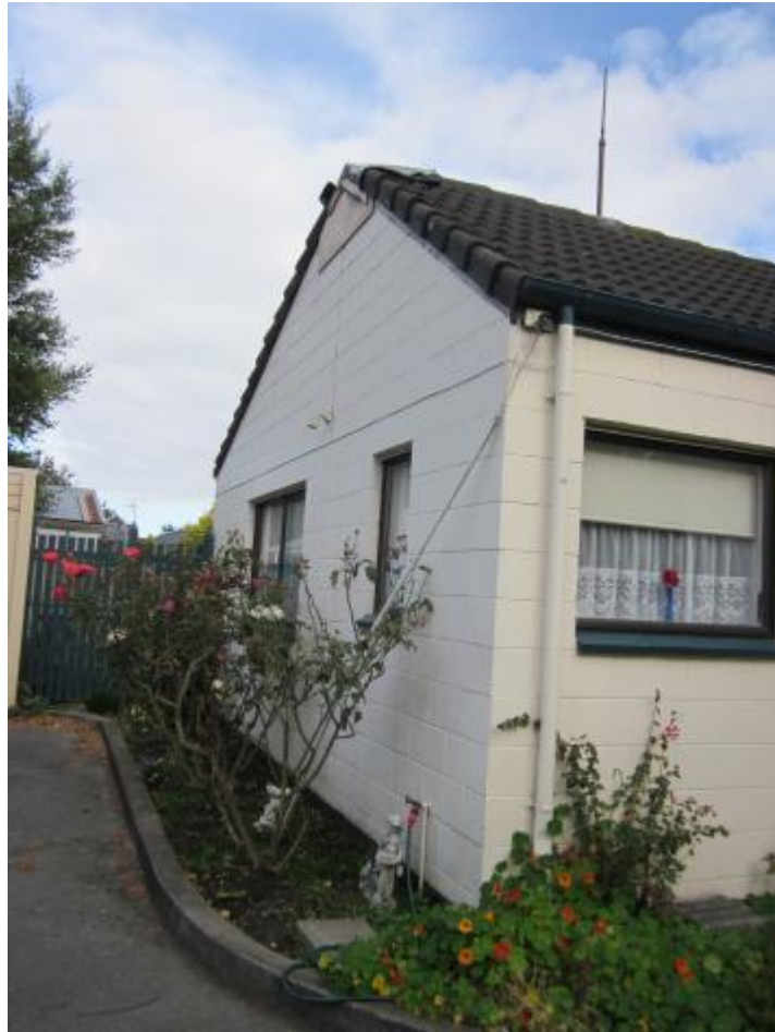
Photo 5 Side View (South of the building).
