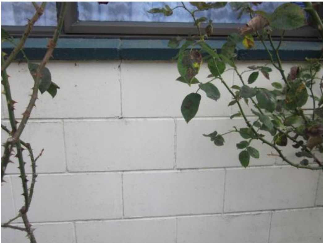
Photo 10 Zigzag cracks at south block masonry wall.
