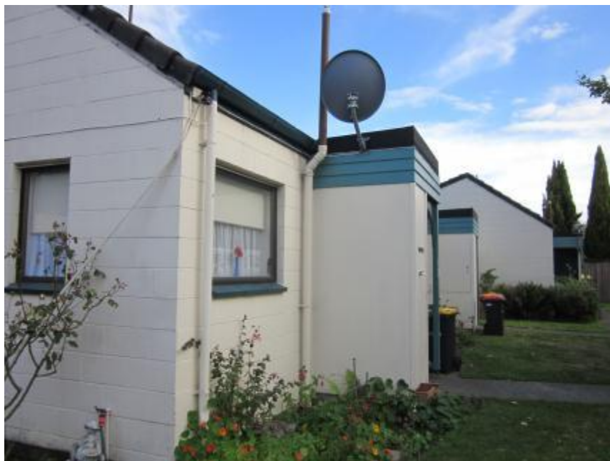
Photo 2 Front View (East of the building).
