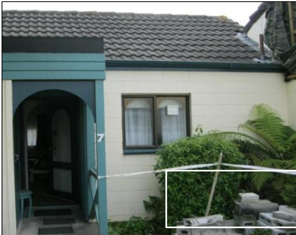
Photo 12 Masonry blocks showing unreinforced gable of Block G, indicative of building style that may have been used in Block H.
