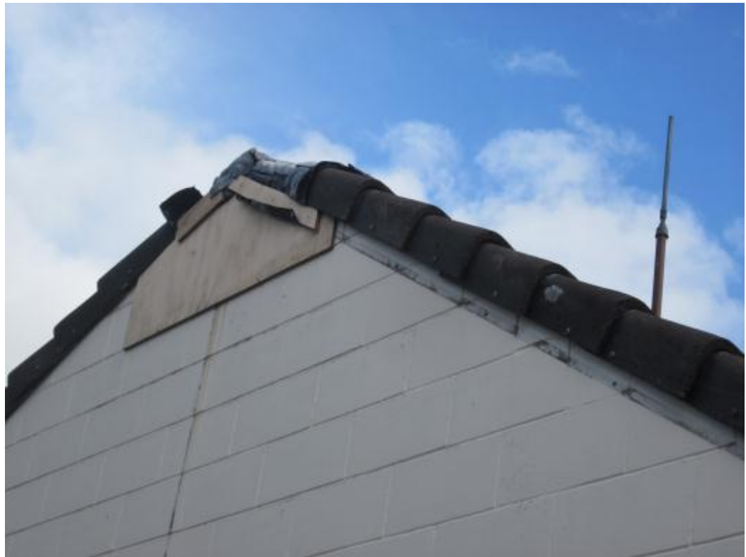
Photo 11 Cracks at apex tip of south gable wall.
