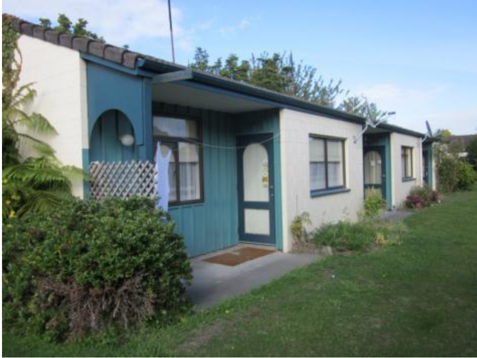
Photo 3 Rear View (North of the building)
