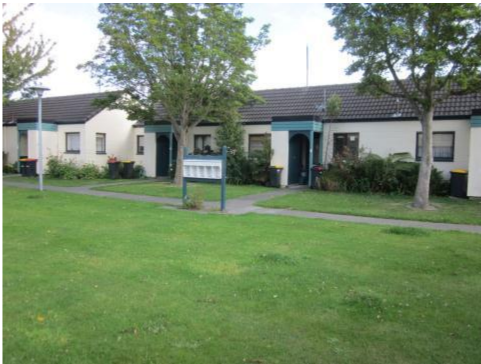
Photo 2 Front View (South of the building)
