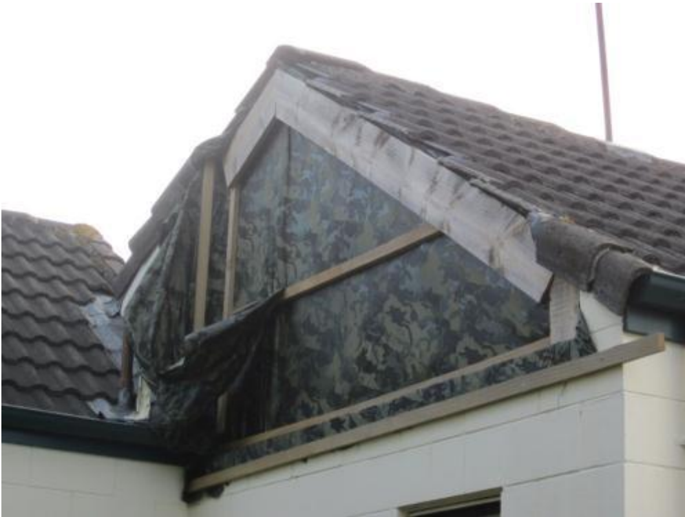
Photo 11 Collapse of west gable wall.
