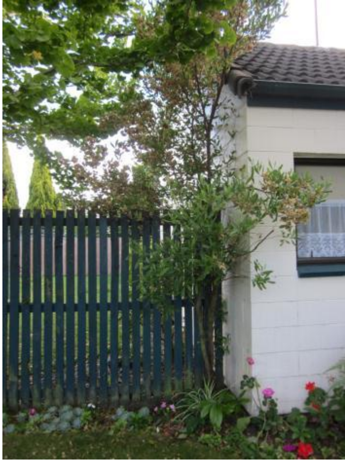
Photo 5 Side View (West of the building)
