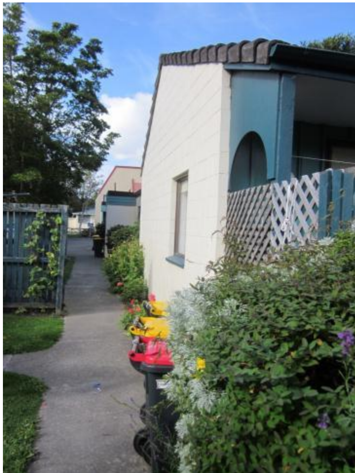
Photo 4 Side View (East of the building)
