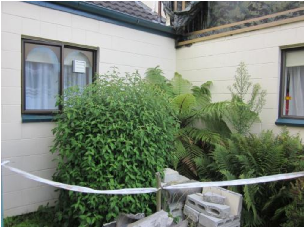
Photo 13 Masonry blocks showing unreinforced gable of Block G. indicative of building style that may have been used.
