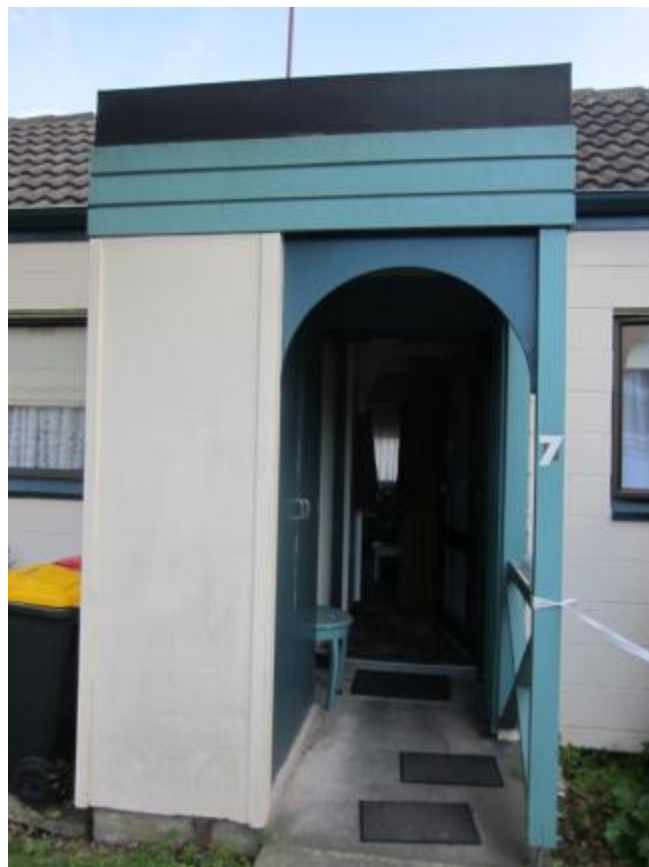
Photo 12 Timber frame porch
