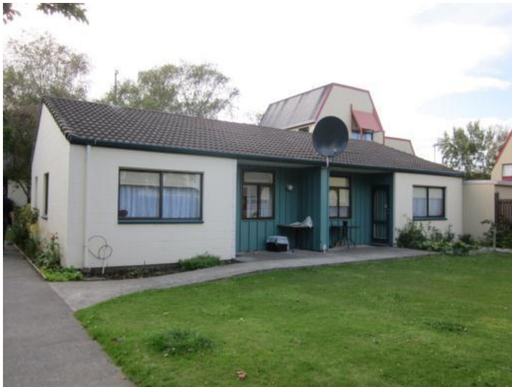
Photo 2 Rear View (West of the building).
