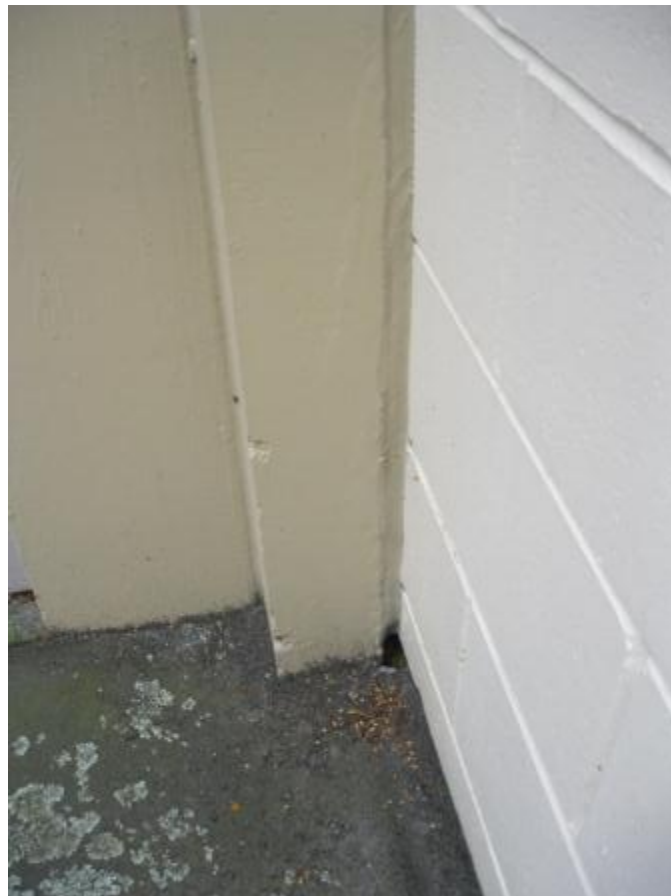
Photo 6 Minimal gap between buildings filled with flexible seal.
