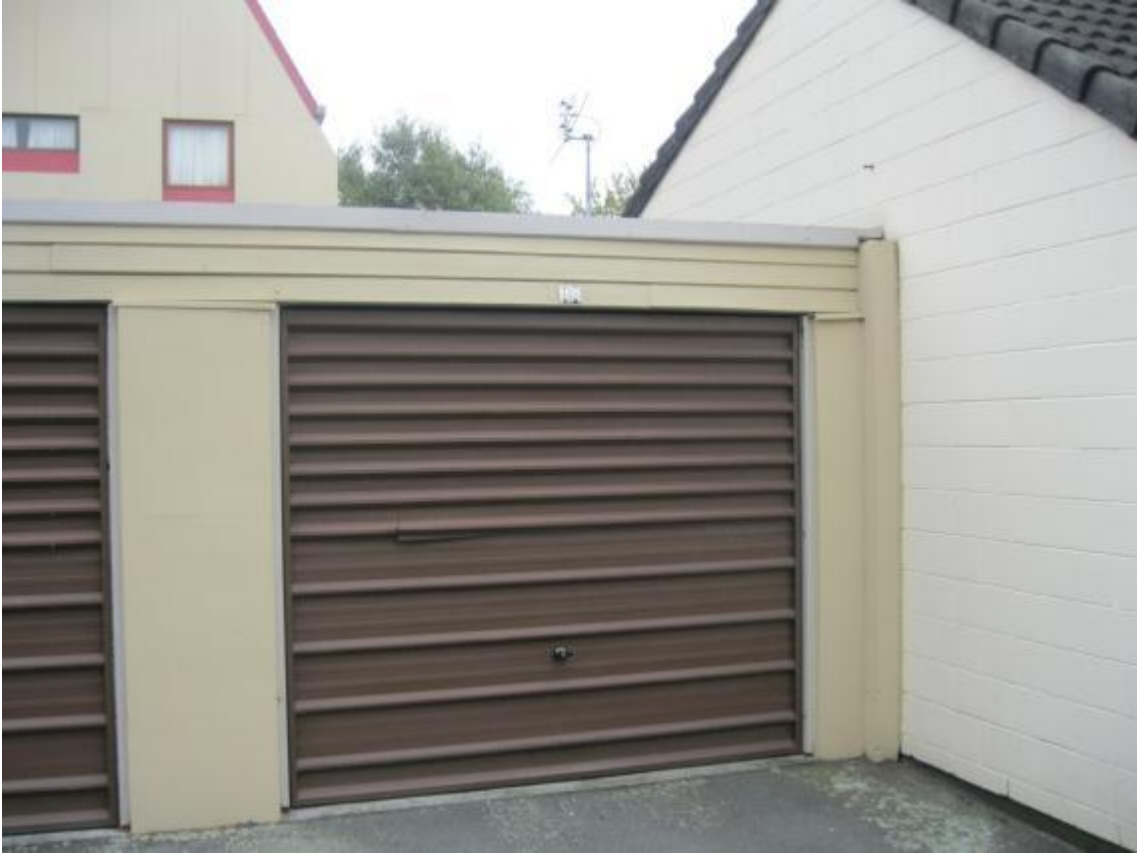
Photo 5 Southern gable of the building adjoining garage Block K.
