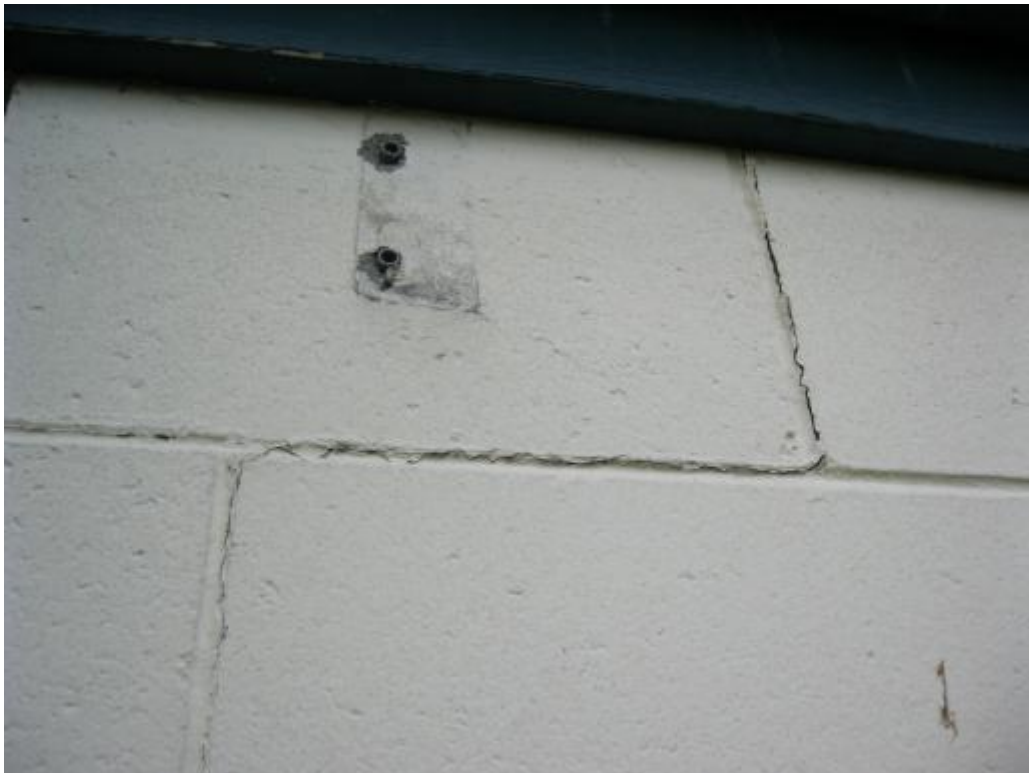
Photo 8 Zigzag cracks at concrete block masonry wall.
