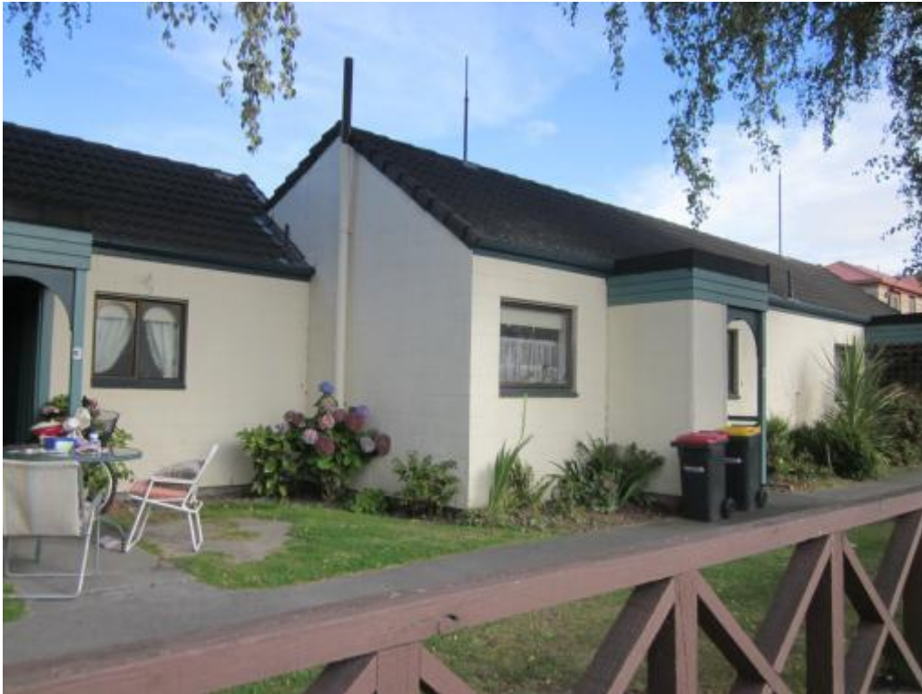
Photo 3 Rear View (East of the building).
