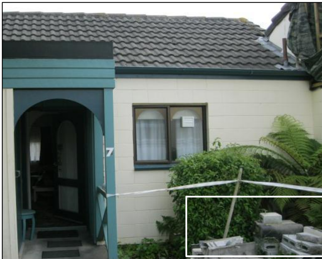
Photo 11 Masonry blocks showing unreinforced gable of Block G, indicative of building style that may have been used in Block E.
