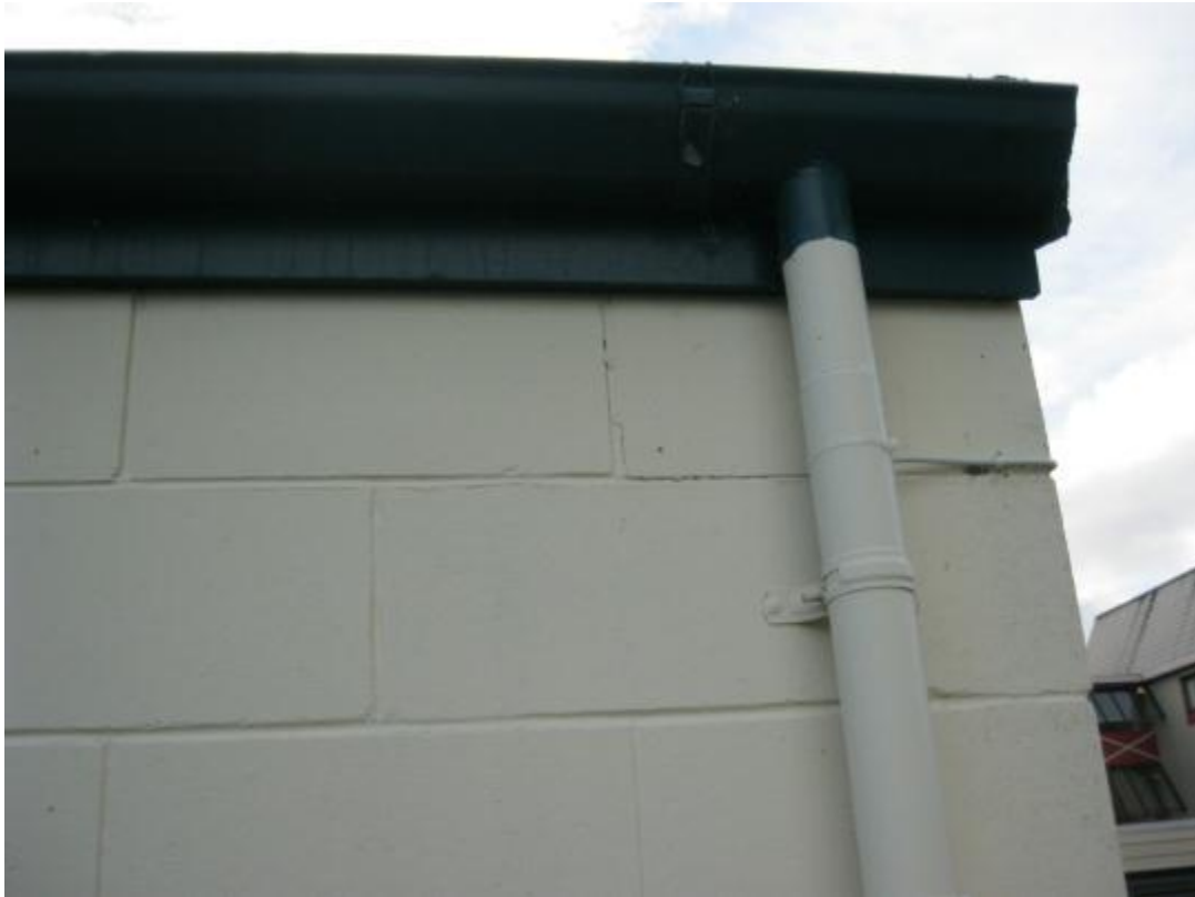
Photo 9 Zigzag cracks at concrete block masonry wall.
