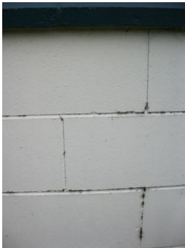
Photo 9 Zigzag cracks at concrete block masonry wall.
