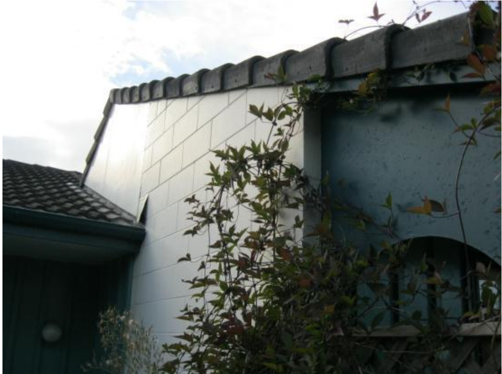
Photo 7 Apex tip of gable wall.
