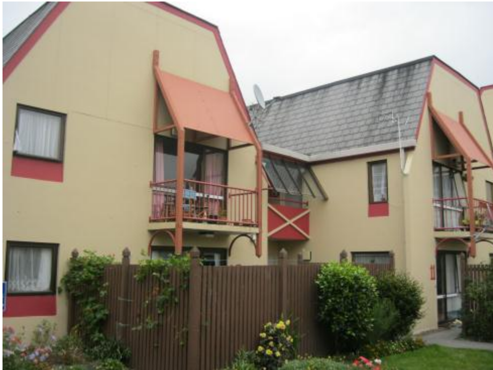
Photograph 1 North elevation of Haast Courts Block C (Units 5-10).
