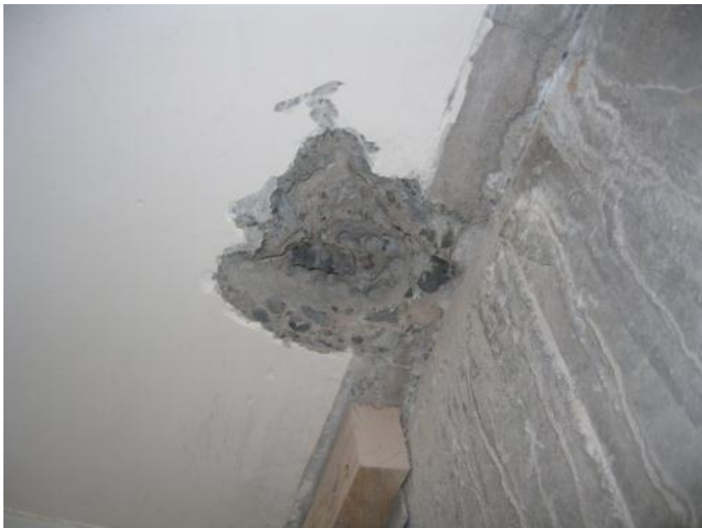
Photograph 22 Opening up to the underside of the second floor suspended slab showed the steel cage reinforcement not tied into the precast wall.
