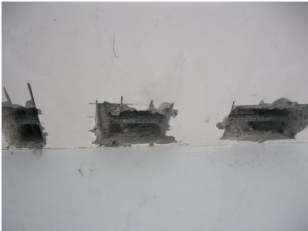
Photograph 24 Further opening up and reinforcement scanning revealed regular spacing of bars tying the slab into the precast panels at 250mm centres along all walls.
