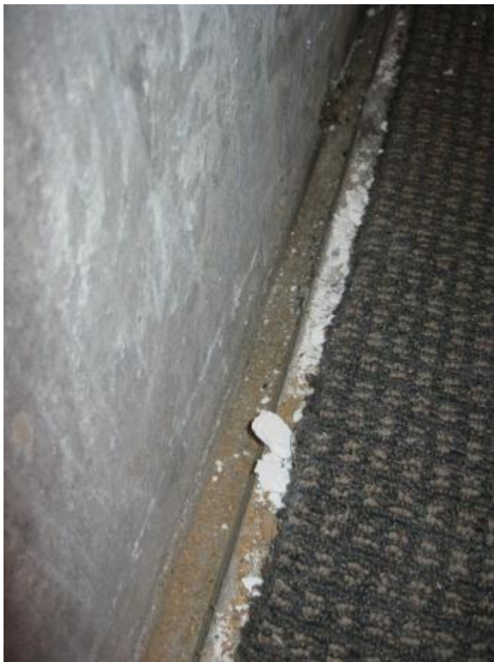
Photograph 14 Connection between cast in situ floor slab and precast panel wall at second floor level.
