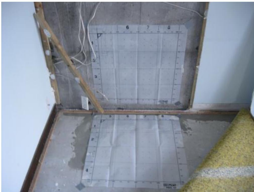
Photograph 18 Scan locations looking for details of connection between the precast panel and the cast in-situ suspended floor slab.
