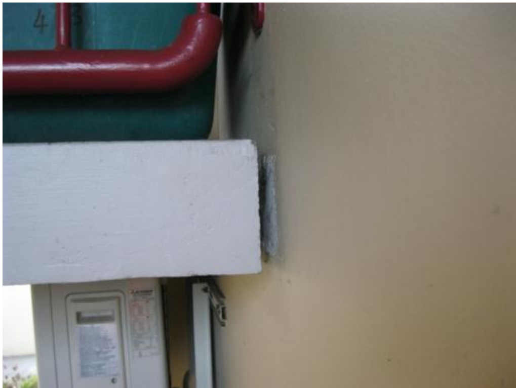
Photograph 7 Seismic gap between stairs landing and precast concrete wall panel.
