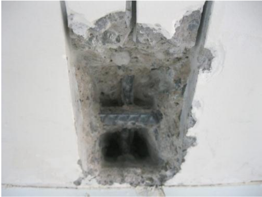
Photograph 23 Opening up in another location revealed a 10mm diameter steel bar tying the suspended slab back into the precast concrete wall panels.
