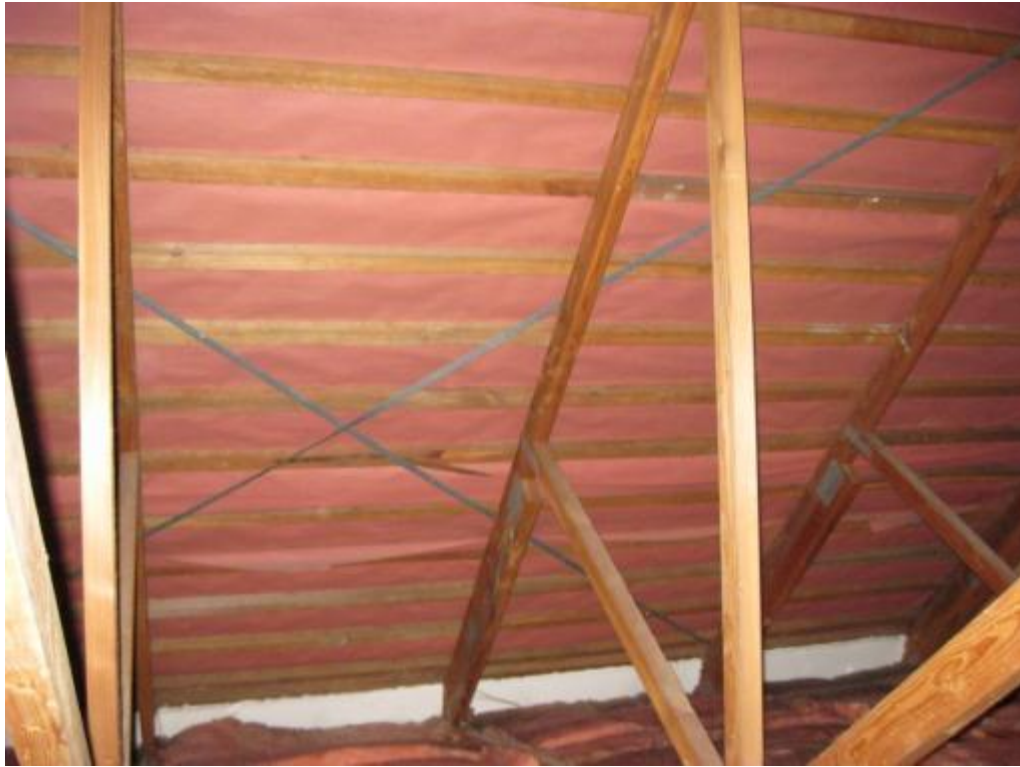
Photograph 11 Flat steel strap roof cross bracing.
