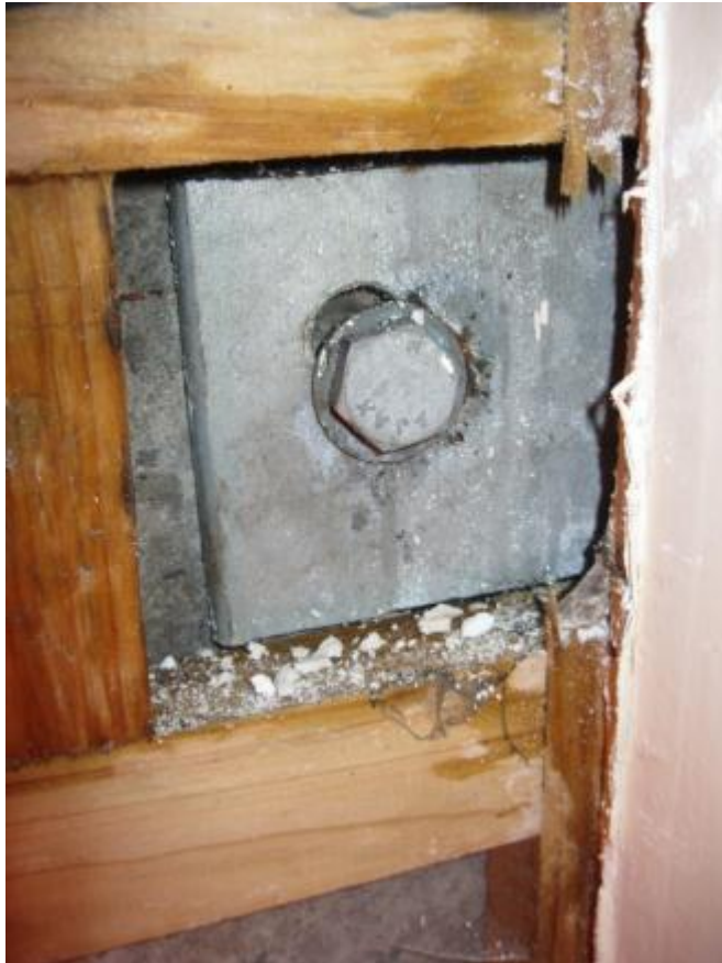
Photograph 15 Angle cleat connection between precast wall panels at second floor.
