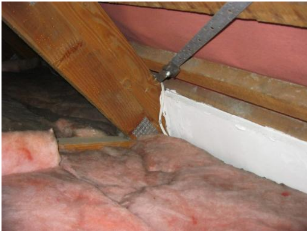
Photograph 11 Flat steel strap roof cross bracing.
