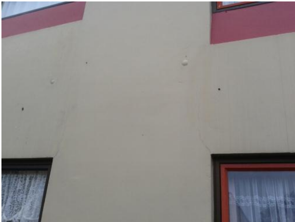
Photograph 2 Cracking to exterior walls at window corners.
