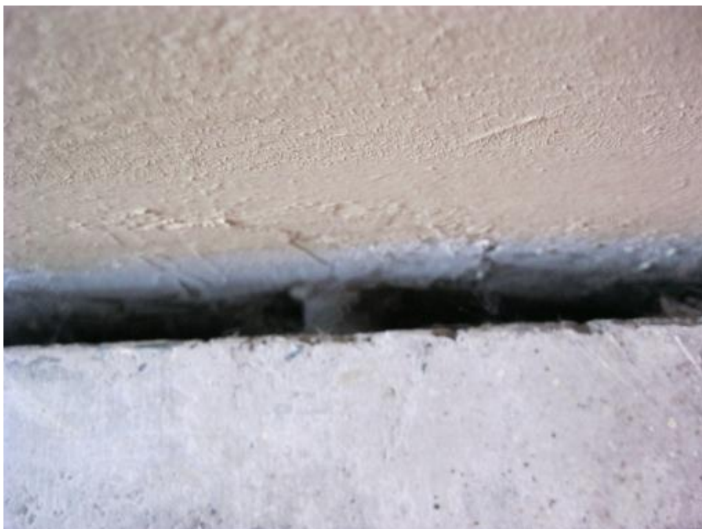
Photograph 7 Seismic gap between stairs landing and precast concrete wall panel.
