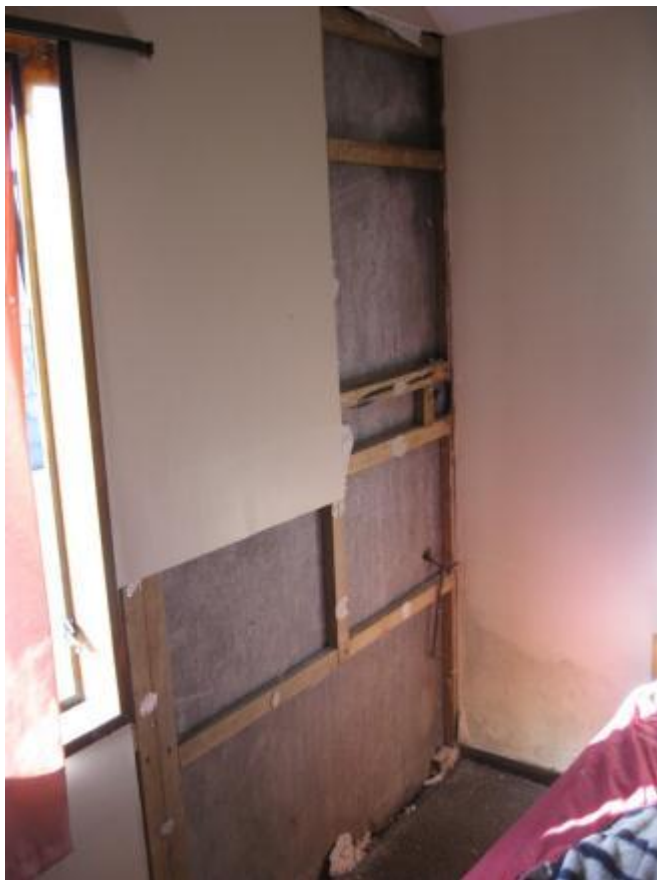
Photograph 16 Wall linings removed to expose angle cleat connection and precast concrete panel at second floor level.
