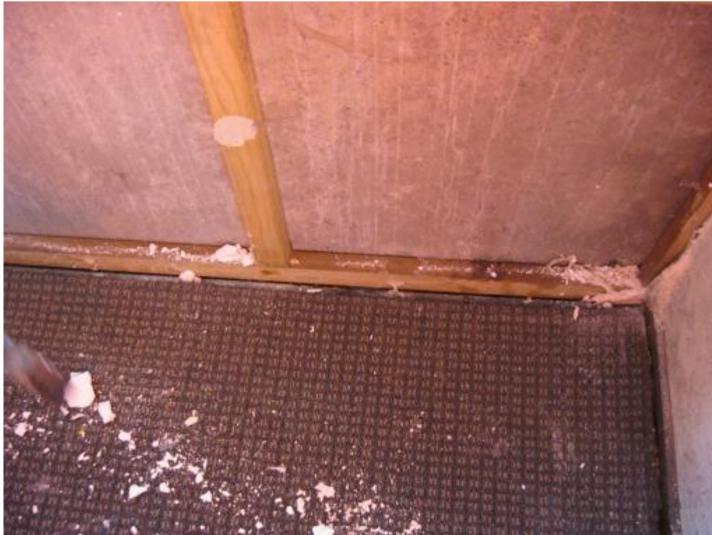
Photograph 13 Removal of wall linings to expose concrete panel wall to allow scanning for reinforcement details at second floor level.
