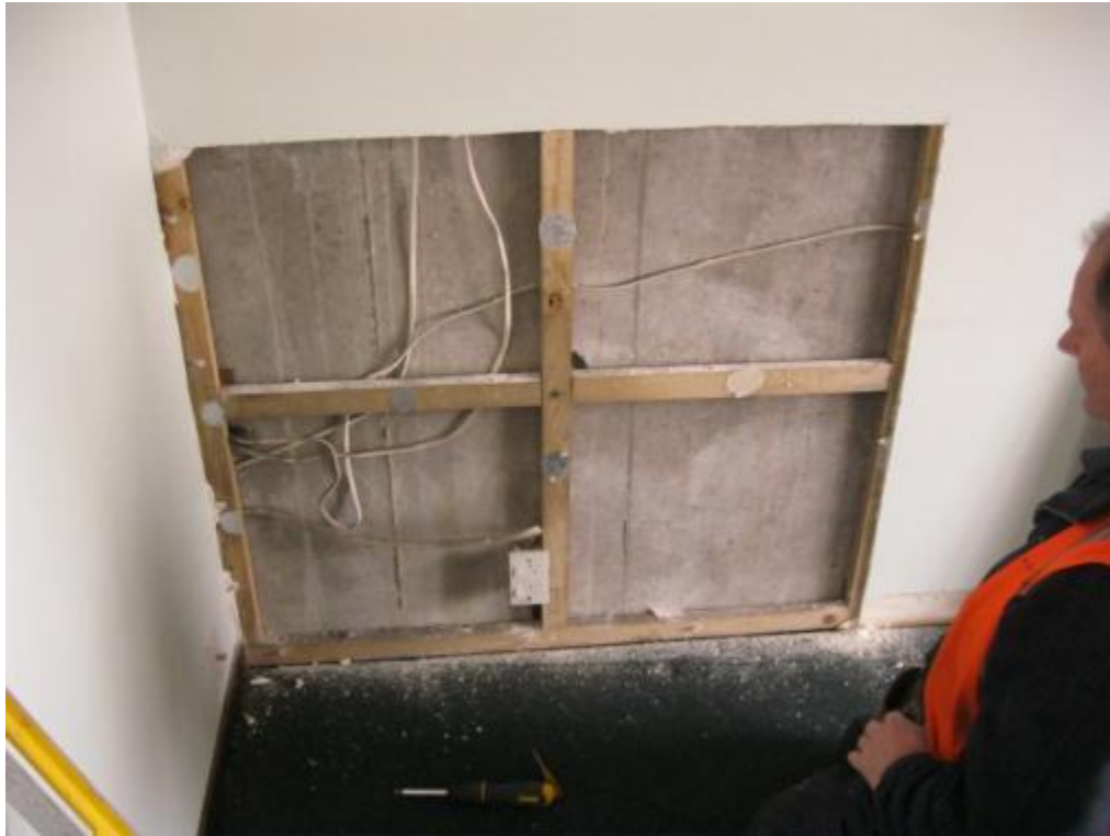
Photograph 17 Removal of wall linings in first floor apartment to expose precast concrete wall panel to scan for reinforcement.
