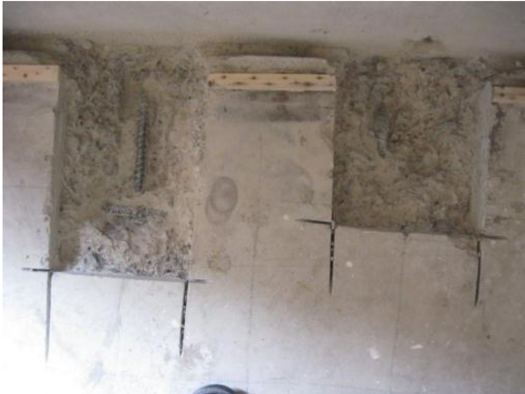
Photograph 21 Further opening up of the suspended slab showed the steel reinforcement cage not to be tied into precast wall from the top.
