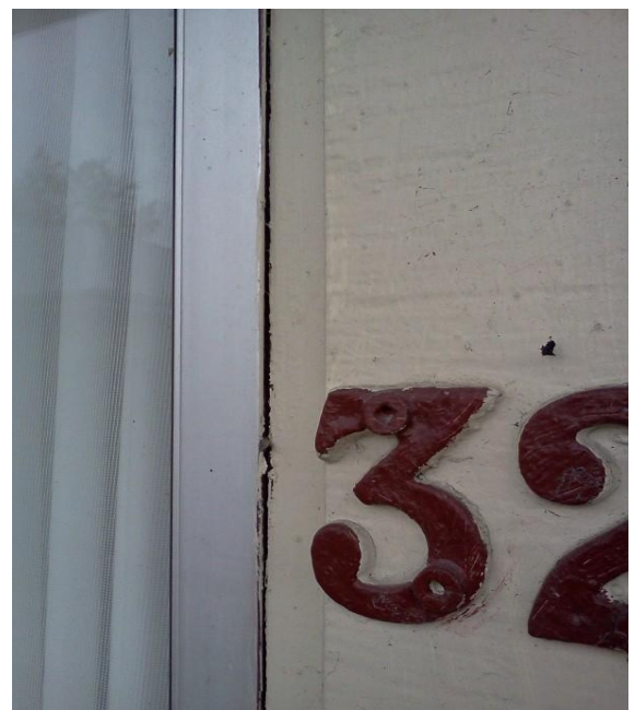
Photo 6: Gap opening up between window frame and timber wall on the north wall of Unit 32 (typical).
