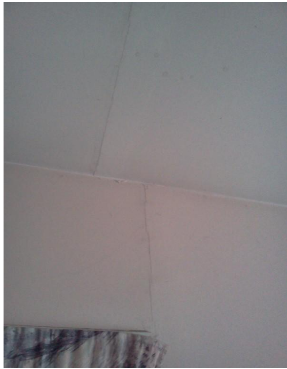
Photo 9: Cracks in internal wall and ceiling lining.
