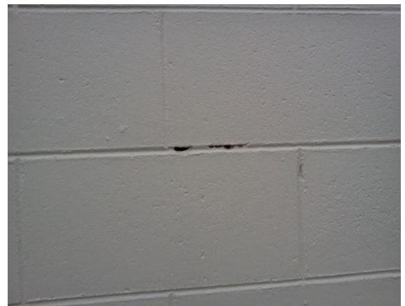
Photo 12: Existing low quality pointing of masonry on East wall.
