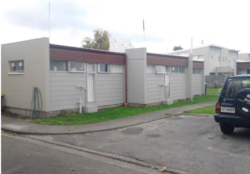
■ Figure 7 Overview of the block units on site
