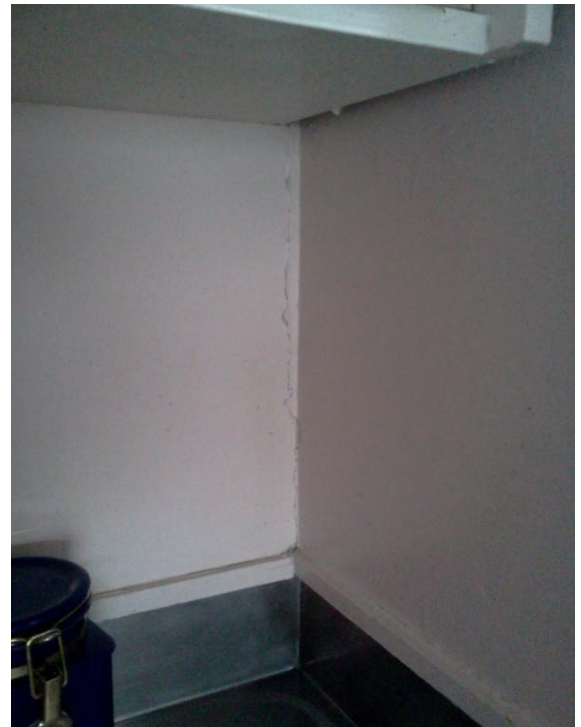
Photo 10: Cracks in wall lining and paint tearing at corners.
