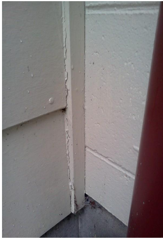
Photo 13: Cracks in external timber wall on south side in corners.
