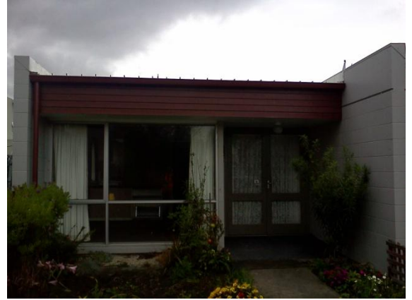
Photo 2: Front elevation of a typical unit with masonry walls either side and light timber framed internal structure
