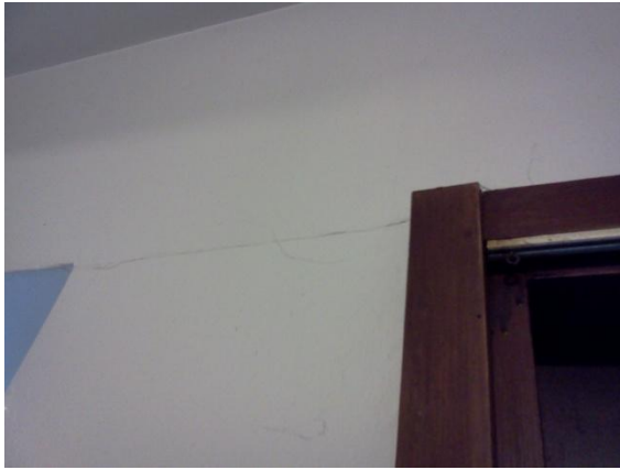
Photo 13: Horizontal cracking between wall penetrations
