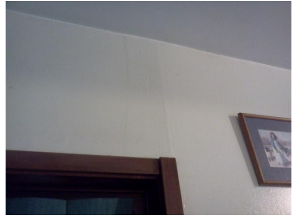
Photo 14: Vertical separation between plaster boards
