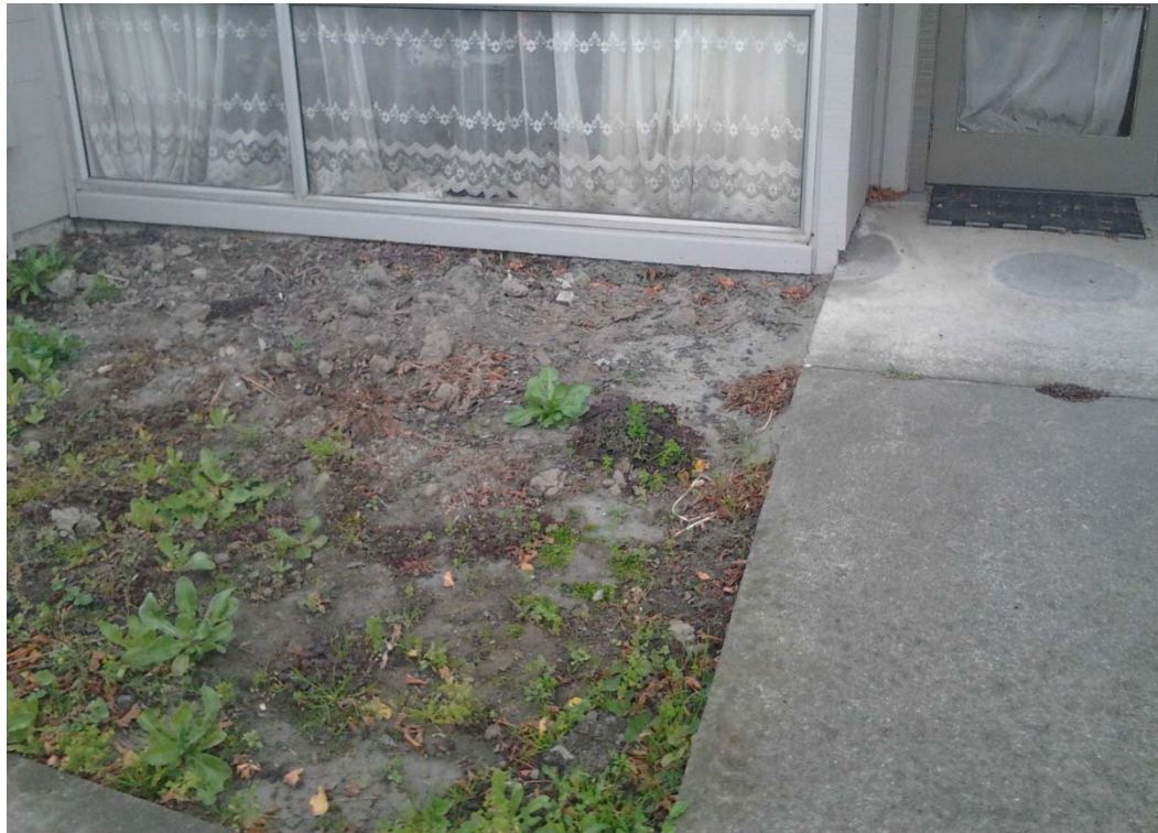
■ Figure 10 Remaining evidence of liquefied material ejecta
