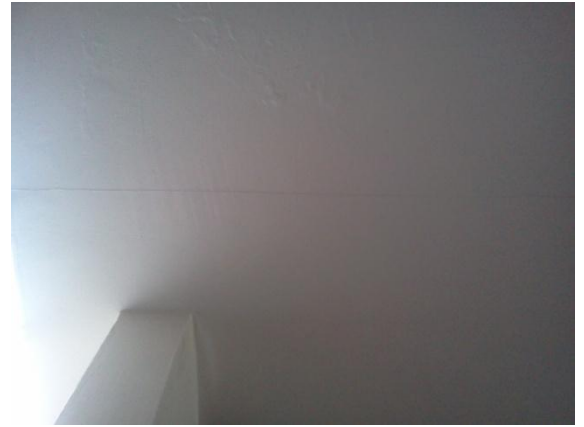
Photo 10: Separation along the plasterboard sheet joint
