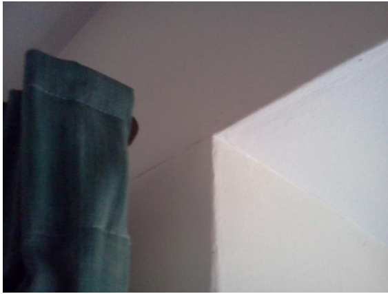
Photo 9: Horizontal cracking through the plasterboards
