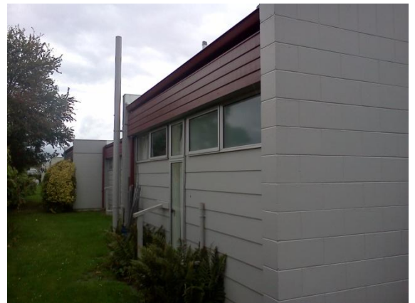
Photo 4: Rear of the buildings are light timber framed and weatherboard clad
