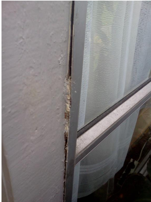
Photo 7: Separation along the window framing which appears pre existing
