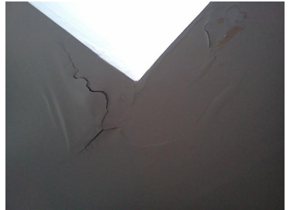
Photo 12: Damage to the ceiling lining around the base of the skylight due to moisture
