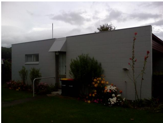
Photo 3: Side elevation of an end unit
