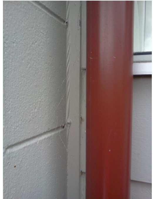
Photo 6: Paint distress along the light timber frame and masonry wall junction
