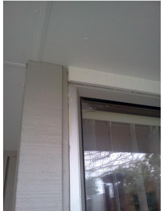
Photo 8: Minor gap opening around the aluminium window framing
