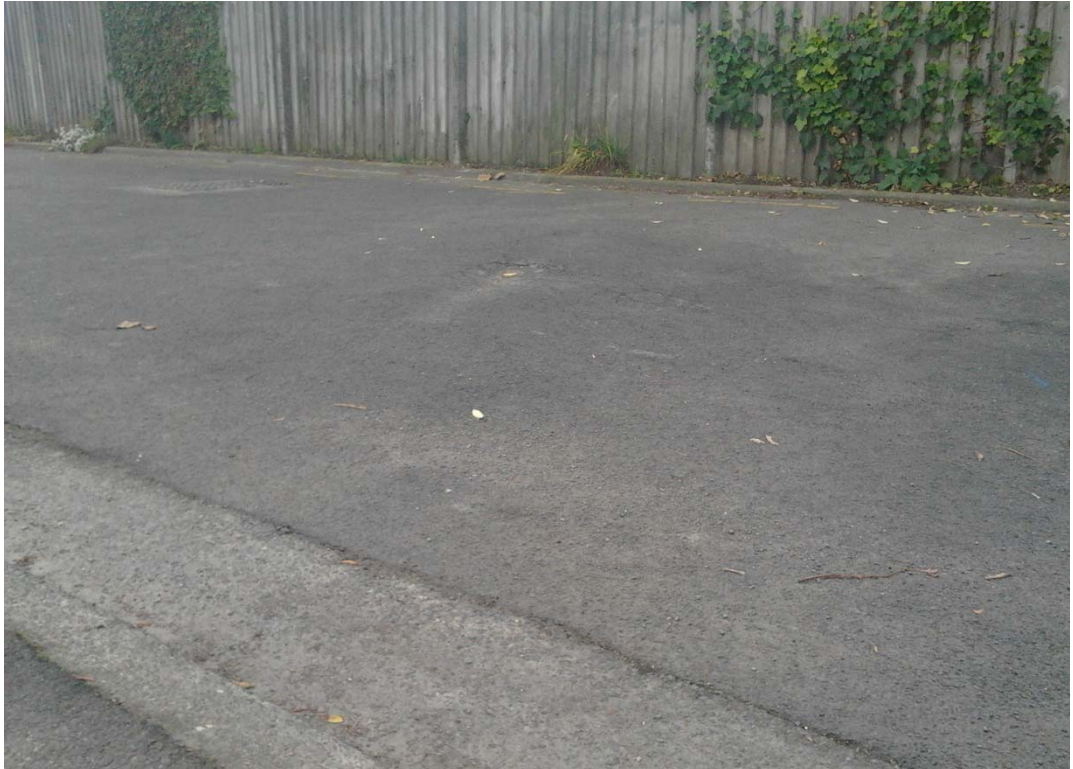
■ Figure 8 Observed undulations on driveways
