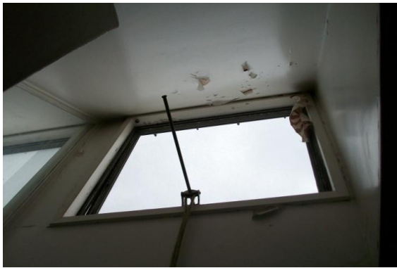
Photo 5: Moisture damage to the paint in the skylight
