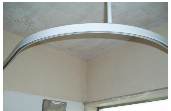
Photo 10: water damage and wall ceiling junction lining separation
