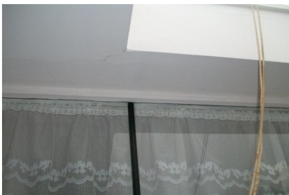
Photo 9: Separation between wall and ceiling linings
