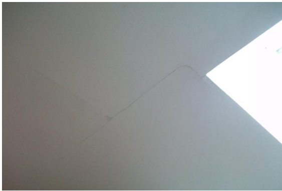
Photo 7: Separation along the
