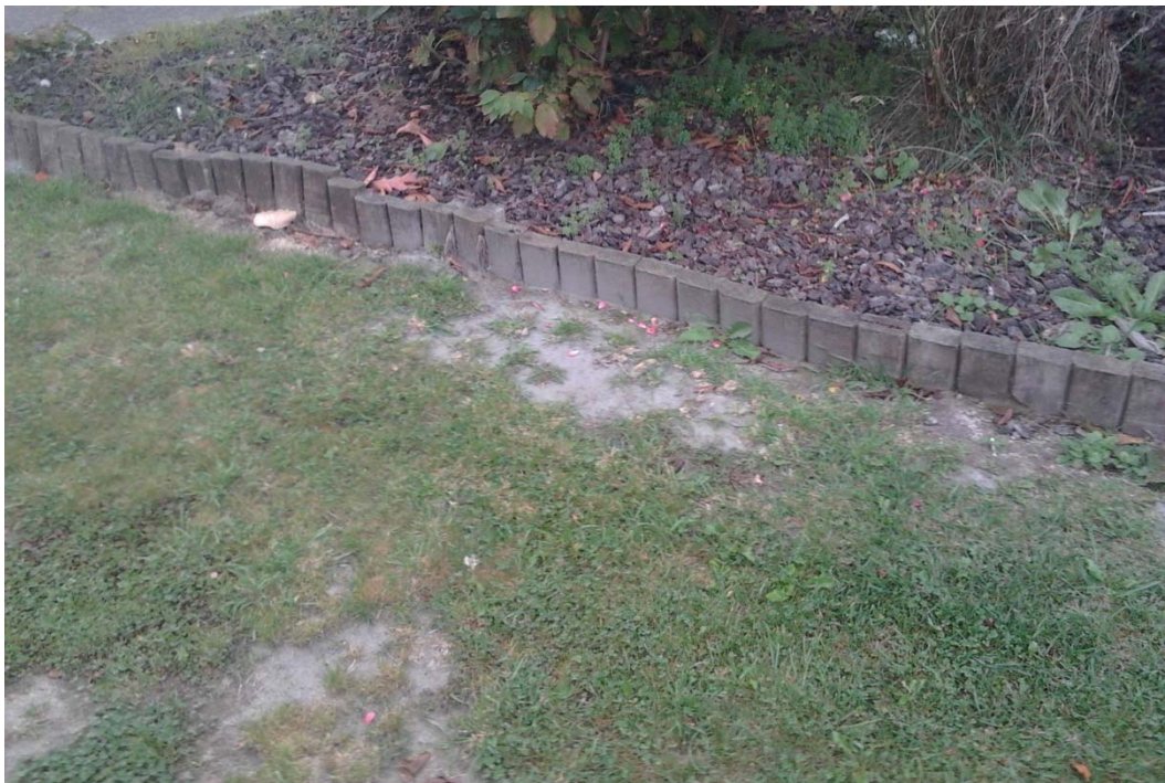
■ Figure 9 Remaining evidence of liquefied material ejecta
